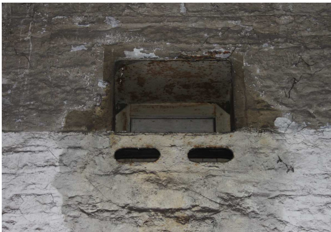
Plate 20: Bearing box with stone surround set in the wall of the preparation block
