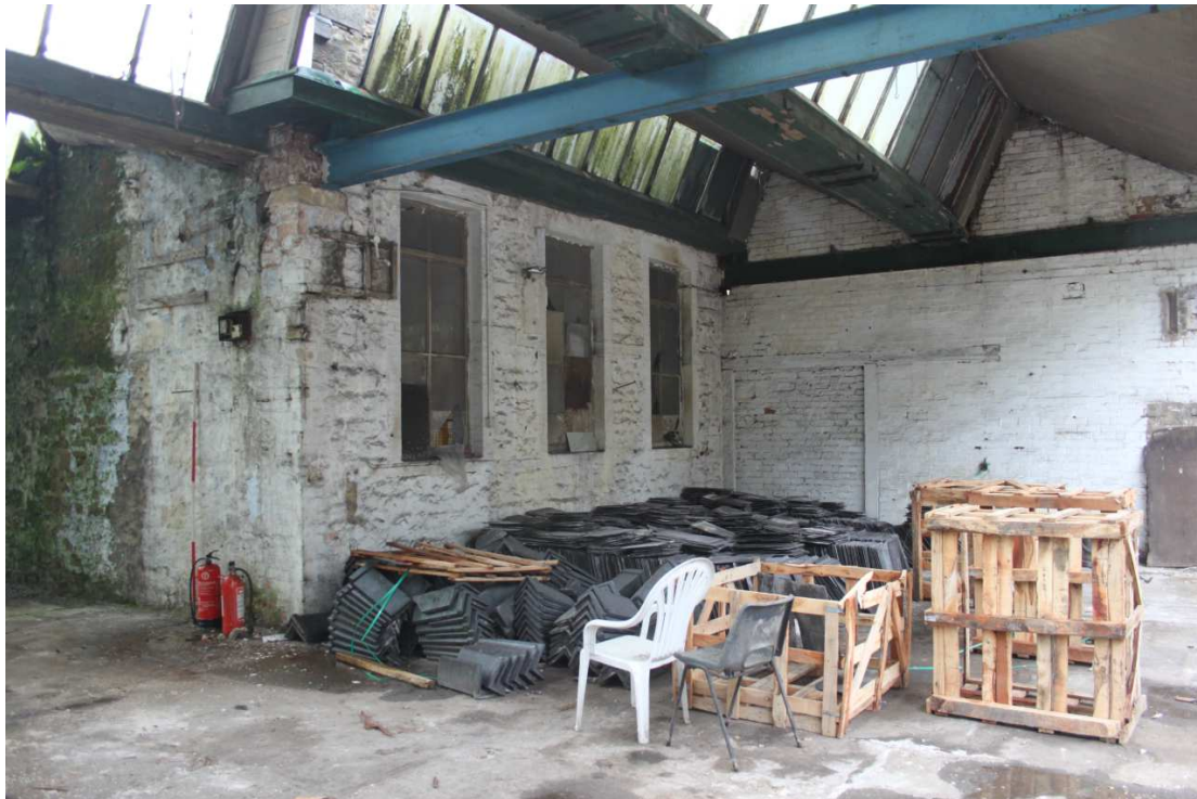
Plate 17: Northern bays of the weaving shed
