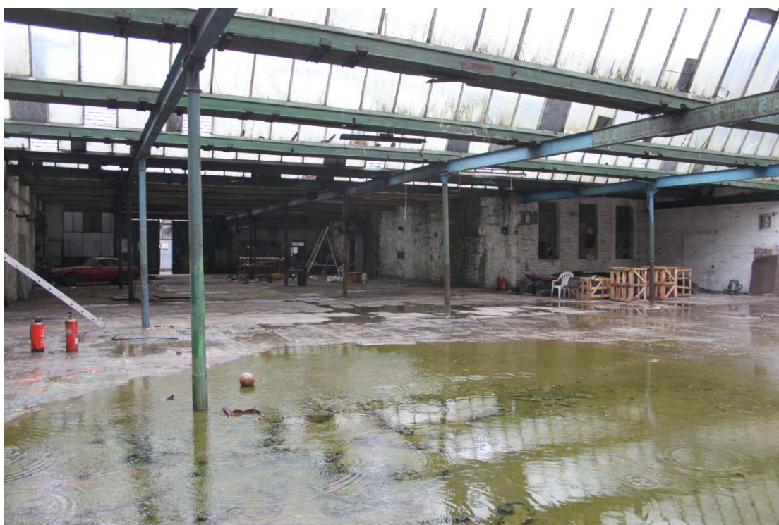
Plate 25: The roof of the c 1910 weaving shed, showing T-section cast-iron glazing bars
