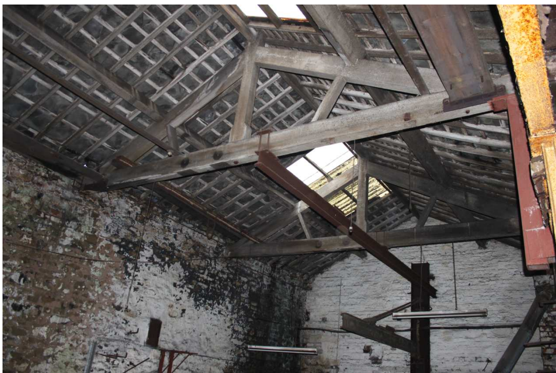
Plate 22: Roof structure in the warehouse
