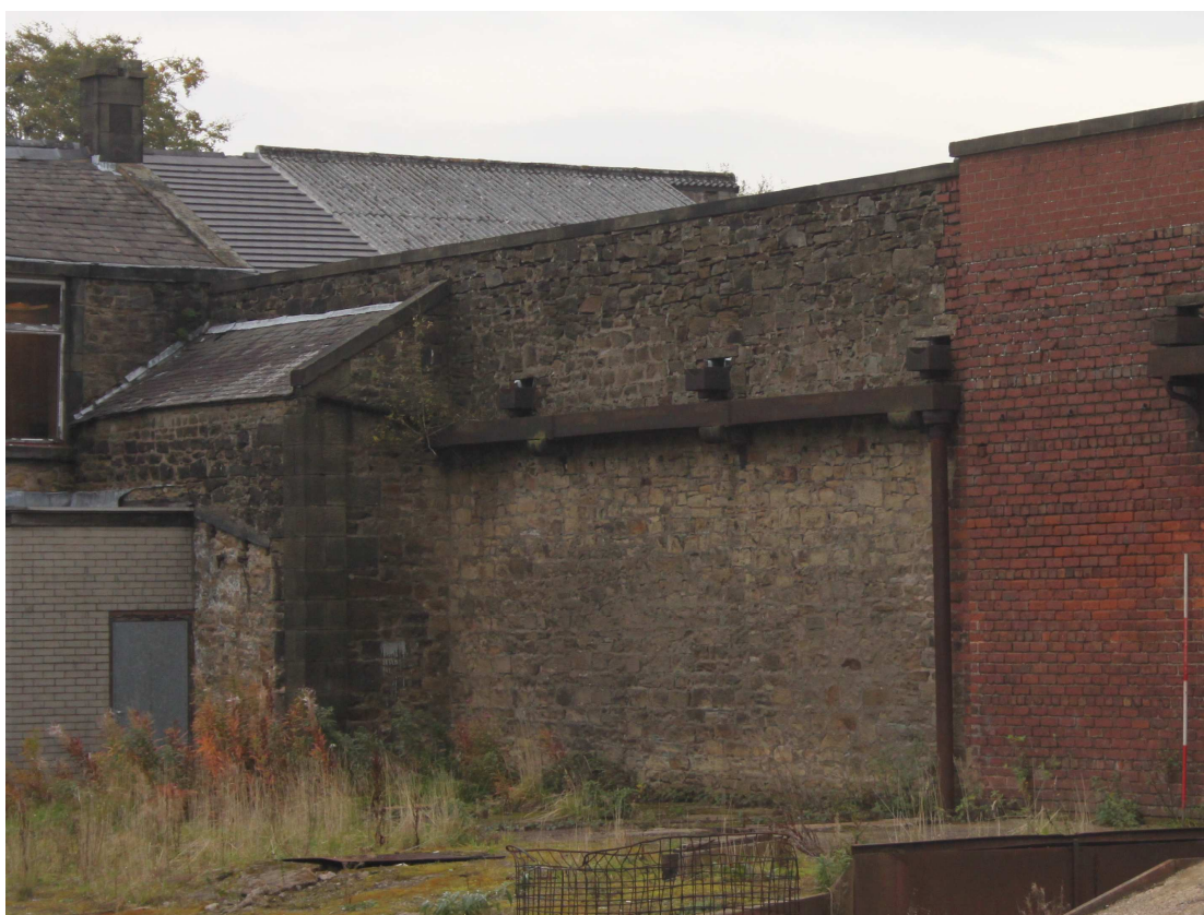
Plate 10: The stone-built section of the weaving shed, with the lean-to structure at its northern end
