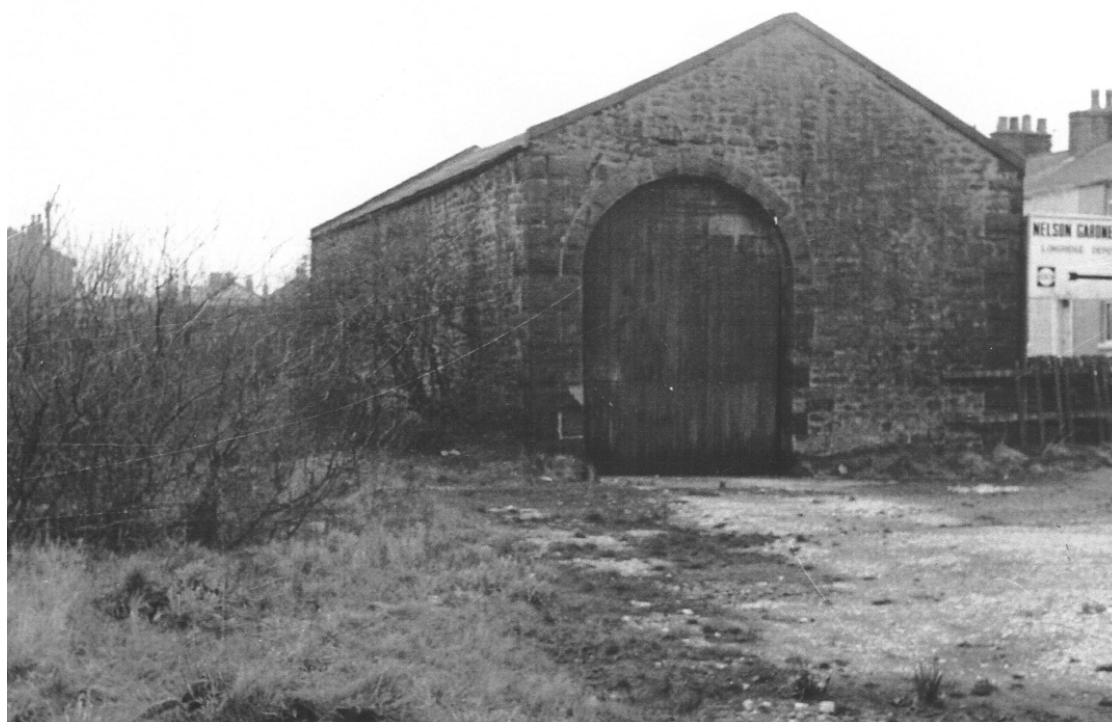
Plate 3: George Whittle's warehouse adjacent to the railway siding on the western side of Silver Street
