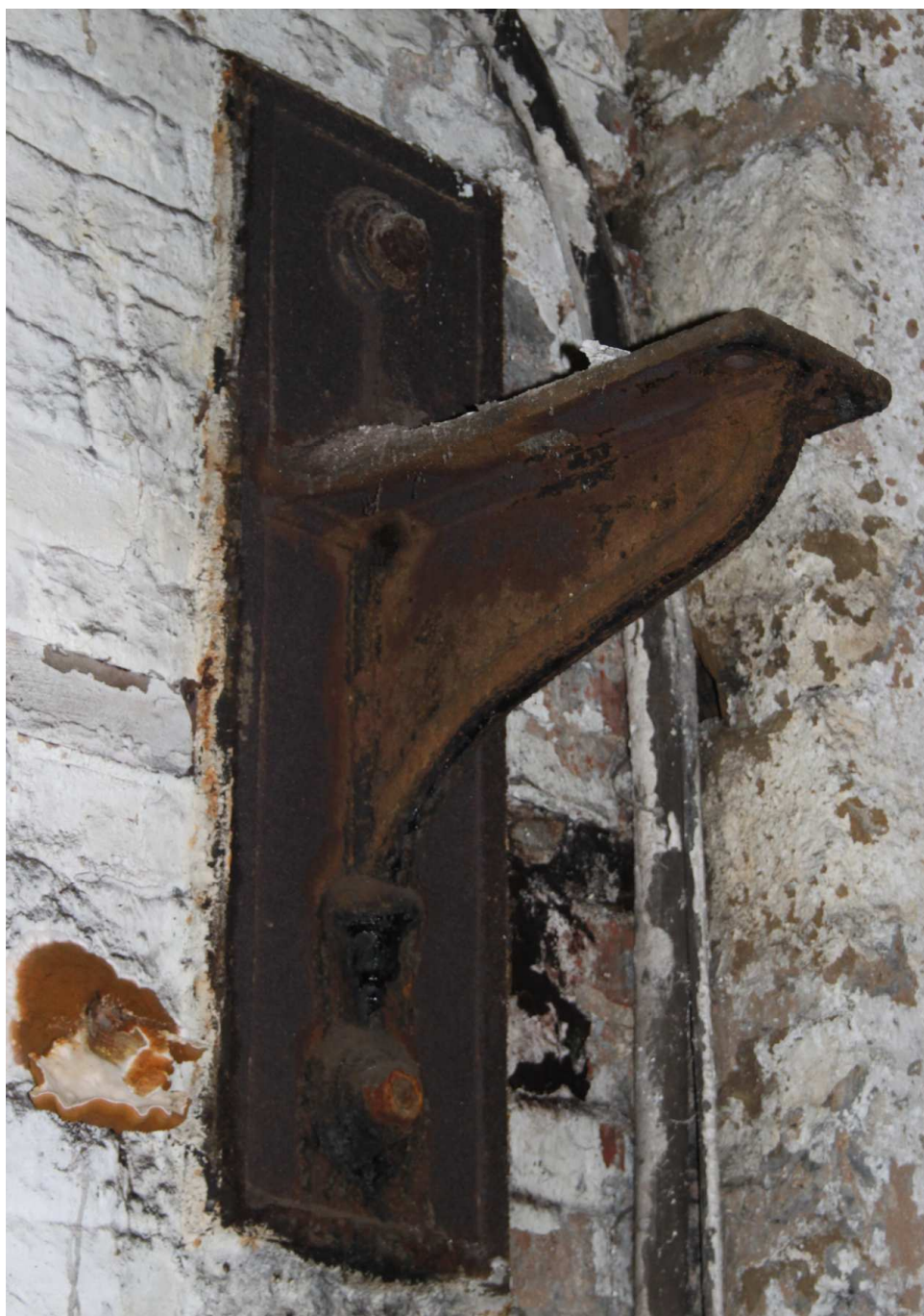
Plate 21: Corbelled cast-iron hanger
