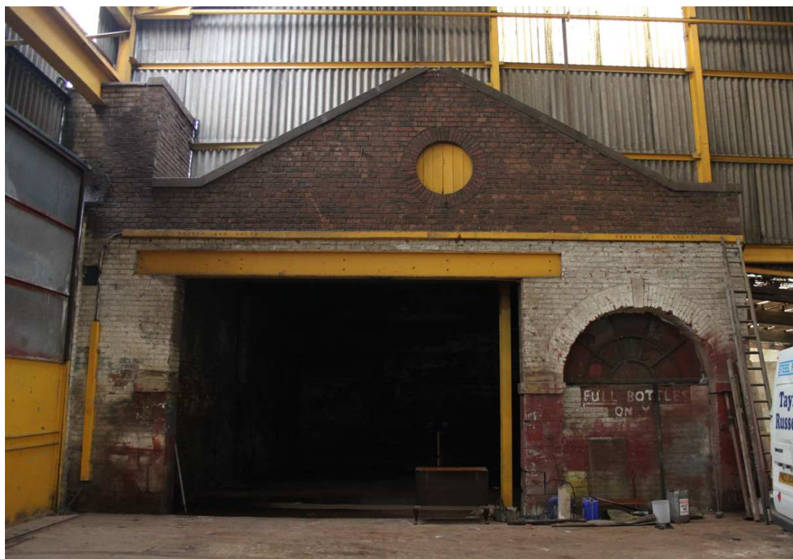
Plate 19: The boiler house added in 1877, with original fanlight window and square base of the brick-built chimney
