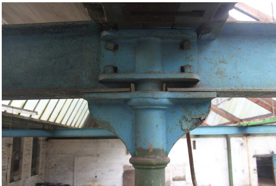
Plate 24: Column head and bolting plate in the c 1910 weaving shed
