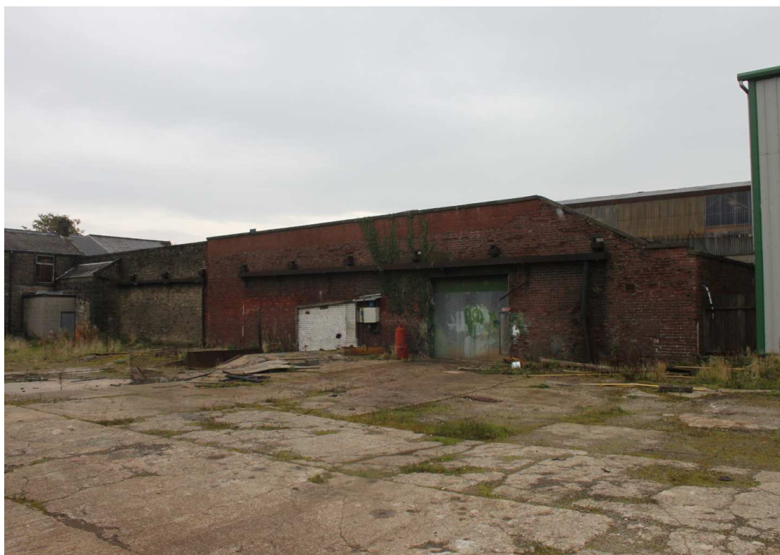
Plate 9: The west-facing elevation of the weaving shed, showing the two phases of construction
