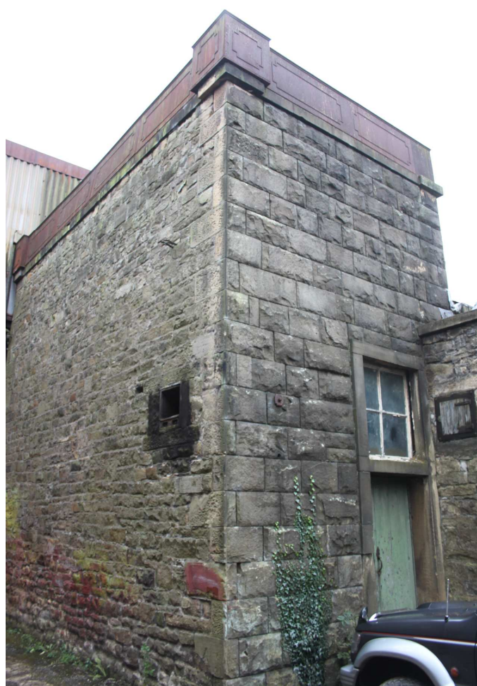
Plate 16: Two-storey structure against the north face of the weaving shed
