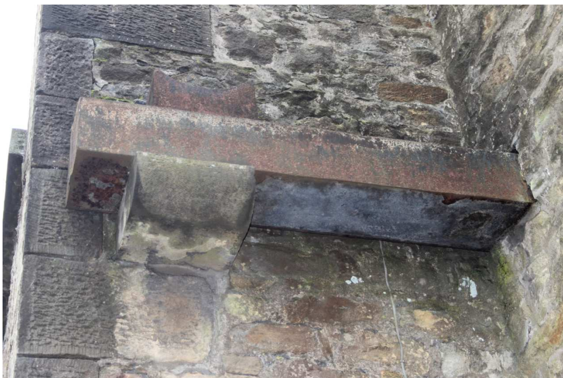
Plate 13: External gutter in the north-west corner of the weaving shed
