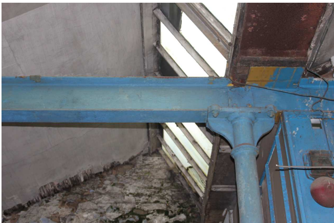
Plate 18: Detail of column head in the stone-built part of the weaving shed
