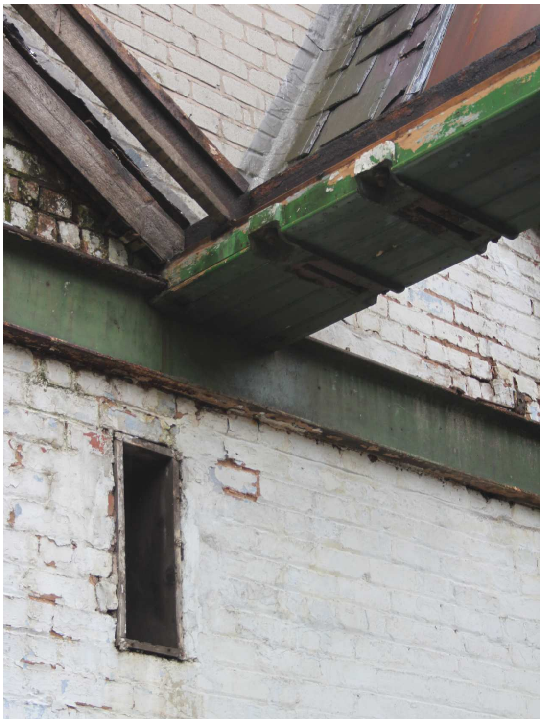
Plate 26: Hanger brackets mounted on the valley beams in the c 1910 weaving shed
