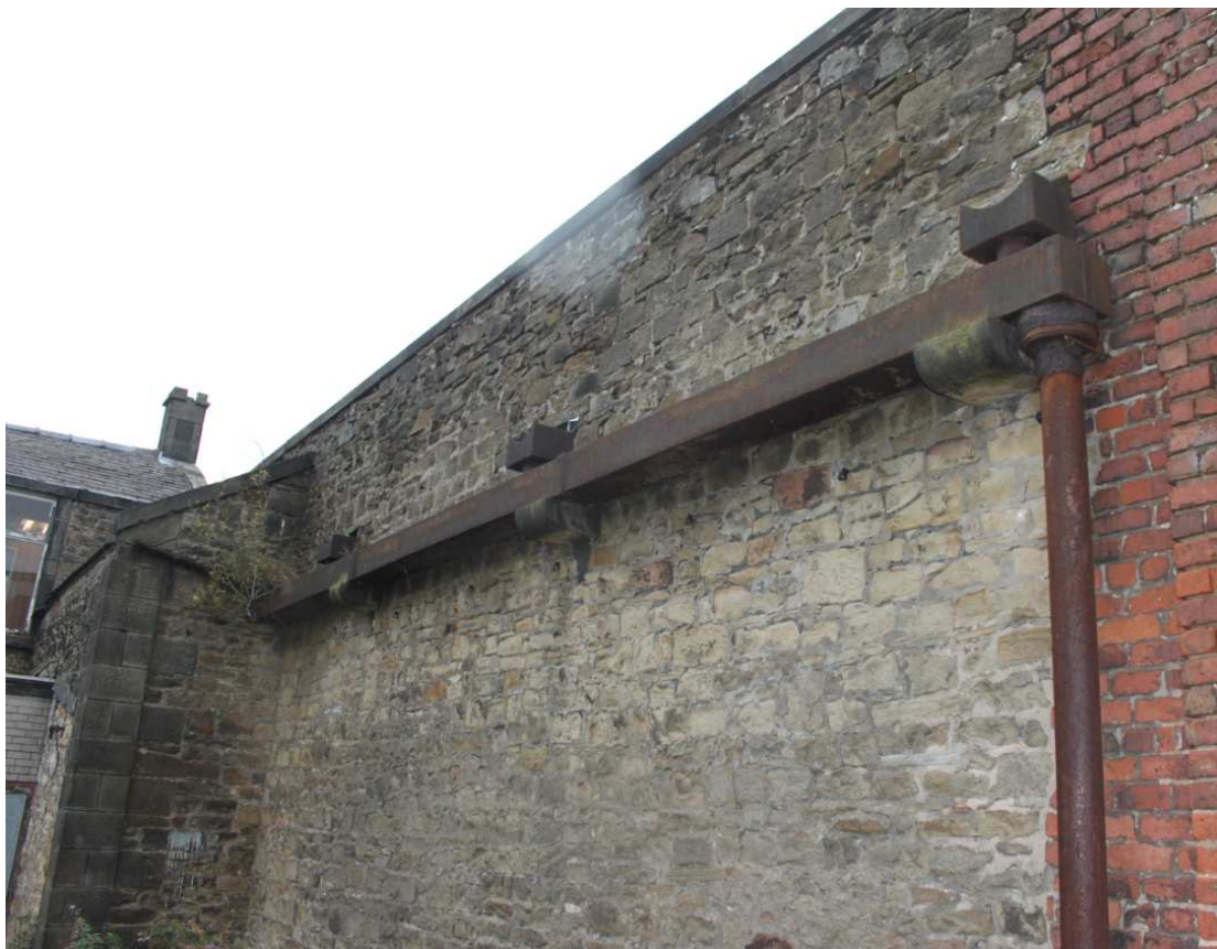
Plate 11: Detail of cast-iron gutter attached to the western wall of the stone-built section of the weaving shed, with the lean-to structure to the rear
