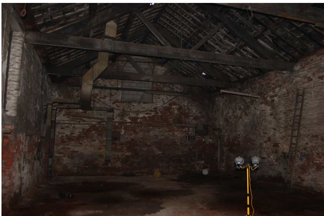
Plate 23: Roof structure in the boiler house
