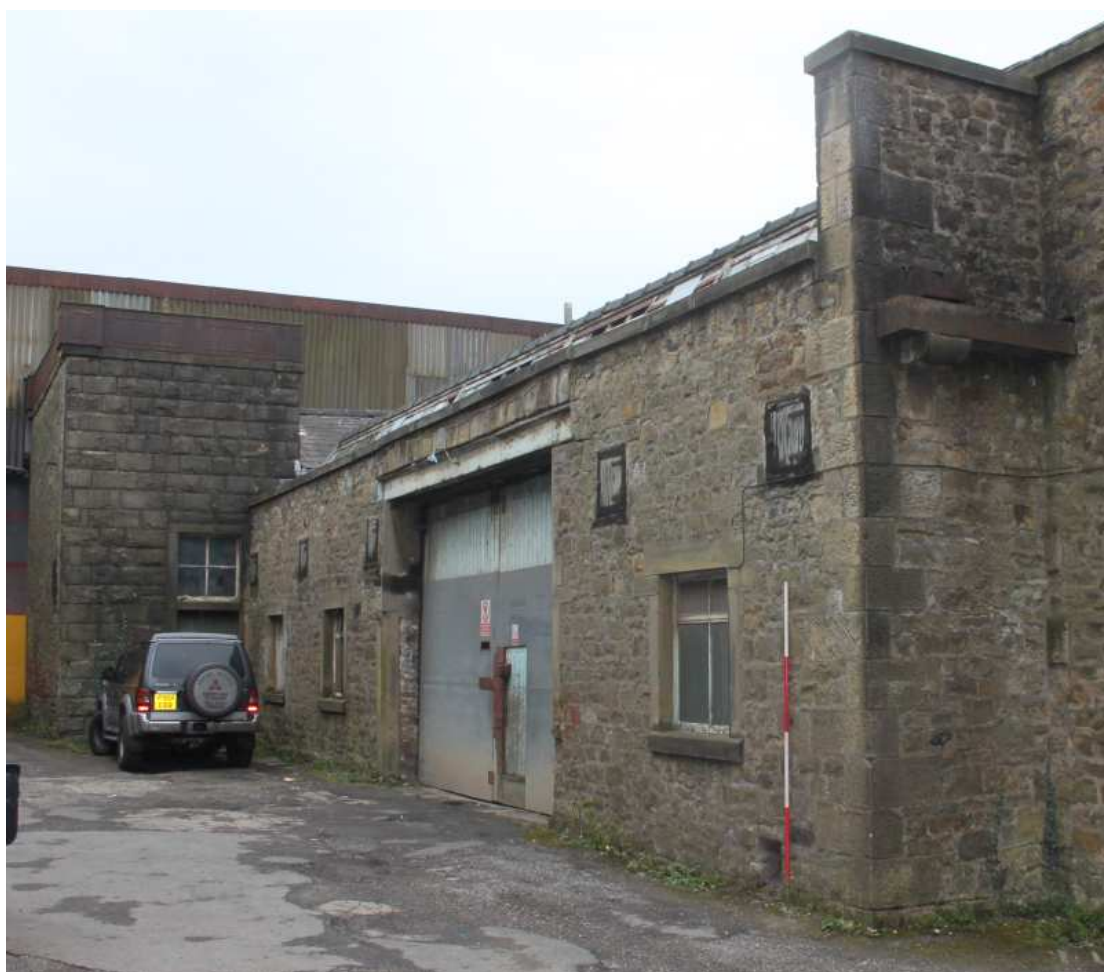
Plate 14: The northern elevation of the weaving shed
