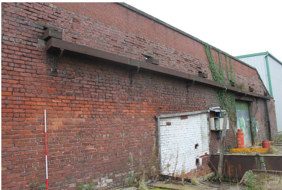
Plate 12: Detail of cast-iron gutter attached to the brick-built section of the weaving shed. The rebuilt parapet wall can also be discerned
