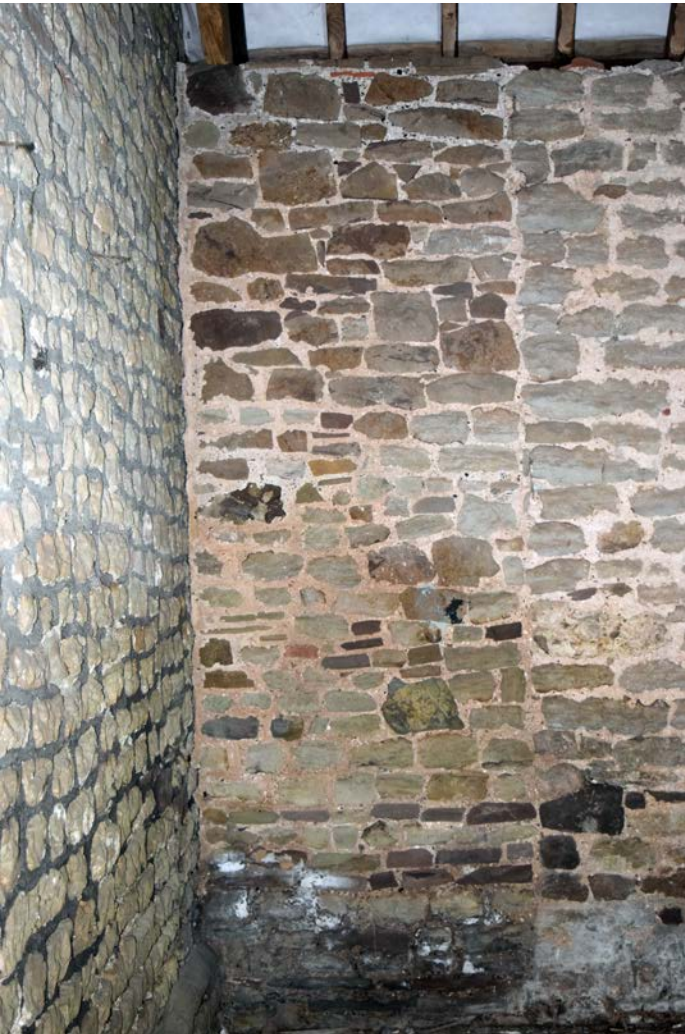
Plate 58: The break in masonry on the interior of the barn, looking north
