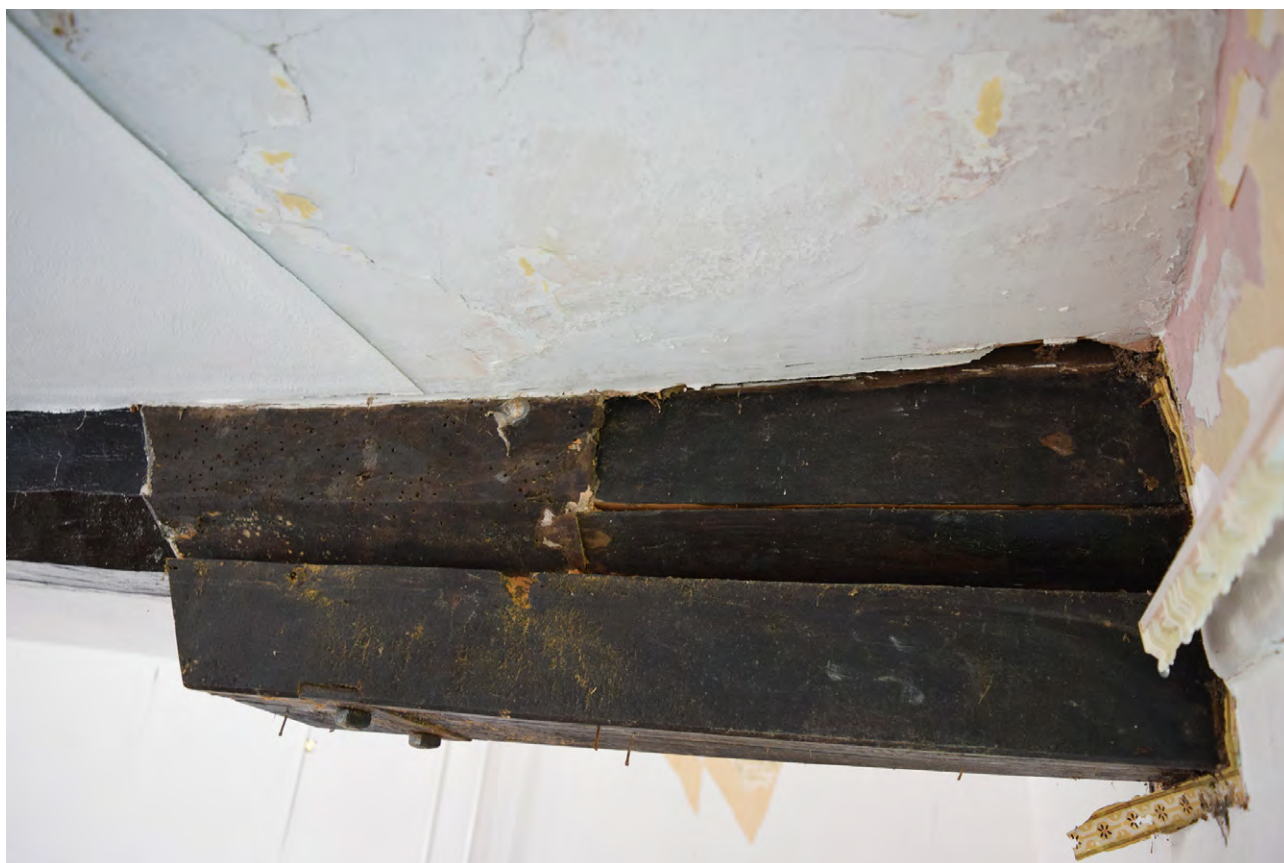
Plate 60: The west end of the ceiling beam in the south bedroom of Shepperdine farmhouse, looking south (What appears to be a break in the beam on the far left is in fact an impression left by the removed paneling)
