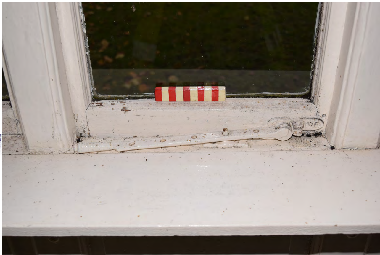
Plate 32: The historic window stay of the window in the west wall of the central reception room of Shepperdine farmhouse, looking west
