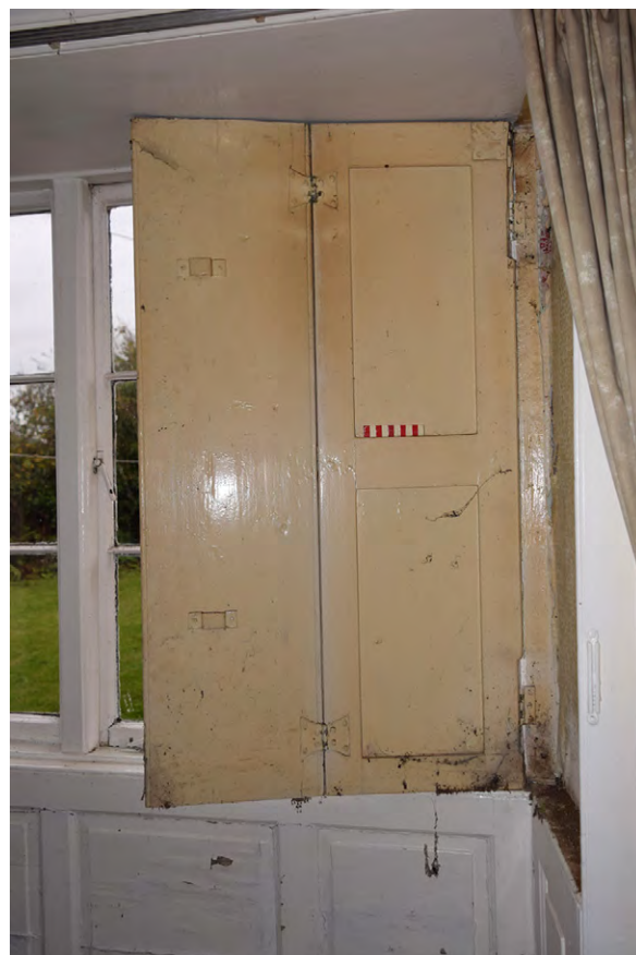
Plate 30: The unfolded pocket shutter of the window in the east wall of the central reception room of Sheppardine farmhouse, looking east
