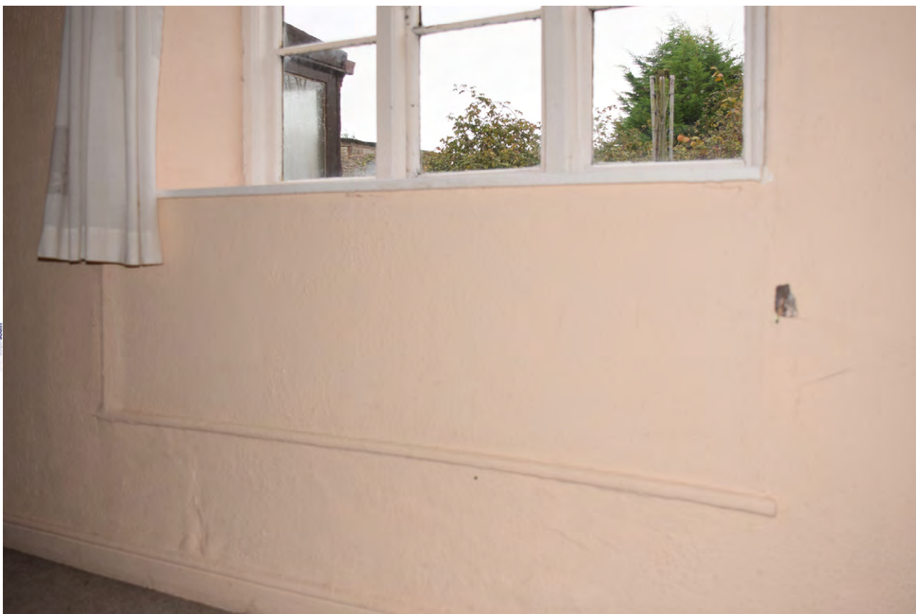
Plate 20: Impression of a window seat that has now been filled in under the east window in the rear corridor of the ground floor of Shepperdine farmhouse, looking north-east
