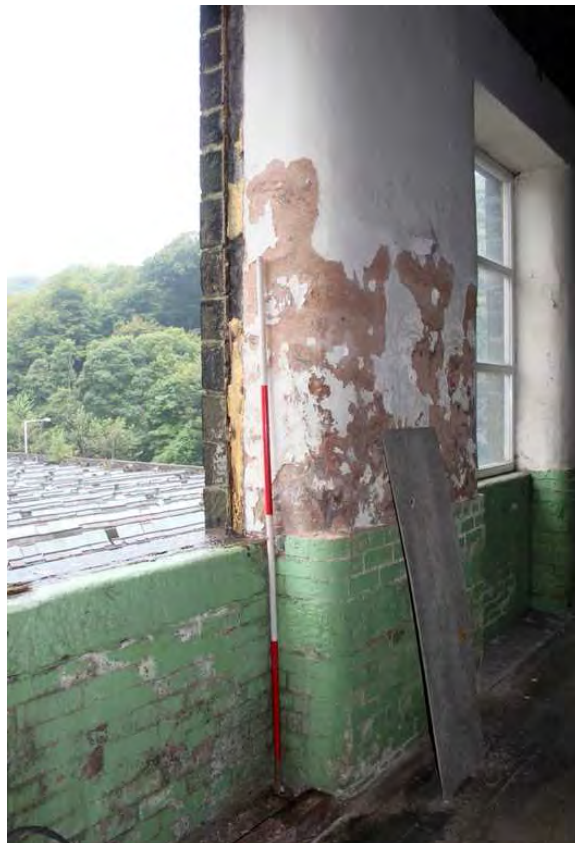
Plate 9: Brick plinth below rendered rubble walls, second floor, spinning block
