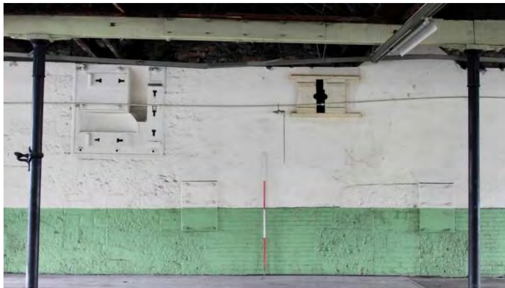
Plate 18: Top bearing and offset line shaft end bearing, second floor of the spinning block
