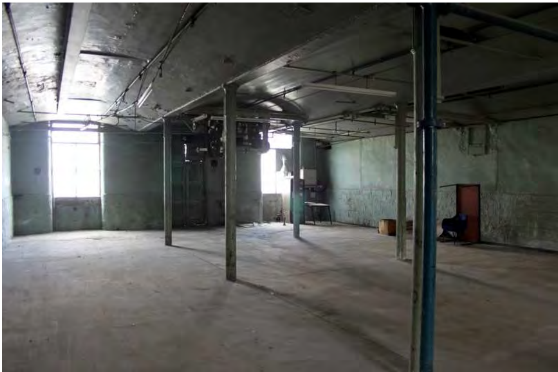
Plate 21: Fireproof brick arch construction with straining rods within eastern bays of original mill, first floor, preparation block
