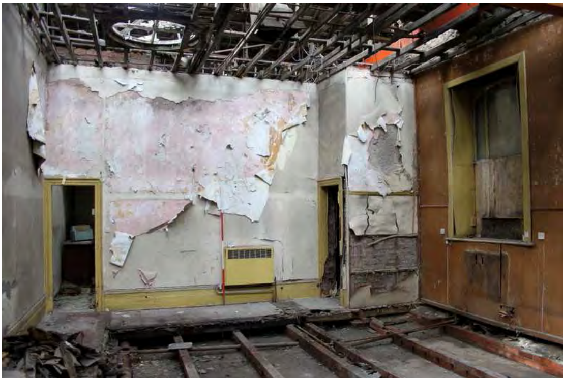
Plate 69: Sprung floor of office and entrance vestibule
