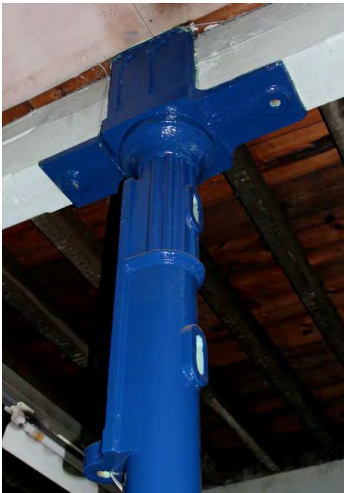
Plate 15: Casting for through bolts opposite bolting face on first-floor column in the spinning block
