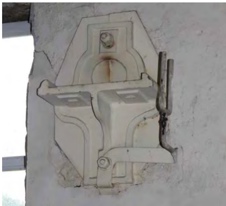
Plate 48: Ornate end bearing of line shaft, second floor, eastern extension of mill
