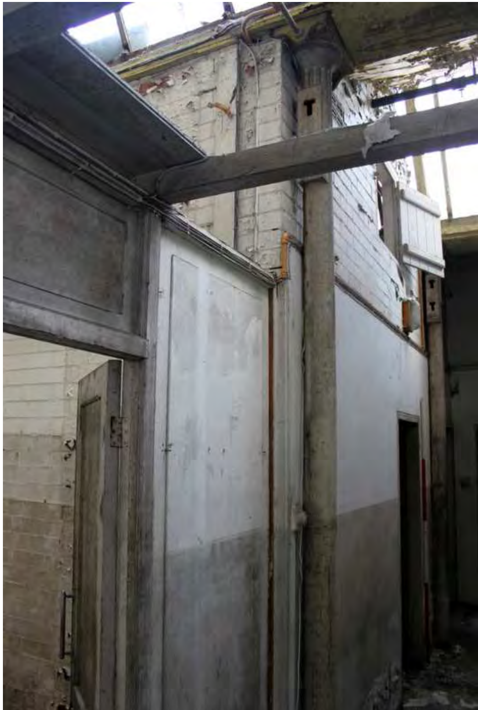
Plate 76: Inserted brick and timber partitions enclosing original columns within weaving shed
