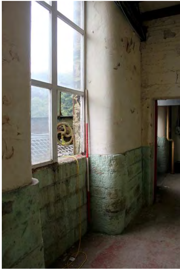
Plate 8: Sandstone plinth below rendered rubble walls, first floor, spinning block
