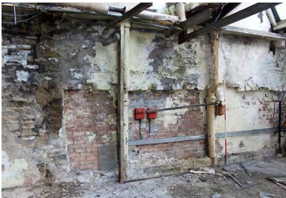
Plate 77: Ragged brick-lined rebate within west wall of weaving shed
