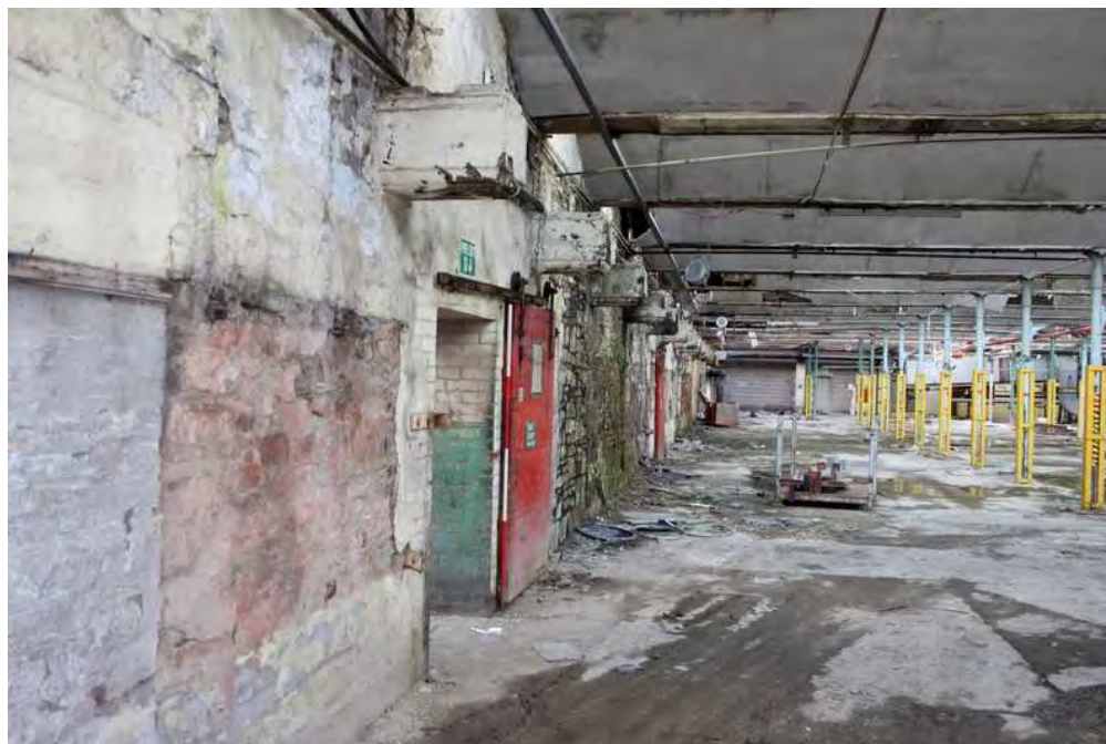
Plate 84: Sandstone corbels for drive shaft bevel gears, east wall of western weaving shed
