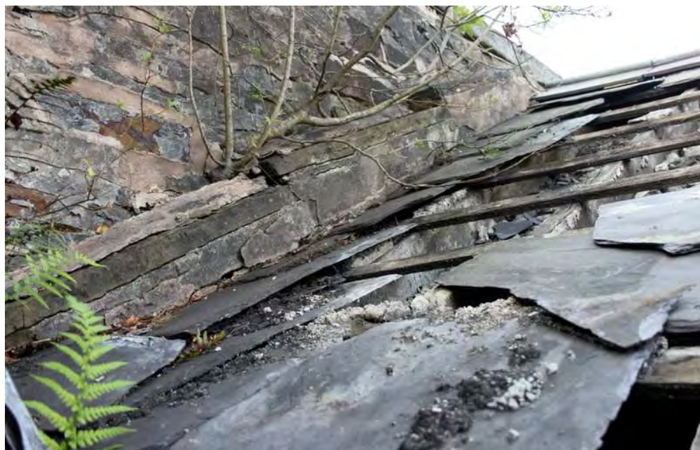
Plate 54: Original sandstone flag roof tiles, western weaving shed
