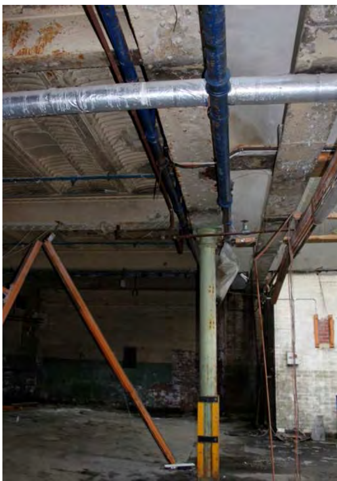
Plate 92: Rivetted I-section beams and late columns carrying first floor workshops
