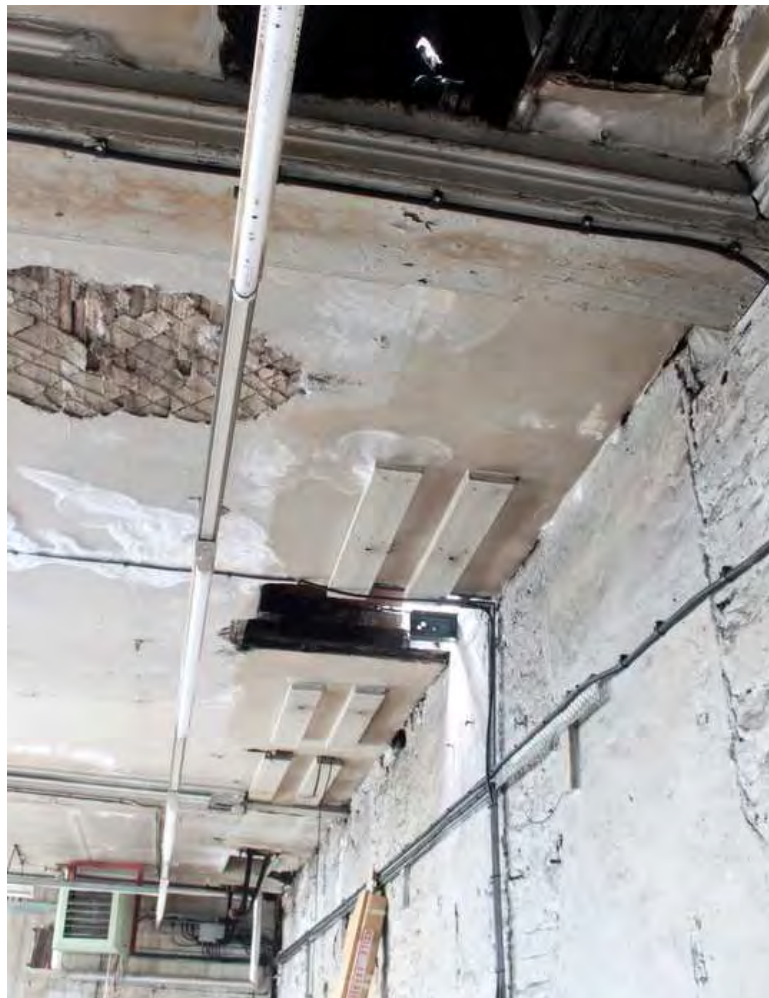
Plate 102: Detailed of decorative ceiling, feeding holes, and line shaft hanger mountings
