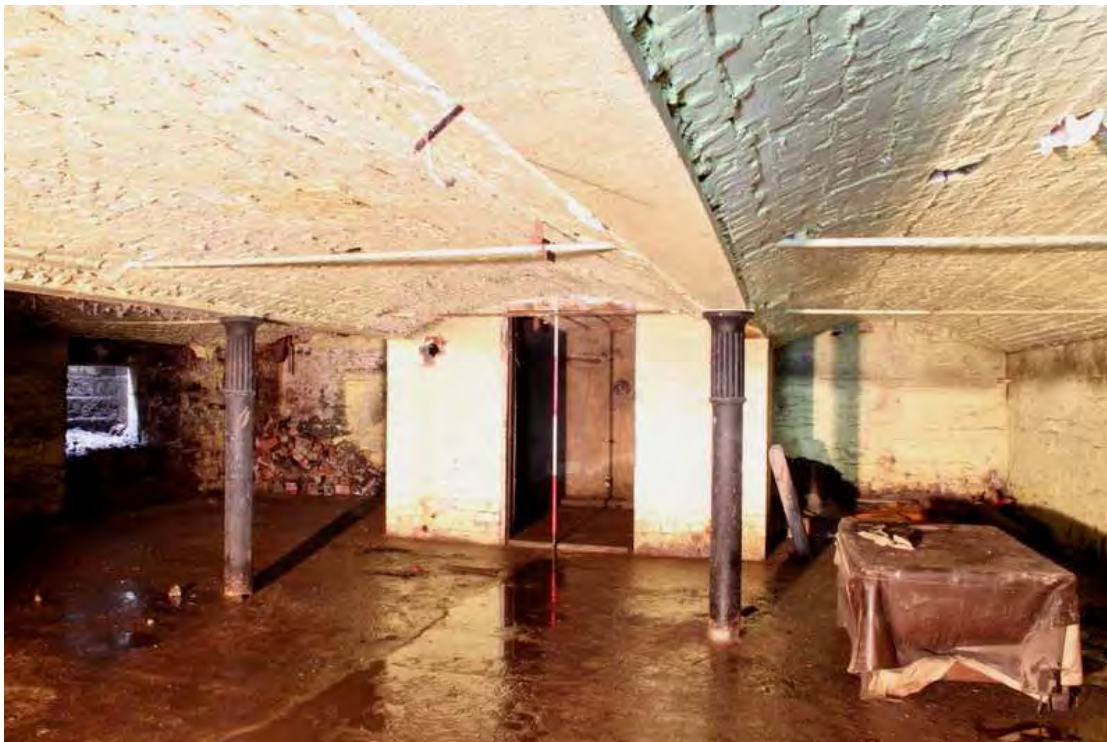
Plate 79: Eastern cellar, with cellar light to alley, and inserted brick chamber
