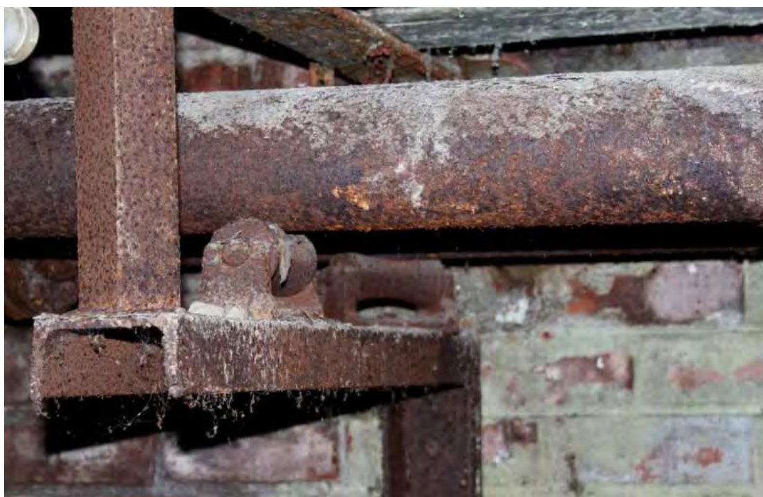
Plate 61: In-situ water pipe on later bracket, incorporating similar rollers to those attached to columns elsewhere within the complex
