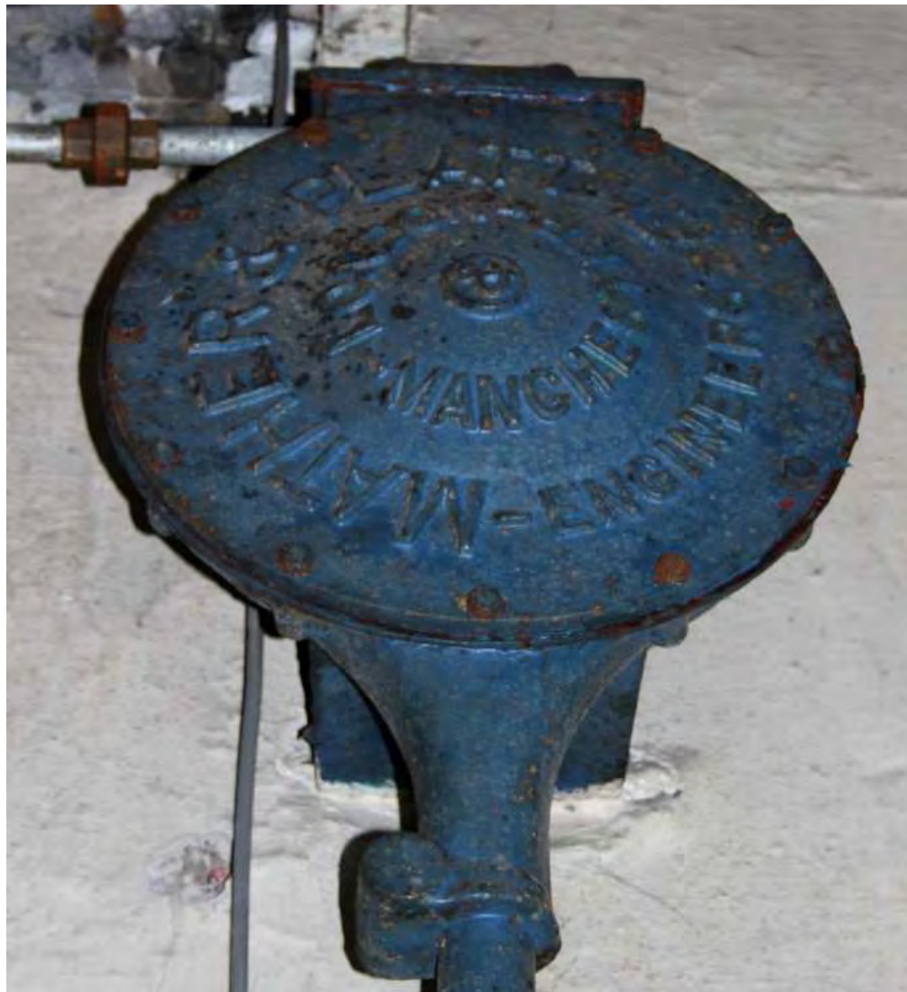
Plate 66: Mather & Platt cover plate for sprinkler system alarm bell
