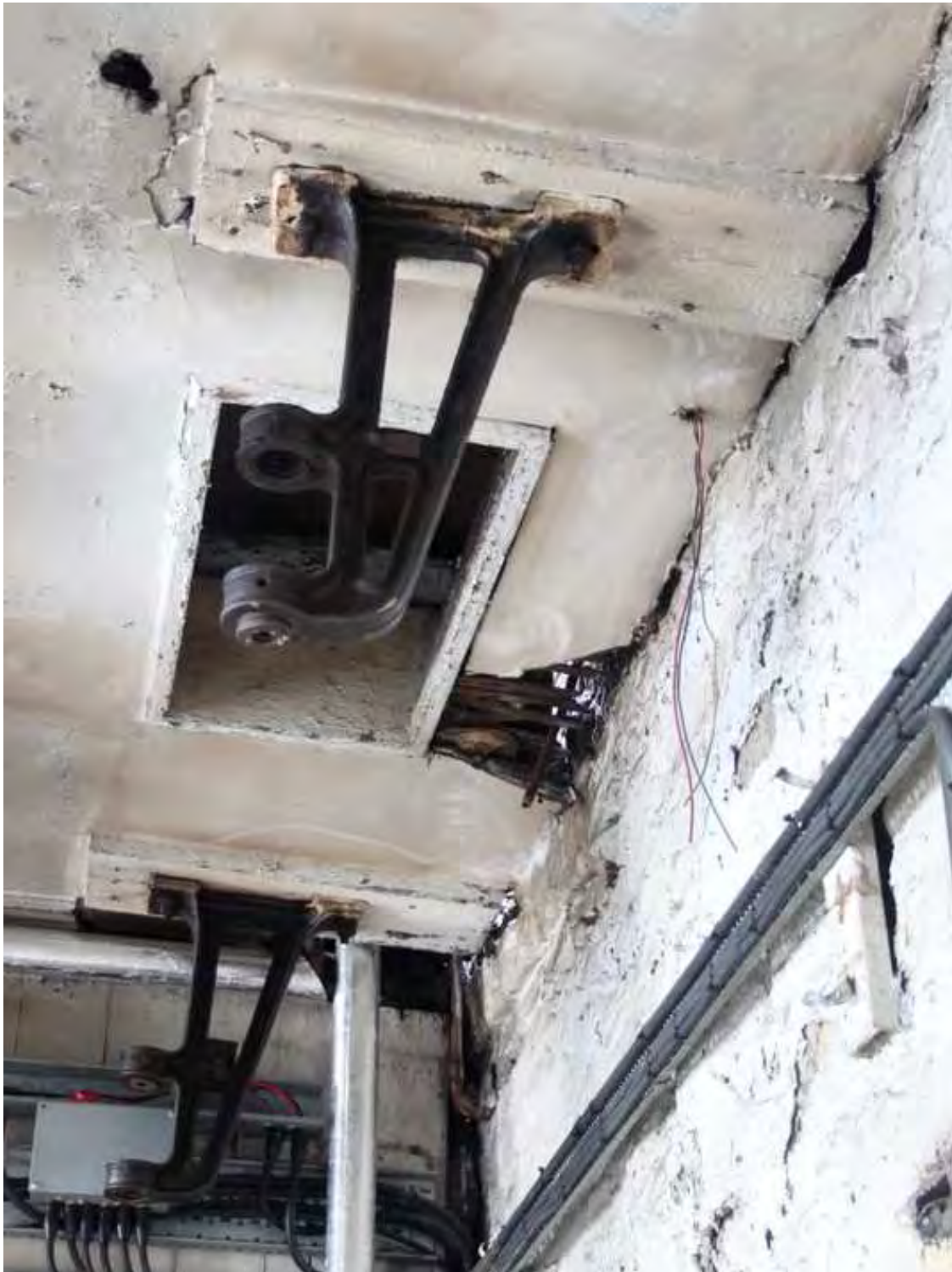
Plate 105: In-situ line shaft hangers, stable block
