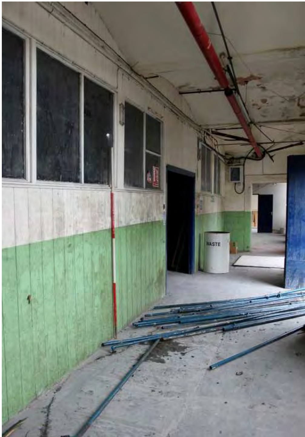
Plate 25: Timber partition and flagstone floor, first floor, preparation block
