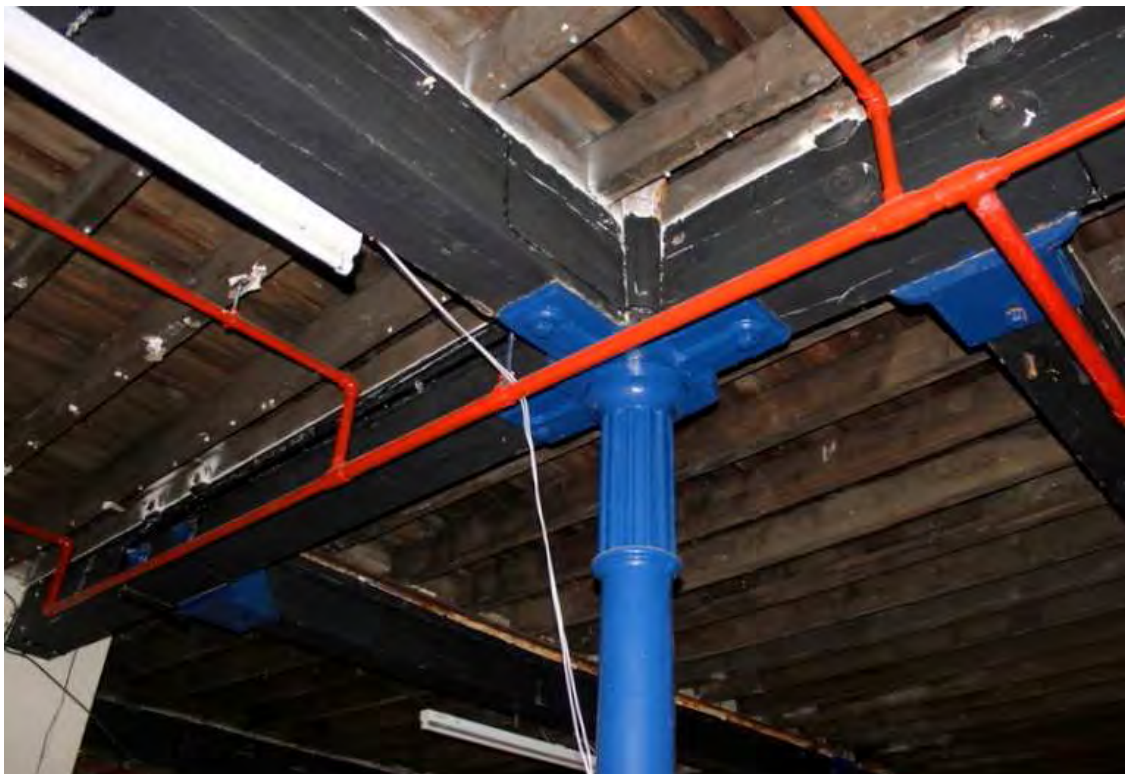
Plate 46: T-shaped column capital, and hangers for ceiling beams, eastern extension of mill
