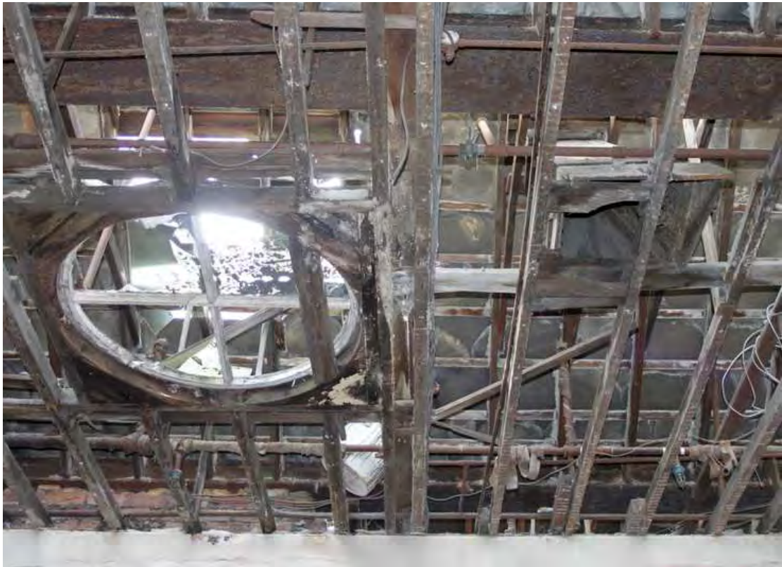
Plate 74: Skylight and ventilation hood within main office
