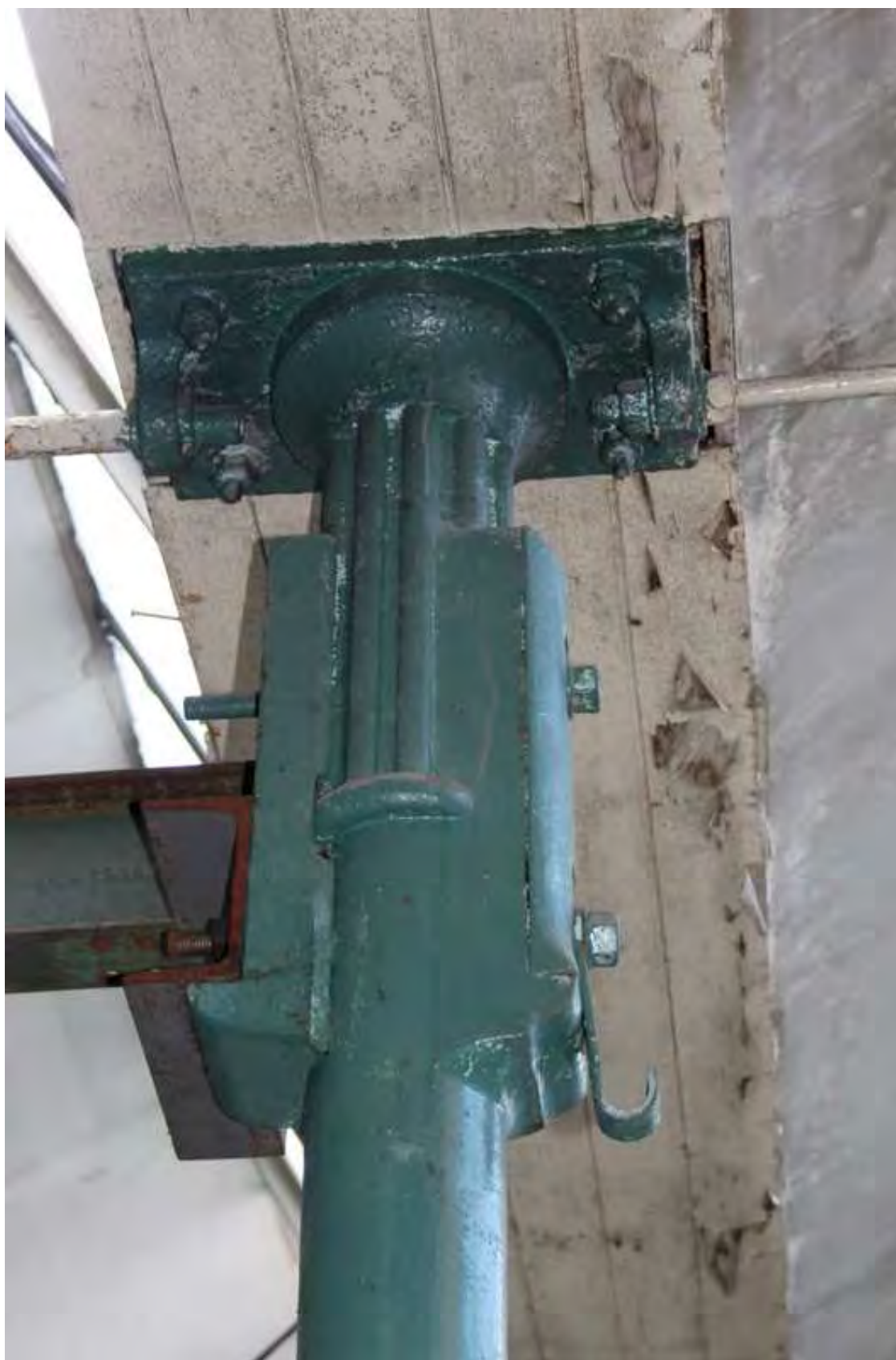
Plate 63: Detail of weaving shed column capital in 16 th bay, with double bolting plate
