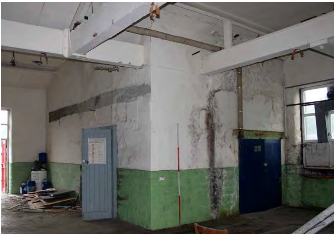
Plate 43: Ceiling beams housed in return of north wall of eastern extension of mill
