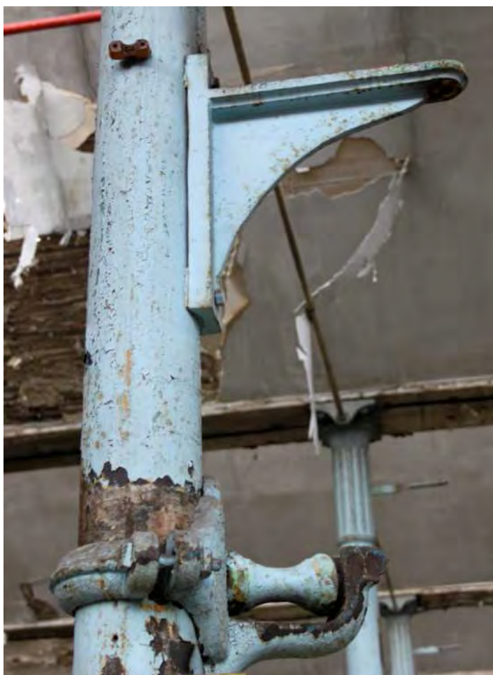
Plate 59: Heating pipe bracket with additional concave-ribbed bracket above, weaving shed
