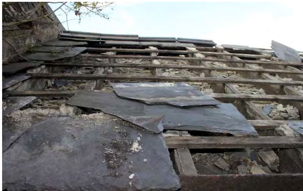
Plate 53: South pitch of saw-toothed roof, weaving shed
