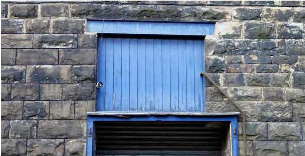
Plate 86: Infilled drive shaft aperture to right of fanlight
