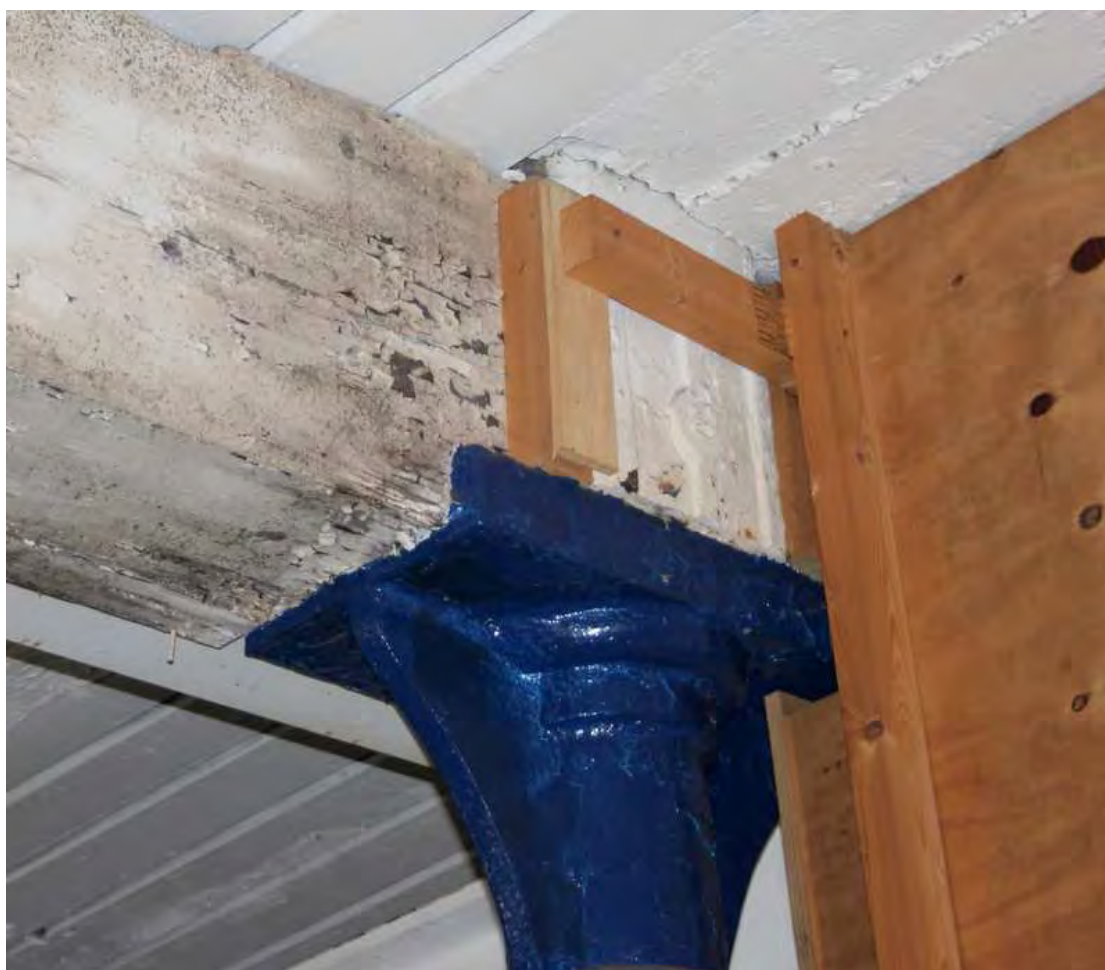
Plate 39: Typical Victorian column capital in extension of three-storey mill
