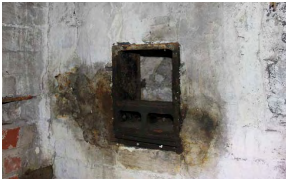
Plate 28: In-situ small end bearing for hoist, first floor, stair tower
