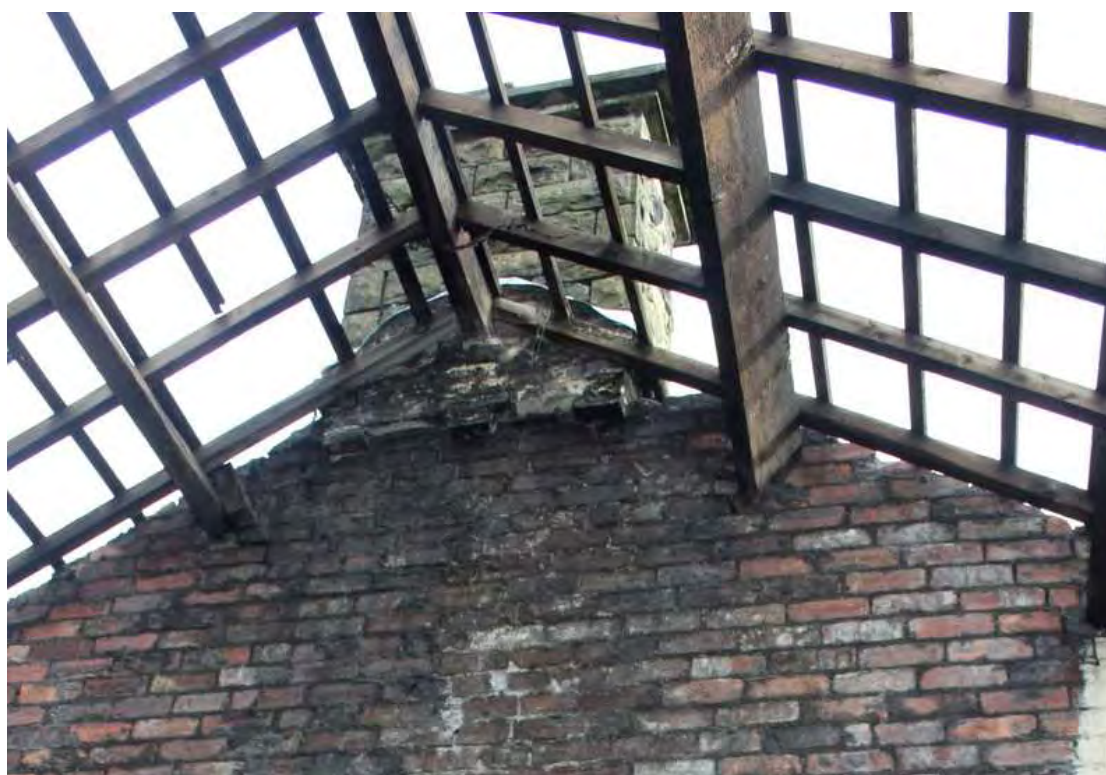
Plate 109: Dressed stone chimney stack, above brick partition wall
