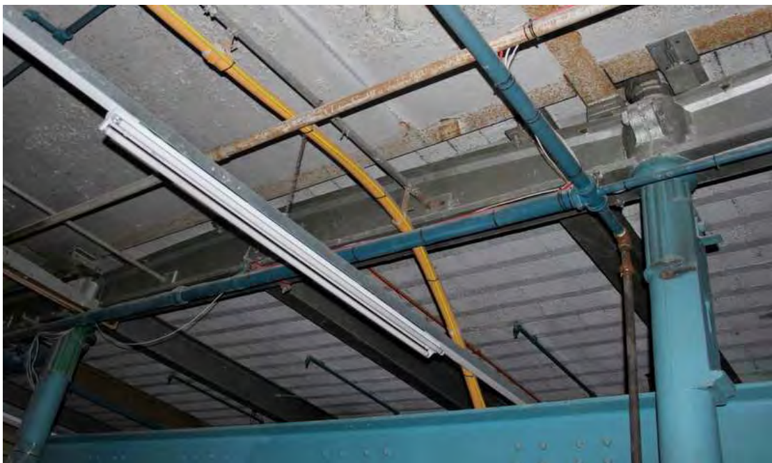
Plate 22: Fireproof brick arch construction showing inverted fish-bellied beams, ground floor, preparation block
