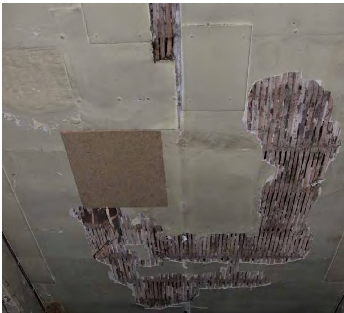
Plate 11: Detail of lath and plaster ceiling on the ground floor of the spinning block
