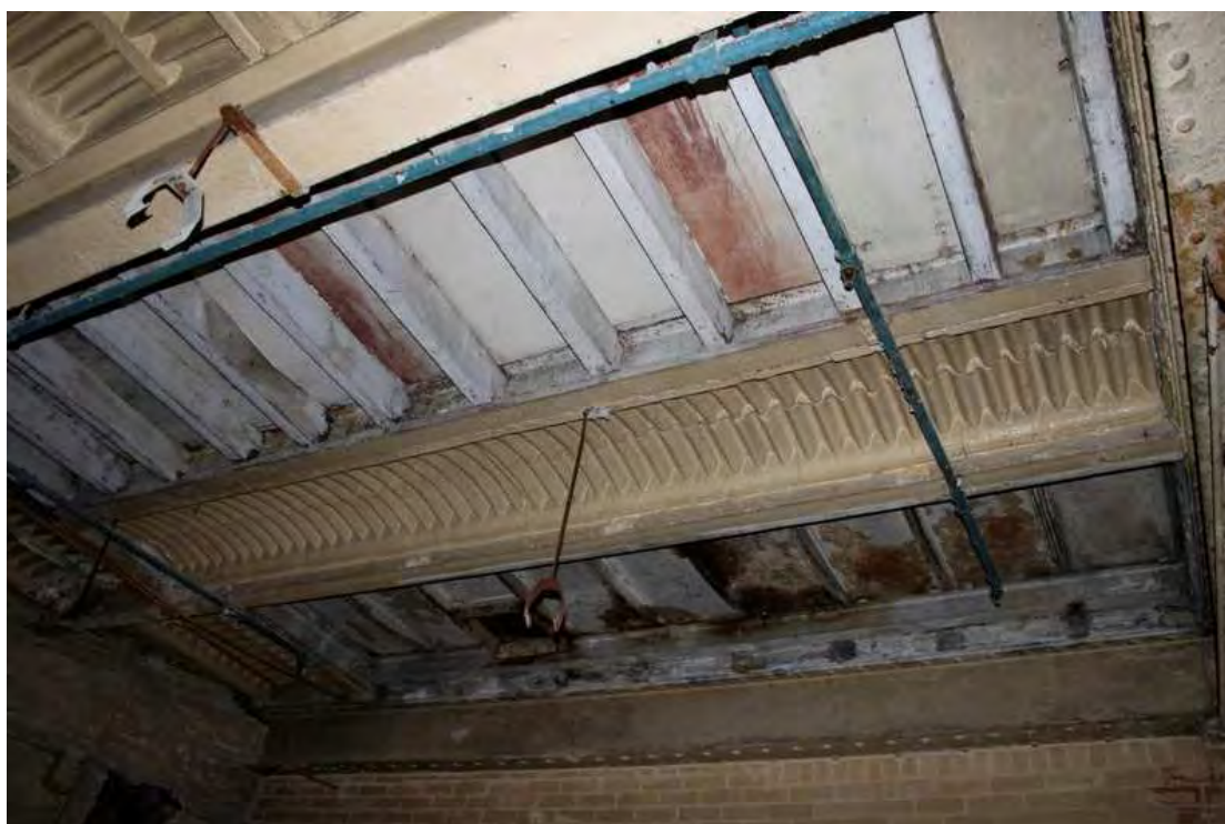
Plate 93: Concrete, timber, and iron sheet floor of first-floor workshops
