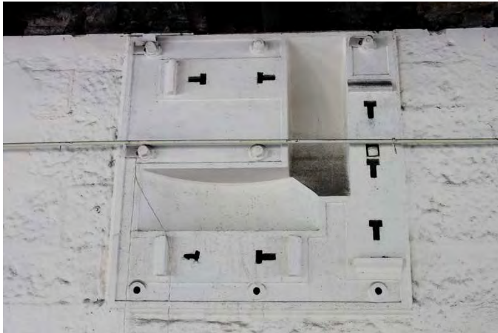
Plate 17: Top bearing for upright shaft in the spinning block, with recesses for bevel gears
