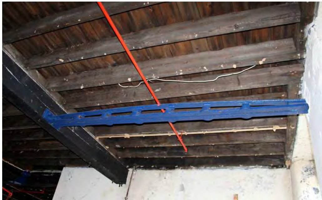
Plate 47: Perforated fish-bellied beam with bolts for line shaft hanger on adjacent beam, eastern extension of mill
