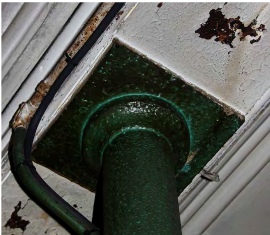
Plate 104: Detail of column capital, stable block
