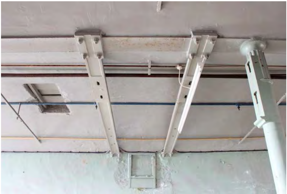
Plate 23: Bearing box and associated fish-bellied beams for bevel gear hanger, first floor, preparation block
