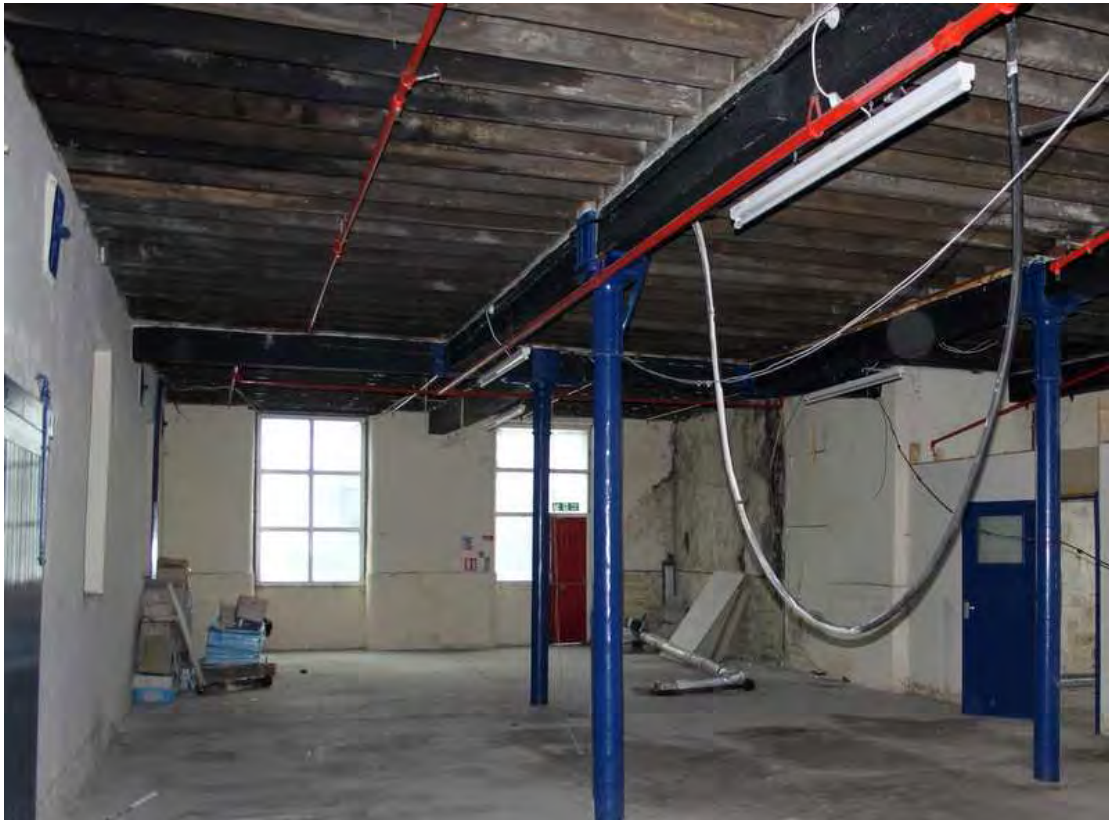
Plate 45: Offset beams within ceiling construction within eastern extension of mill, first floor
