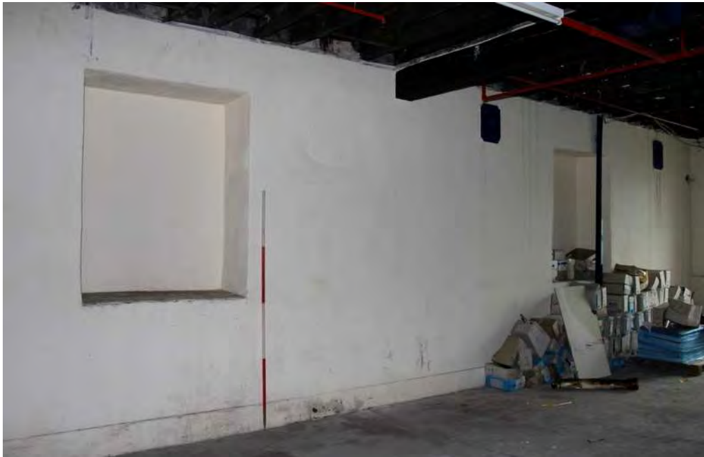
Plate 26: Blocked window apertures in external face of original gable wall, first floor, preparation block
