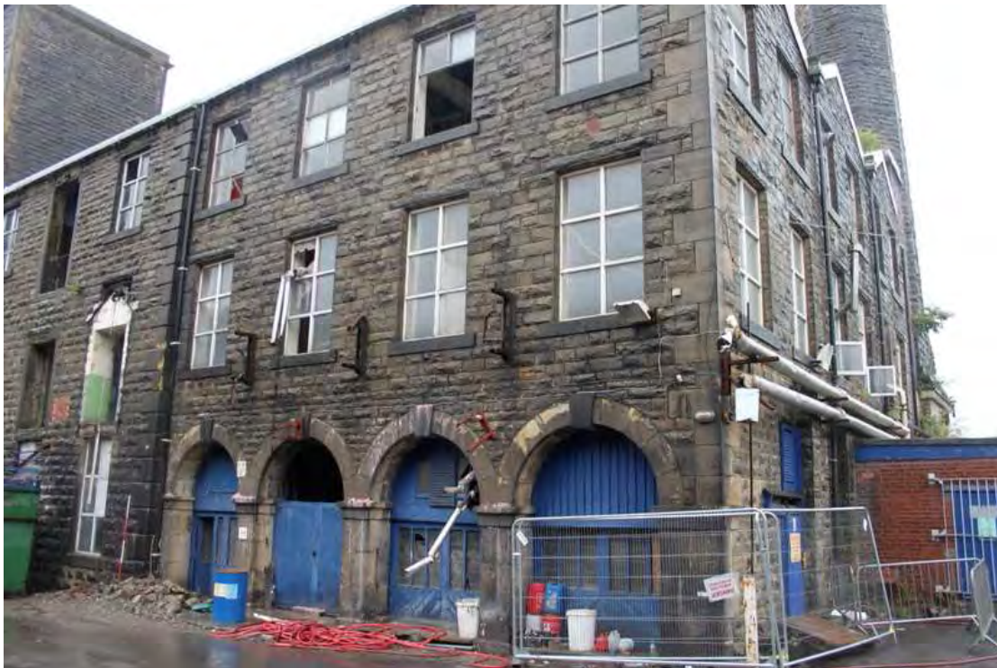
Plate 36: Southern face of the extension to the main mill building, principally erected as a boiler house
