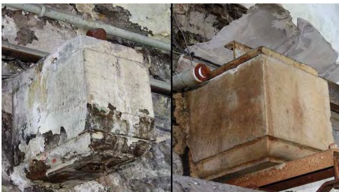
Plate 90: Original drive shaft corbel (left) and secondary corbel (right)
