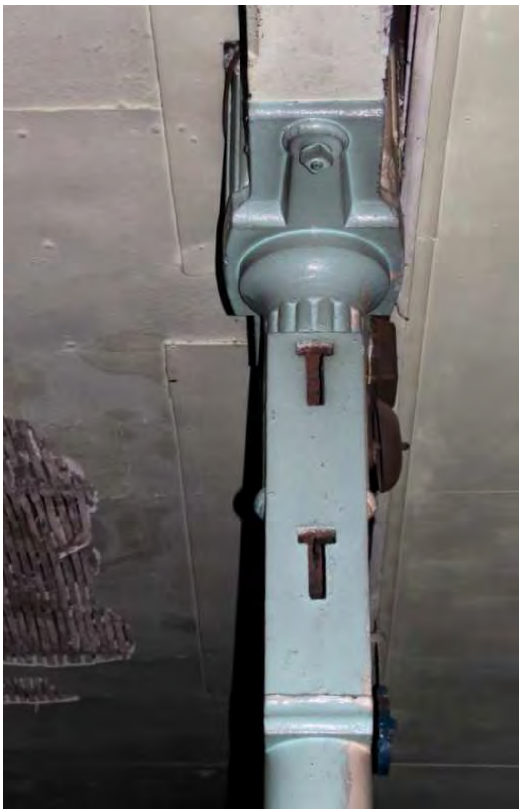
Plate 14: Bolting face on ground-floor column in the spinning block
