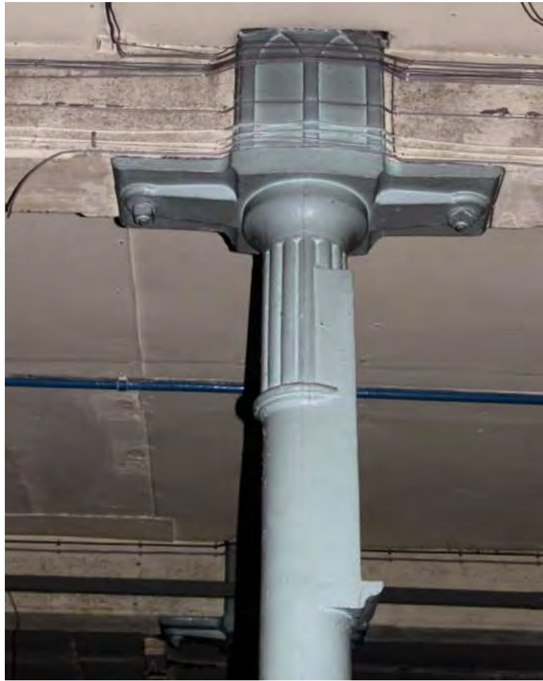
Plate 12: Detail of ground-floor columns in the spinning block
