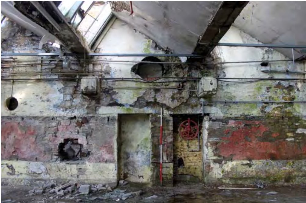
Plate 87: Privy entrances in east wall of western weaving shed, with aperture for removed stone trough
