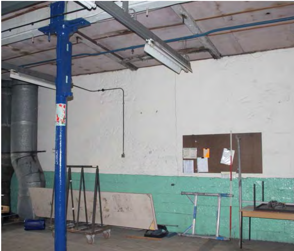
Plate 16: Blocked aperture in east wall of spinning block at first-floor level, with ceiling trimmer above, and line shaft brackets on the adjacent column
