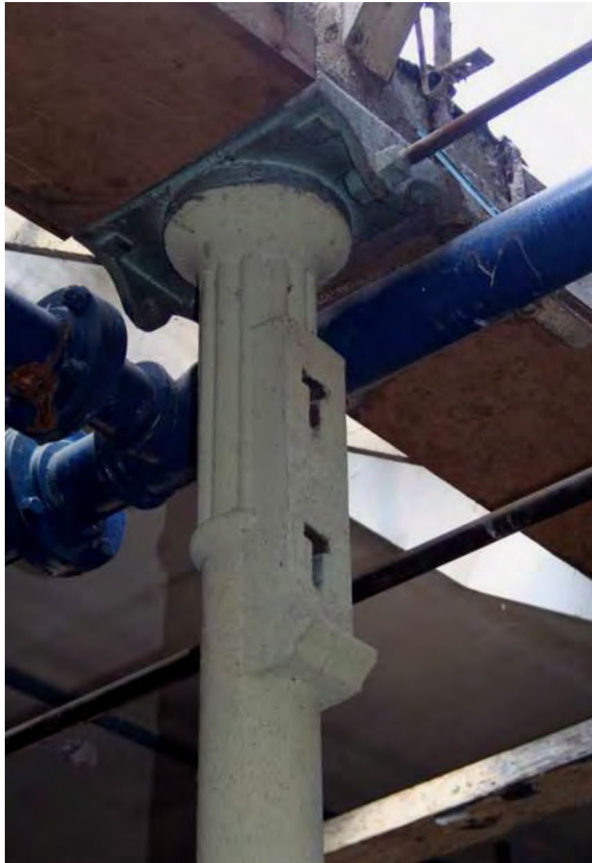
Plate 50: Column capital in original weaving shed, with line shaft bolting plate
