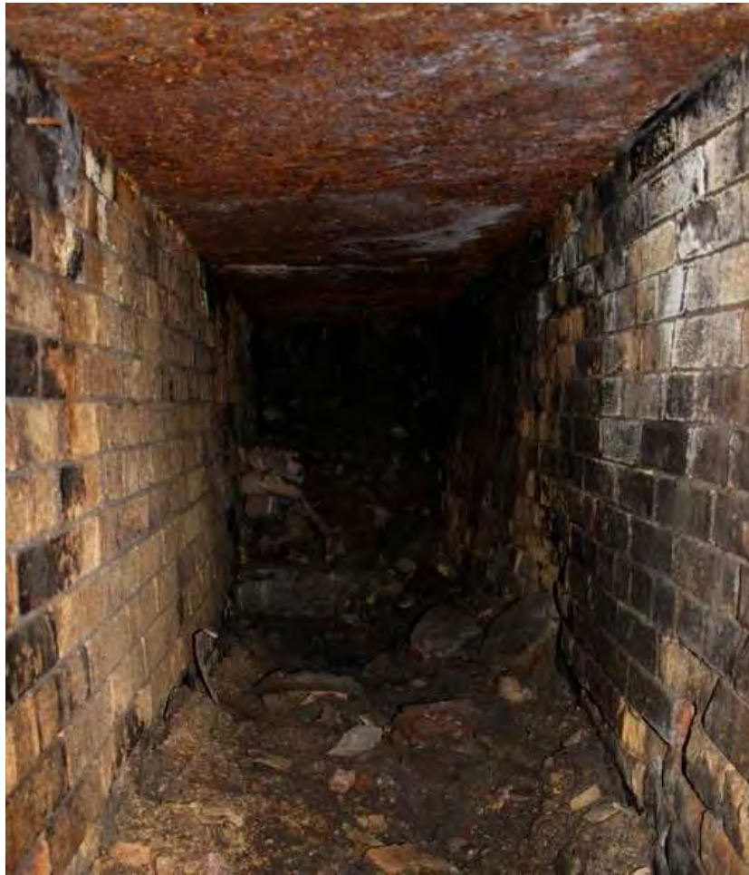
Plate 42: Detail of bypass flue
