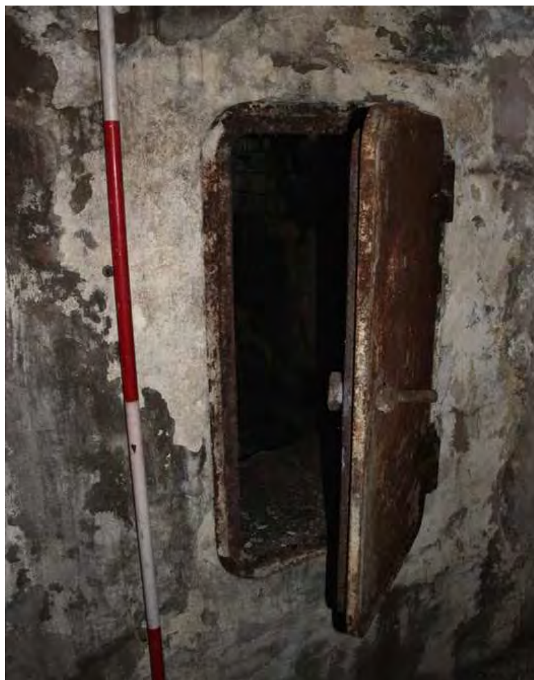
Plate 41: Iron door on access / bypass flue from boilers to chimney
