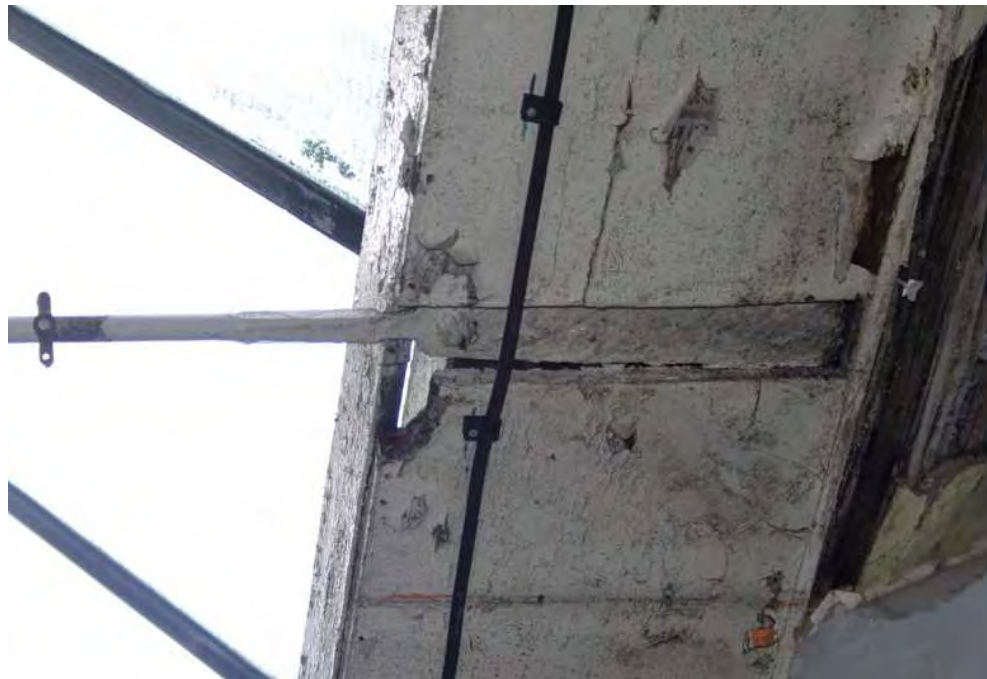
Plate 64: Stirrup for straining bar attachment to valley beam
