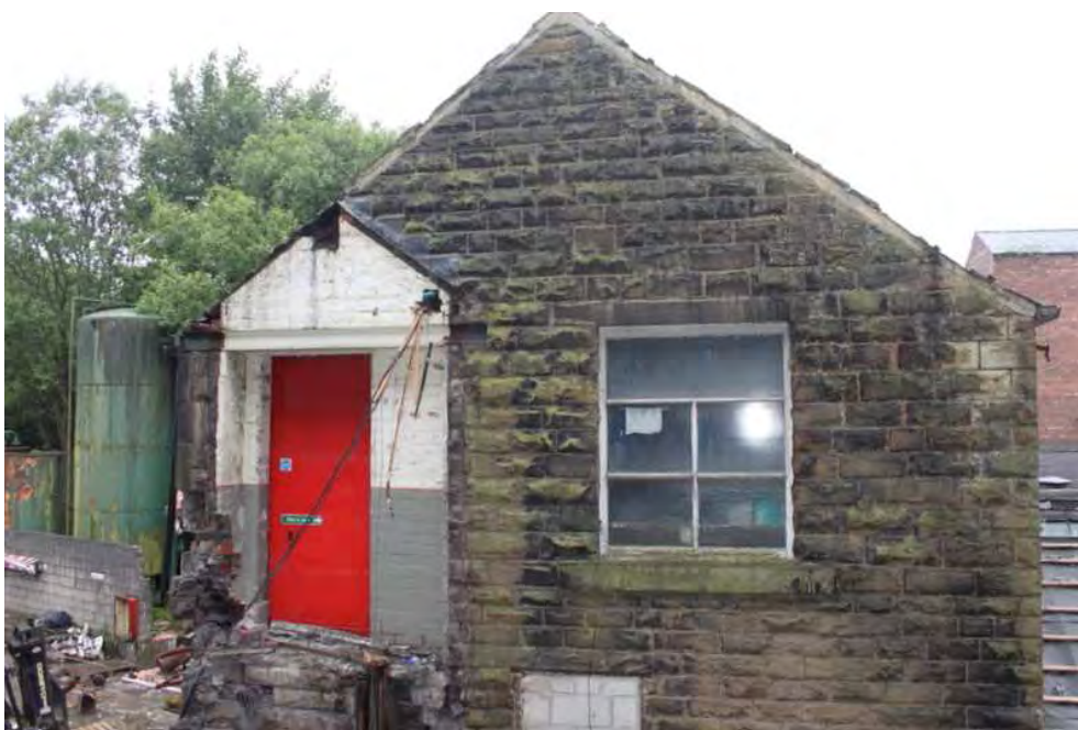
Plate 97: Doorway and wall scar for walkway between main mill and workshops above weaving shed
