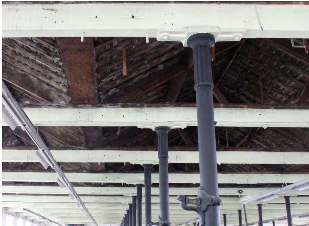
Plate 19: Bolts protruding from soffit for line shaft hangers, with further hanger attachment bolt holes in beam face
