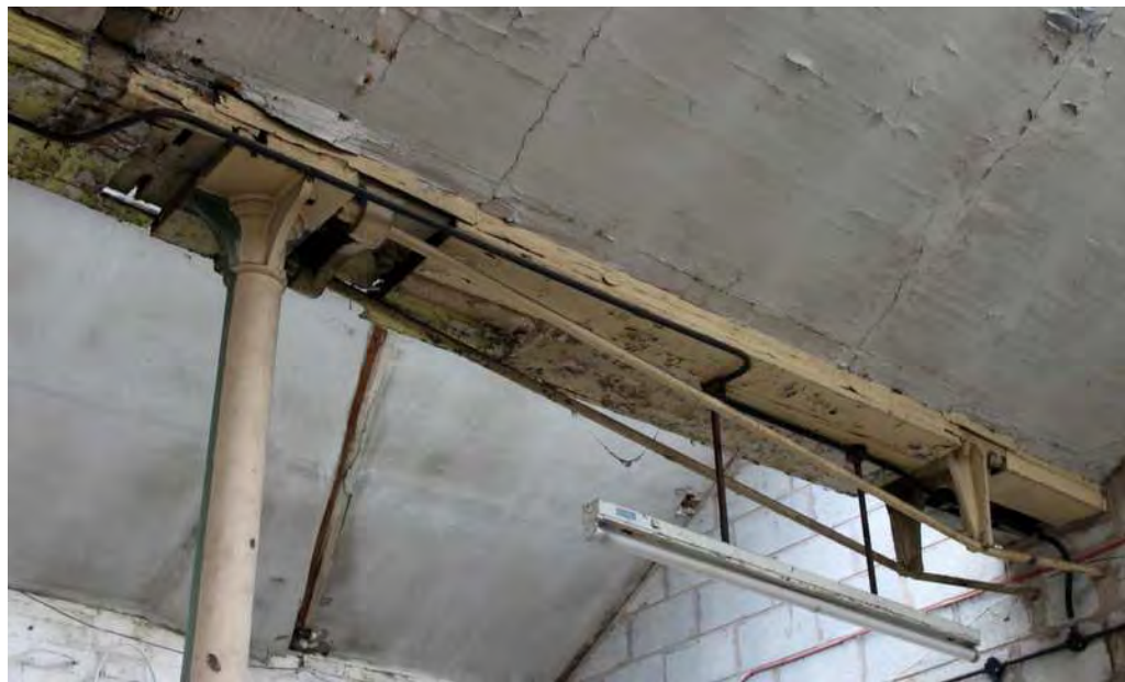
Plate 65: Replaced column with longitudinal tensioning bar
