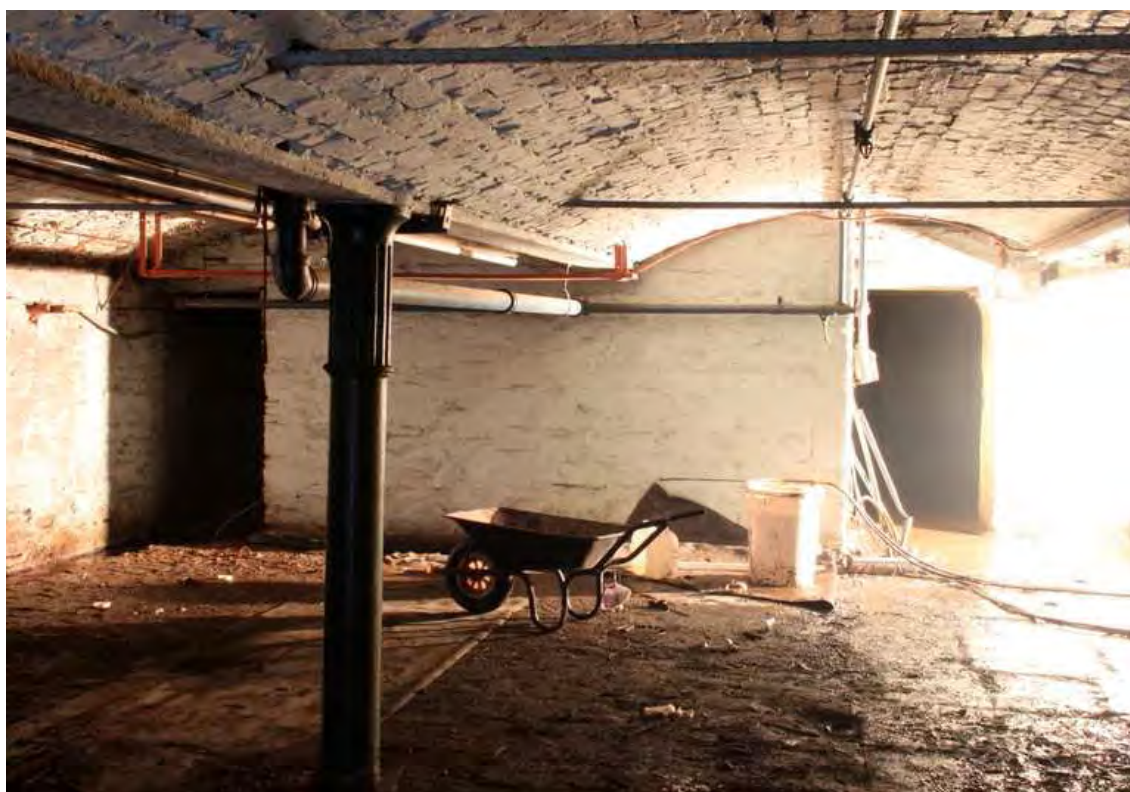
Plate 78: Brick arched ceiling and stair wall within western part of cellar
