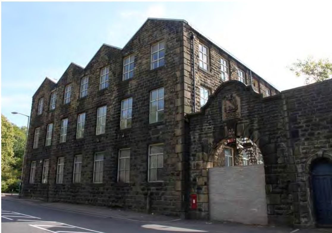
Plate 6: Spinning block from Burnley Road, with quadruple-span roof and dressed quoins
