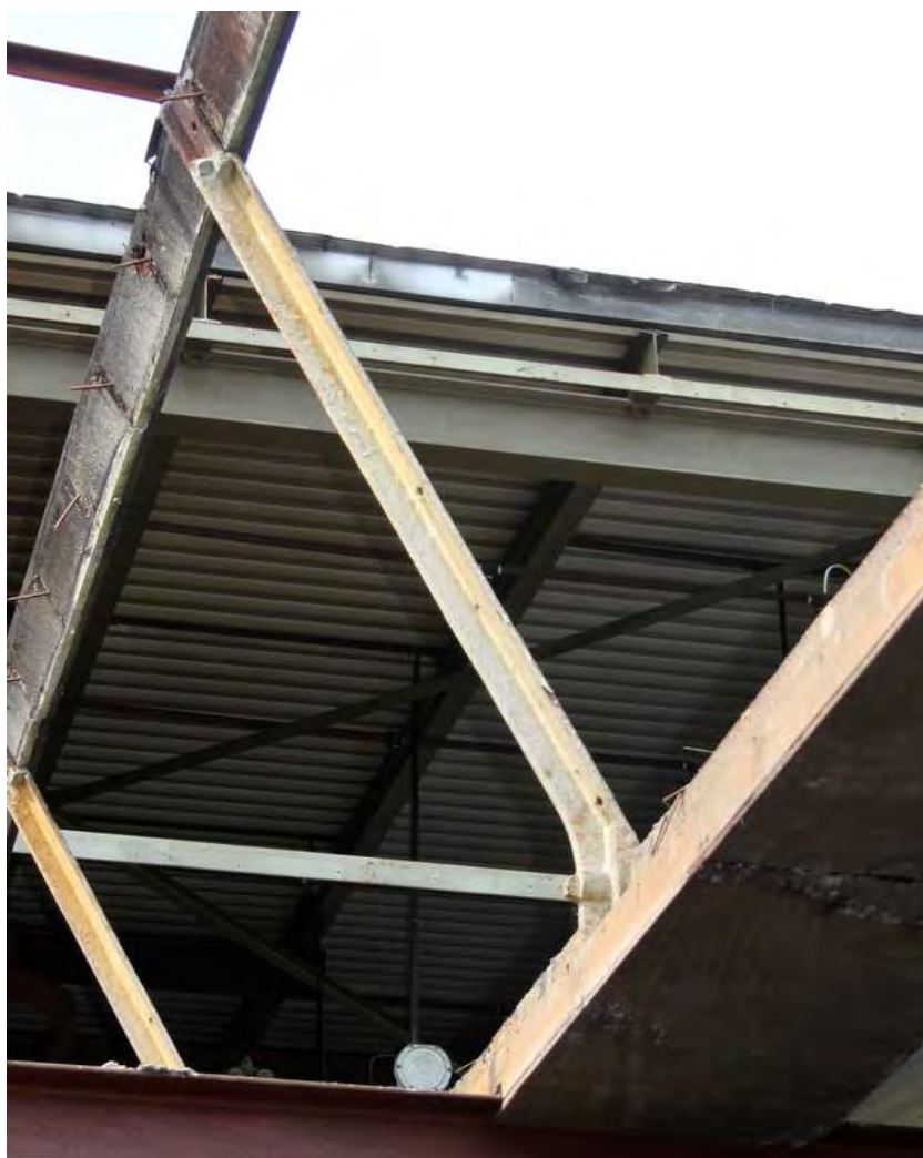
Plate 89: T-section cast-iron rafters of weaving shed extension
