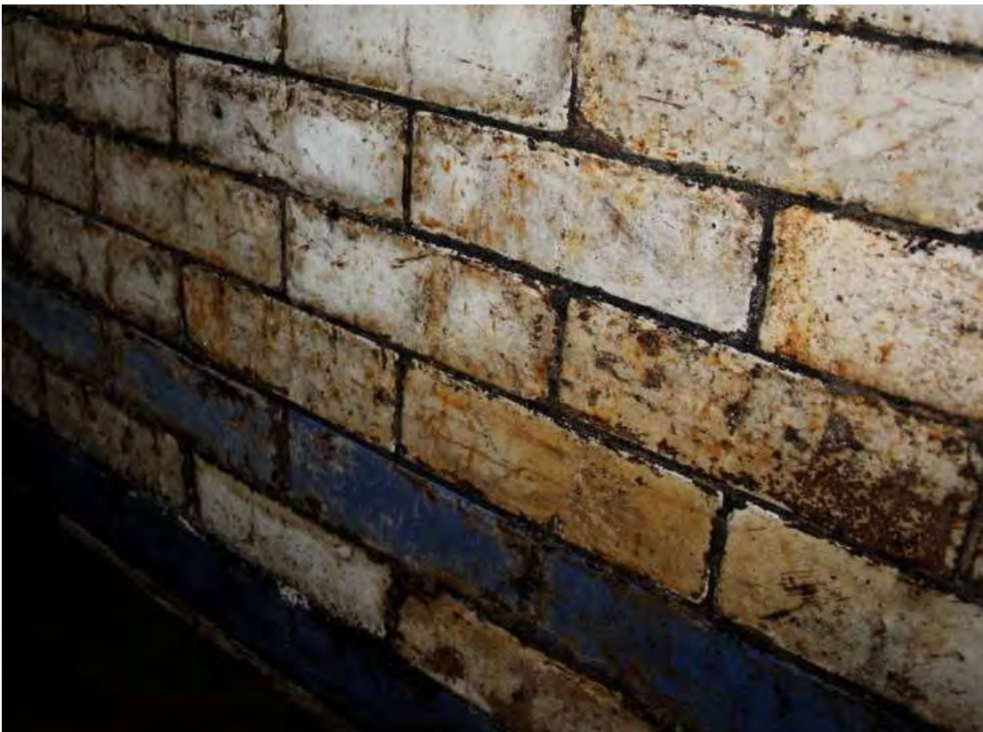
Plate 82: Detail of glazed decorative brickwork within tunnel
