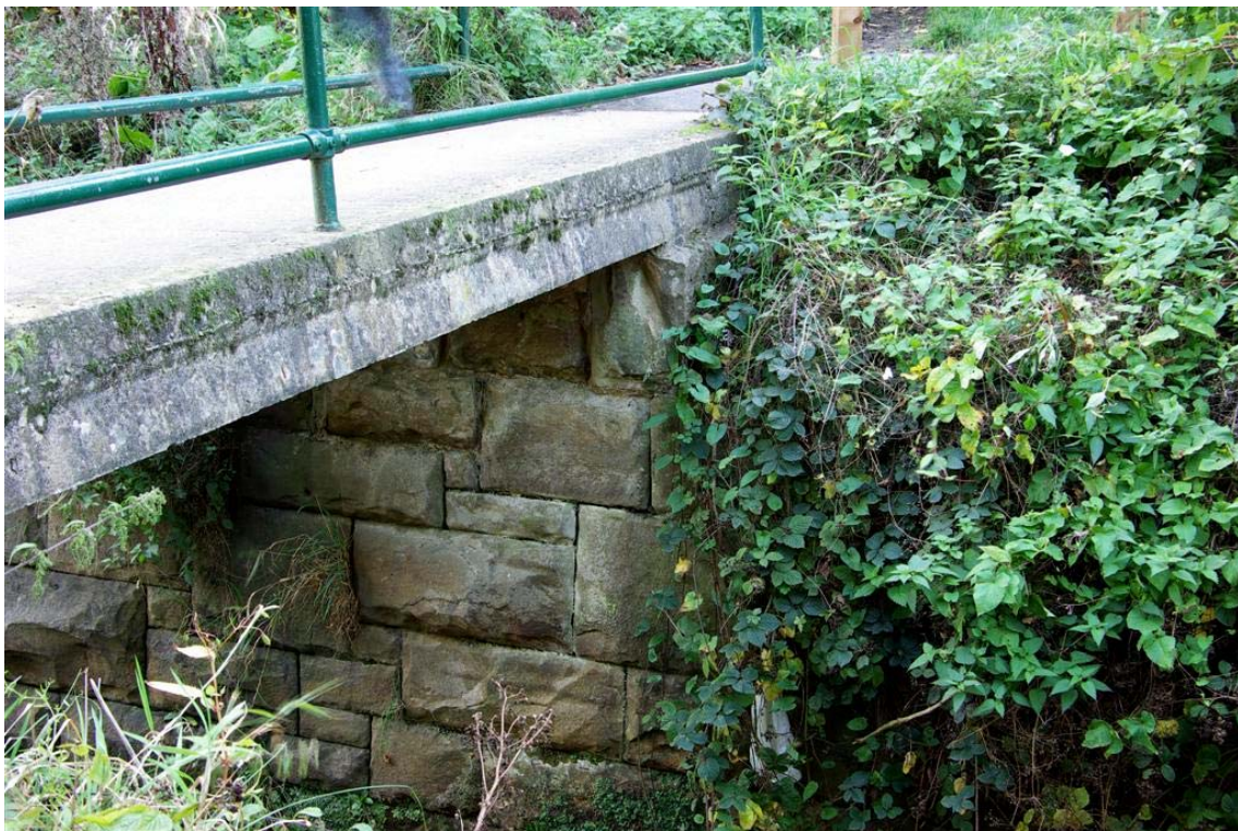
Plate 14: Possible former bridge footings and abutment
