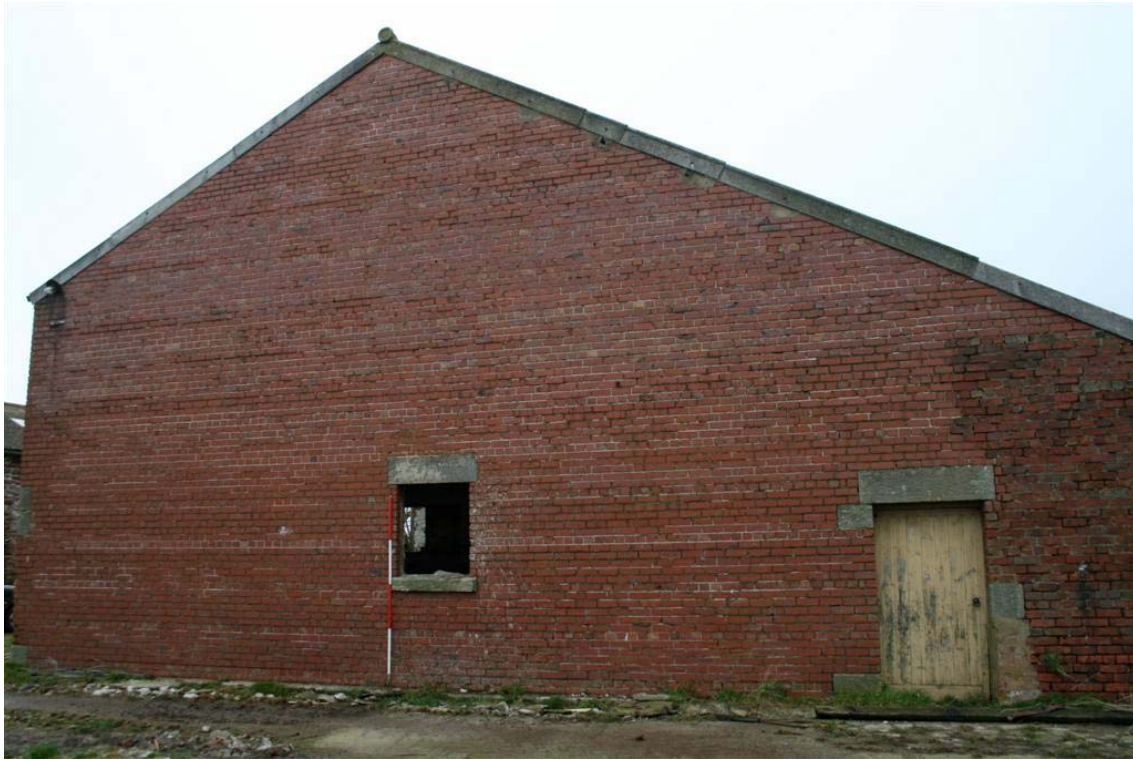
Plate 11: South elevation of Barn B
