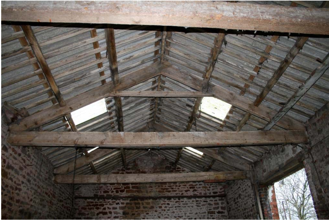
Plate 3: Roof truss in Barn A
