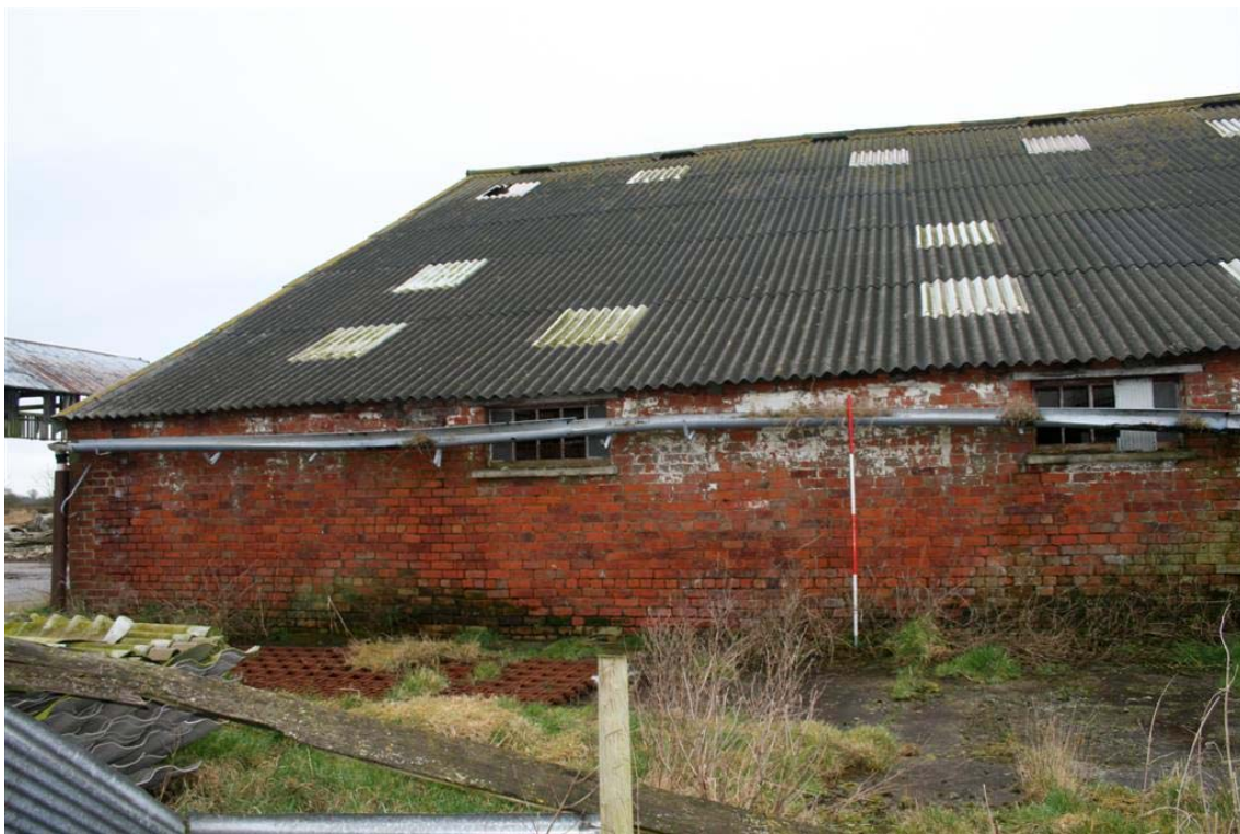
Plate 12: East elevation of Barn B
