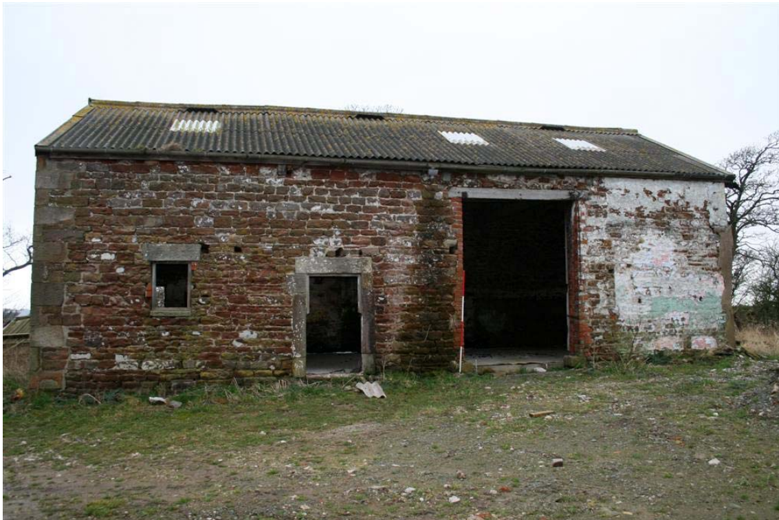
Plate 2: East-facing elevation of Barn A
