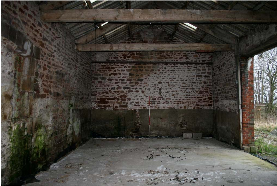
Plate 13: Internal view of Barn A
