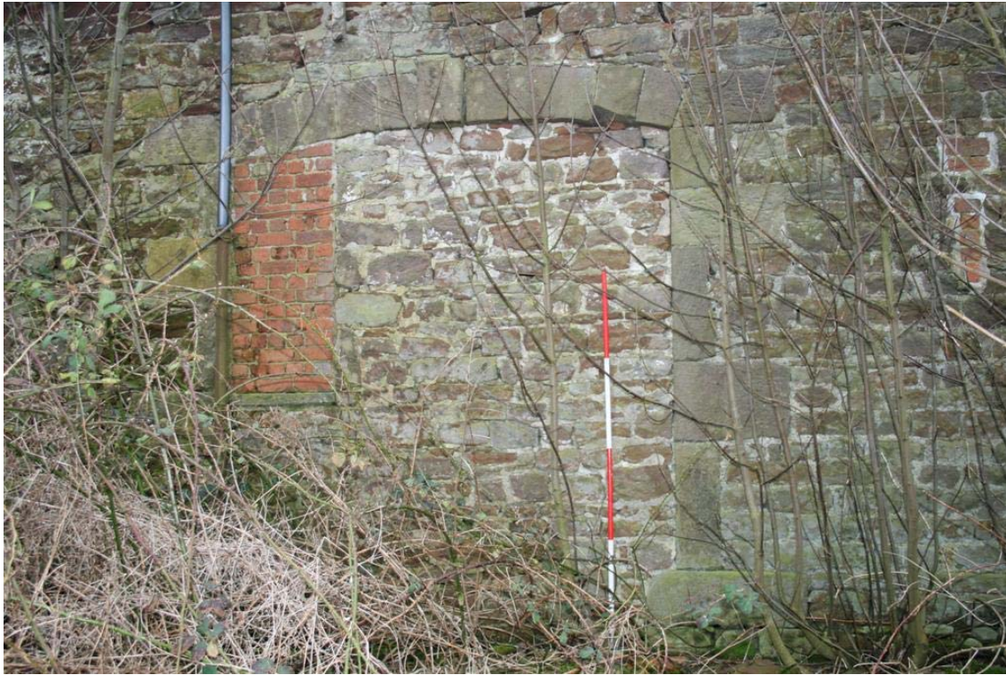
Plate 5: Blocked door and window on the west facing elevation of Barn A
