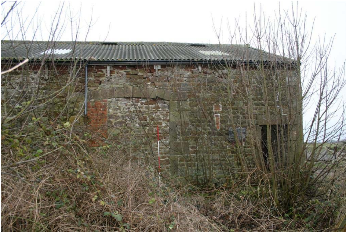
Plate 1: West-facing elevation of Barn A and the farmhouse
