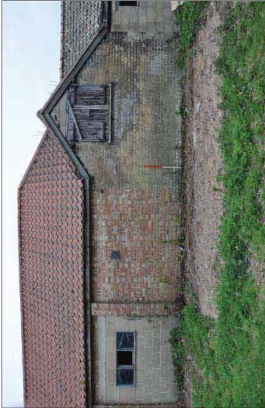
Plate 49: Building 16 showing incorporation of the 19th century range.
