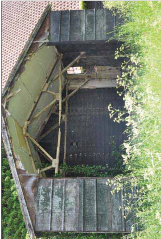
Plate 46: Internal structure of annexe on the west side of the barn
