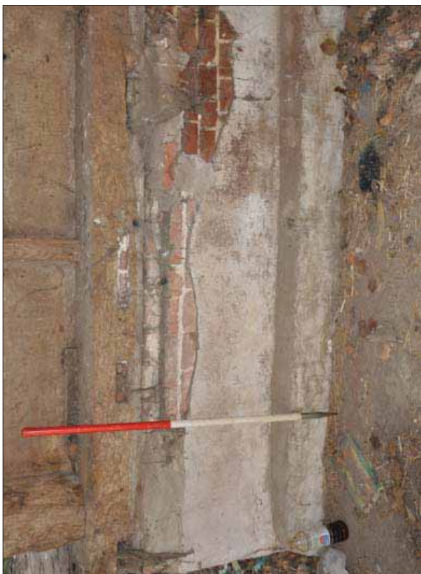
Plate 26: Detail of brick partition
