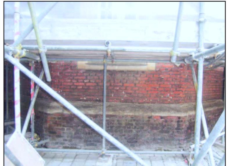
Plate 8: Type T brickwork on plinth
