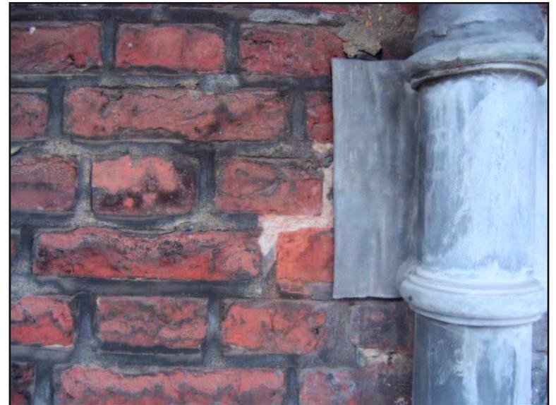
Plate 12: Red wash on bedding mortar, face 5
