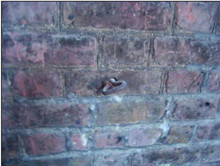
Plate 3: Type I Wren brickwork on face 1
