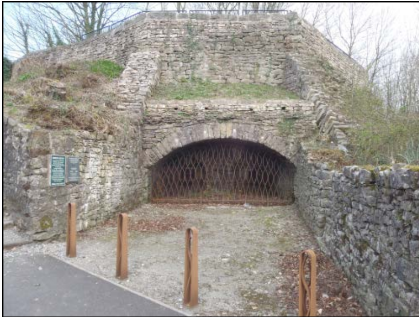
Plate 4: View of the lower part of the surviving lime kiln at Kendal Fell
