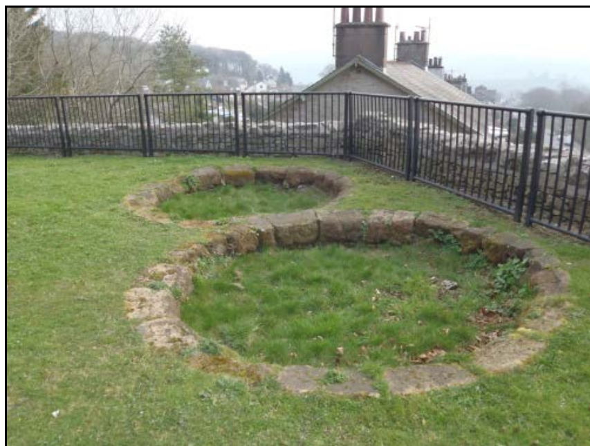
Plate 5: View of the upper part of the kiln pots from the charging platform of the surviving lime kiln at Kendal Fell
