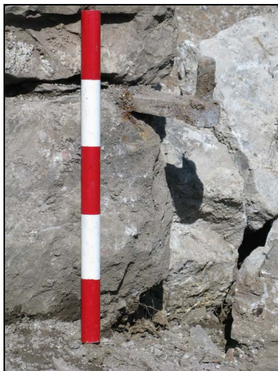
Plate 14: Hinge or lintel in wall 8, looking north-east
