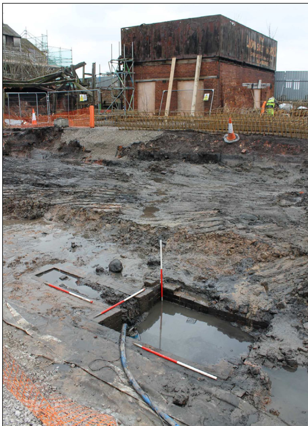
Plate 9: Brick flywheel pit uncovered during groundworks, looking north
