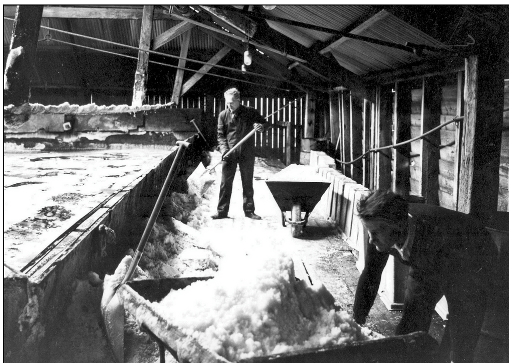
Plate 2: Removing salt crystals from the evaporating pan at Lion Salt Works
