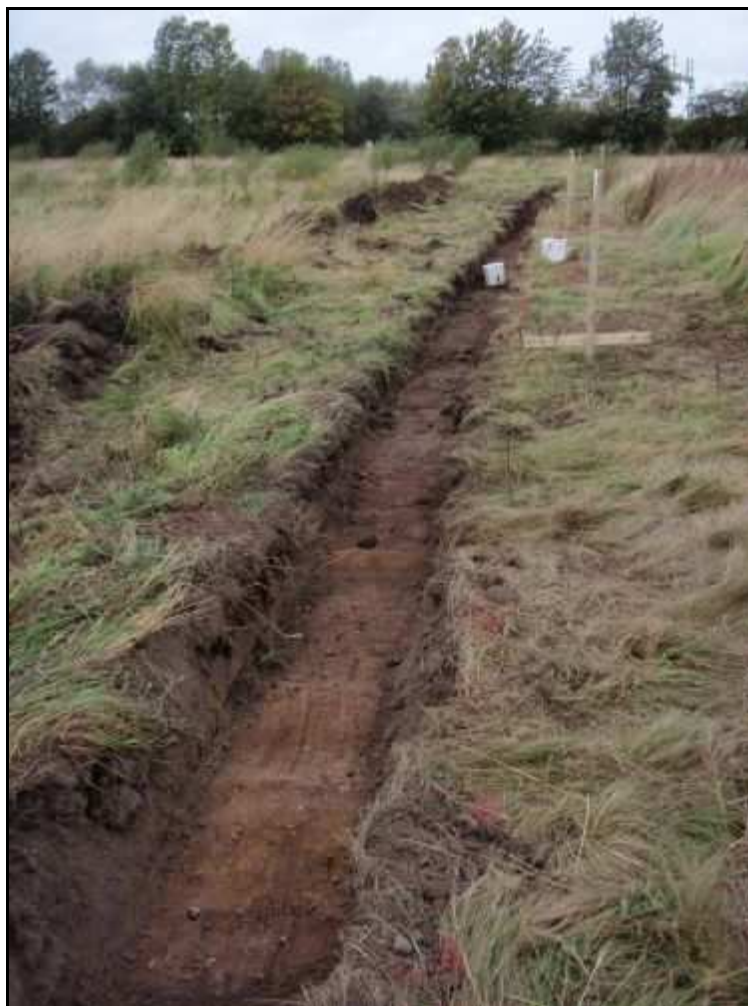
Plate 1: Example of drainage trench to the south of the railway, looking north
