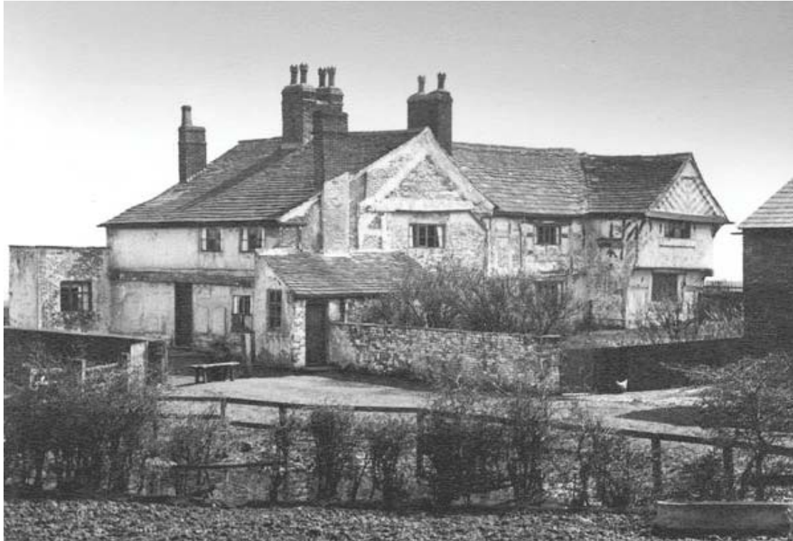
Plate 12: Wharton Hall; timber-framed building showing two cross-wings and central range c 1939
