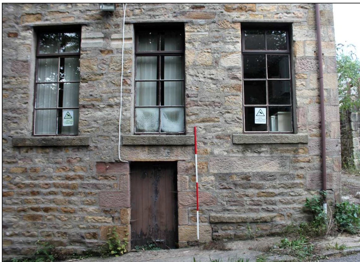
Plate 12: The first-floor windows and cast-iron lintels in the southern façade
