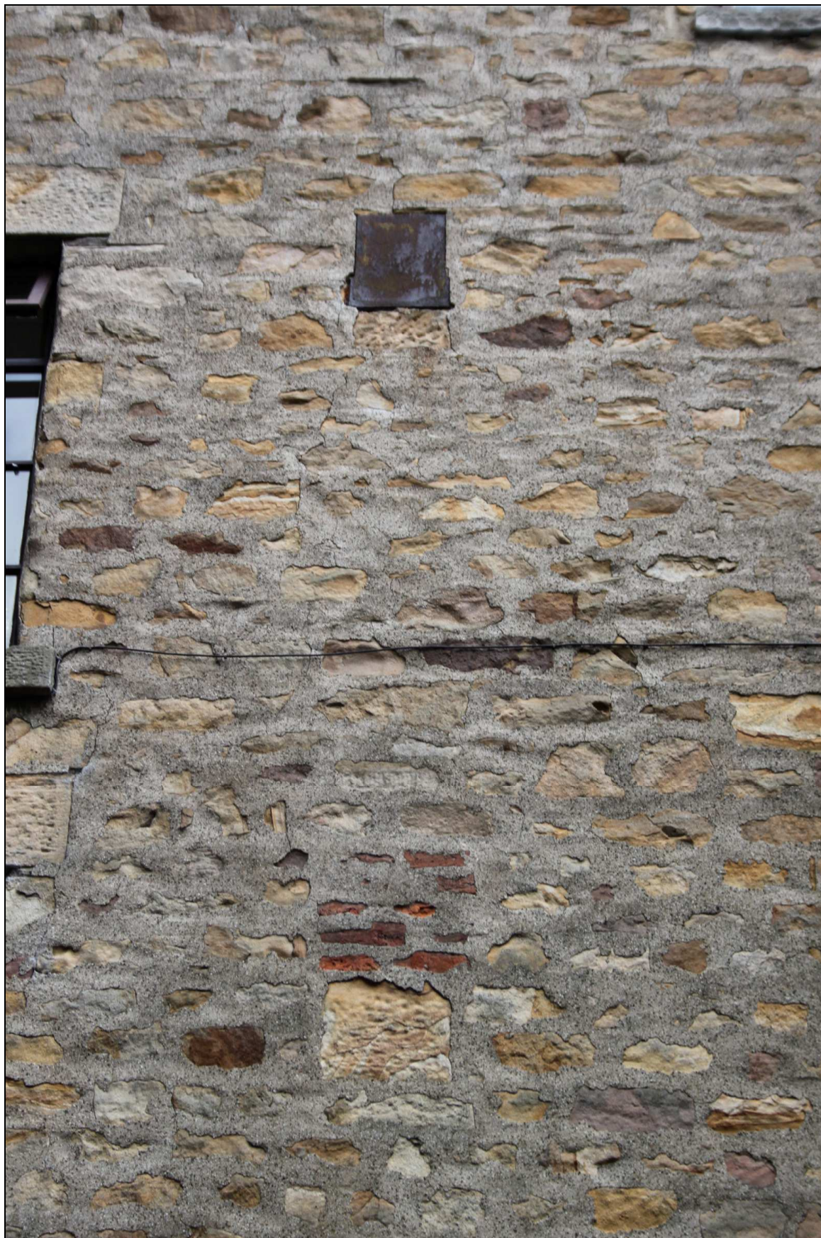
Plate 6: Brick blocking above a stone corbel at first-floor level in the west elevation of the building
