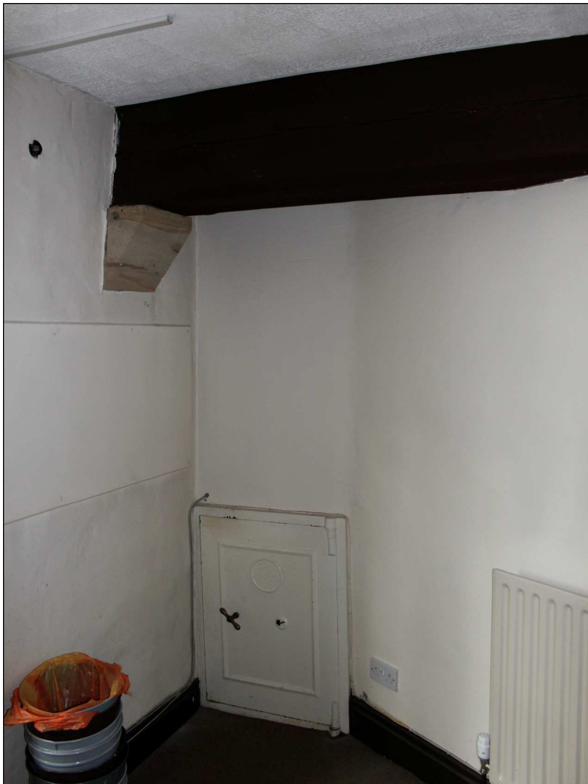
Plate 22: Ceiling beam on first floor supported on dressed, angled sandstone corbel, above cast-iron safe
