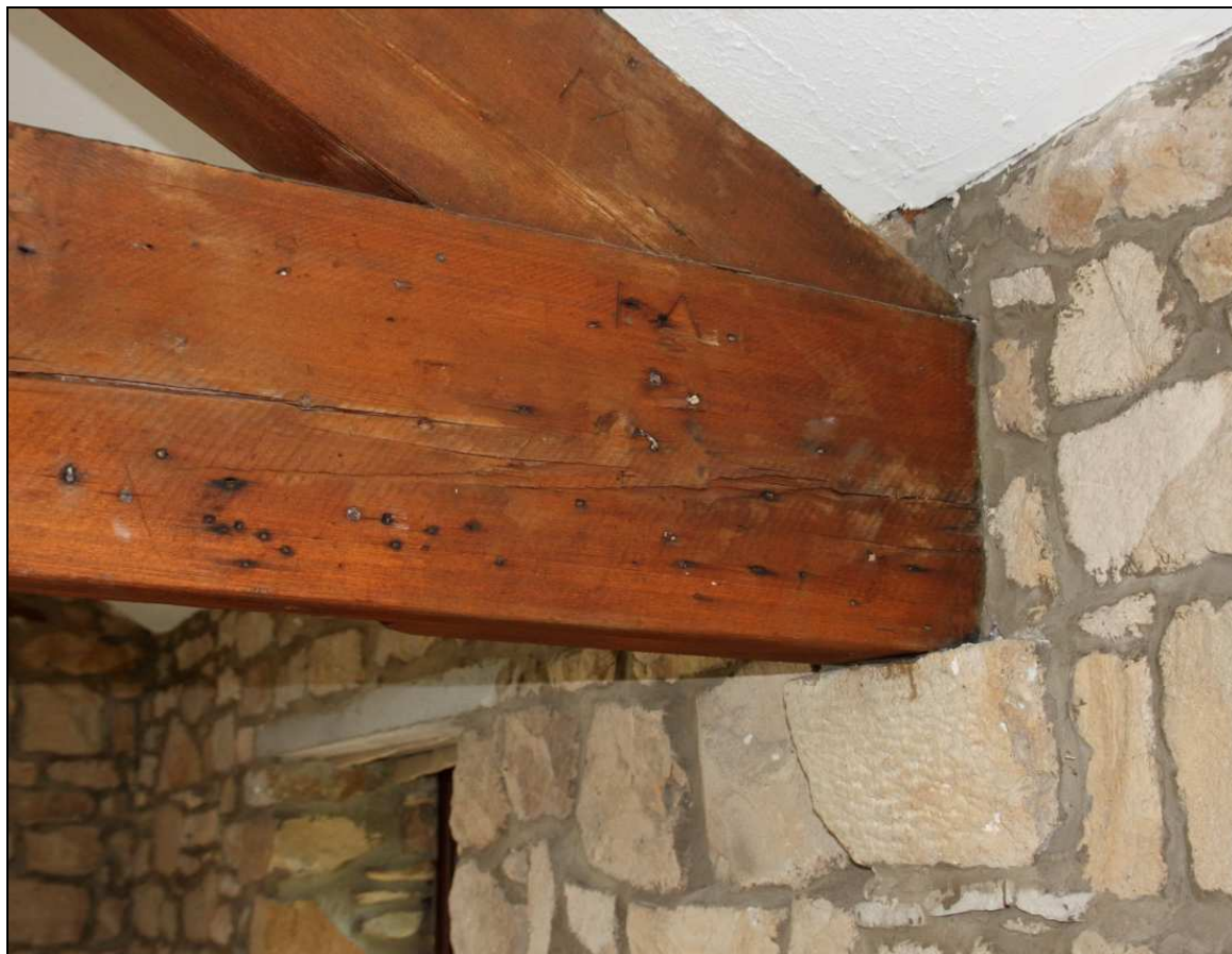
Plate 27: Detail of the timber beam and stone corbel on the third floor
