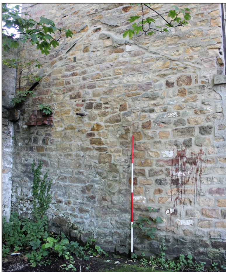
Plate 8: Wall scar at the northern end of the western façade
