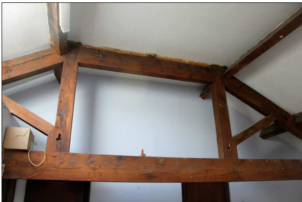
Plate 28: One of the three queen-post trusses supporting the roof
