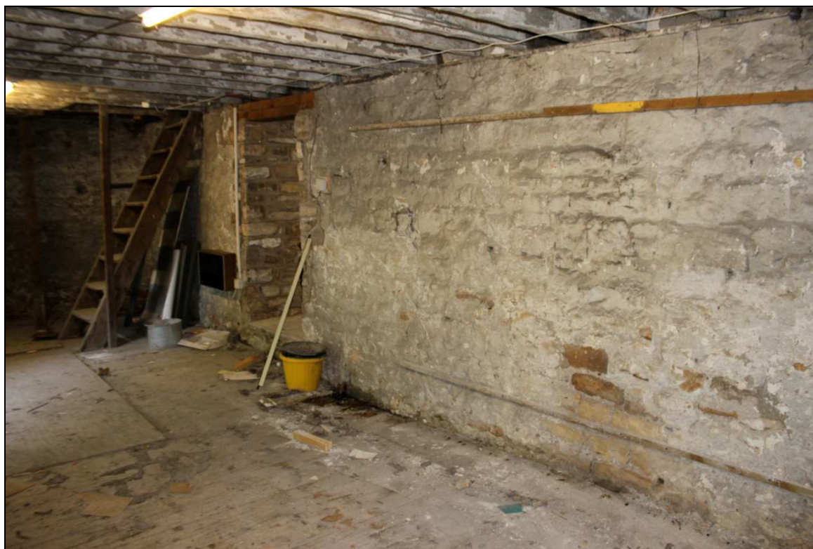
Plate 18: The western room on the ground floor, showing the central spine wall and inserted doorway
