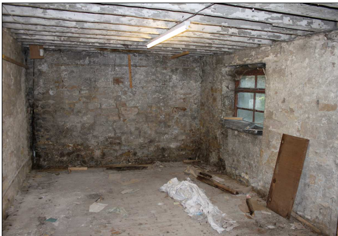
Plate 17: The southern end of the western room on the ground floor, showing window in blocked doorway
