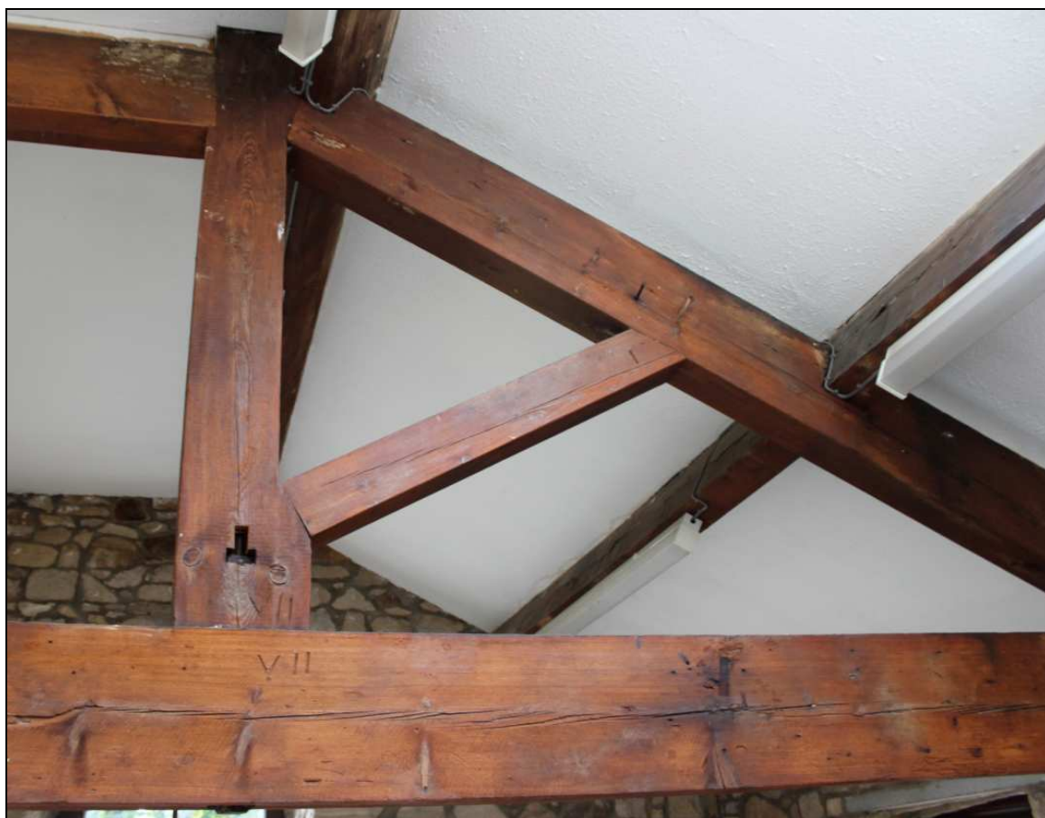
Plate 29: King ties and carpenters' assembly marks on the roof truss
