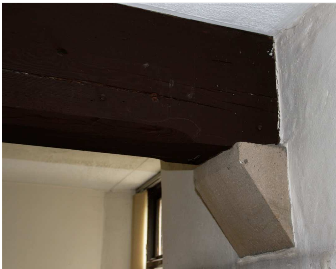
Plate 23: Detail of angled sandstone corbel set into the east wall on the first floor
