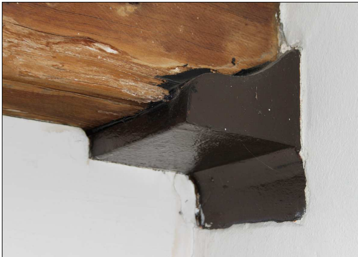
Plate 25: Detail of cast-iron bracket supporting the ceiling beam on the second floor
