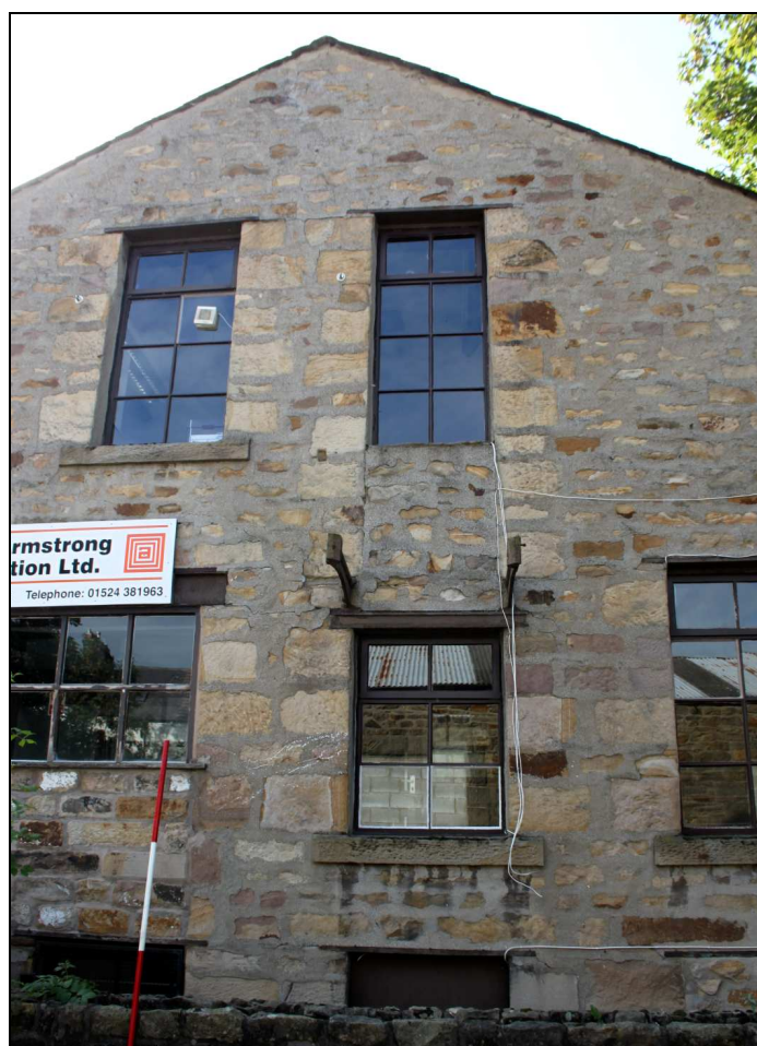
Plate 15: The remodelled loading loop in the northern facade
