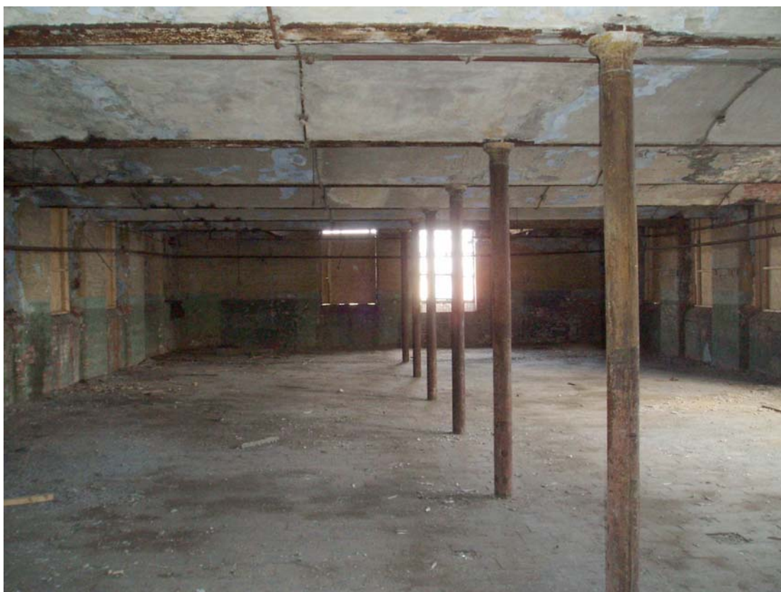
Plate 4: View across the top floor of the West Wing Mill, showing brick-vaulted ceiling and single row of cast-iron columns
