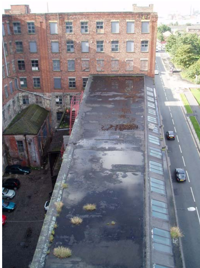
Plate 14: View along the roof of the Bradford Road block, showing inclined sky-lights
