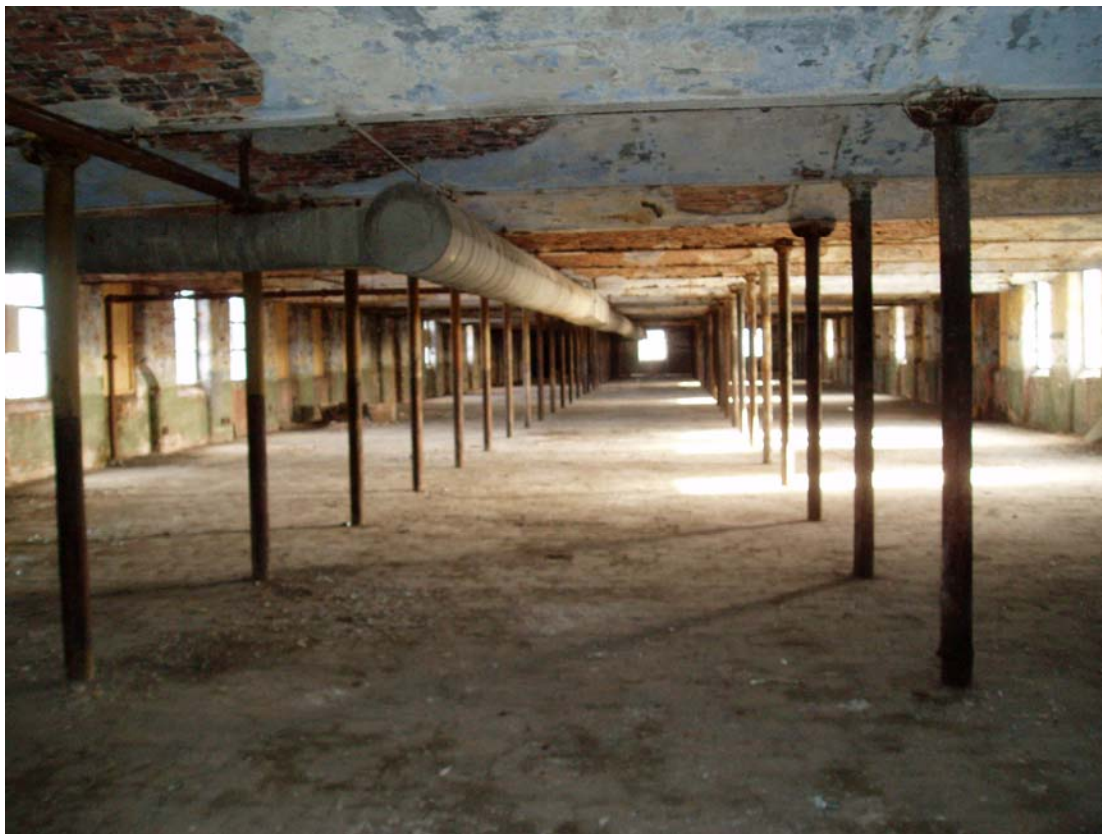
Plate 3: The top floor of the main spinning block, showing the fireproof construction
