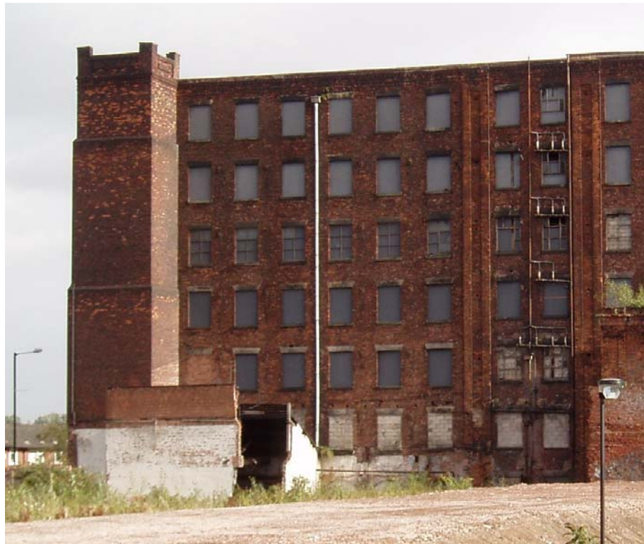
Plate 12: west-facing elevation of the mill, showing the late 19 th century dust flue
