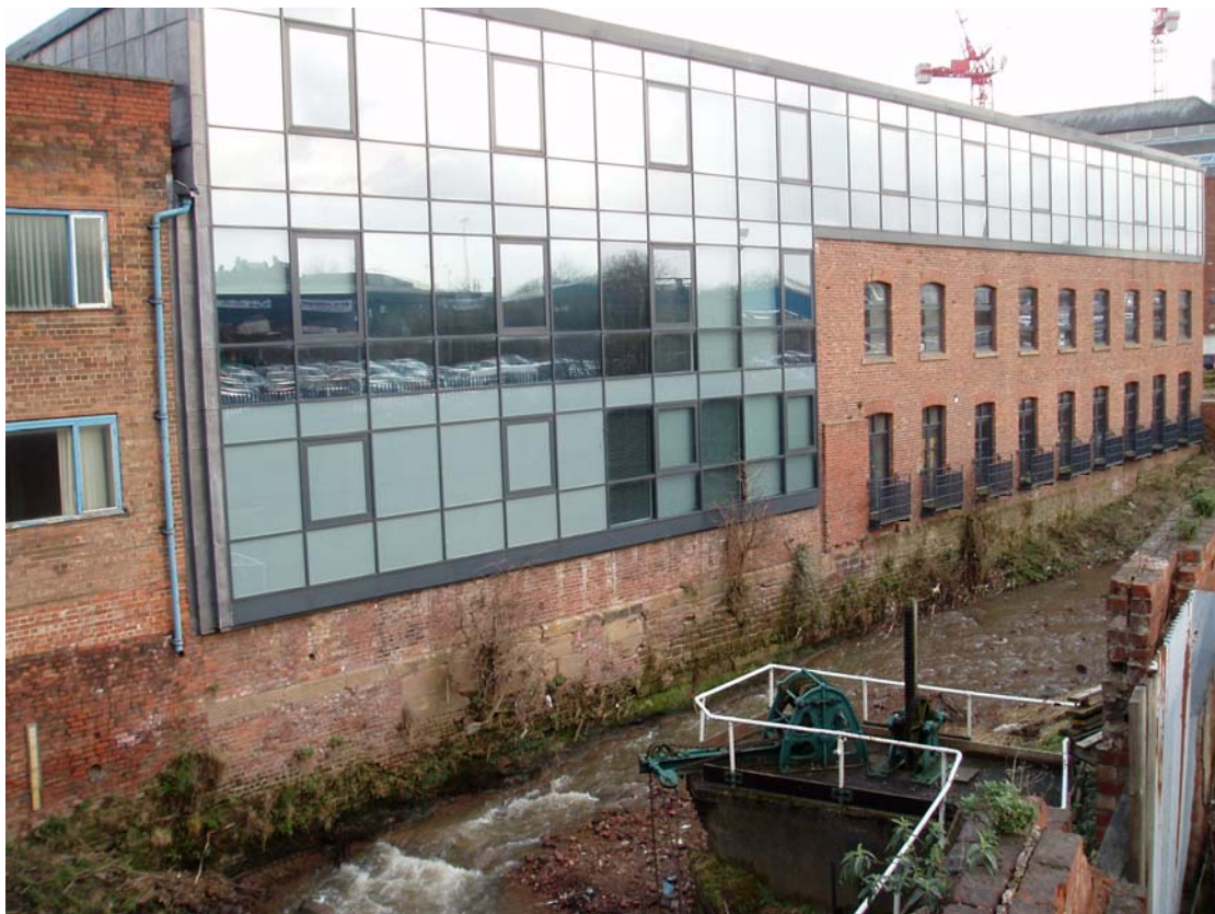
Plate 4: The south-western elevation of the Knott Mill Bridge block and adjacent modern development, showing stone blocks surviving in the original foundations
