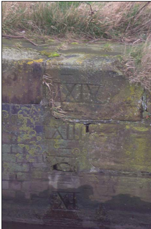
Plate 10: Detailed view of depth markers on the north-western end of Frodsham Lock (Site 22 ), looking north
