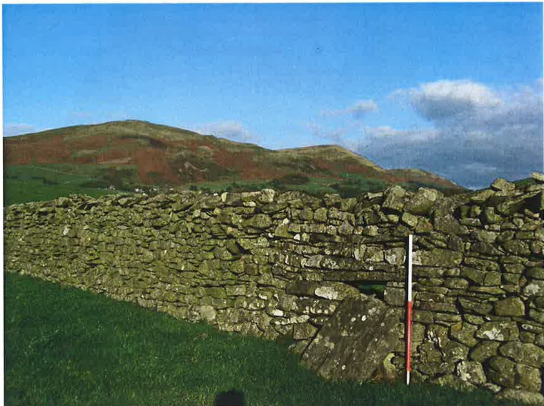
Plate 7: Sheet smoot looking north-east
