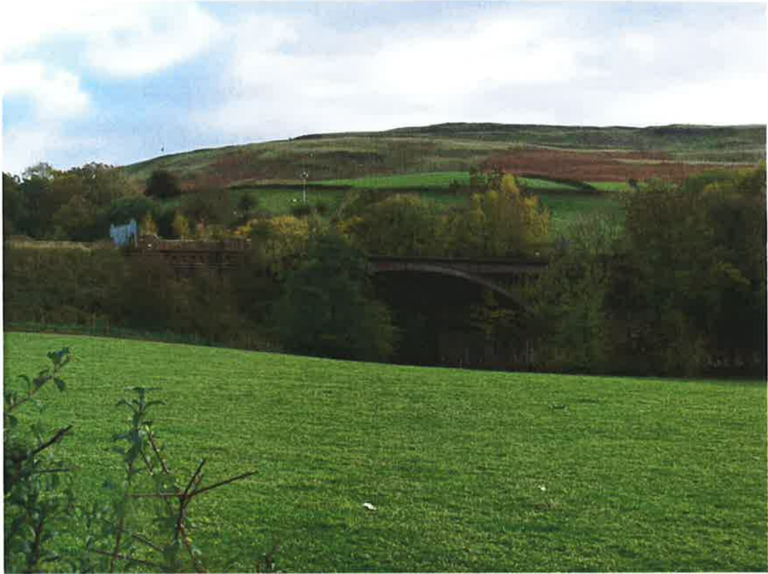
Plate 8: Rawthey Railway Bridge (Site 02), looking south
