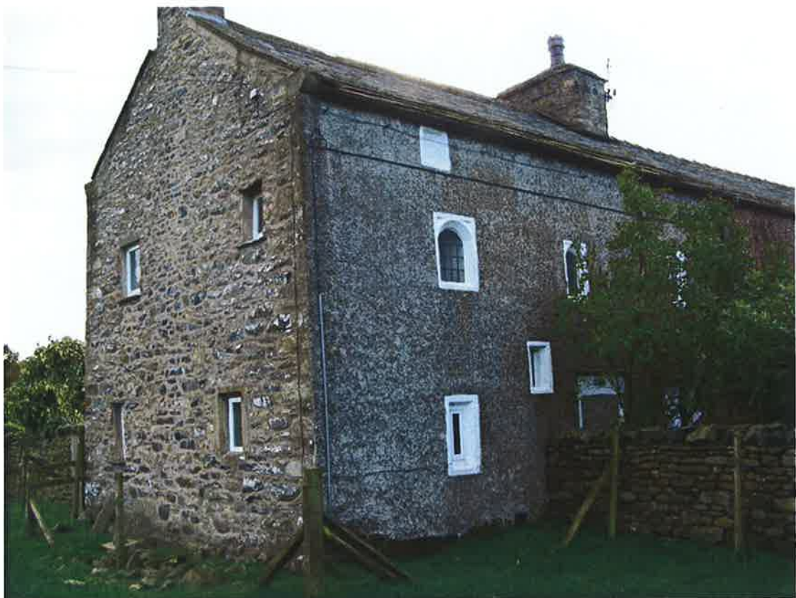
Plate 9: Low Brigflatts Farm looking south-west
