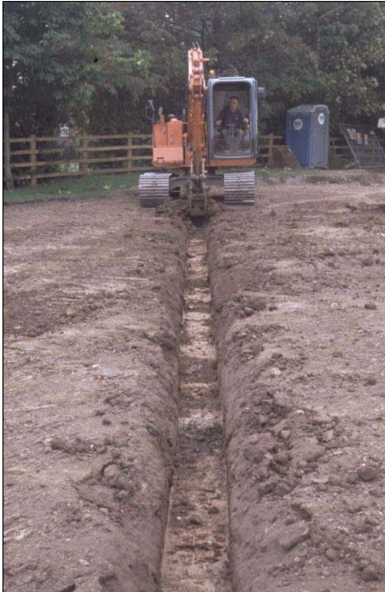
Plate 3: Excavation of field drain
