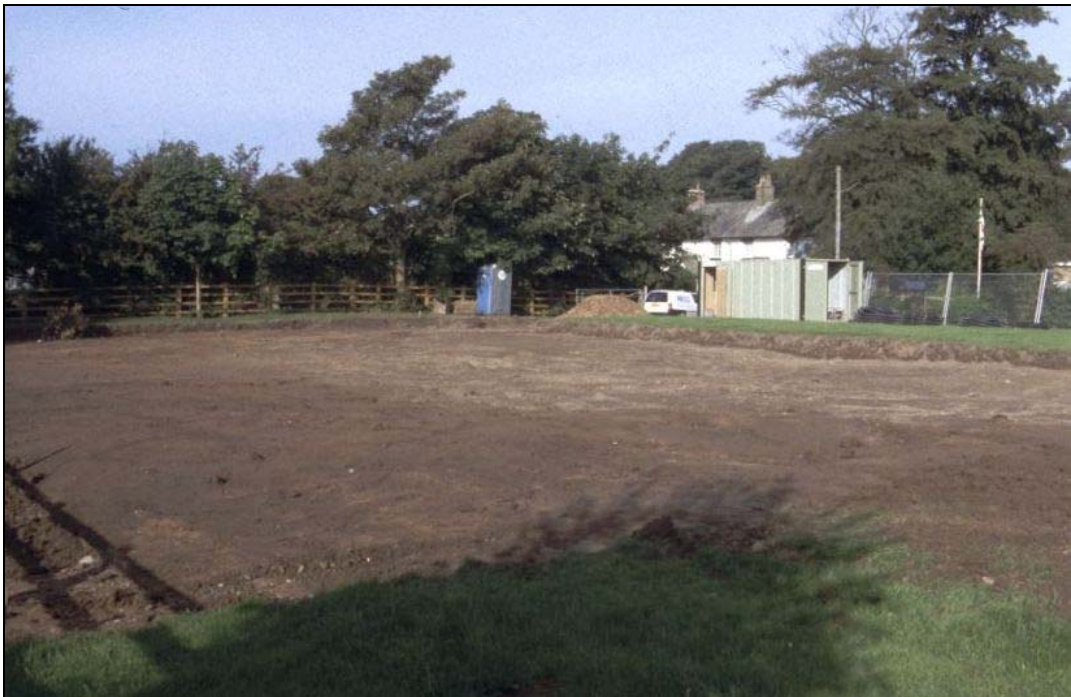
Plate 2: View of complete site topsoil stripped
