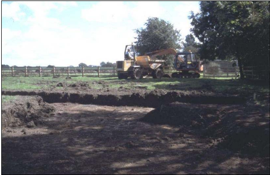
Plate 1: Topsoil stripping of site
