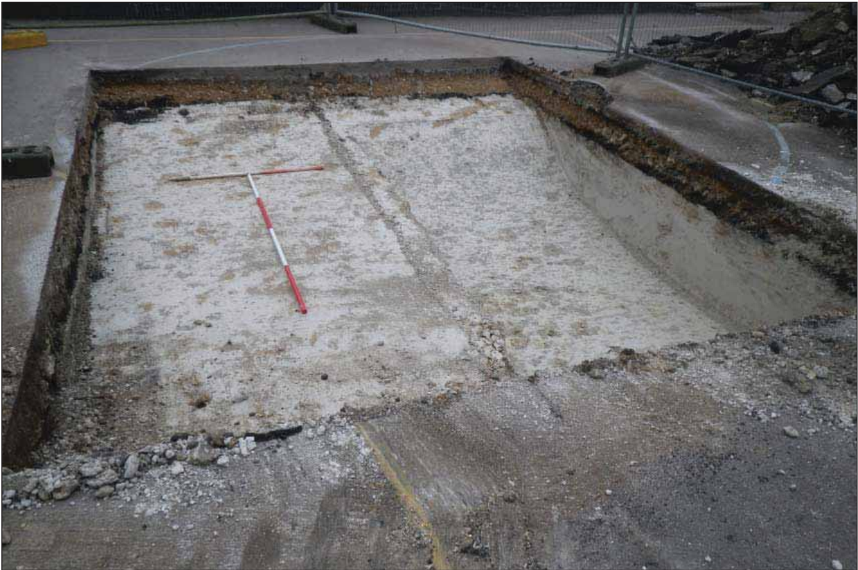
Plate 1: View of Trench 1 from the north
