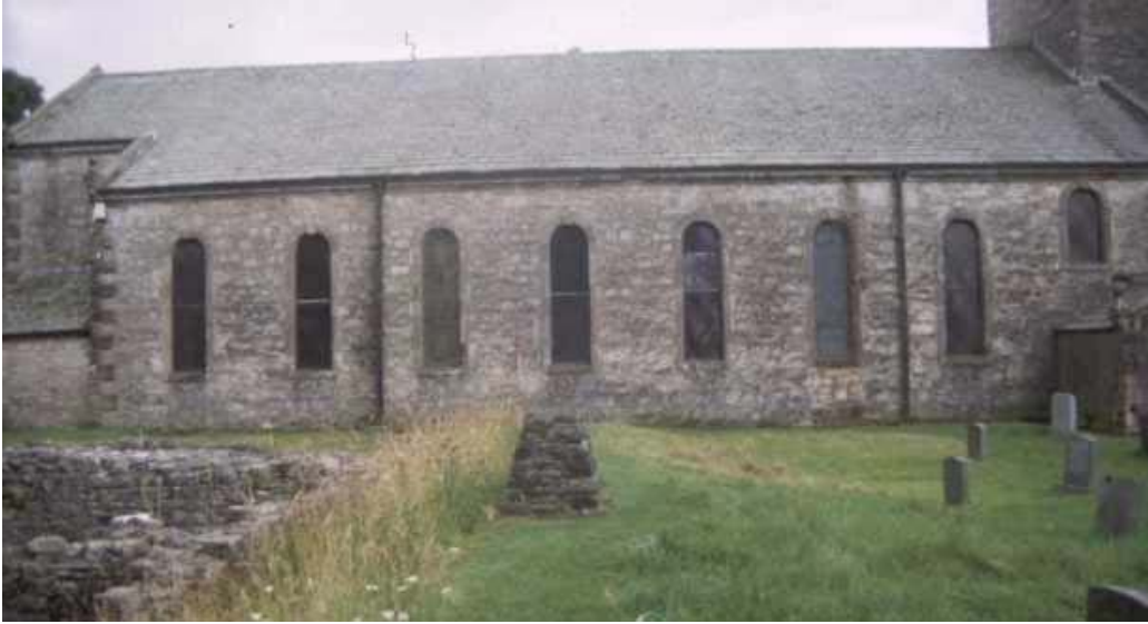
Plate 6: Rectified photograph of the north elevation
