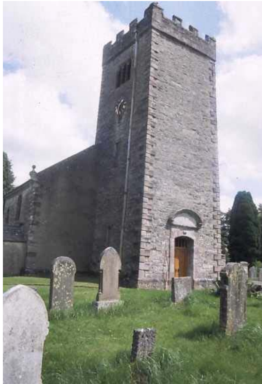
Plate 4: The tower, looking south-east
