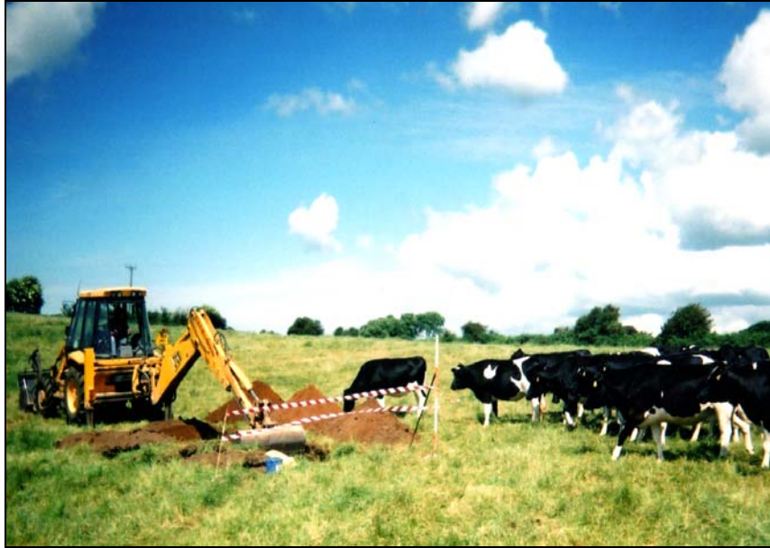
Plate 5: Excavation of Trench 4 in progress
