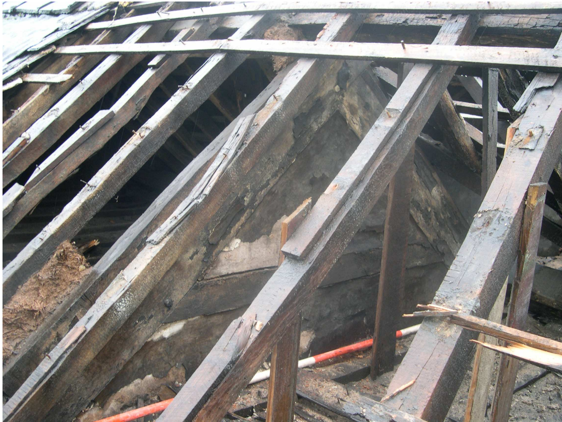
Plate 26: Daub above truss in roof space
