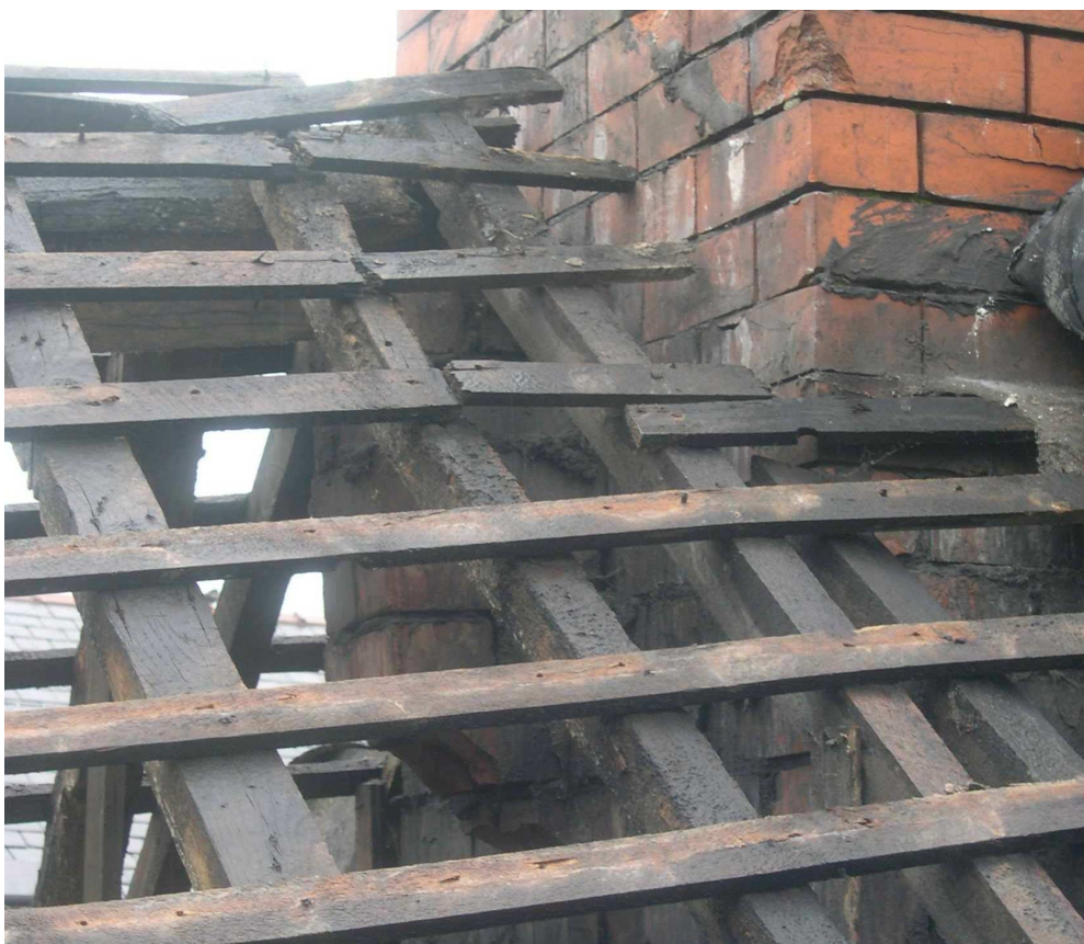
Plate 22: Brick corbel supporting northern end of ridge purlin
