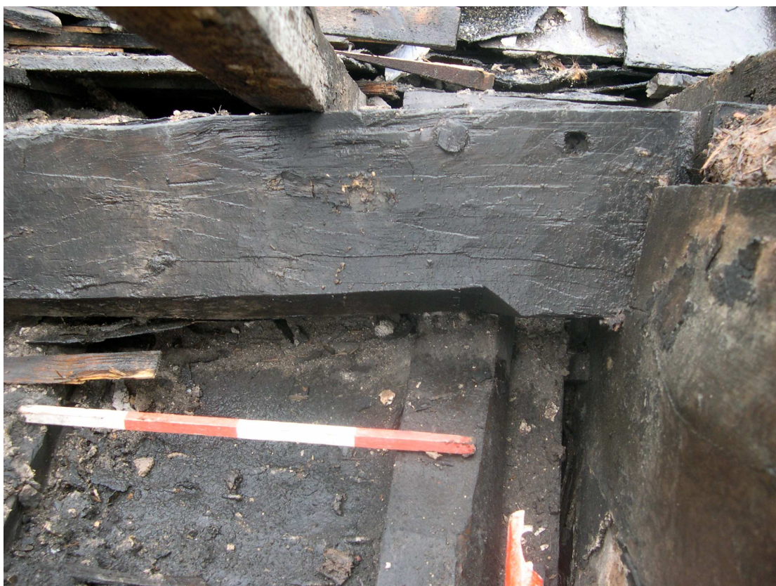
Plate 19: Stop chamfered purlin in roof space
