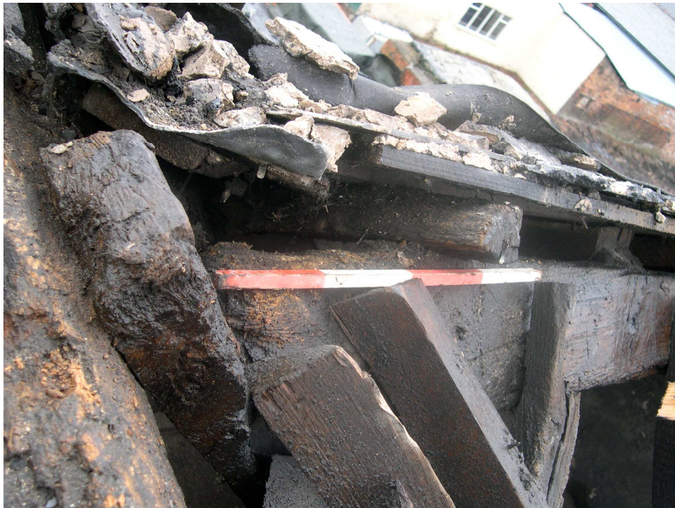
Plate 24: Junction of ridge purlins between main roof and south wing
