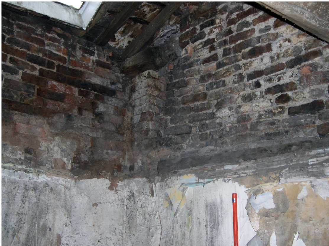
Plate 17: Early brickwork in east elevation of Room 8
