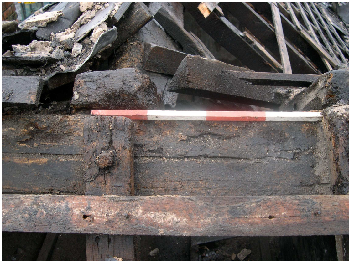
Plate 21: Timber peg through rafter into ridge purlin
