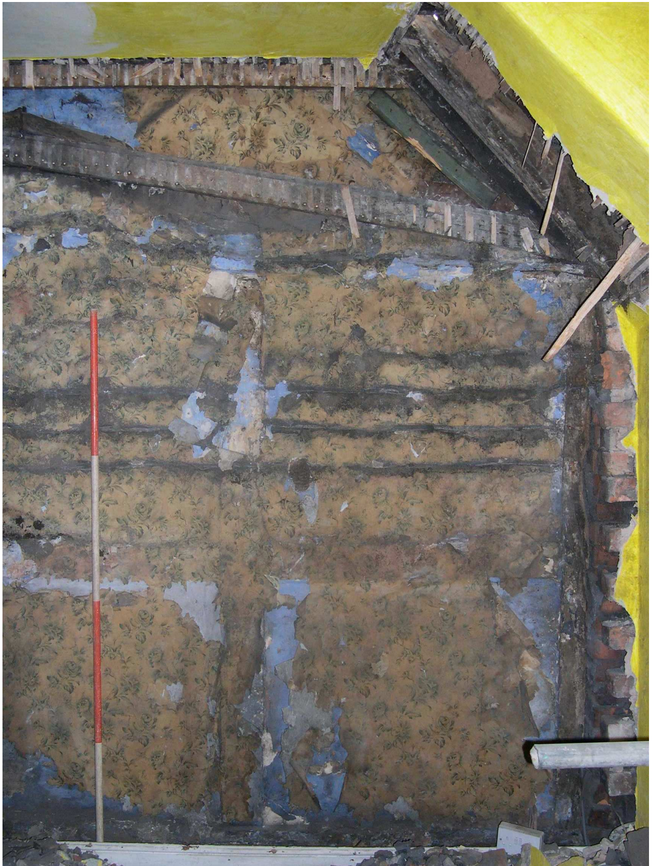
Plate 28: Wallpaper covering timber-framed cross-wall in Room 6
