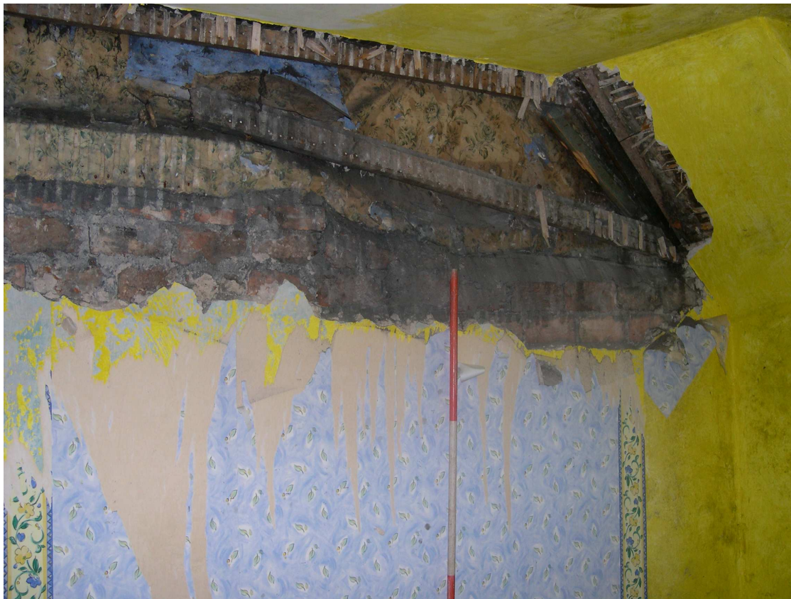
Plate 27: Tie-beam and brick wall in Room 6
