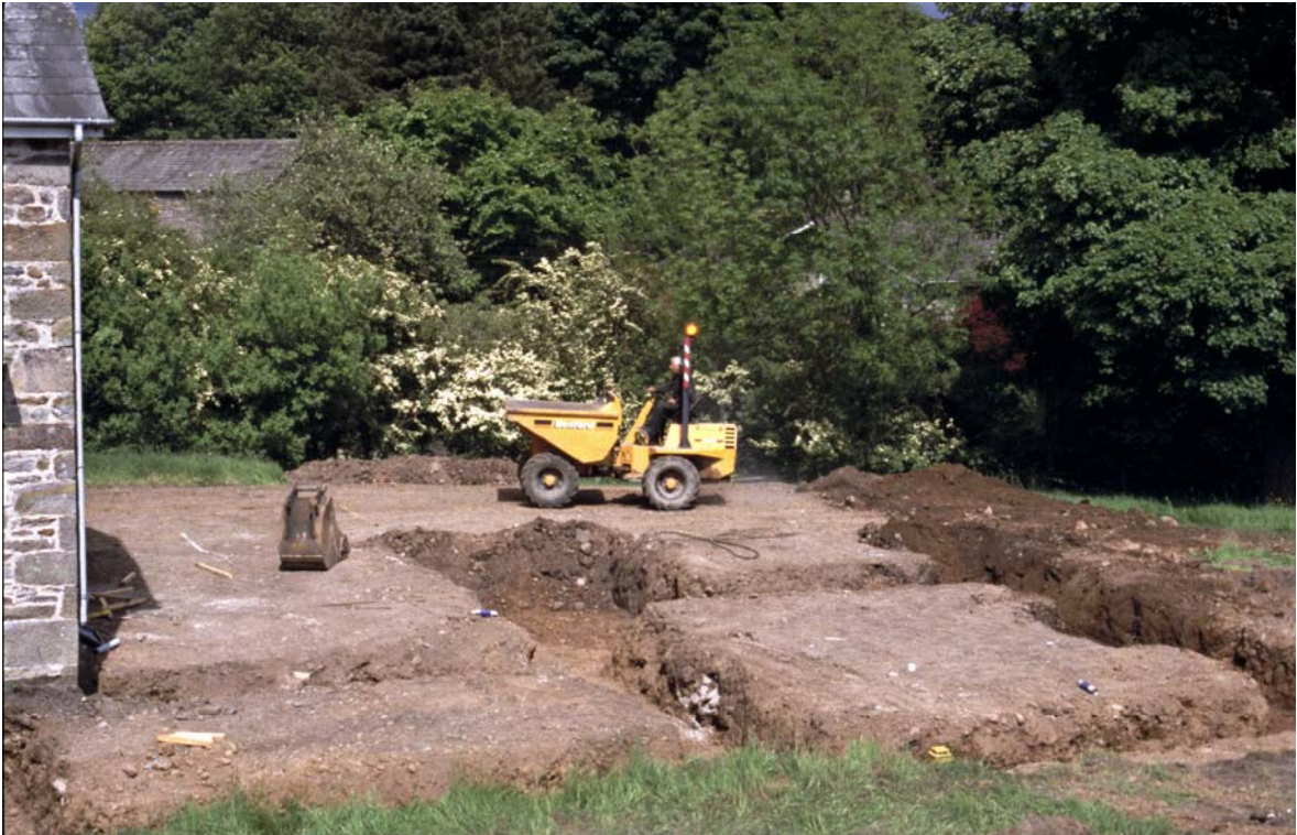
Plate 1: View of total stripped area and foundation trenches
