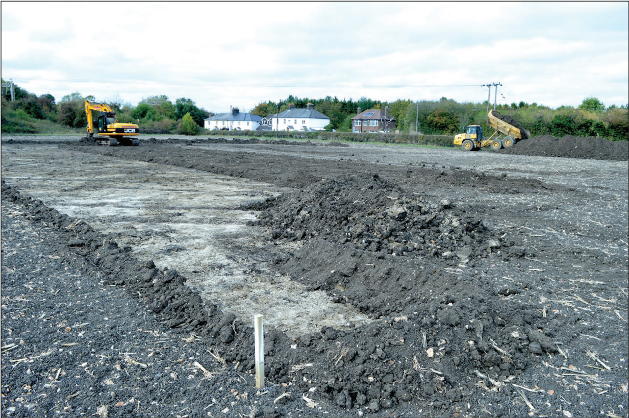
Plate 1: Machine stripping being undertaken on site, looking northwest
