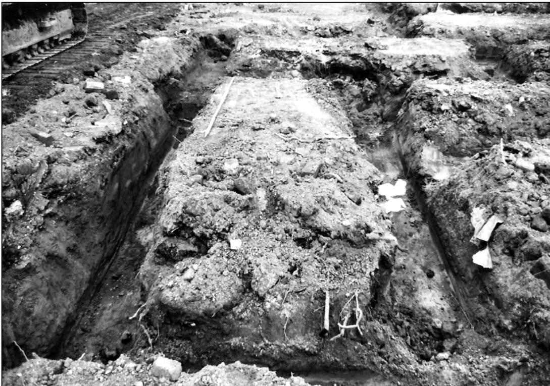
Plate 13: Excavation of slot trenches for house footings under permanent presence watching brief
