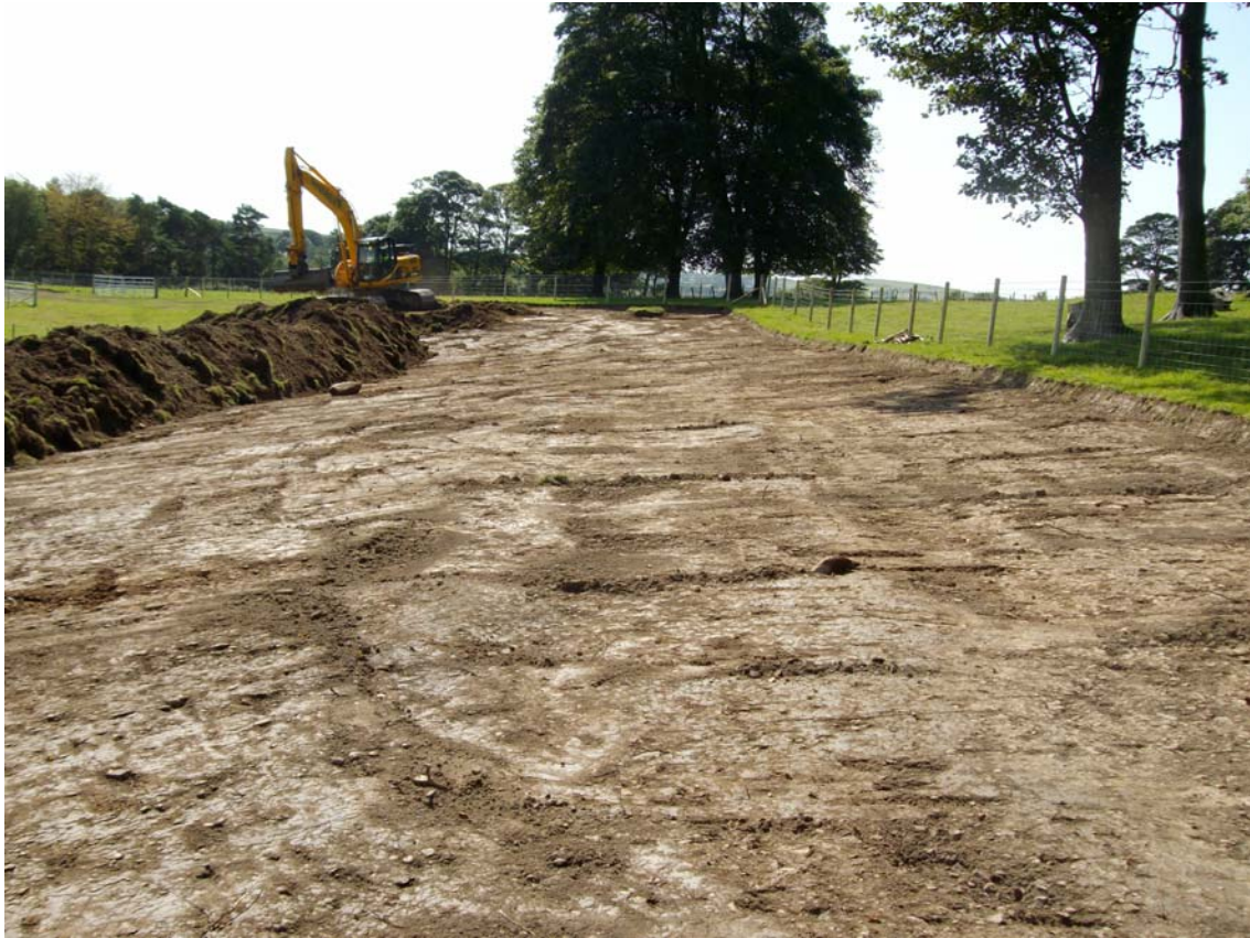
Plate 1: General shot of the easement during topsoil stripping activities
