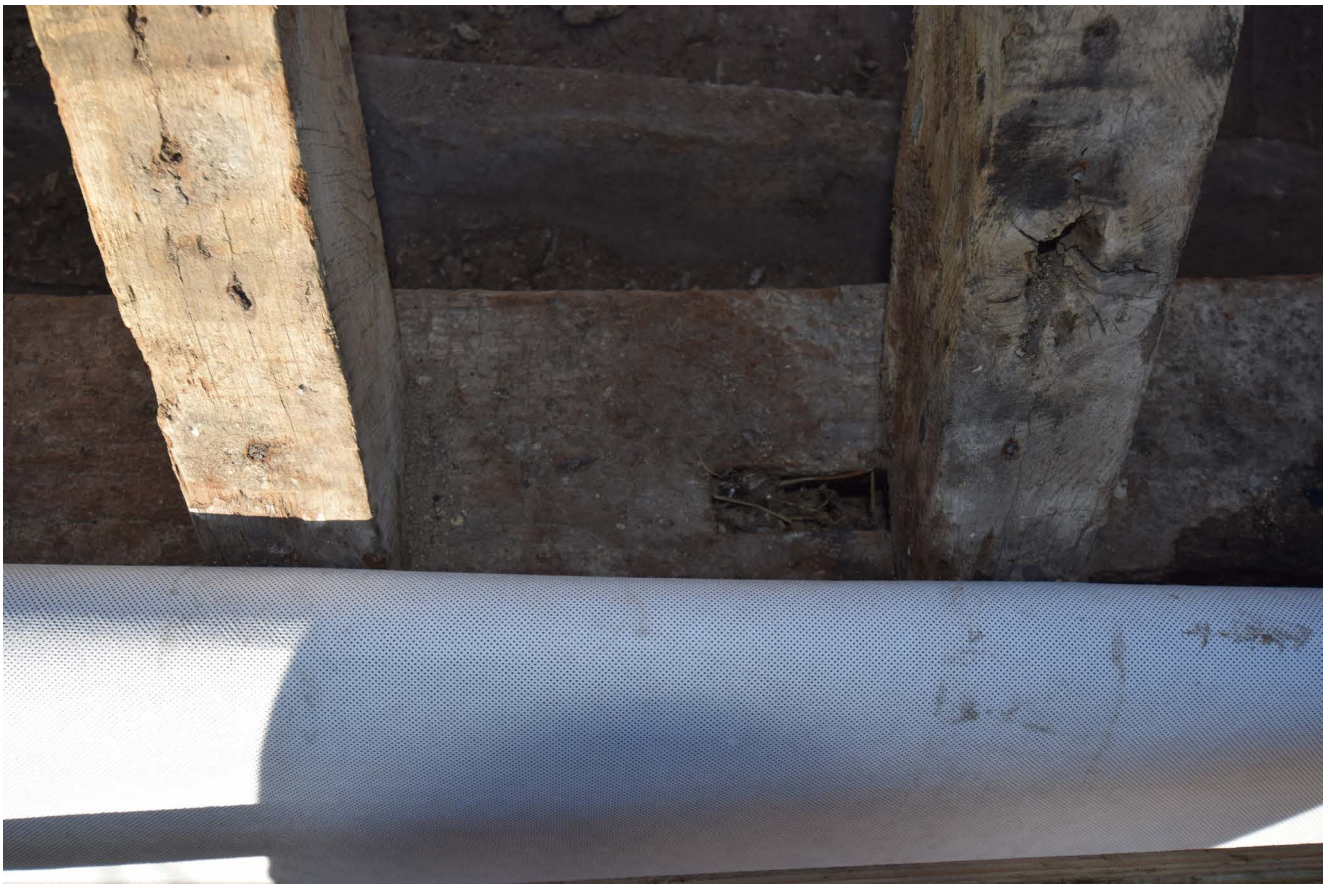
Plate 37: Reused timber used as a wallplate in the southern return of the northernmost wing
