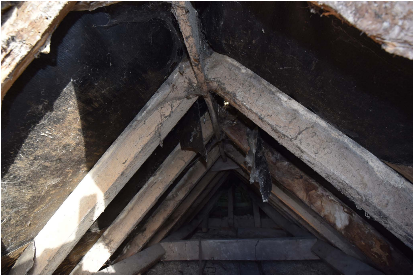
Plate 46: The roof structure of the northernmost central bay
