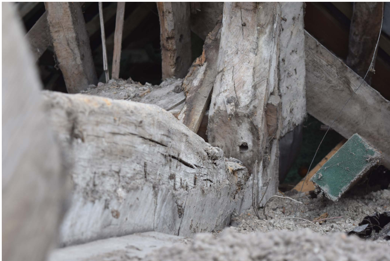
Plate 30: Damage or rework to 14th-century timbers, southernmost join of rafter and tiebeam
