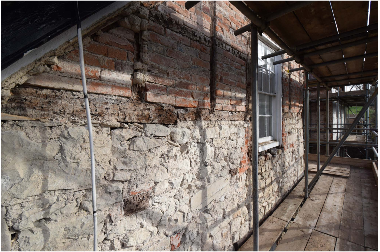
Plate 7: The stone and timber frame of the south west elevation of the northern wing
