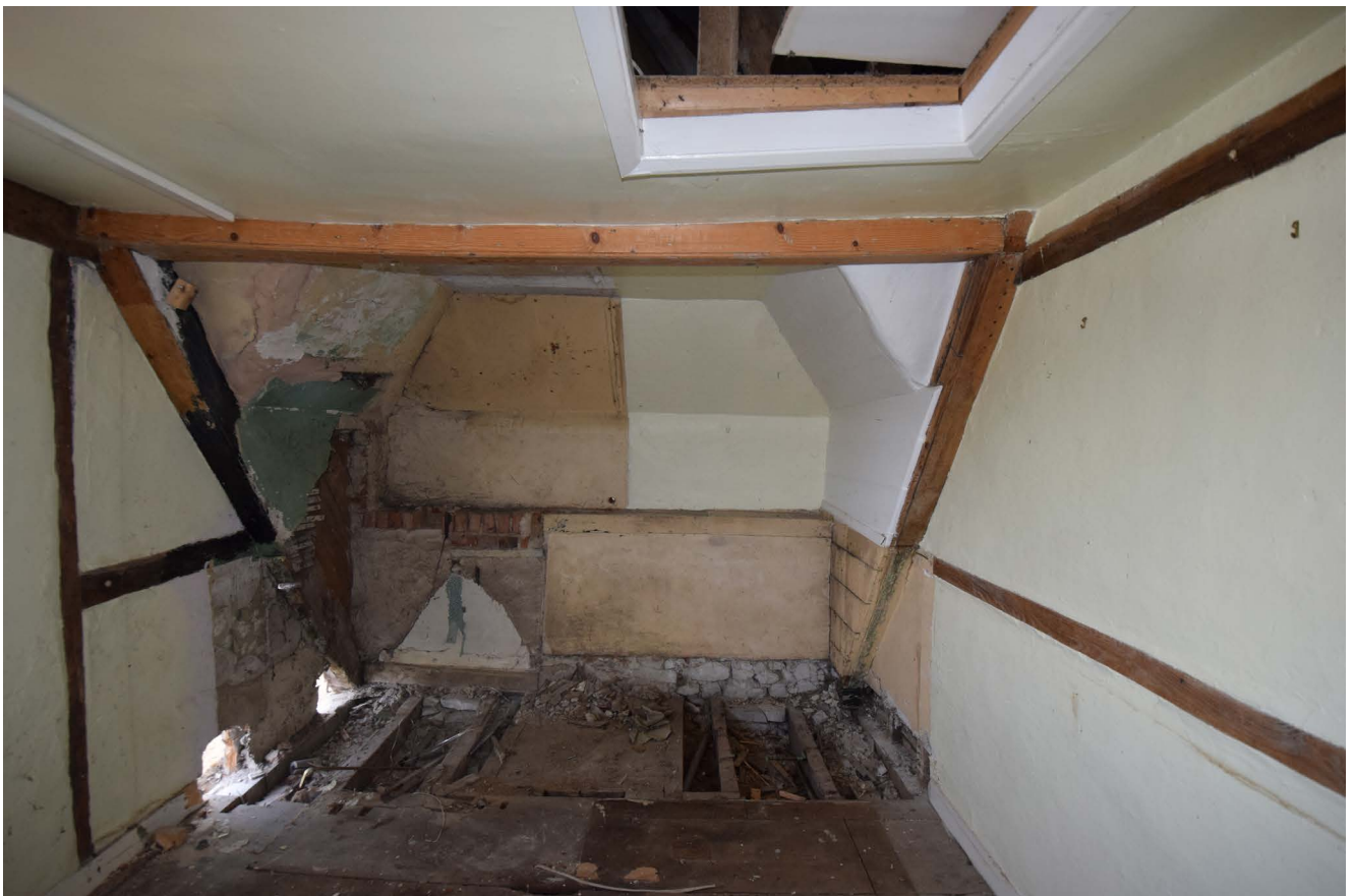
Plate 66: The visible brickwork and stonework in the south east wall of the second floor study
