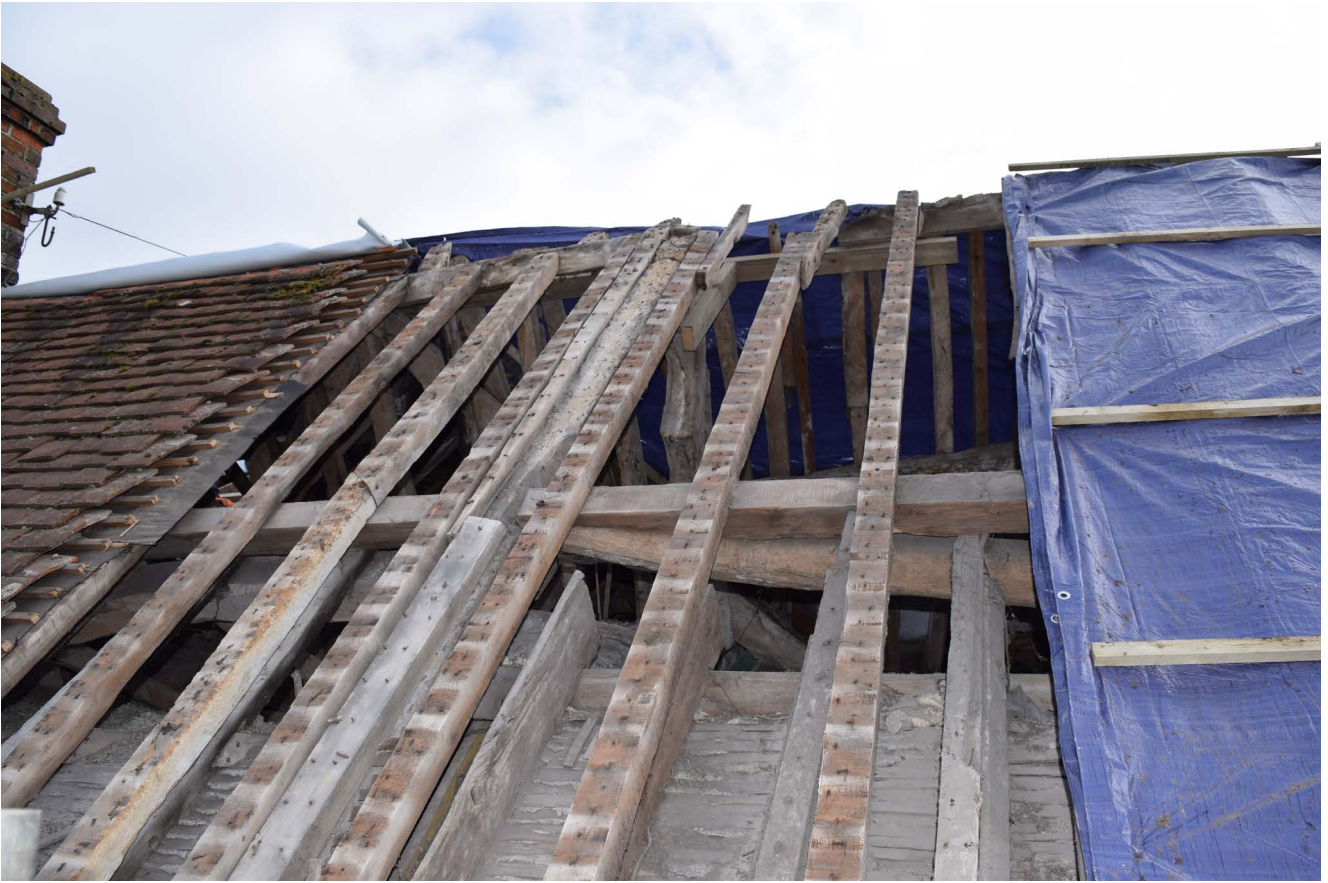
Plate 27: The 14th-century timbers and ceiling structures in the northernmost wing
