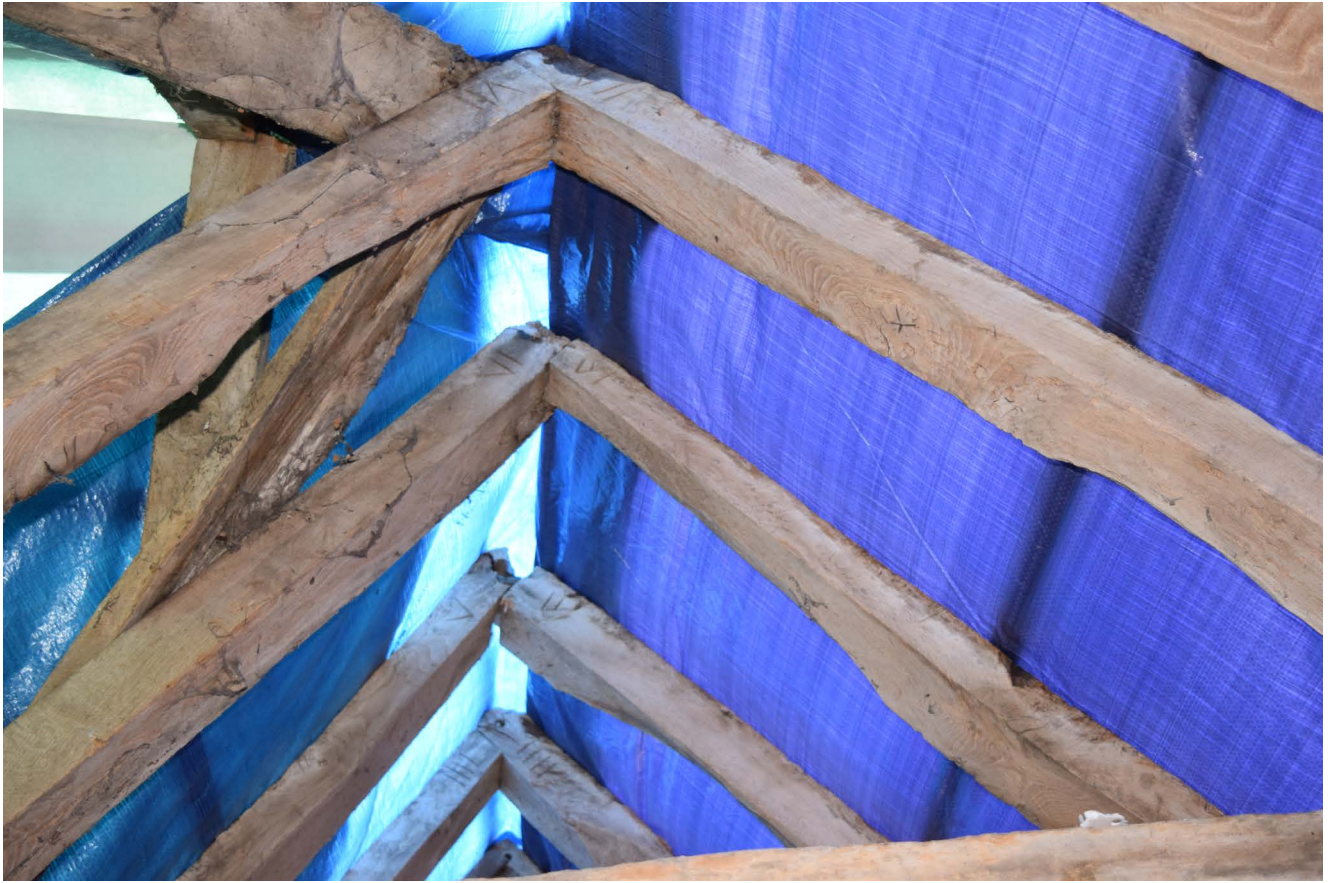
Plate 45: The joints and carpenters' marks in the rafters of the southernmost wing
