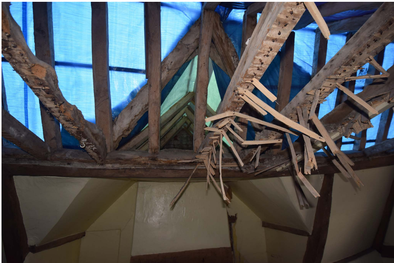
Plate 40: The roof structure of the link dormer of the southernmost wing
