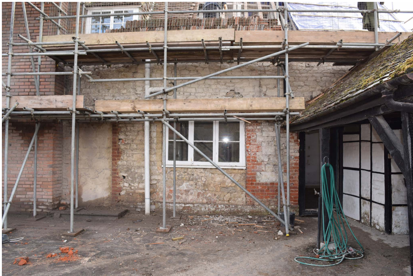
Plate 22: The south west end of the north west elevation after removal of the render
