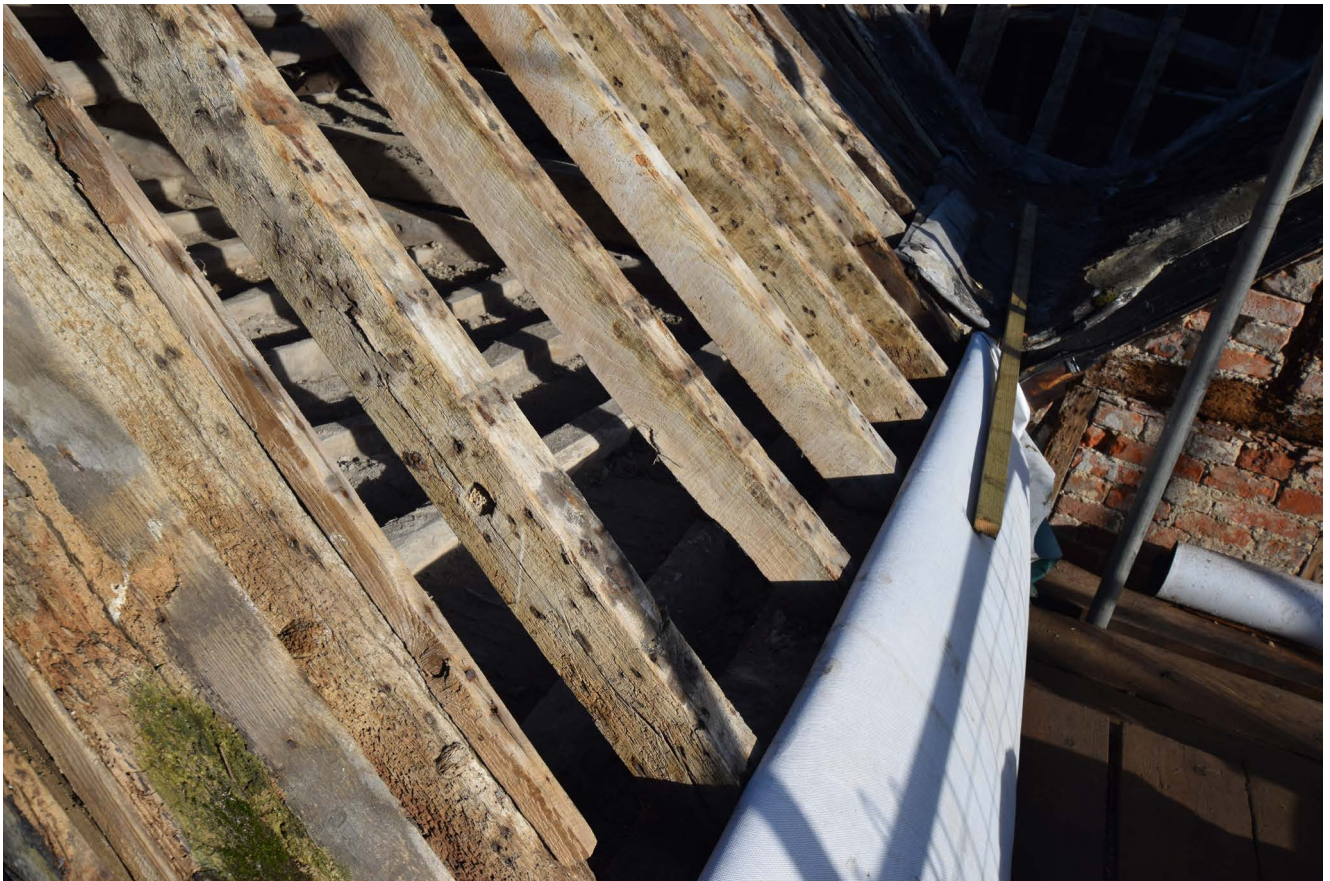
Plate 36: Reused rafters in the southernmost pitch of the northernmost wing
