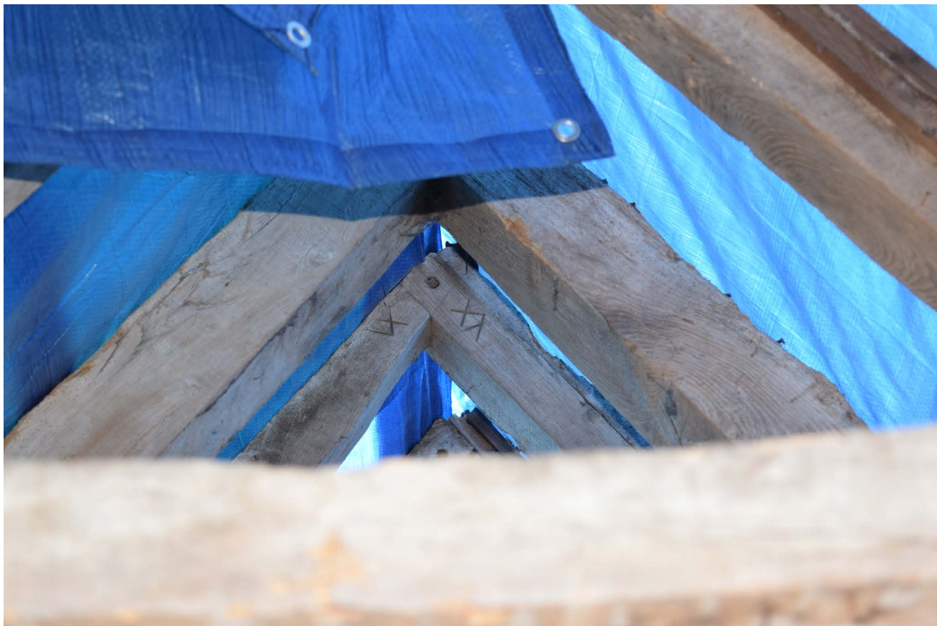
Plate 44: The joints and carpenters' marks in the rafters of the southernmost wing
