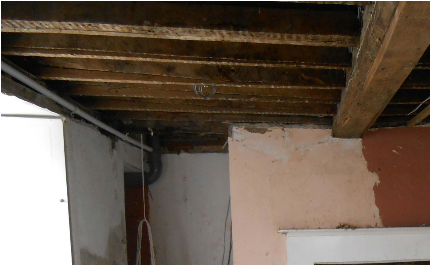
Plate 60: The old repairs to the Library ceiling joists, after plaster stripping. Photograph provided by Nigel Hutt, Clerk of Works
