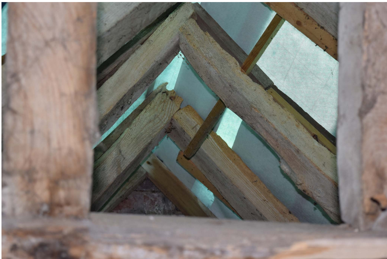
Plate 41: A carpenters' mark on a rafter of the link dormer of the southernmost wing
