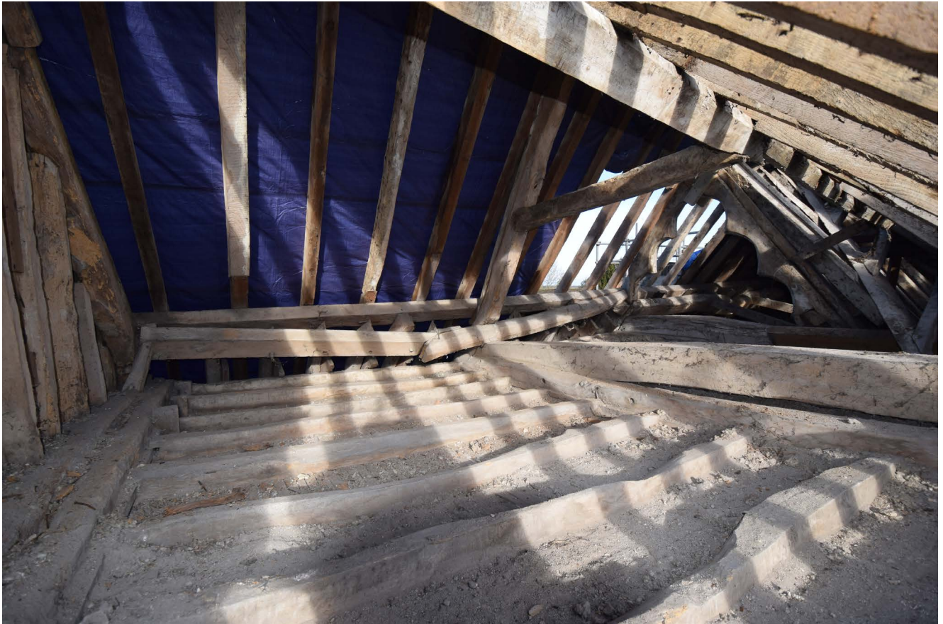
Plate 25: The roof structure of the northernmost wing and 14th-century timbers, looking north
