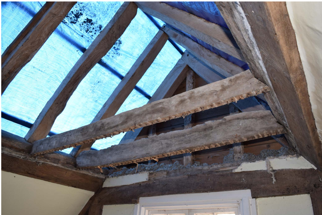
Plate 42: An example of the roof structure of the southernmost wing
