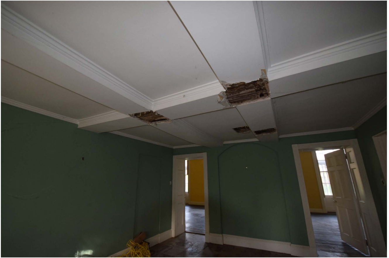
Plate 53: The investigation work to the beams in the Reception Hall
