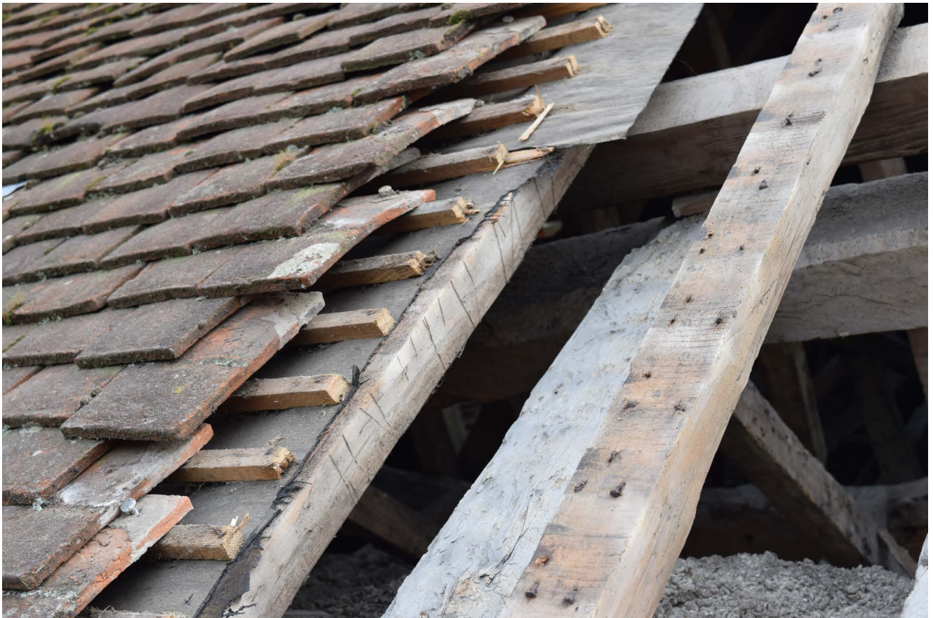
Plate 34: Baltic timber marks in one of the northernmost rafters of the northernmost wing
