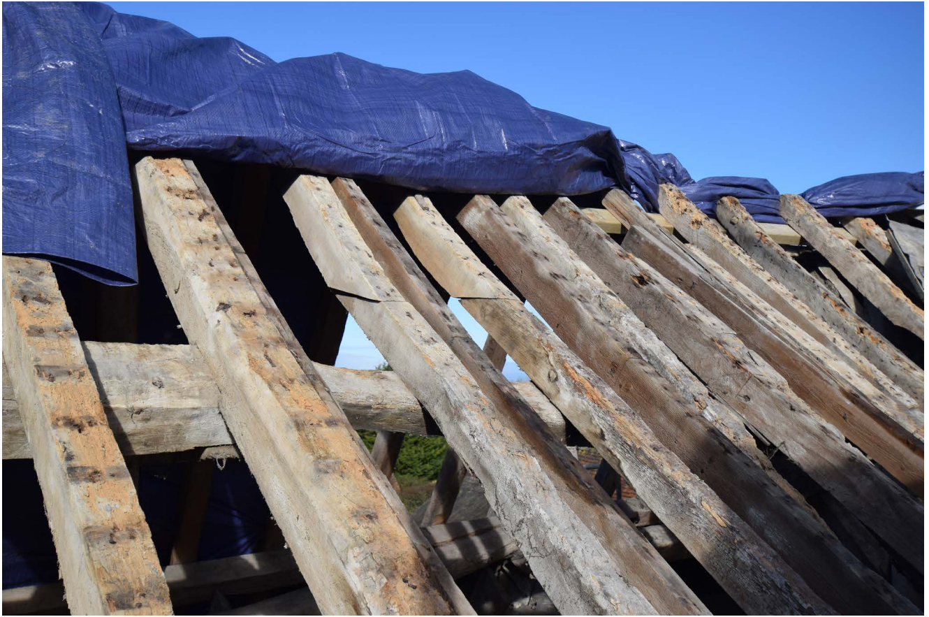
Plate 35: Joined timber to form rafters in the southernmost pitch of the northernmost wing
