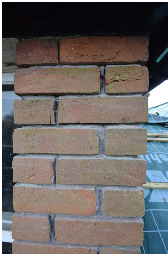
Plate 21: The exposed original mortar of the 18th-century extension before repointing
