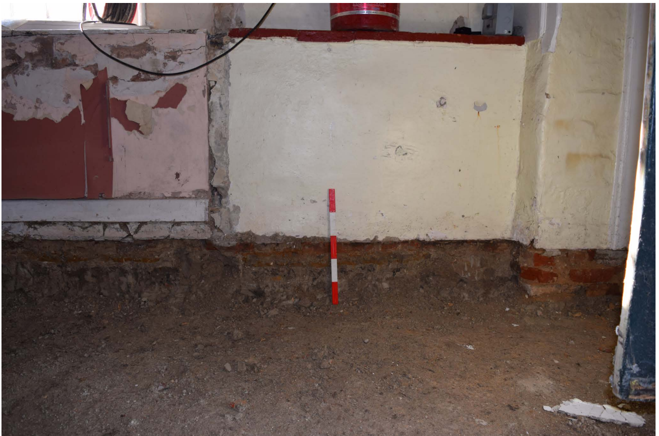
Plate 58: The base of the front wall of the Library after floor excavation
