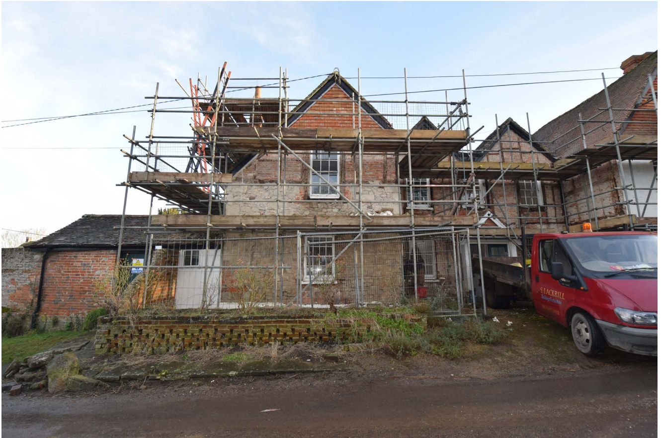
Plate 5: The south west elevation of the northernmost wing after removal of the render
