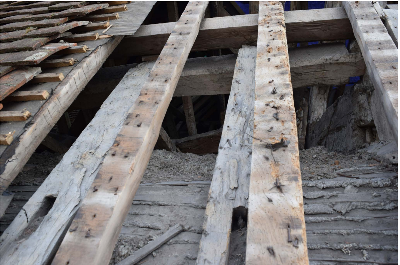
Plate 28: The redundant sockets in an earlier phase of roof timbers in the northernmost wing
