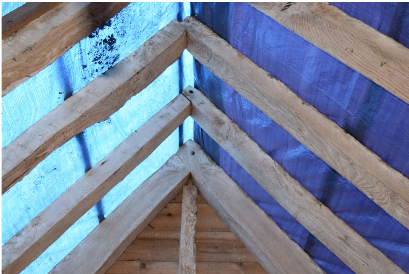
Plate 43: The joints and carpenters' marks in the rafters of the southernmost wing
