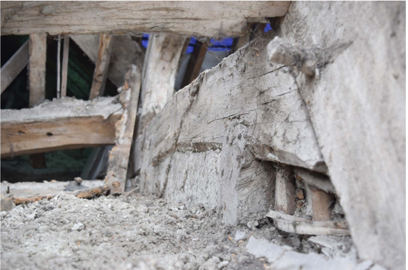
Plate 31: Damage or rework to 14th-century timbers, north eastern face of tiebeam
