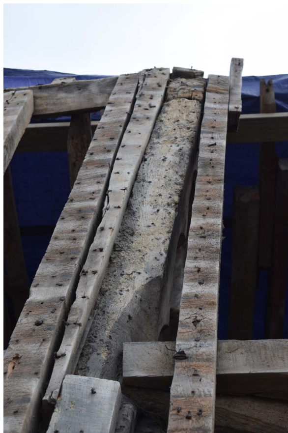
Plate 29: Damage or rework to 14th-century timbers, northernmost edge of principal rafter
