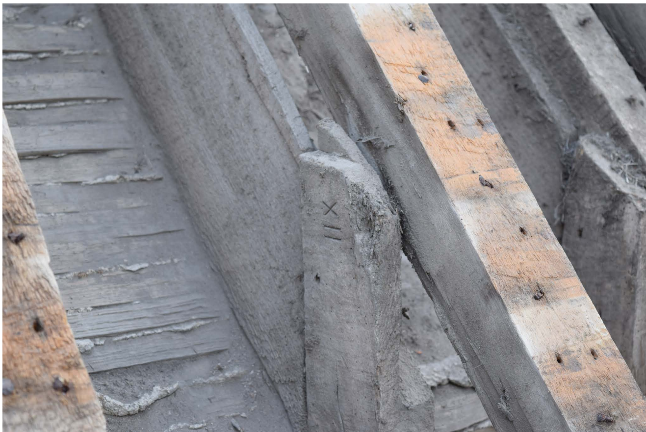
Plate 39: A carpenters' mark in a reused piece of timber in the northernmost pitch
