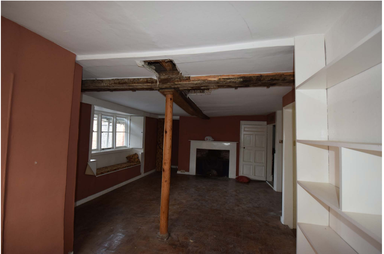
Plate 59: The investigation work to the beams in the Library
