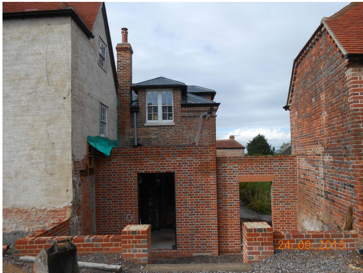
Plate 24: The construction of the new conservatory and new lime render. Photograph provided by Nigel Hutt, Clerk of Works
