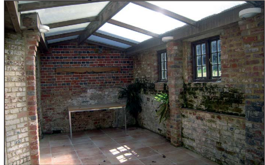
Plate 26 Conservatory showing efflorescence to the stable wall and ferns growing from walls
