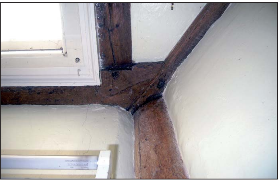
Plate 53 An example of a carpenter's mark in the study
