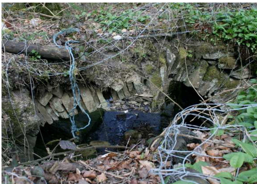
Plate 18: collapsed section of bridge, showing instability of arch to west
