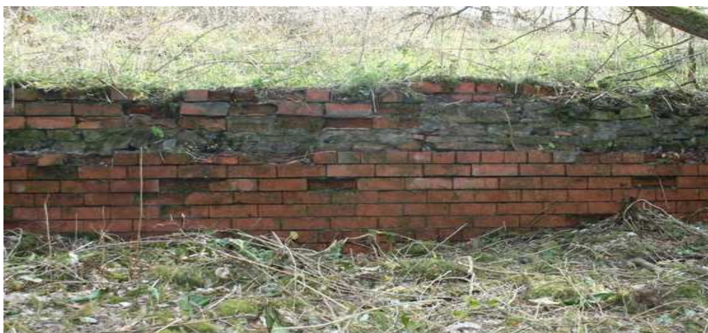
Plate 26: Section of Wall A2_13, with 'Accrington' brick refacing
