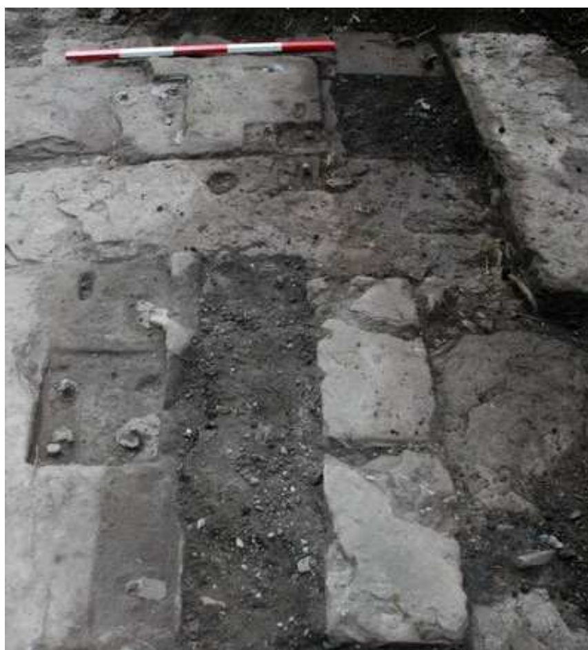
Plate 32: Fixing bolts and housings within dressed blocks of machine base
