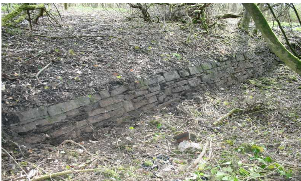
Plate 27: Battered retaining wall at the western end of Area 2
