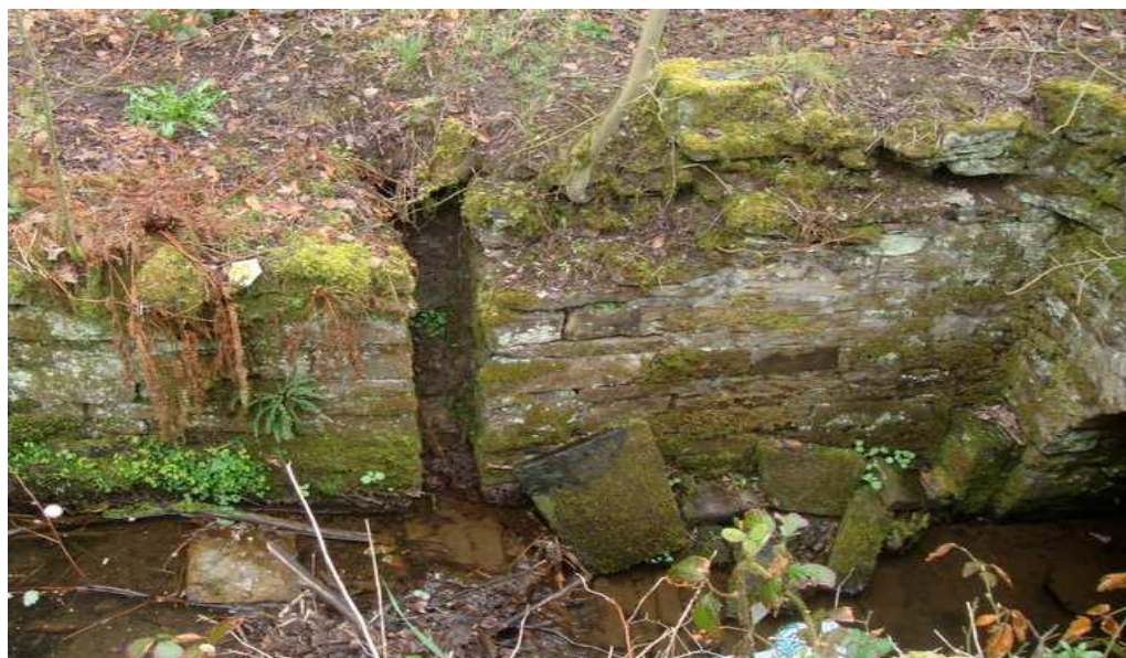
Plate 13: South wall of sluice (A1_3) with rebate for sluice gate
