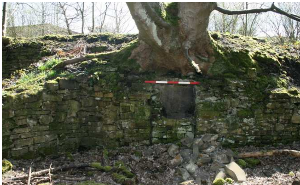
Plate 25: Wall A2_7, with partially blocked aperture, and invasive large tree
