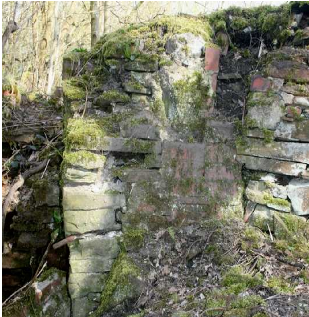
Plate 24: Blocked aperture for leat in Wall A2_4, and attachment bolt protruding from face
