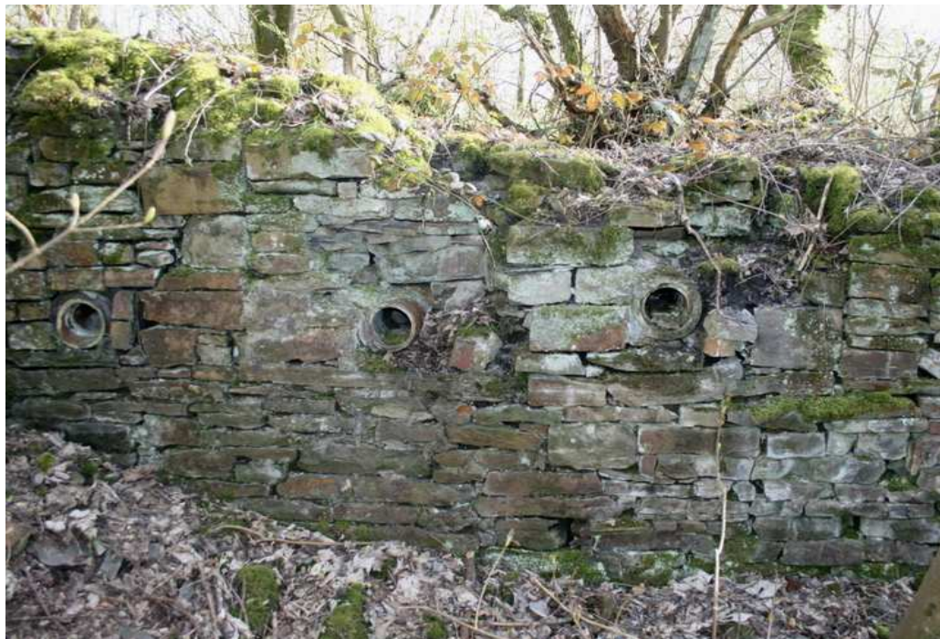
Plate 22: Wall A2_2, with blocked window apertures and inserted ceramic pipes
