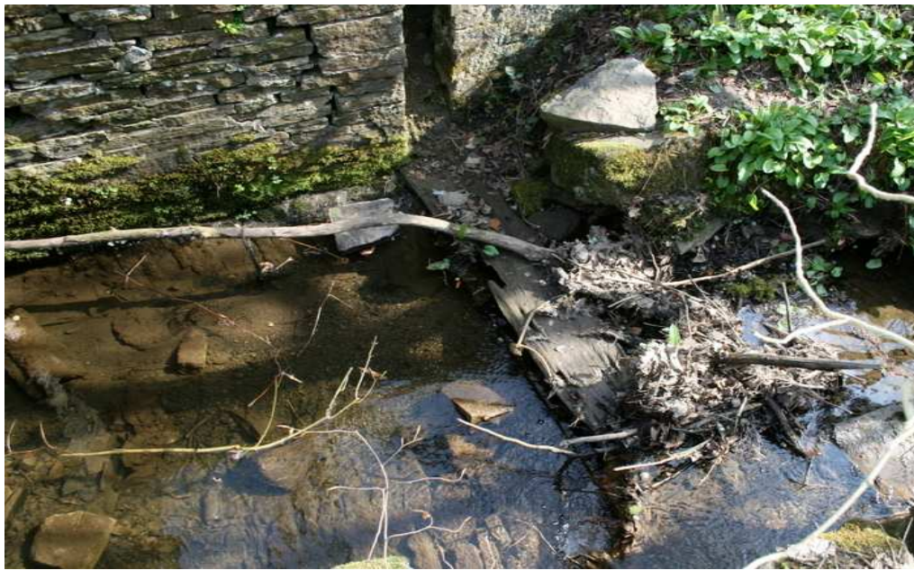
Plate 12: Timber sluice board, with stone flooring to the left
