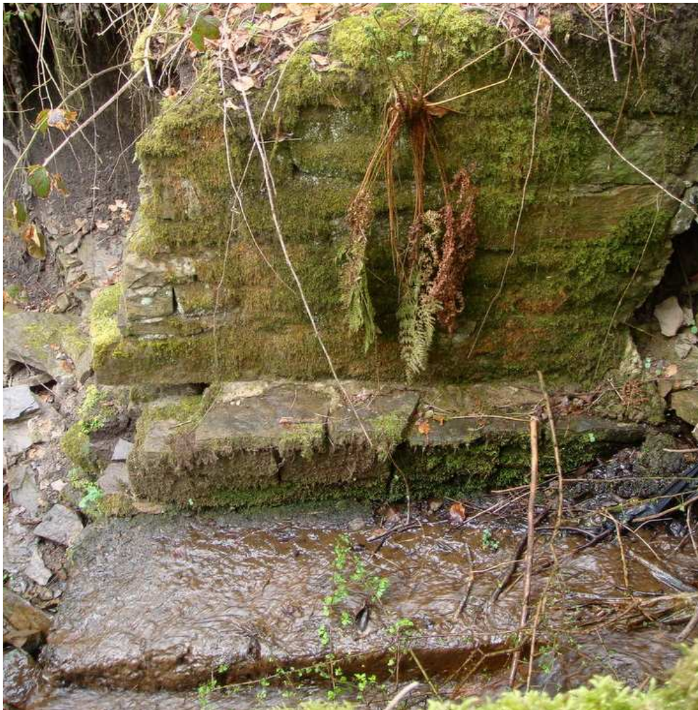
Plate 14: North wall of sluice (AI_4) with concrete sluice channel
