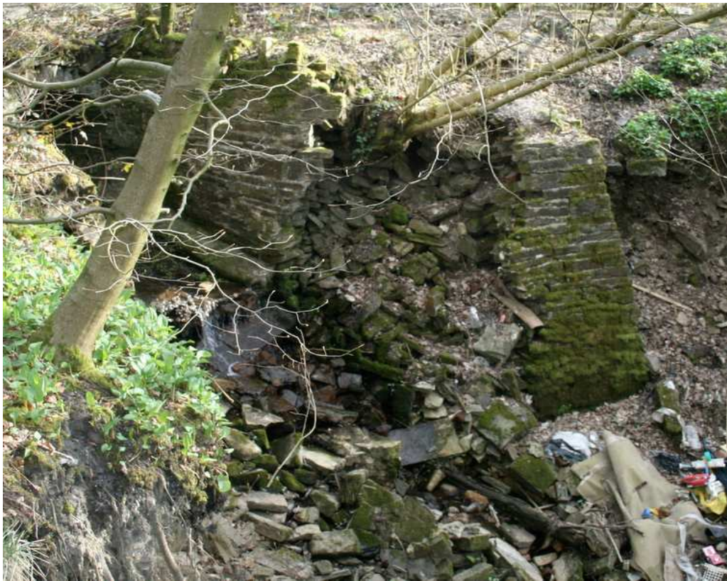
Plate 19: Buttressed retaining wall on the south side of the ravine
