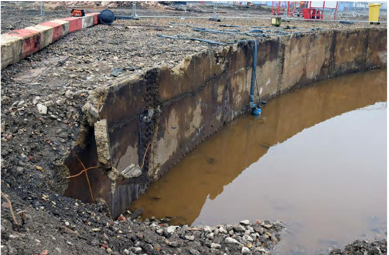
Plate 14: Base of holder 4 after demolition of tank
