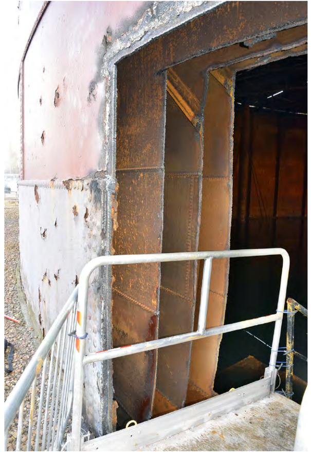
Plate 6: Gasholder 4 detail of lifts after creation of opening in holder
