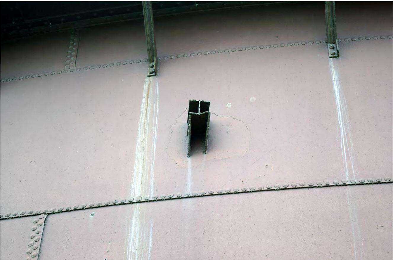
Plate 4: Detail of truncated bracket to gasholder 4
