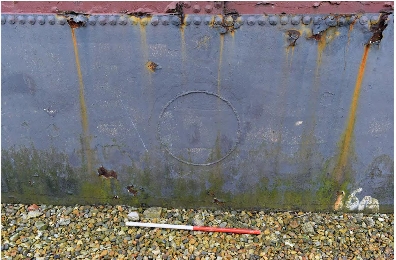
Plate 9: Infilled opening from former pipe in gasholder 4
