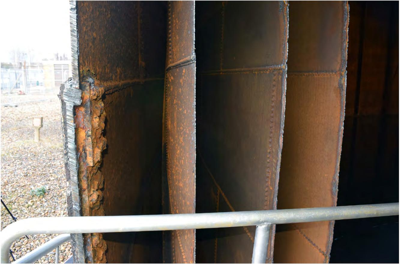
Plate 8: Detail of lifts within tank of No 4 after cutting through
