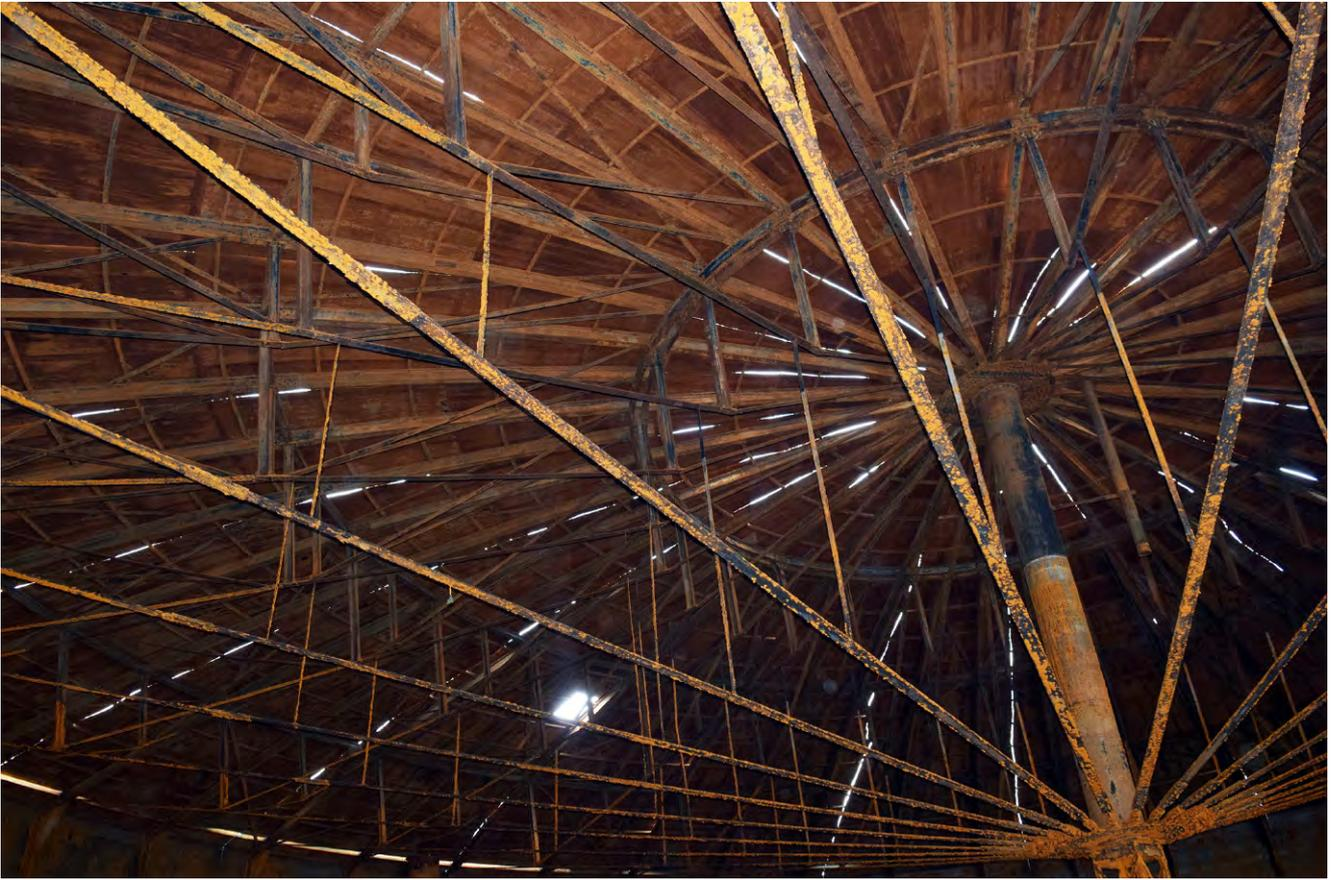
Plate 67: Roof structure within gasholder 9
