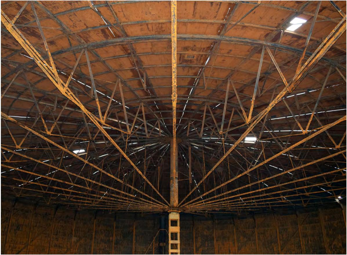
Plate 46: Gasholder 7 roof detail
