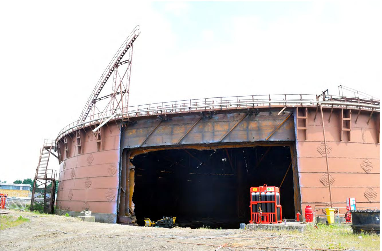
Plate 56: Gasholder 9 during demolition
