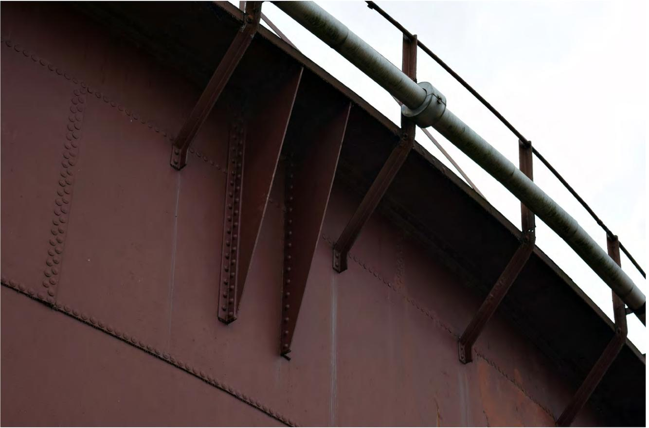
Plate 3: Detail of bracket to gasholder 4
