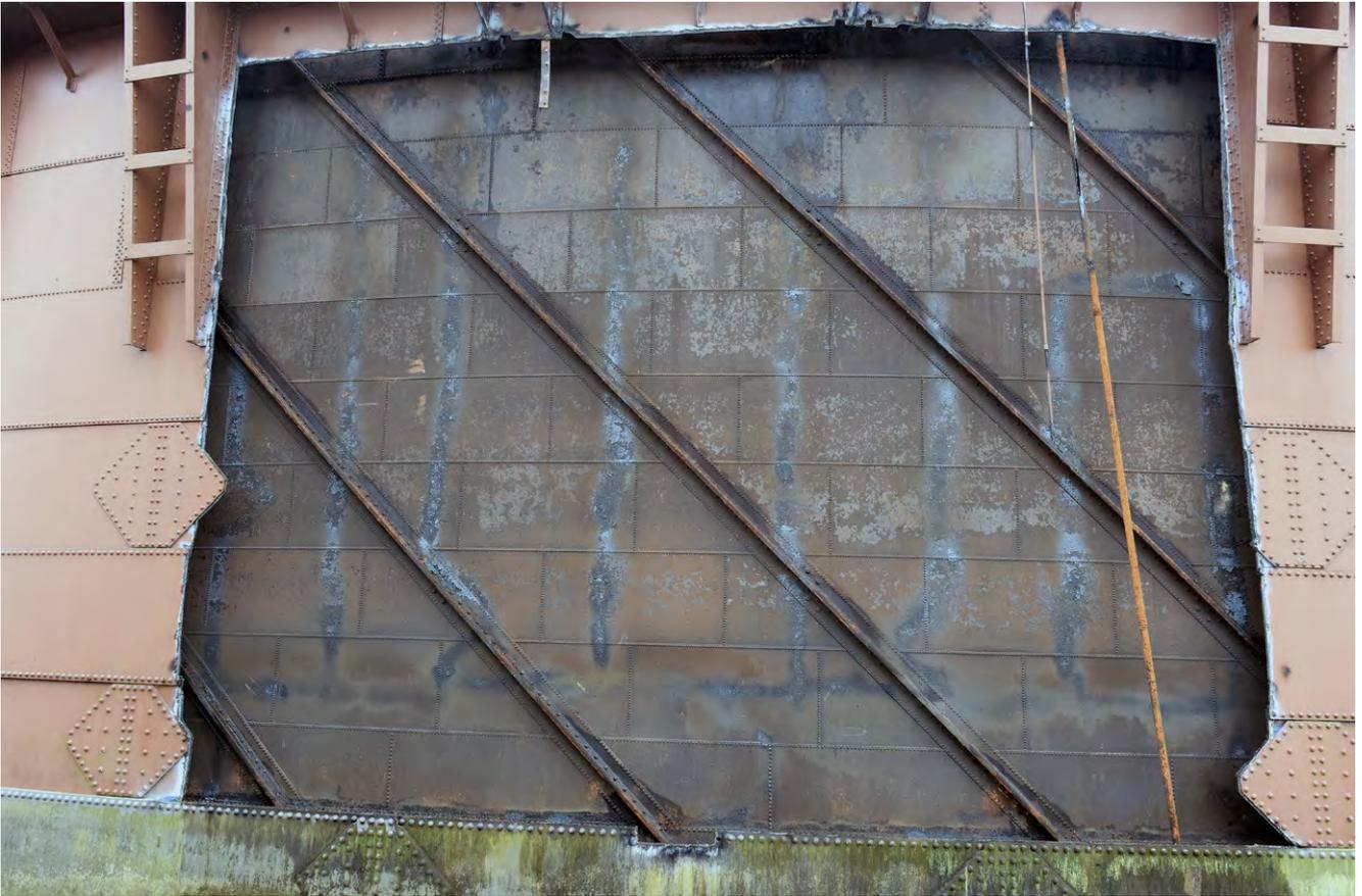
Plate 34: Gasholder 7 after removal of section of outer tank
