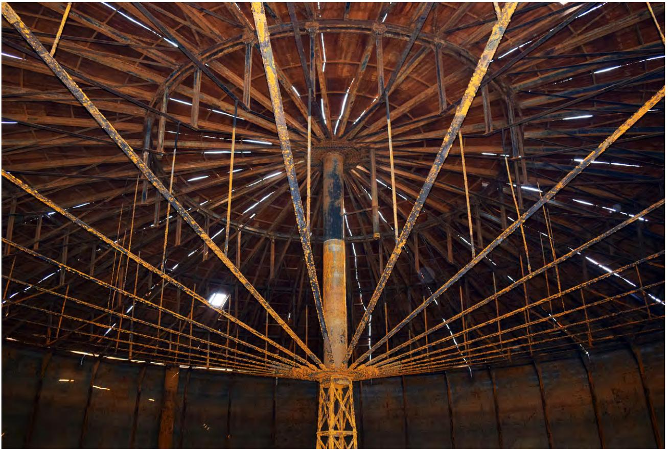
Plate 64: Roof structure within gasholder 9
