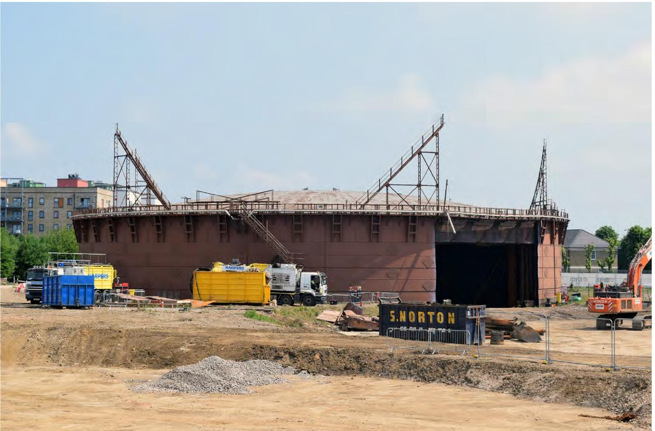
Plate 54: General view of gasholder 9 during demolition
