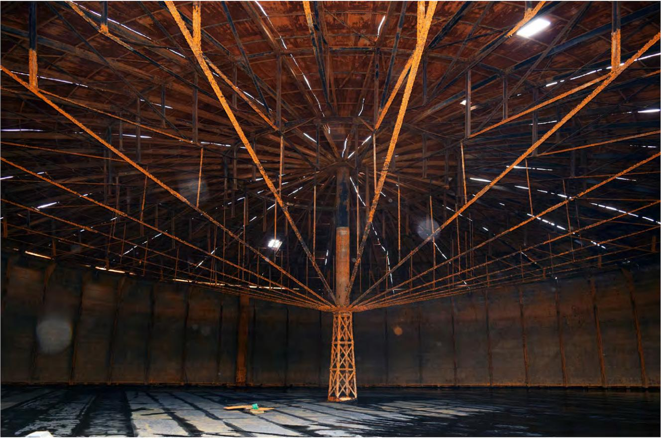
Plate 63: Roof structure within gasholder 9
