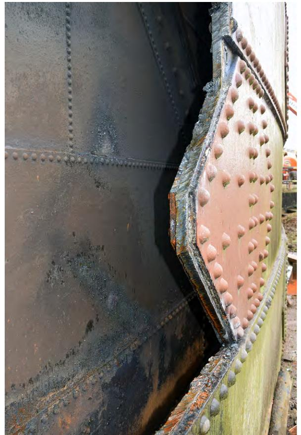
Plate 39: Detail of outer tank during demolition
