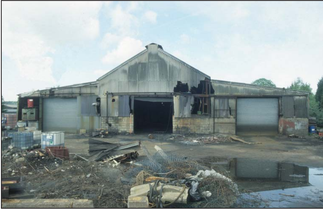
Plate 3: South end of foundry, showing extension 3, 4 and 5
