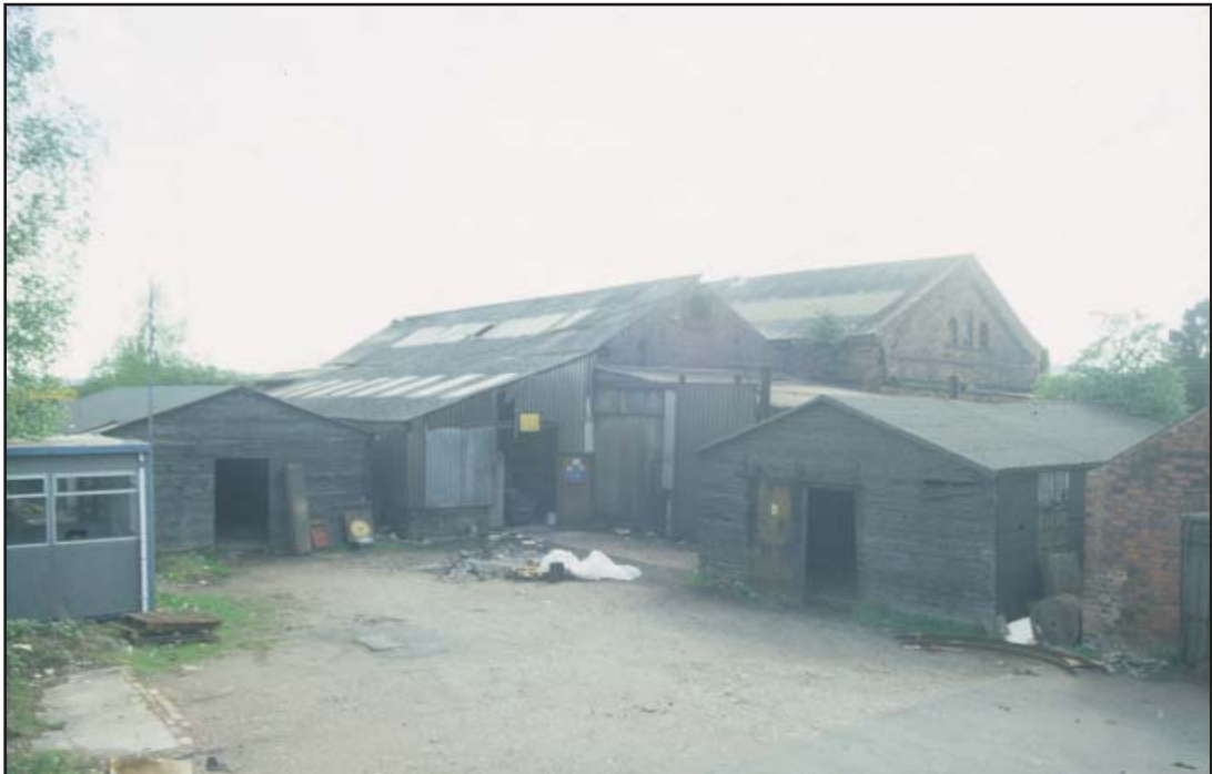
Plate 2: North end of foundry, showing buildings 1, 3, 5, 6 and 7
