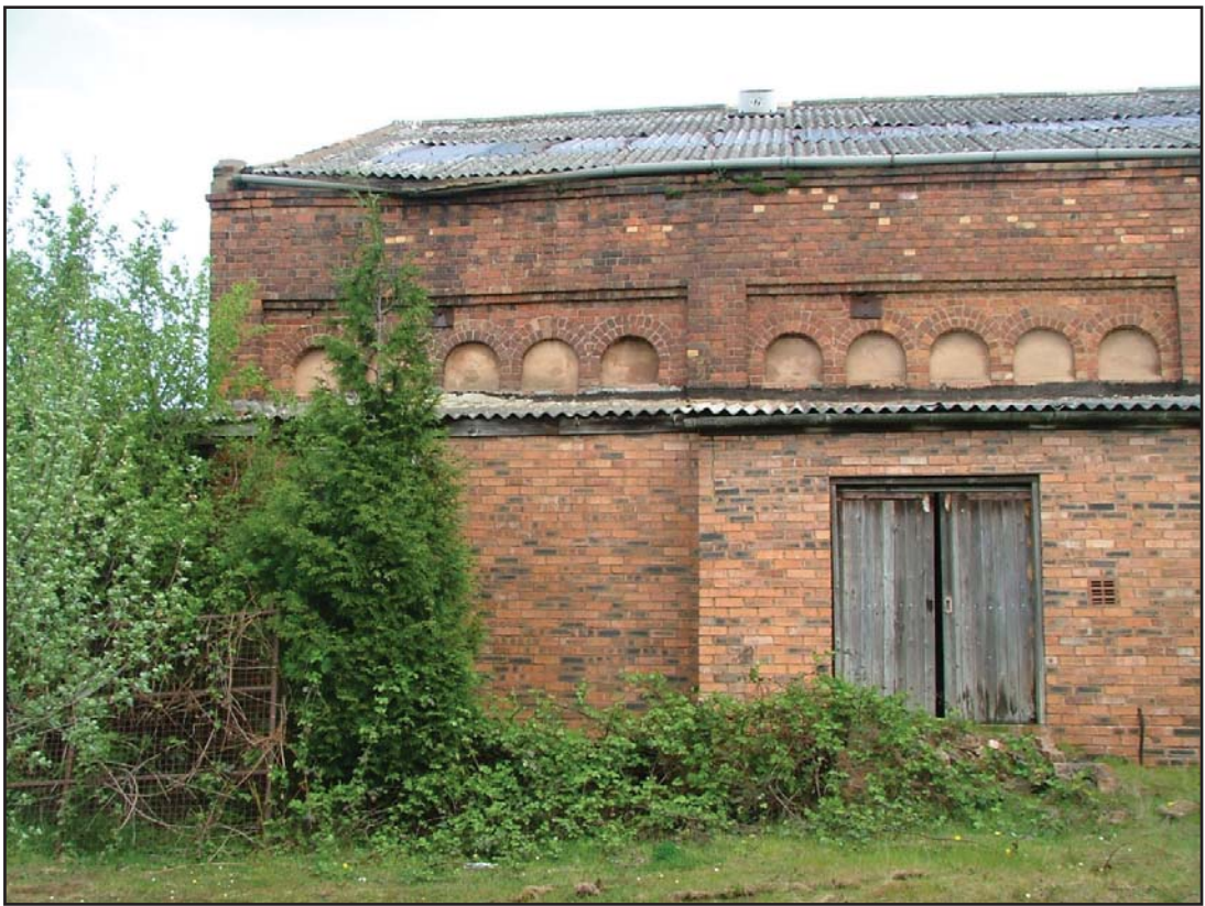
Plate 8: North-western end of building 7, showing round topped windows
