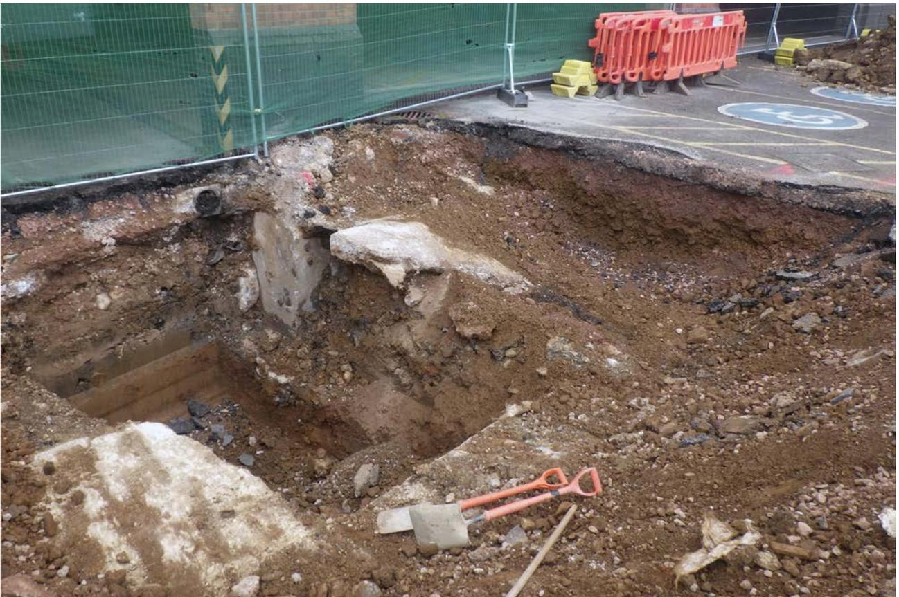
Plate 2: Lift shaft pit excavation, looking west
