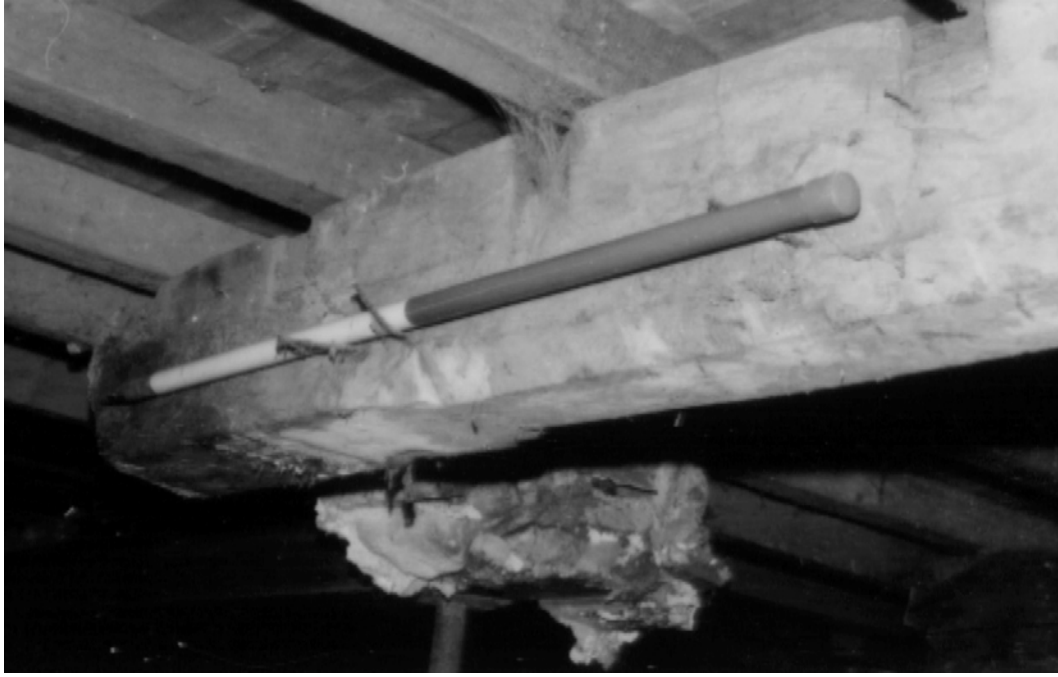
Plate 9: Detail of the beam chamfer in Room 3
