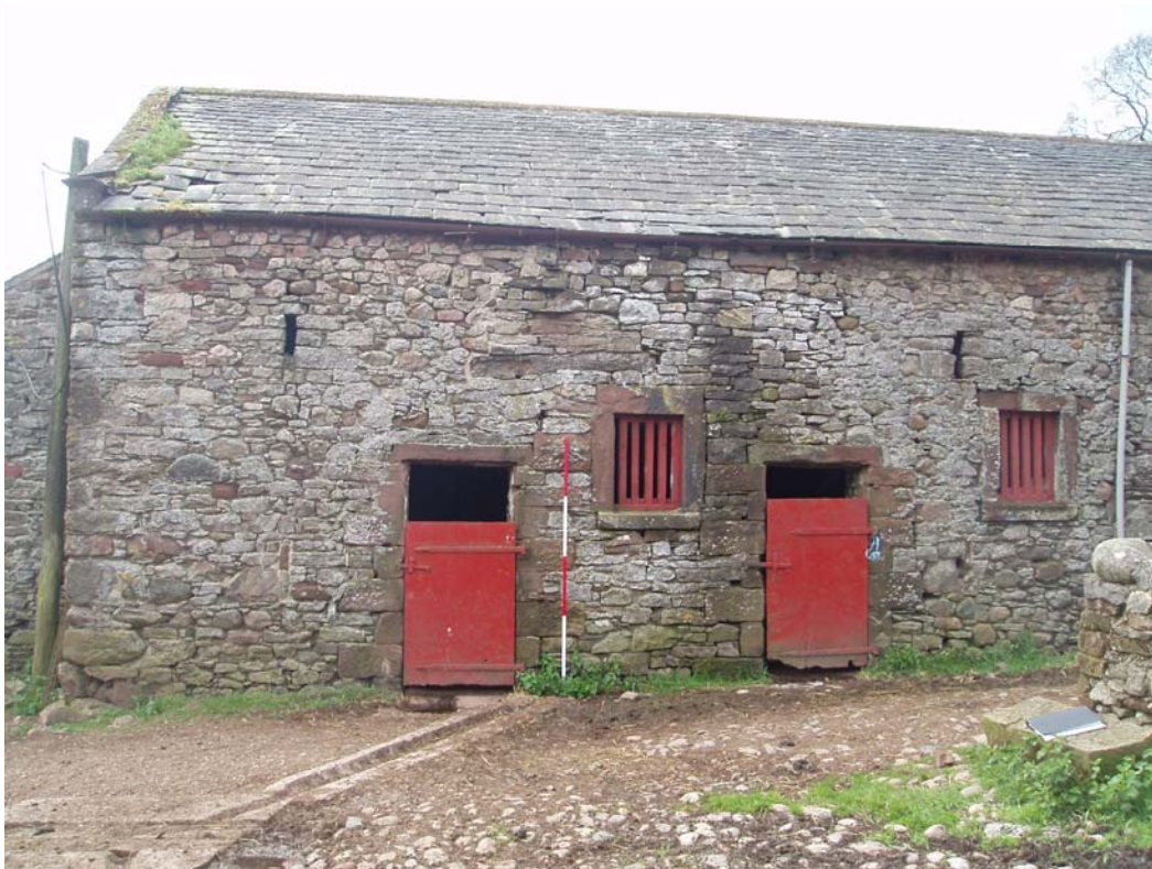
Plate 9: Inserted doorways and windows in the north elevation of the barn
