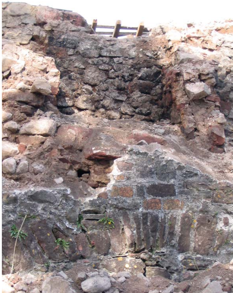
Plate 16: The back of the flue of the large chimney as exposed during demolition
