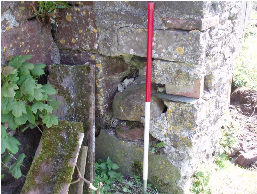
Plate 8: A splayed window jamb in the east elevation of the original hall
