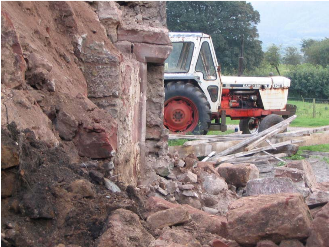
Plate 18: The dressed jamb exposed during demolition in the east stub wall
