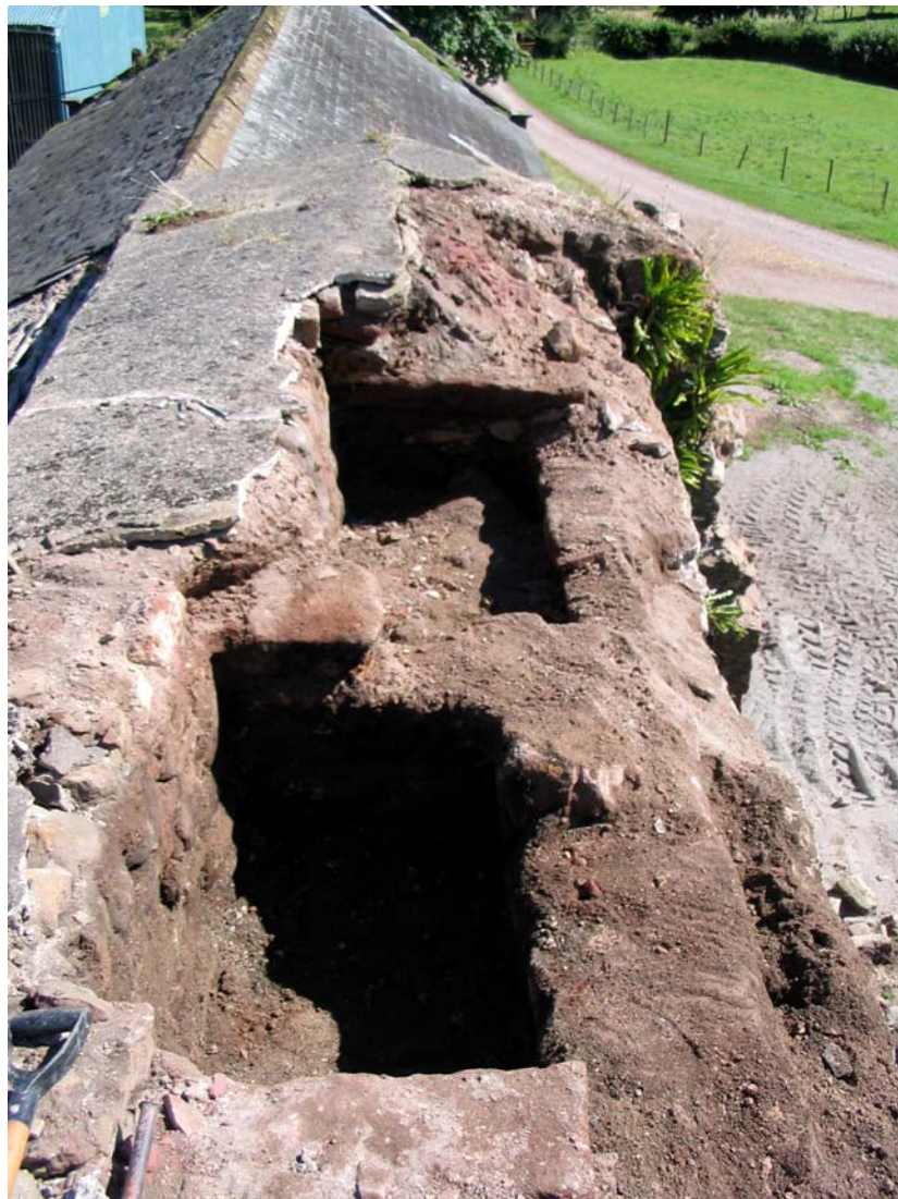
Plate 15: The tops of the two flues as exposed during demolition
