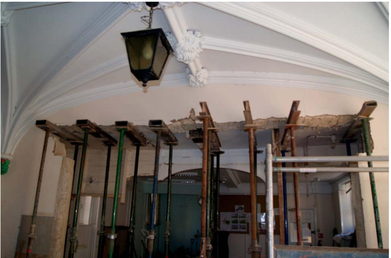
Plate 24: Passage looking east after creation of opening
