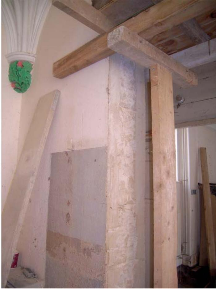
Plate 37: Opening created in wall between passage and Events Office
