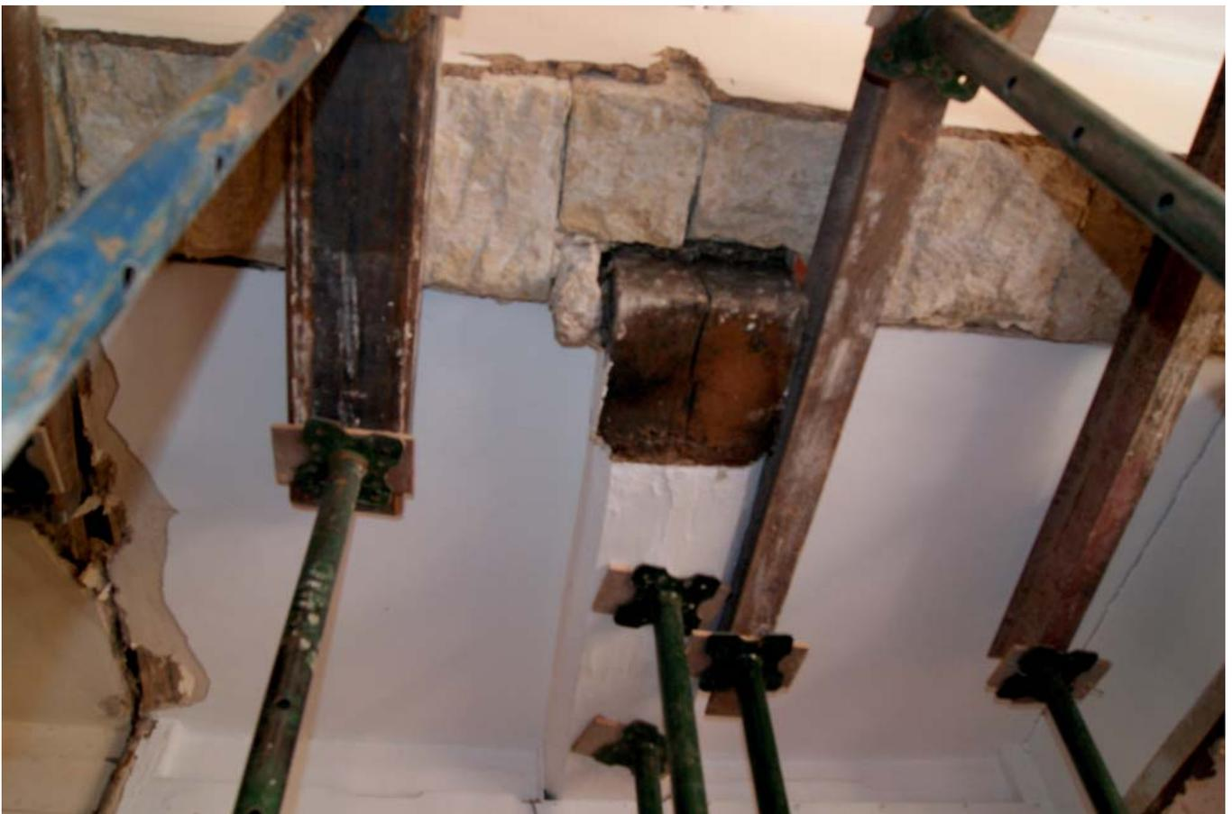
Plate 22: West end of joist in Events Office (after creation of opening)
