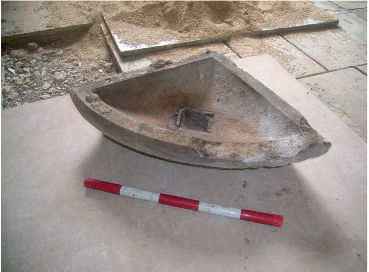
Plate 49: Reused drainage hopper found in wall during excavations
