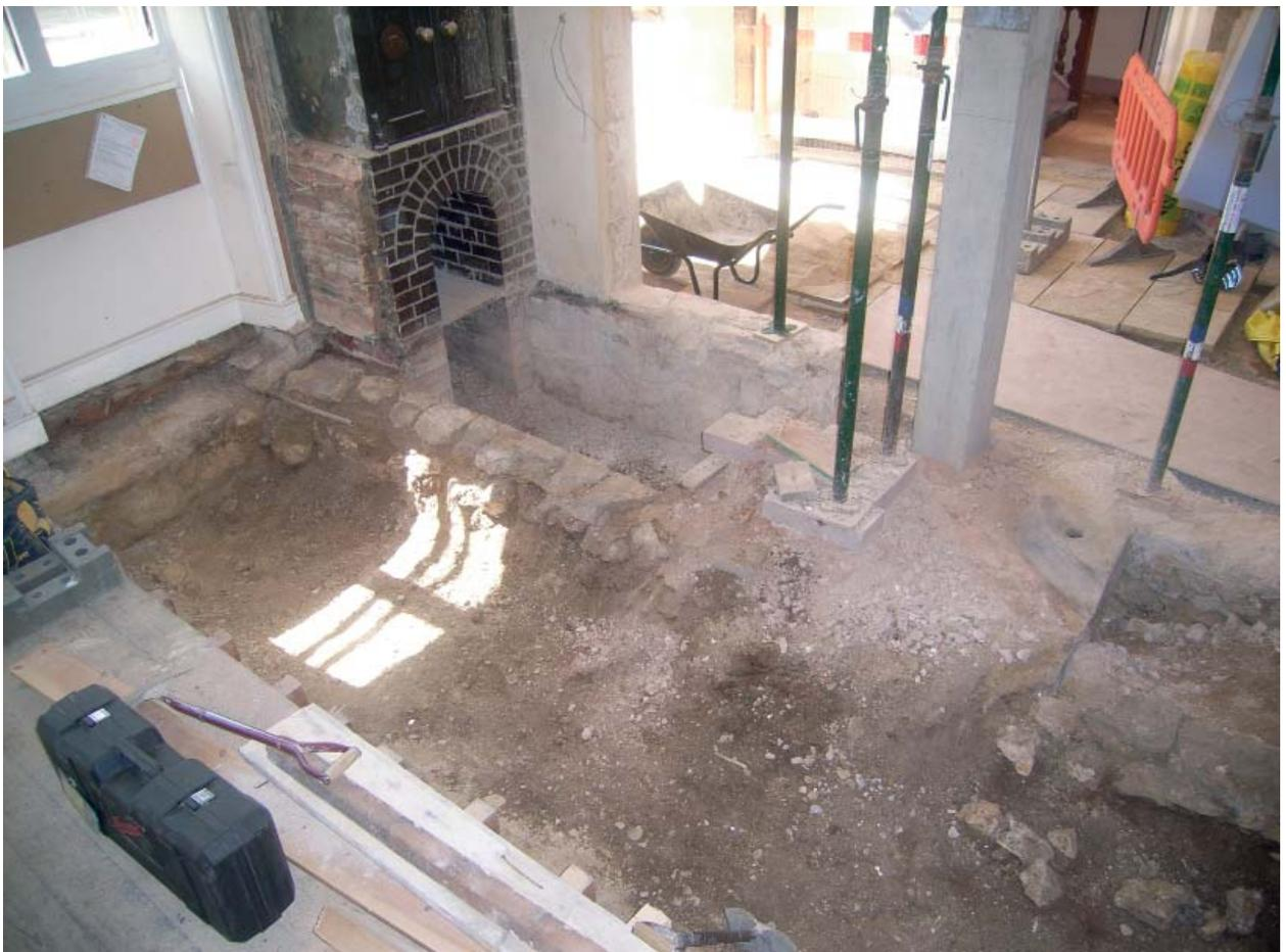
Plate 48: Events Office following floor excavation works
