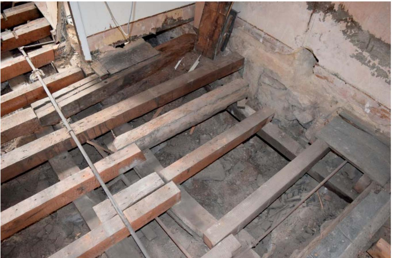
Plate 16: Exposed joists against west wall of Events Office
