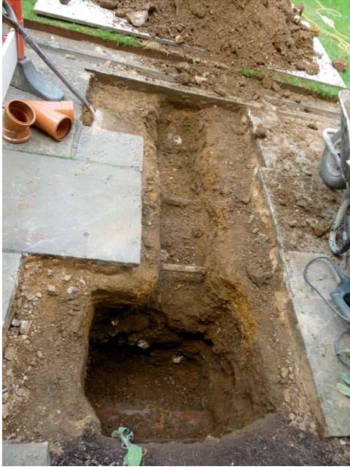
Plate 53: Drainage outlet watching brief at east side of quad
