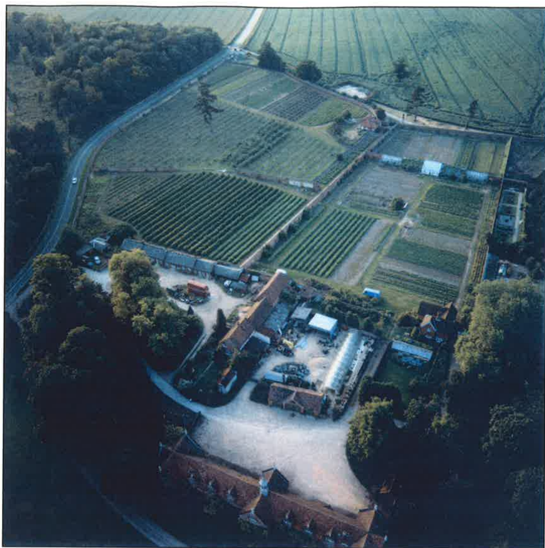
Figure 10 c.1990 Aerial Photograph of Site (English Heritage Archive nd.)
