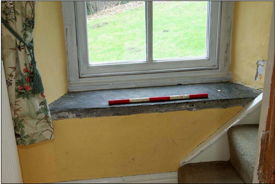
Plate 16: Stone sill of the window on the lower landing in Room 5
