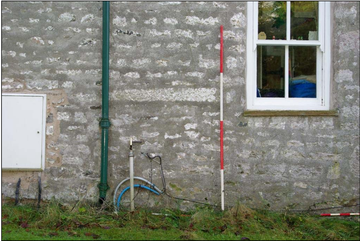
Plate 5: Blocked aperture on the north elevation of Garden Cottage
