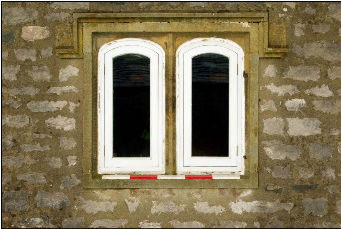
Plate 8: Detail of the ground floor mullioned window on the south elevation
