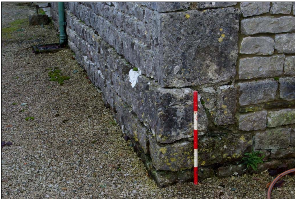
Plate 23: Narrow plinth at the base of the wall on the outbuilding
