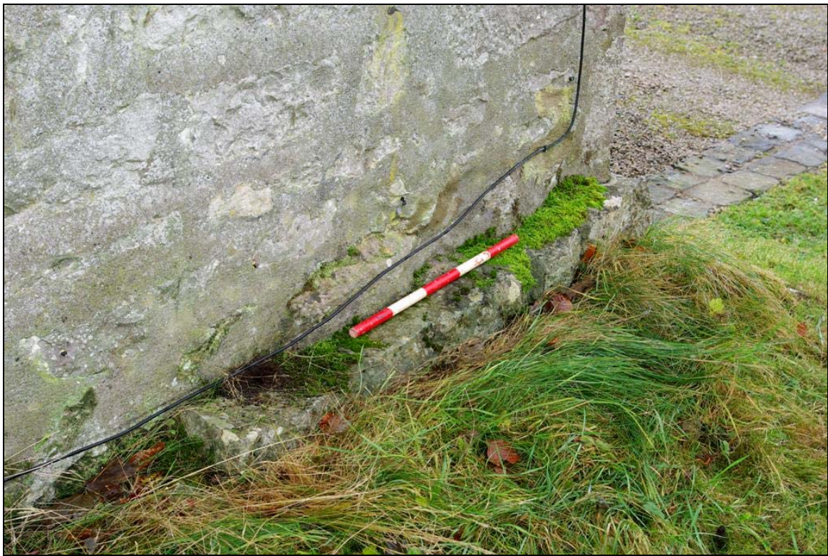
Plate 6: 'Plinth' at the base of the north elevation of Garden Cottage
