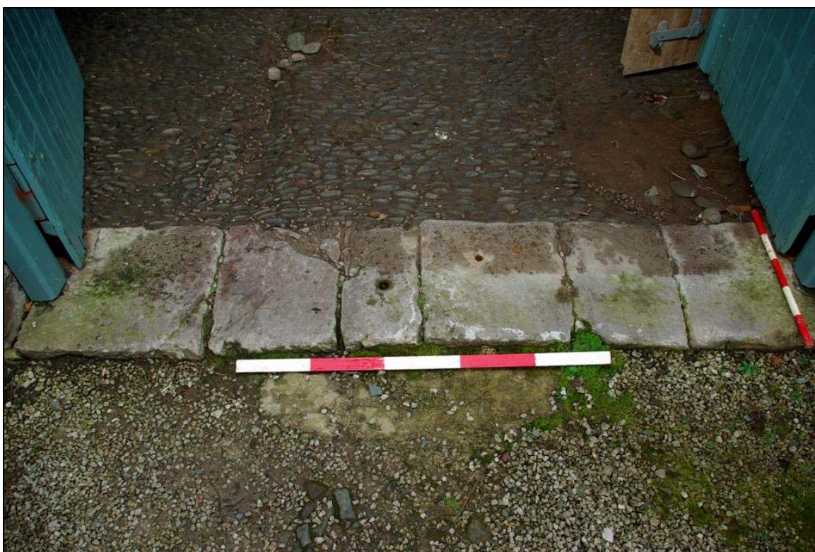
Plate 22: Limestone threshold of the main door of the outbuilding
