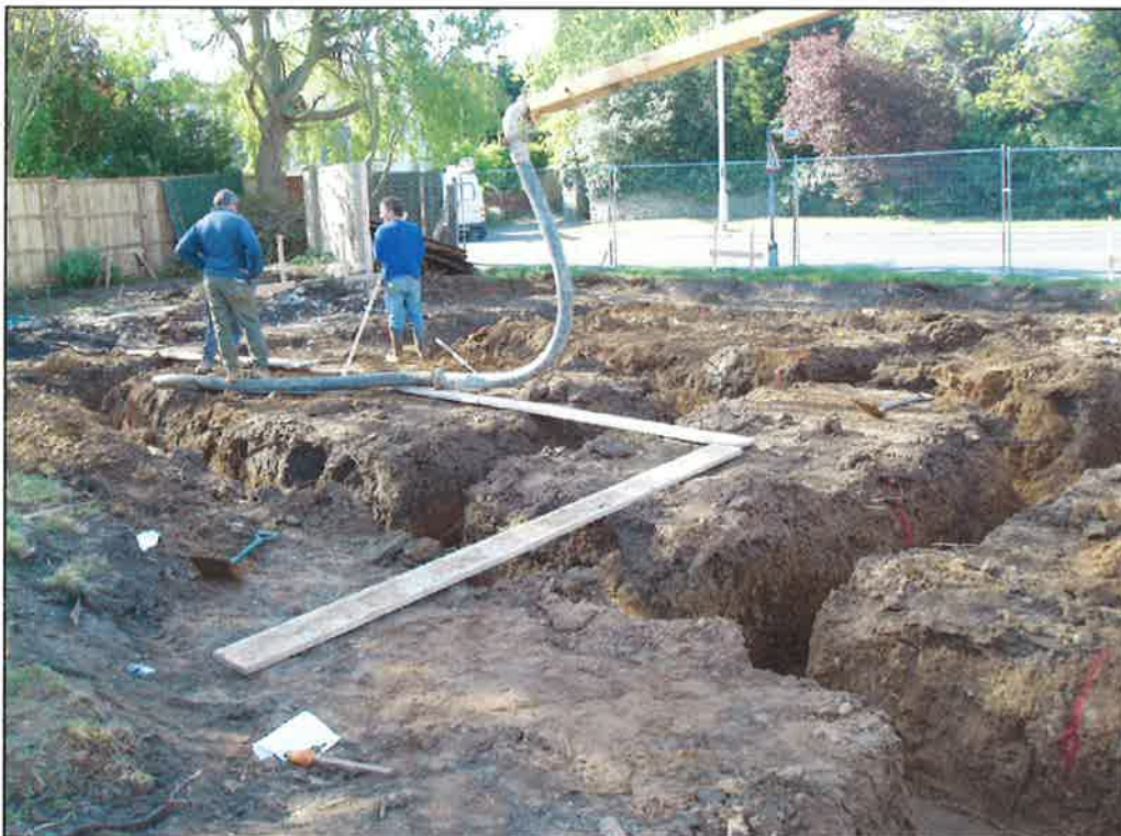
Plate 1 General view of the foundations
