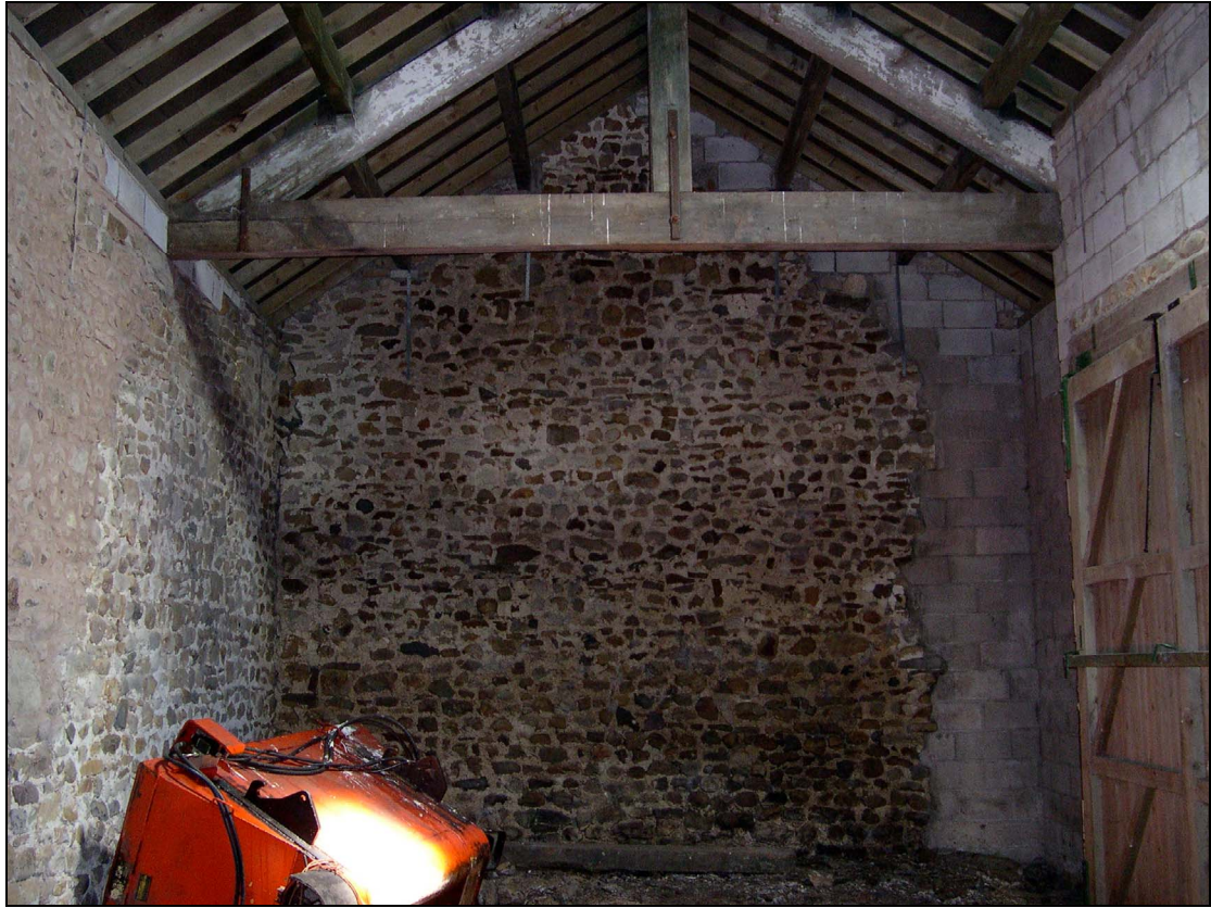
Plate 7: Interior of barn, showing east elevation
