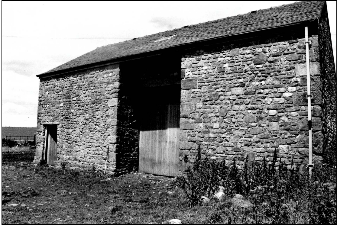
Plate 1: Front elevation of barn, looking north-east
