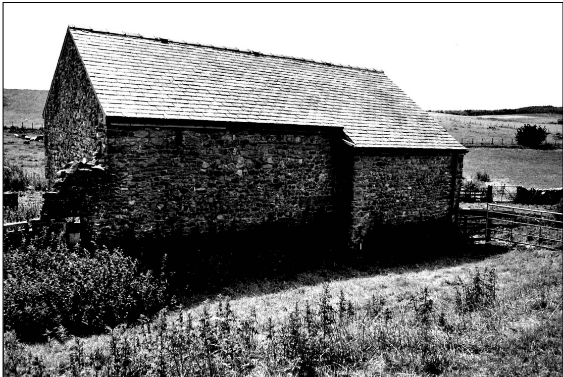
Plate 2: Rear elevation of barn, looking north-west
