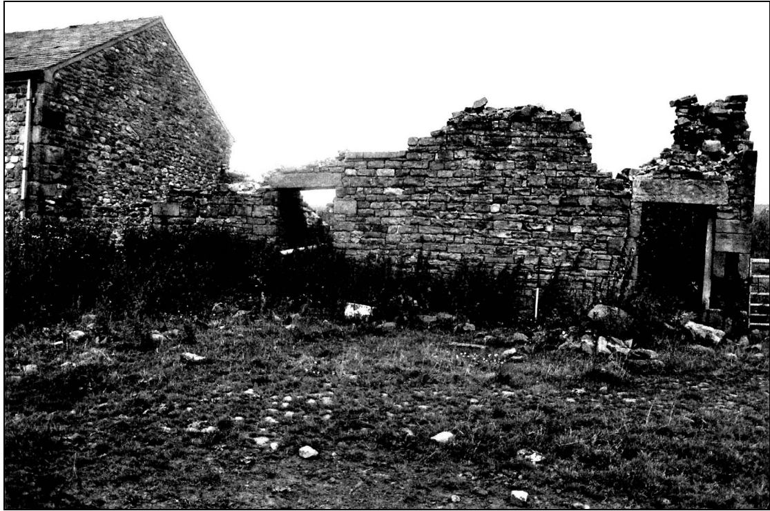
Plate 5: Front elevation of farmhouse remains, looking north
