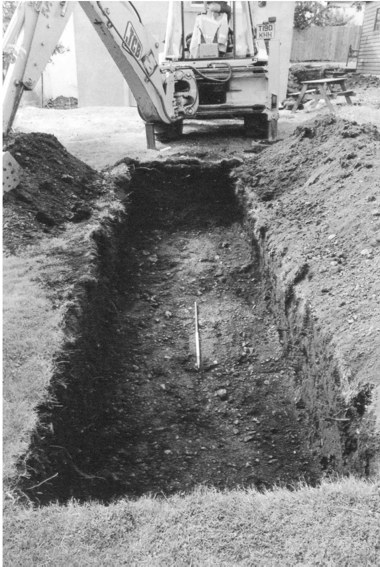
Plate 1: Trench 1 looking north
