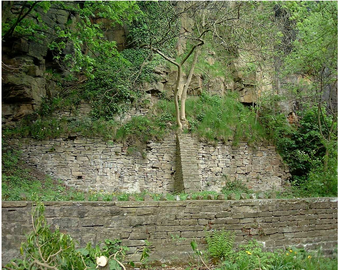
Plate 20: Remains of cottages to north-west of the mill complex, showing buttress
