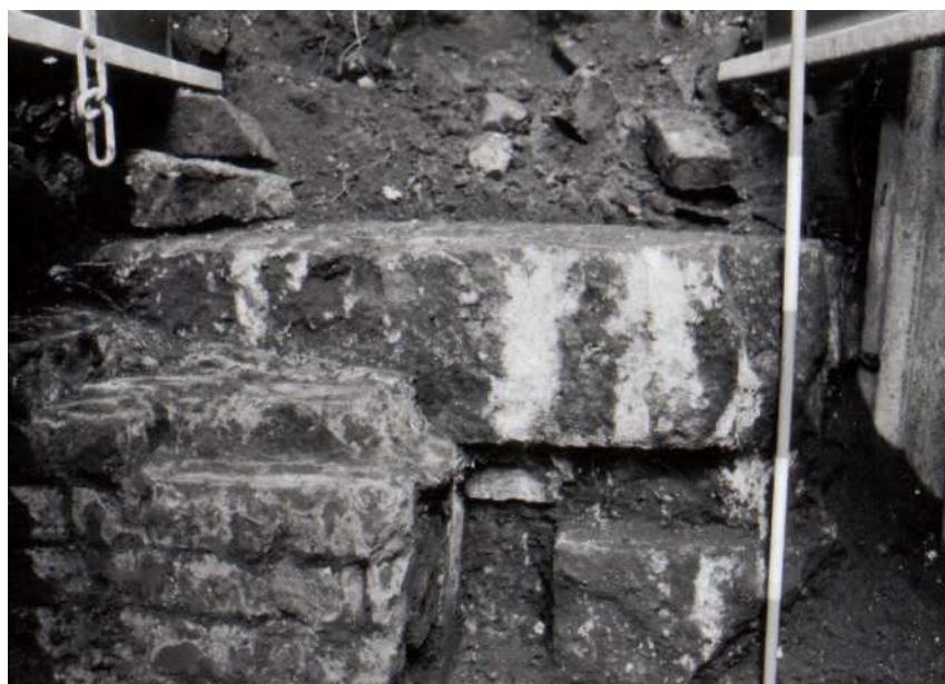
Plate 13: North wall of wheel pit, looking north
