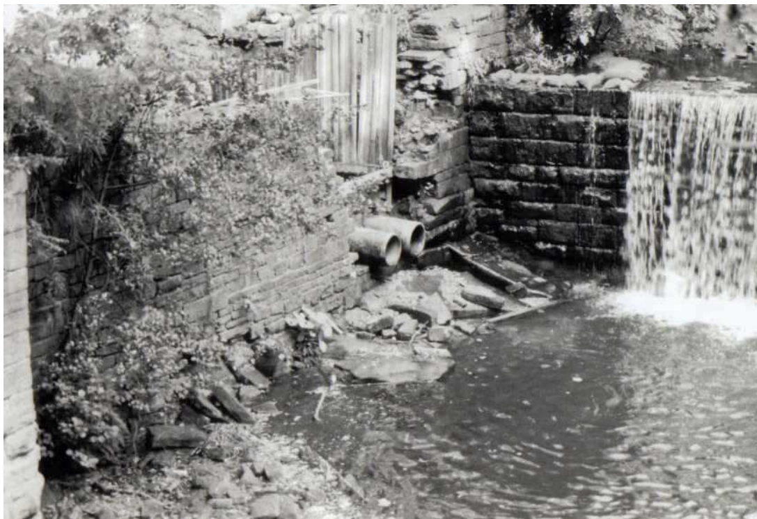
Plate 16: New outflow through retaining wall
