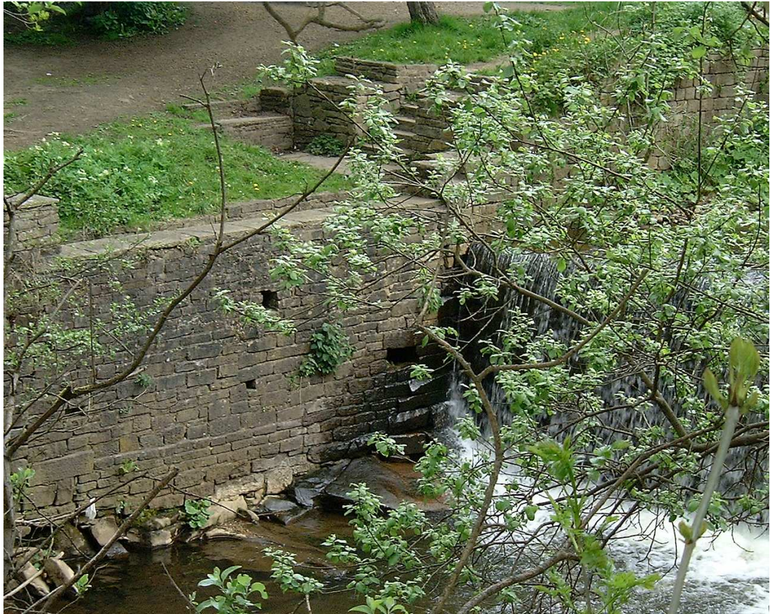
Plate 15: East-west retaining wall prior to excavation
