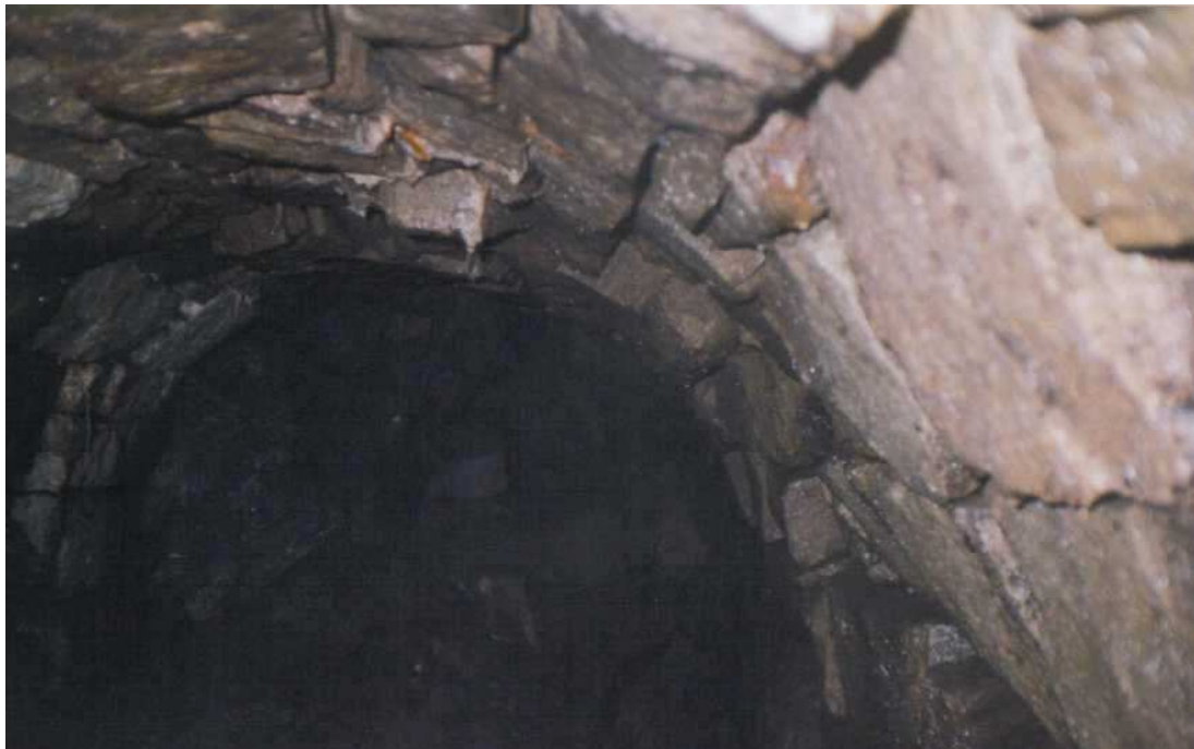
Plate 12: Interior of drain 401
