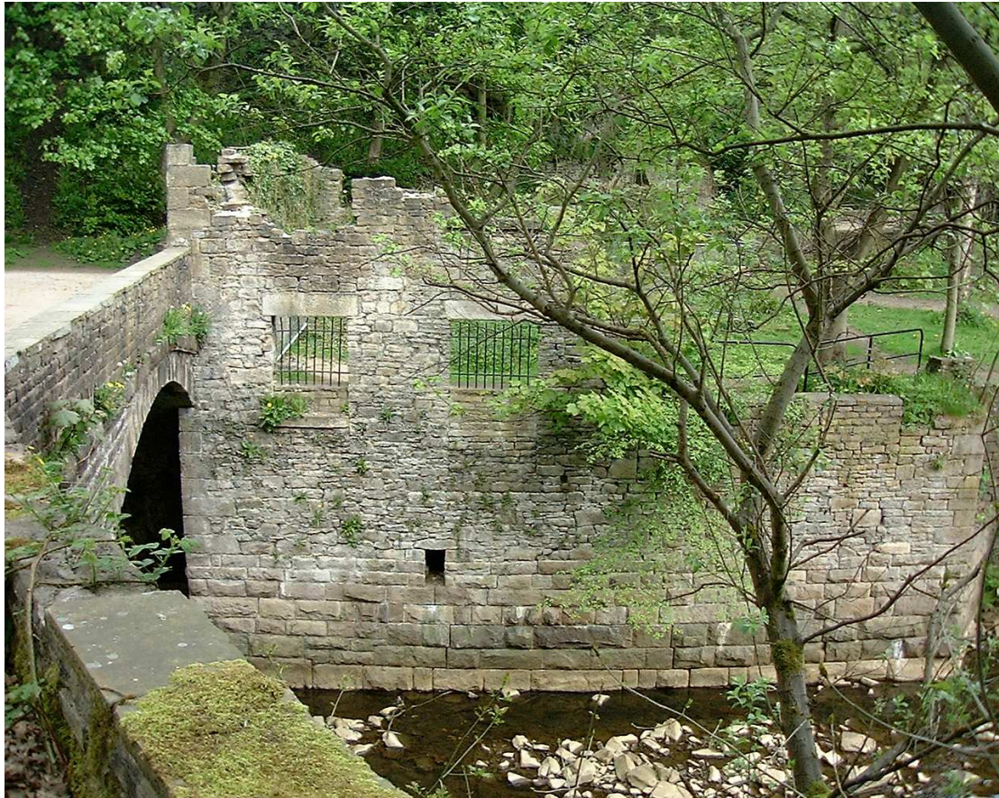
Plate 17: Extenal south wall of yarn warehouse and east parapet of the bridge
