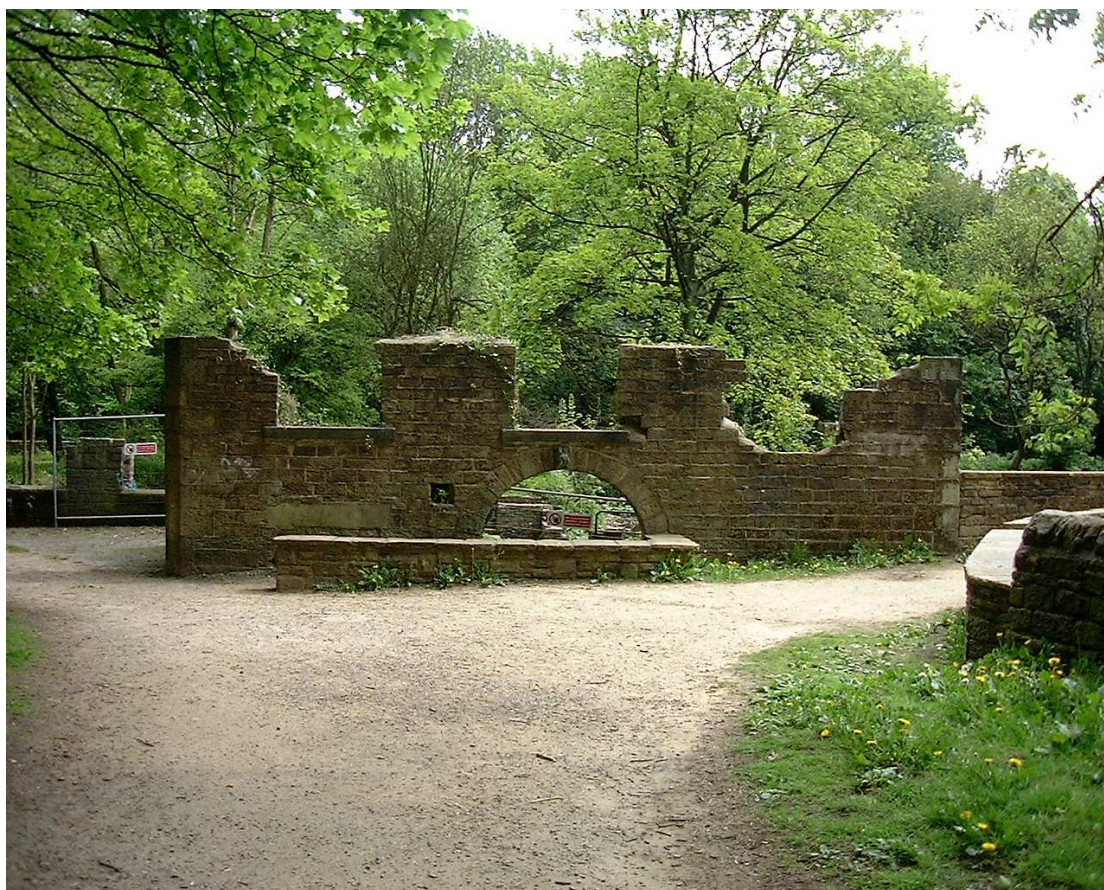
Plate 22: West wall of yarn warehouse
