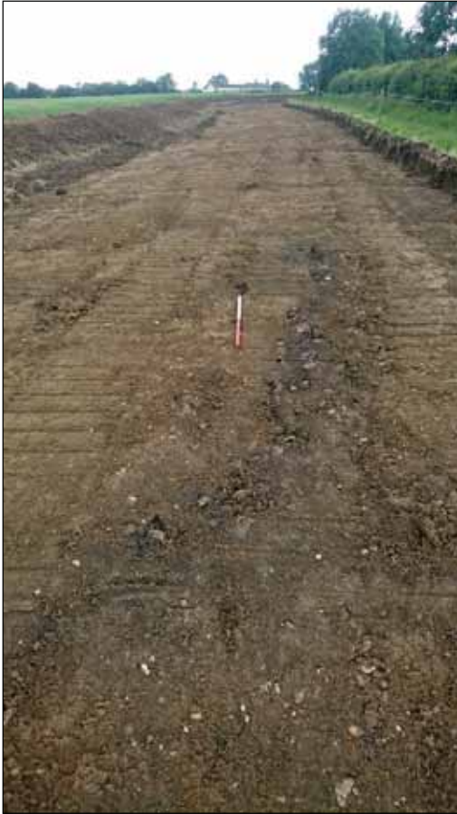
Plate 1: Pipeline scheme strip, looking north-west
