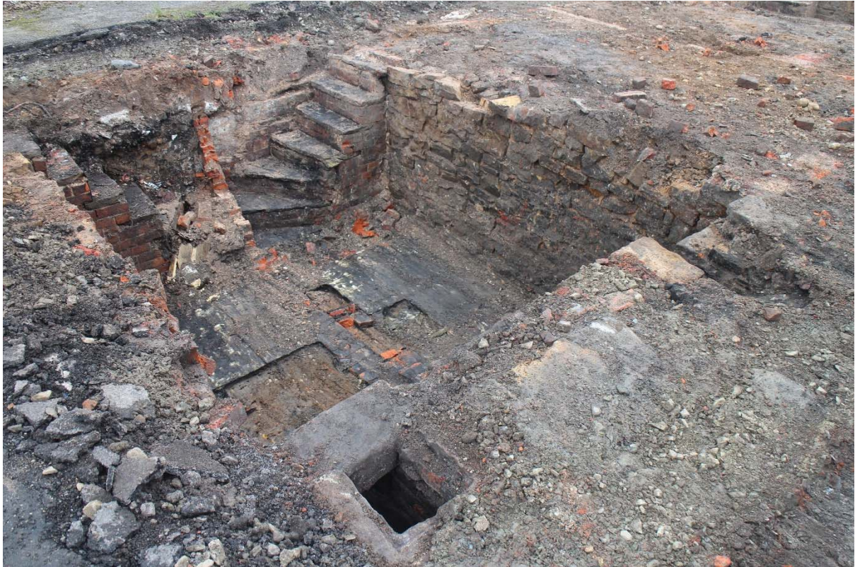
Plate 23. Structure 2018 , featuring the steps set in the southern elevation (background), and coal chute (foreground). Viewed facing south-west.
