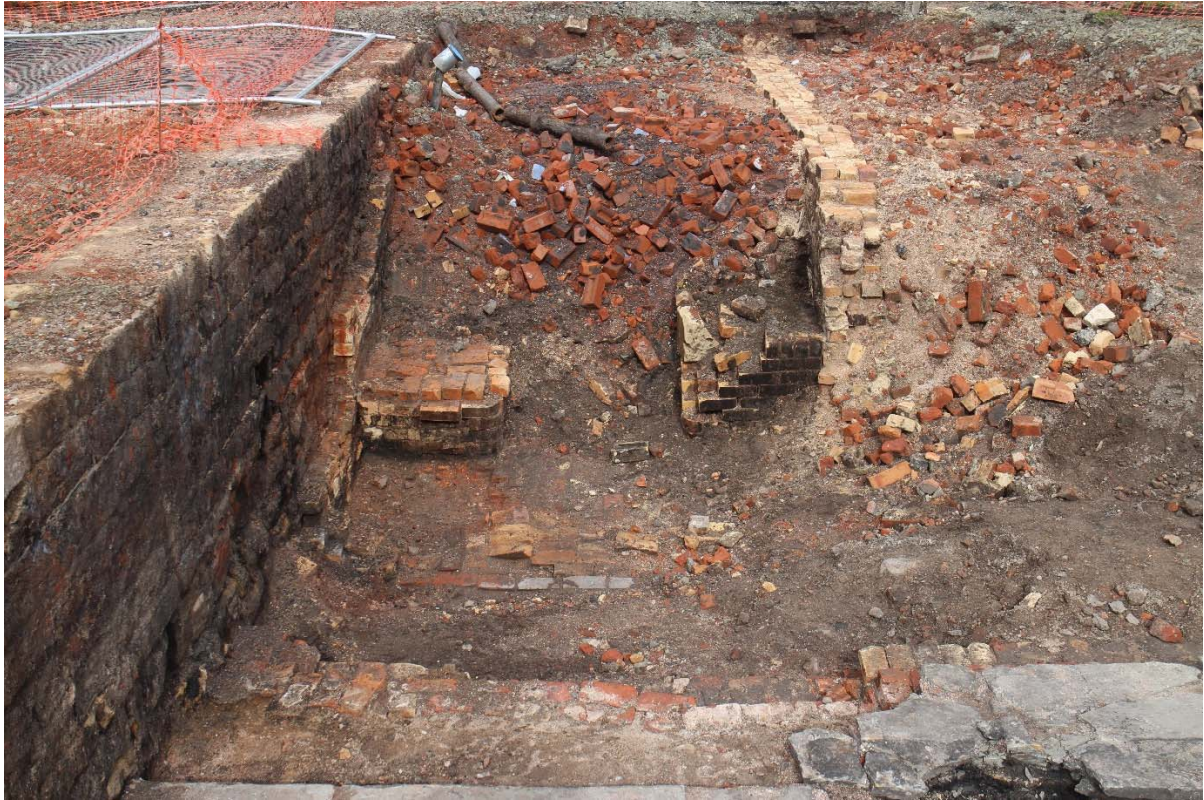
Plate 8: The supporting boiler plinths in the western boiler house bay.
