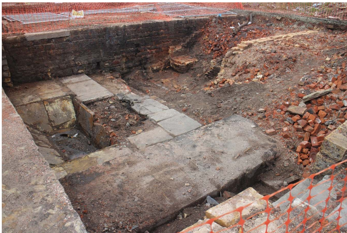
Plate 6: Room 1004 , viewed facing north-west, with main mill wall (bottom left), the eastern boundary wall and stepped access (bottom right), flagstone floor and boiler bays (centre), and dividing wall and room 1005 (background)
