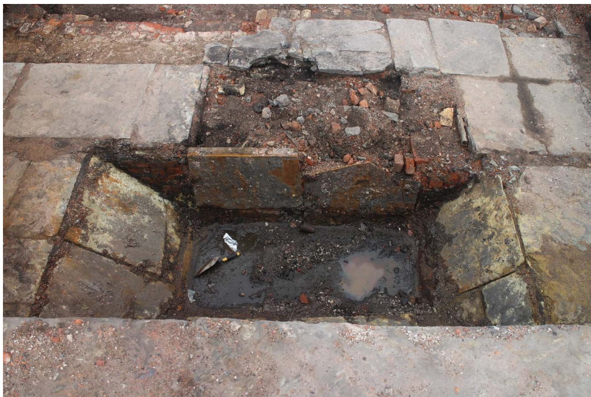
Plate 9. Detail of the sunken coal hopper within room 1004 of the boiler house. Viewed facing north
