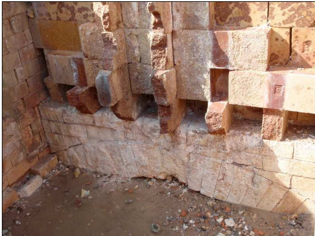
Plate 73: Regenerative blocks within furnace 305, some bearing an inverted '5' stamp (right)
