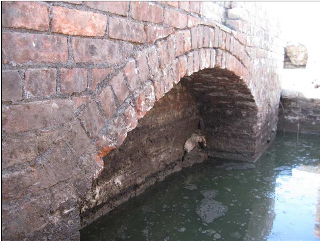
Plate 42: Relieving arch in north wall of 257
