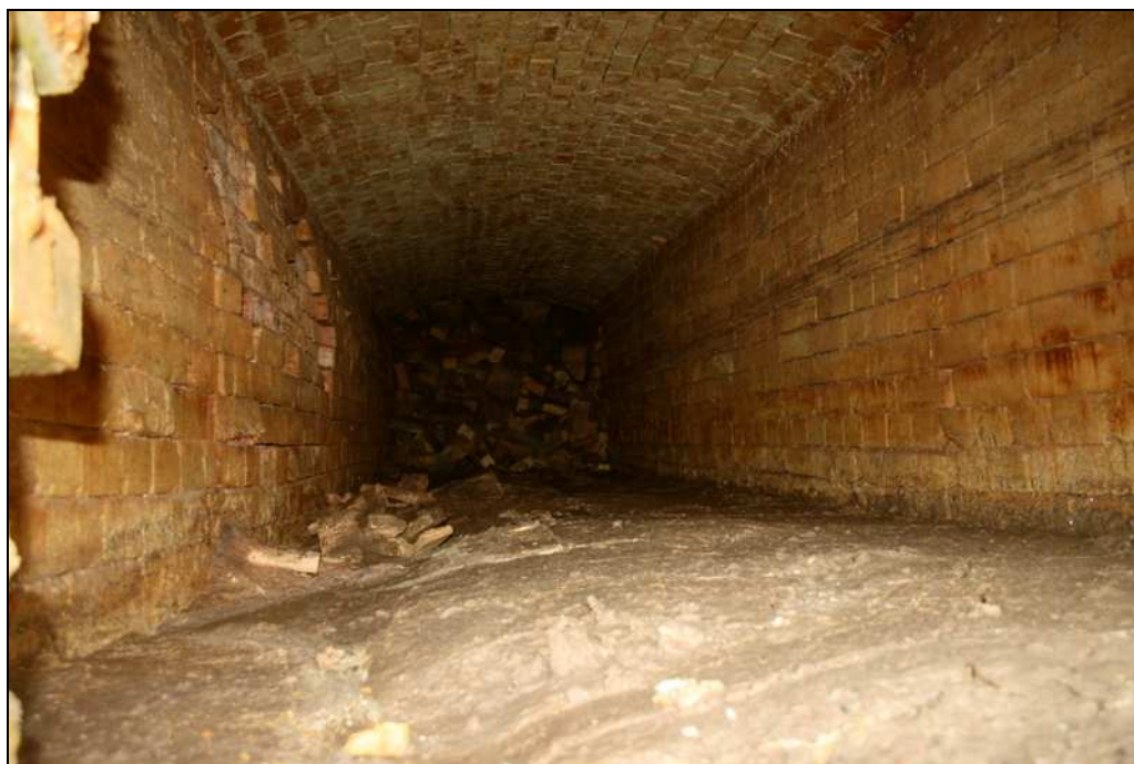
Plate 66: Interior of flue 263, with vertical opening above brick blocking at rear
