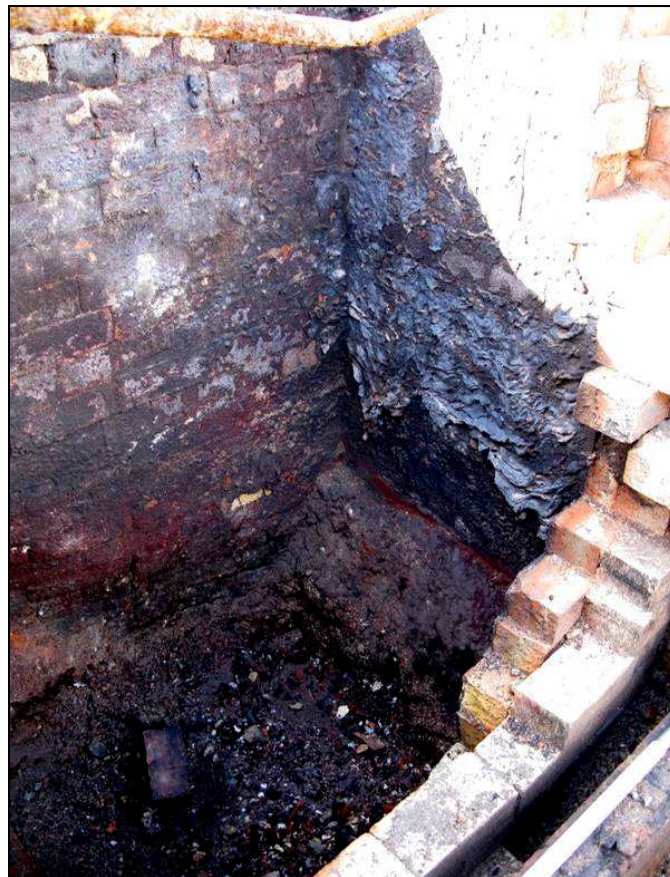
Plate 47: Interior of gas producer 258, with tarring of side walls and ash deposit in base
