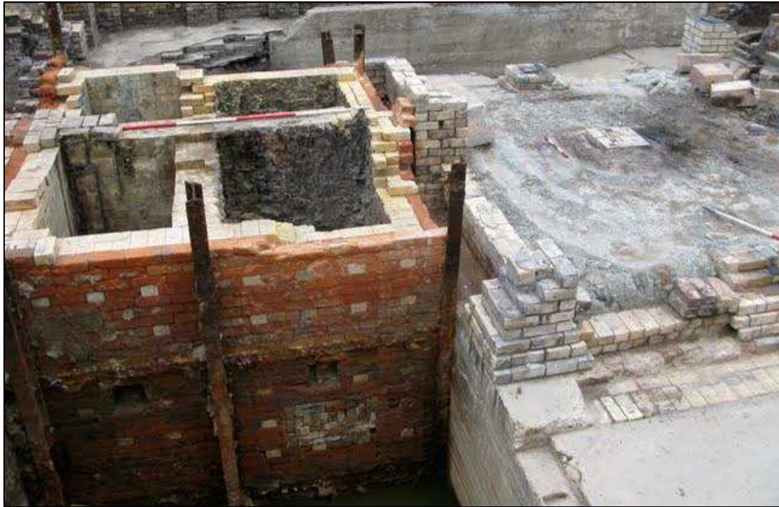
Plate 51: Recuperative stack, 232, on west side of Pyrex furnace
