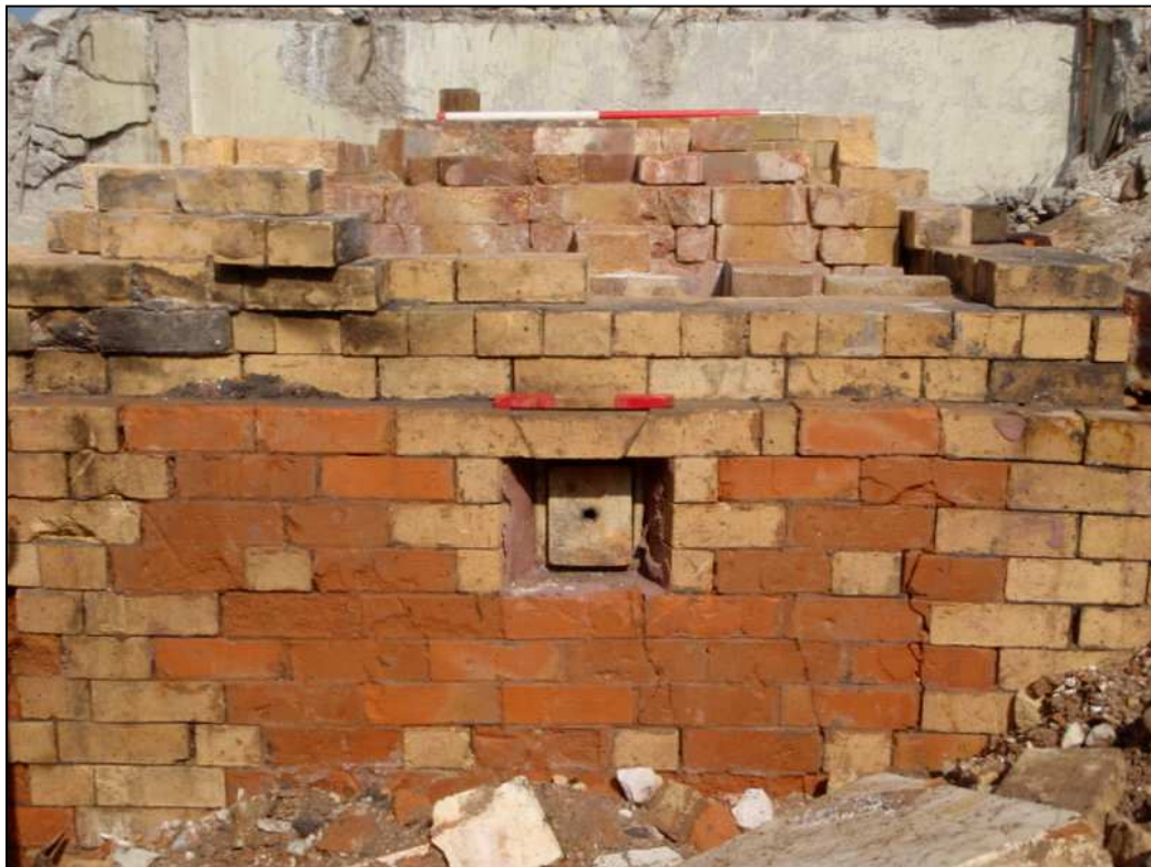
Plate 75: Removable block in the upper south wall of regenerative furnace 305
