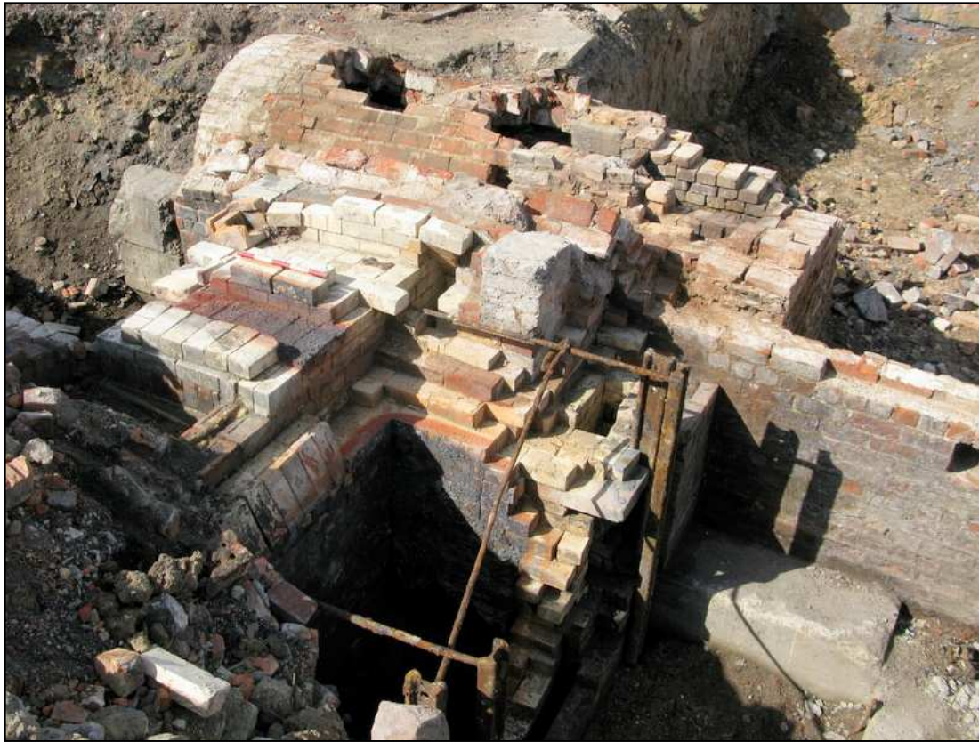
Plate 46: Gas producer 227, in south-eastern section of Area 2
