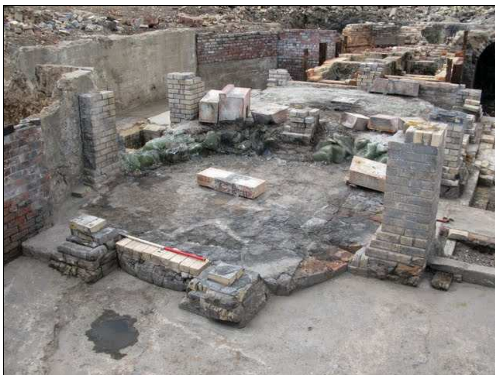
Plate 48: Columns supporting the tank of the Pyrex furnace
