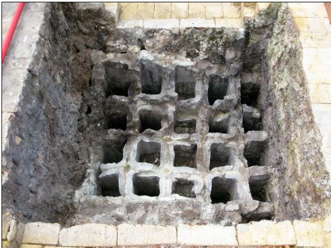
Plate 52: Detail of recuperator tubes
