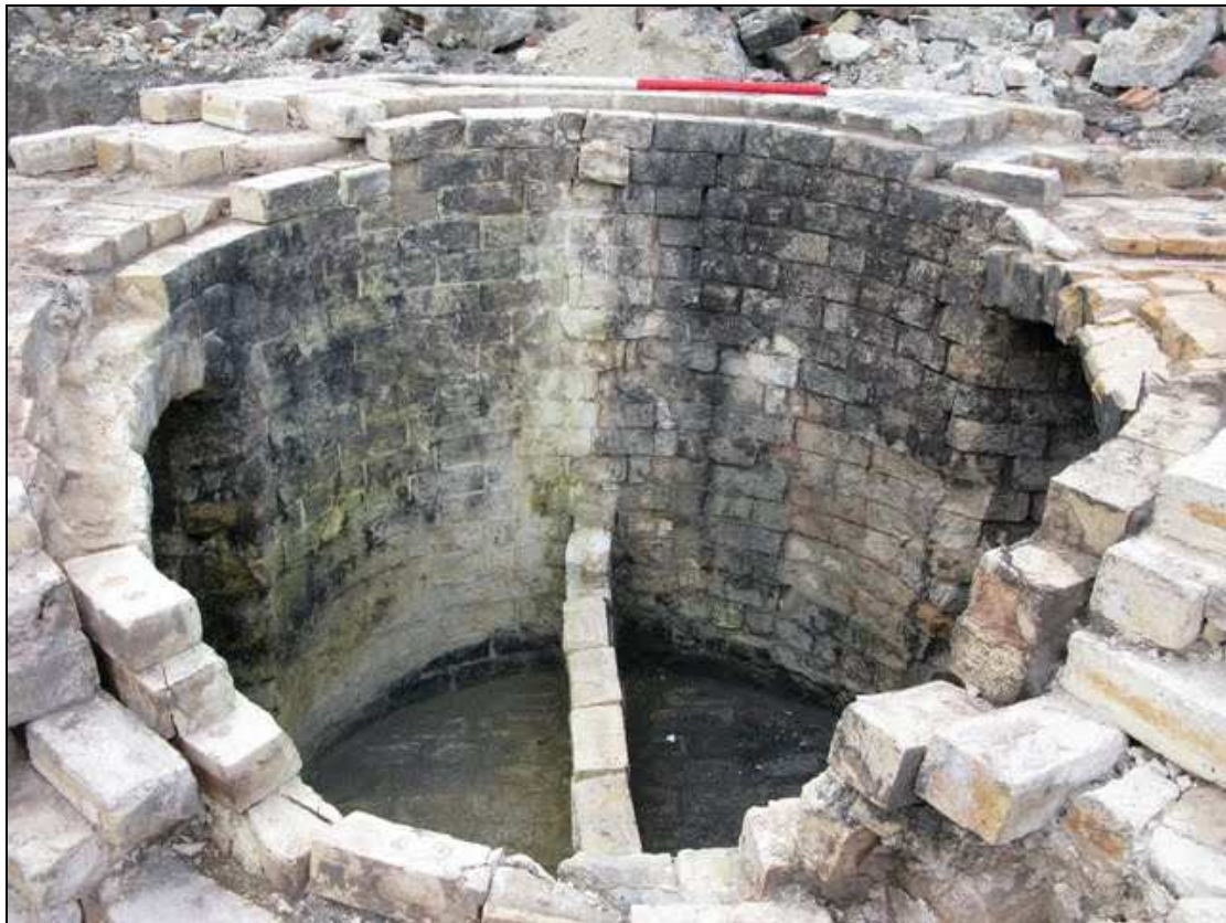
Plate 56: Dividing wall within base of chimney 213
