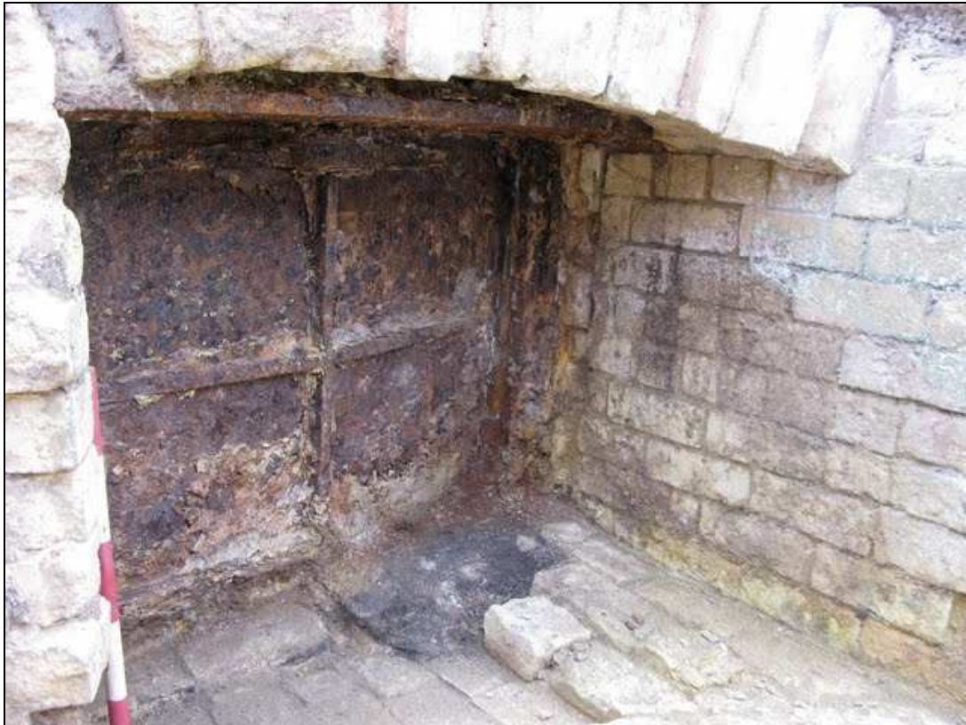
Plate 60: Probable butterfly valve extant within flue 261
