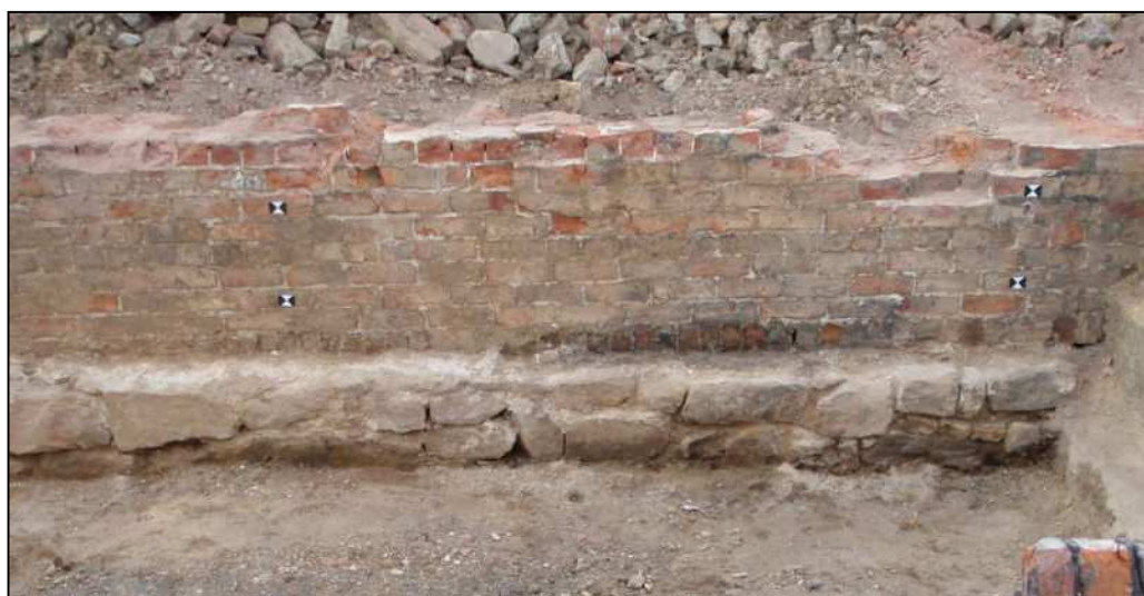
Plate 68: The fabric of wall 303, showing the sandstone plinth
