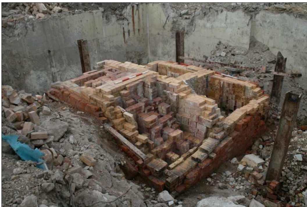
Plate 72: Detail of regenerative furnace 305
