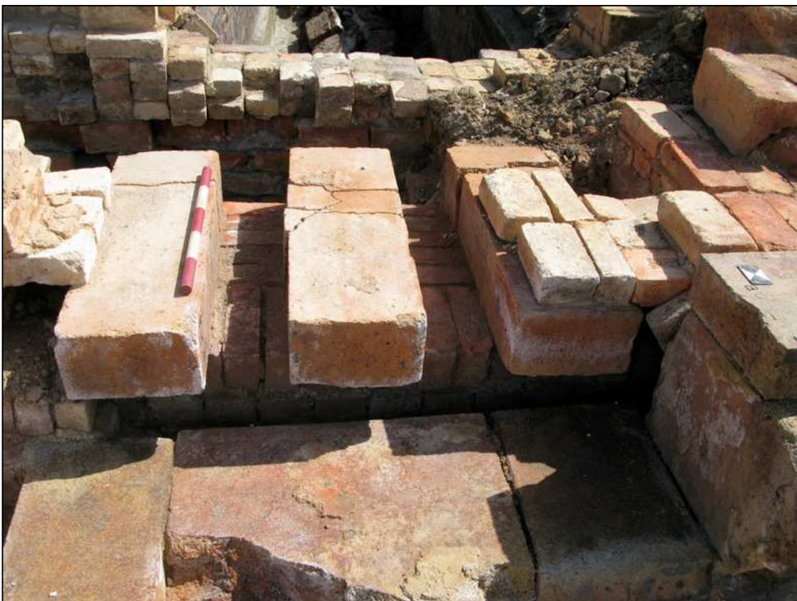
Plate 36: Large refractory blocks forming the end-wall of the tank of the Siemens-type furnace
