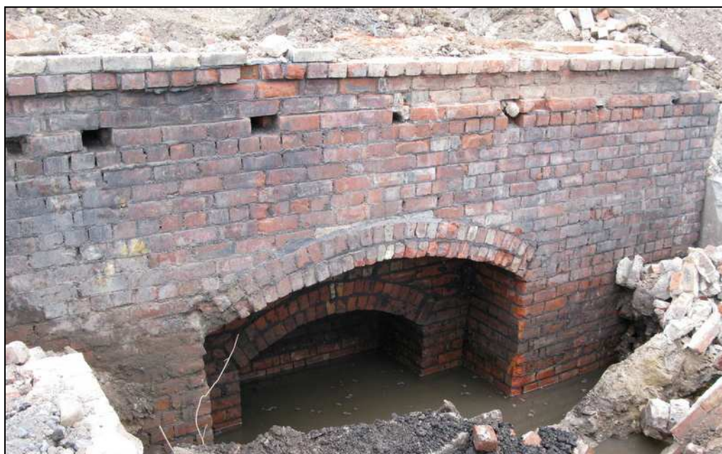
Plate 45: West wall of furnace 258, with central arched aperture and joist sockets above
