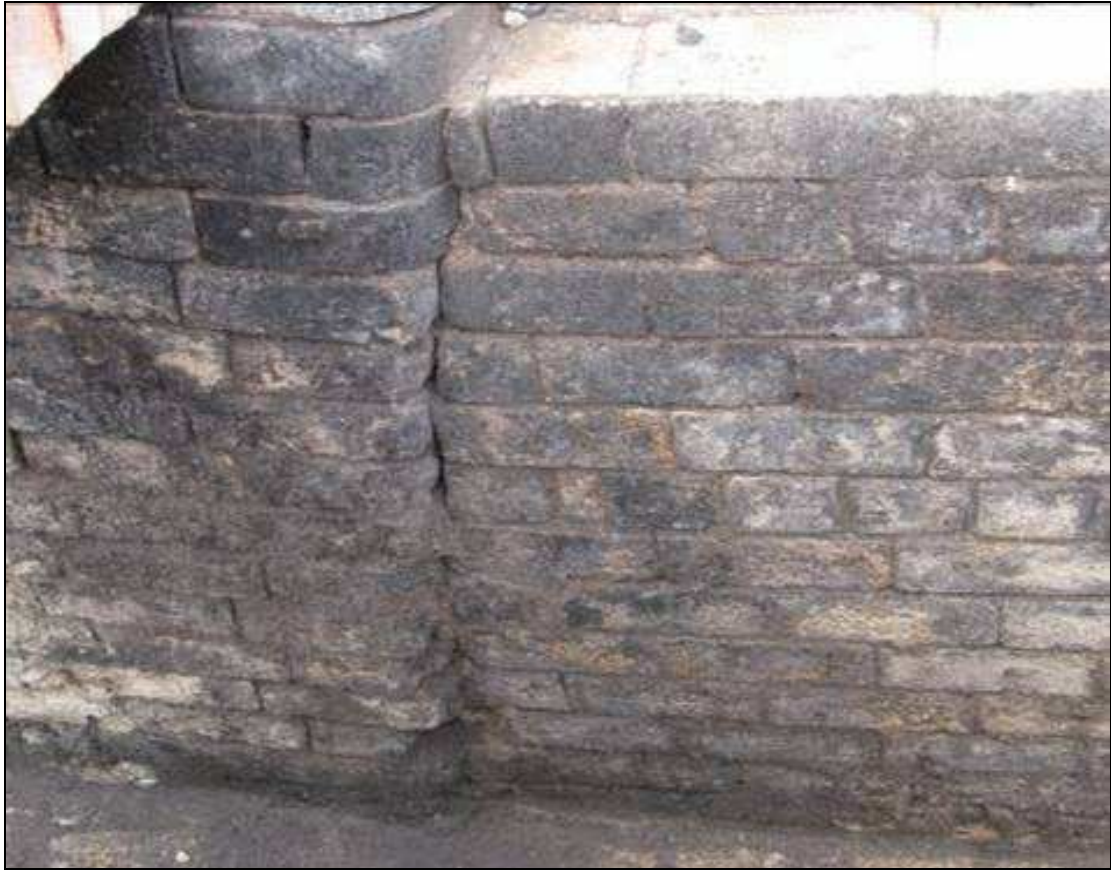
Plate 55: Butt joint between flue 214 and chimney 213
