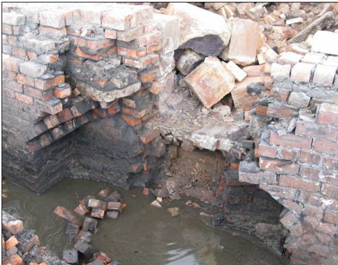
Plate 43: Bottom block of tank furnace behind relieving arch in north wall of 257
