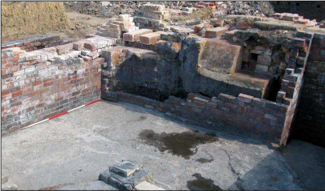
Plate 35: Remains of the Siemens-type furnace
