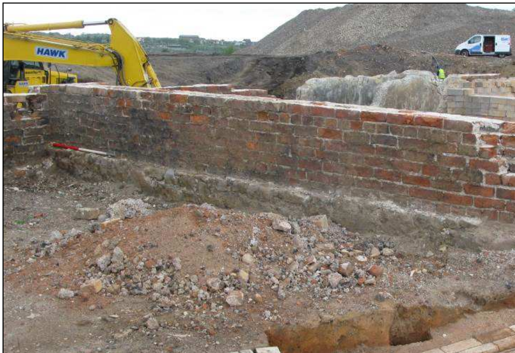
Plate 26: Typical section of Phase 1 wall (246), comprising bricks laid on a stone plinth
