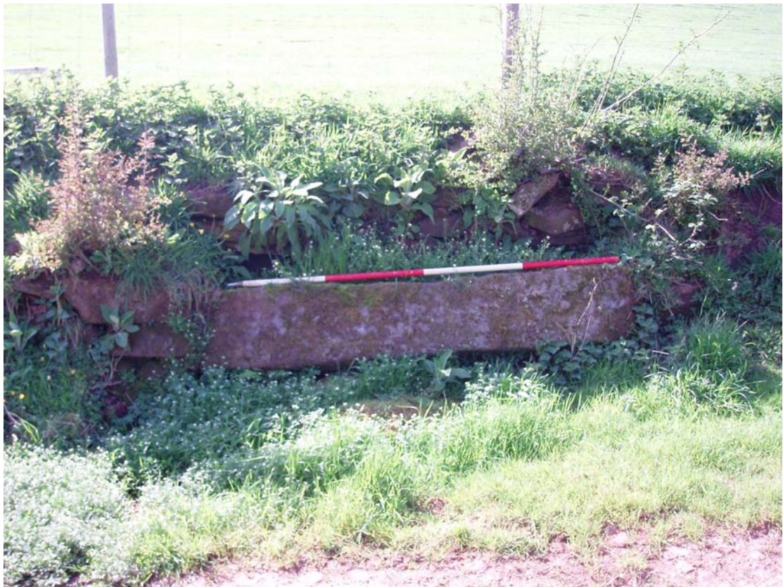
Plate 4: Gate post built into a St Bees-type wall (Site 27 )
