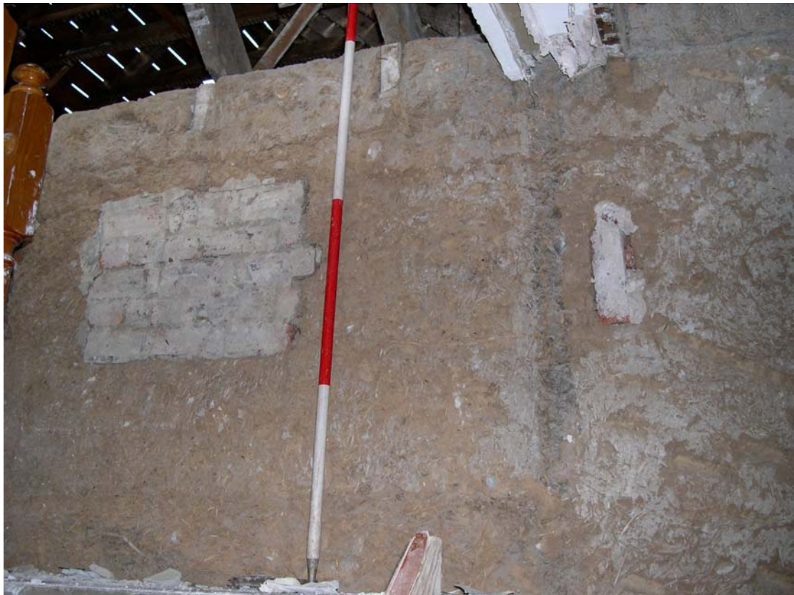
Plate 25: Blocked apertures in north internal elevation, D3
