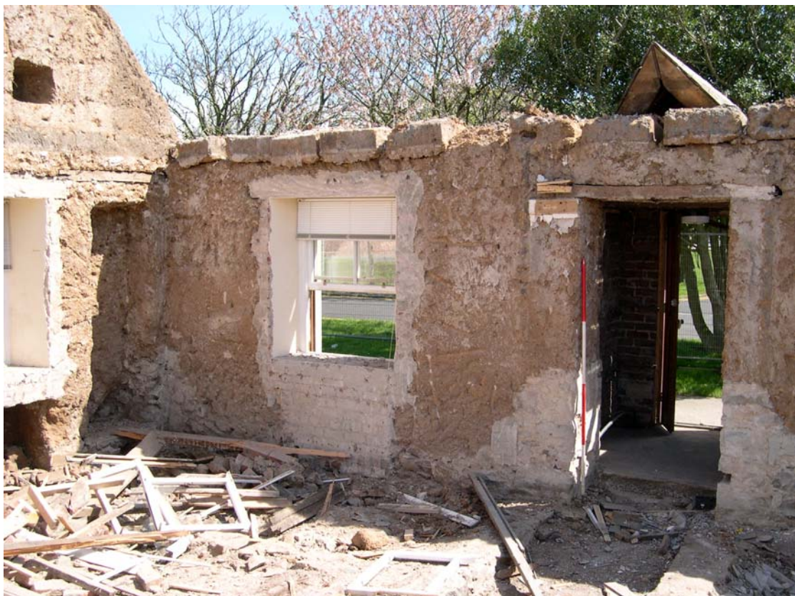
Plate 20: Detail of clay-wall construction, D3
