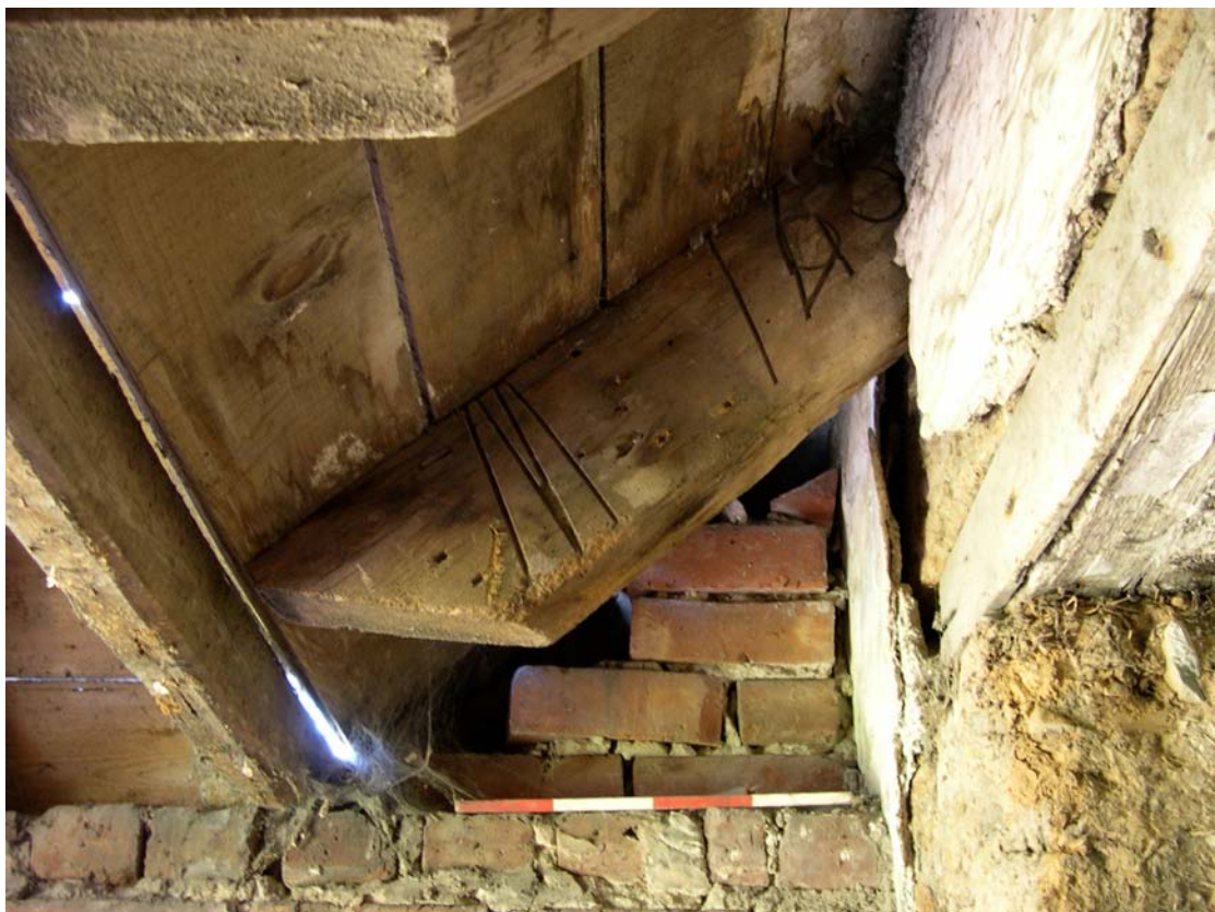
Plate 26: Baltic timber mark in-situ , D3
