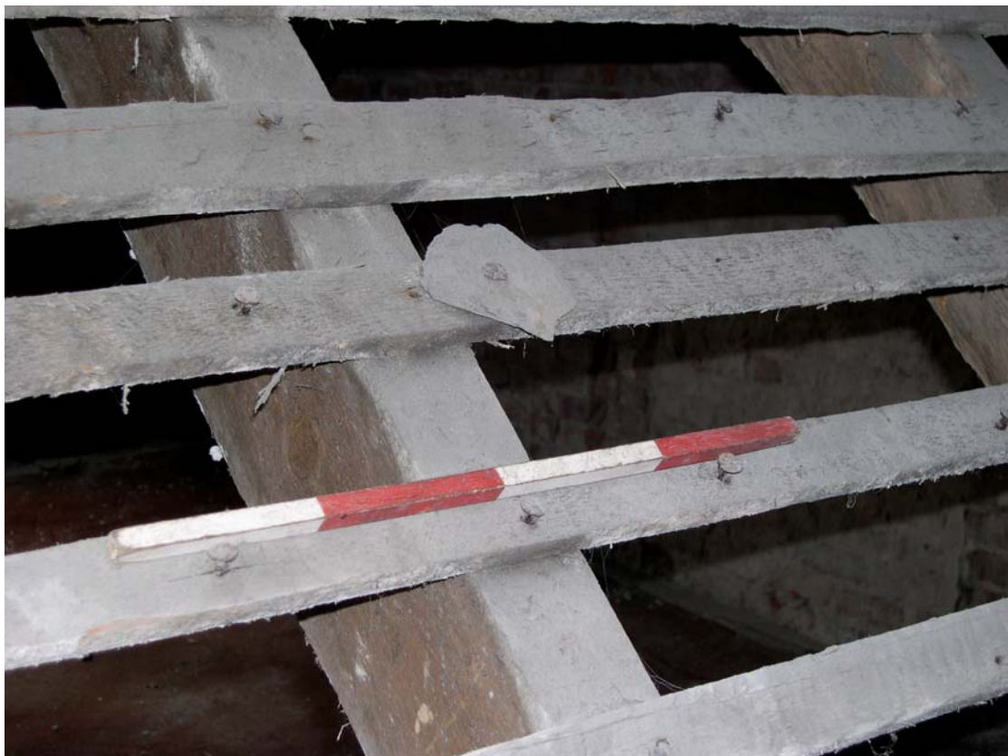
Plate 28: In-situ slate from original roof structure, D3
