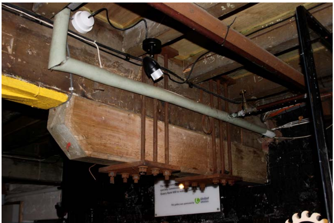
Plate 56: A timber corbel has been inserted under the eastern side of the beam, supported by tie-rods
