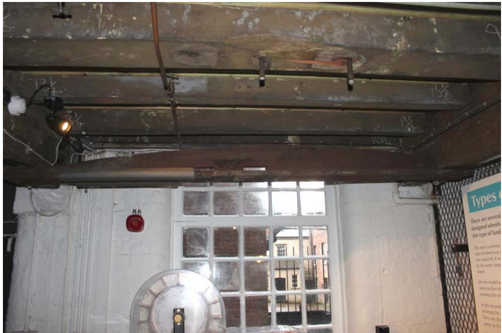
Plate 54: Each bay has 20-light timber windows, including tilting top rows
