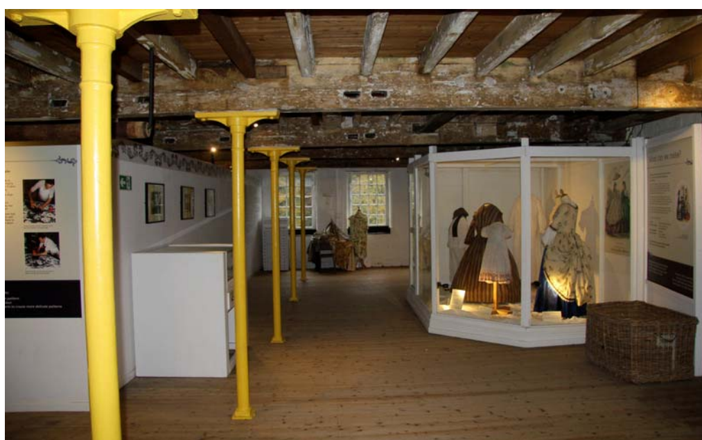
Plate 61: The second floor of the New Mill is carried by six north/south-aligned beams, supported by cast-iron columns similar to those on the other floors
