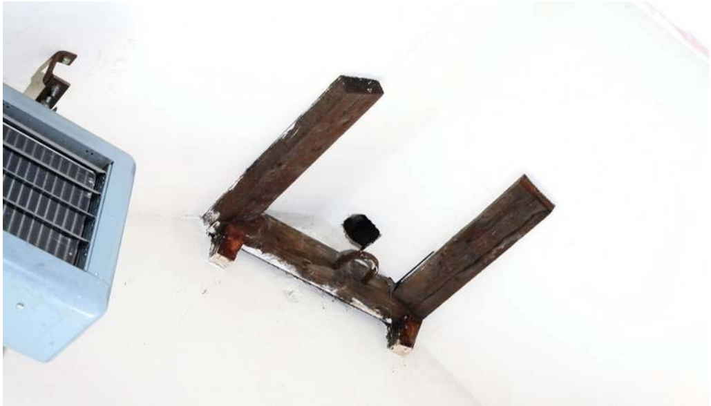
Plate 72: Back plate mounting for an external flagpole on the eastern facade
