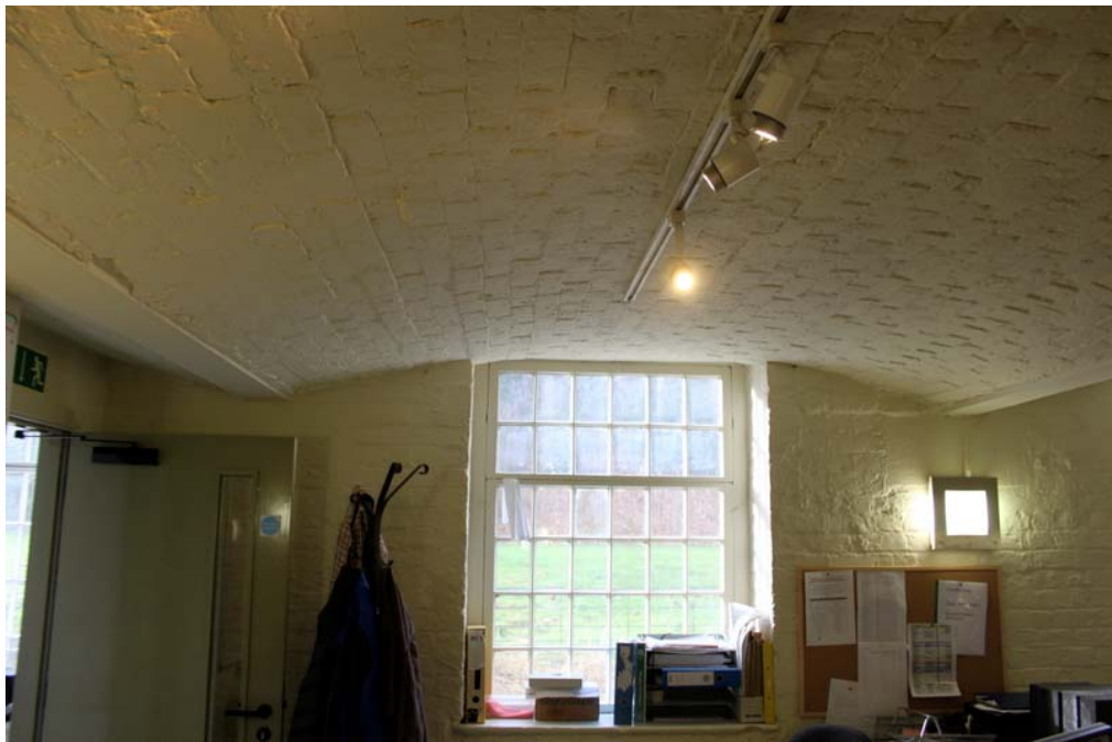
Plate 125: The exposed brick vaulting without tie-rods in the Lower Ground Floor
