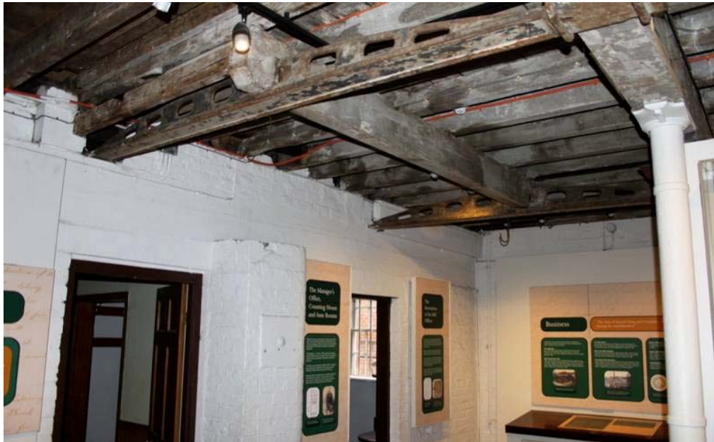
Plate 79: Two cast-iron, open-web, whale-backed T-section beams span from the south-west wall to the adjacent ceiling beam
