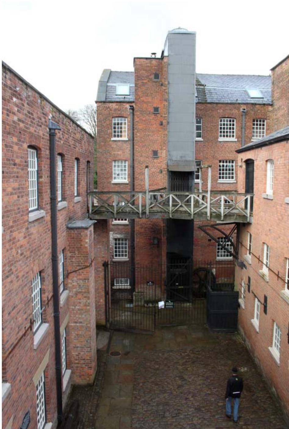
Plate 53: The south wall of the New Mill with privy and hoist towers
