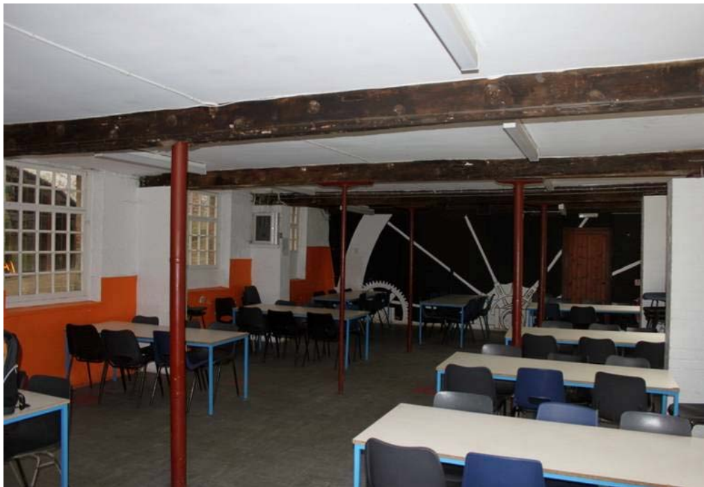
Plate 118: The original timber beams in the southern five bays of the weaving block, supported by later reused columns
