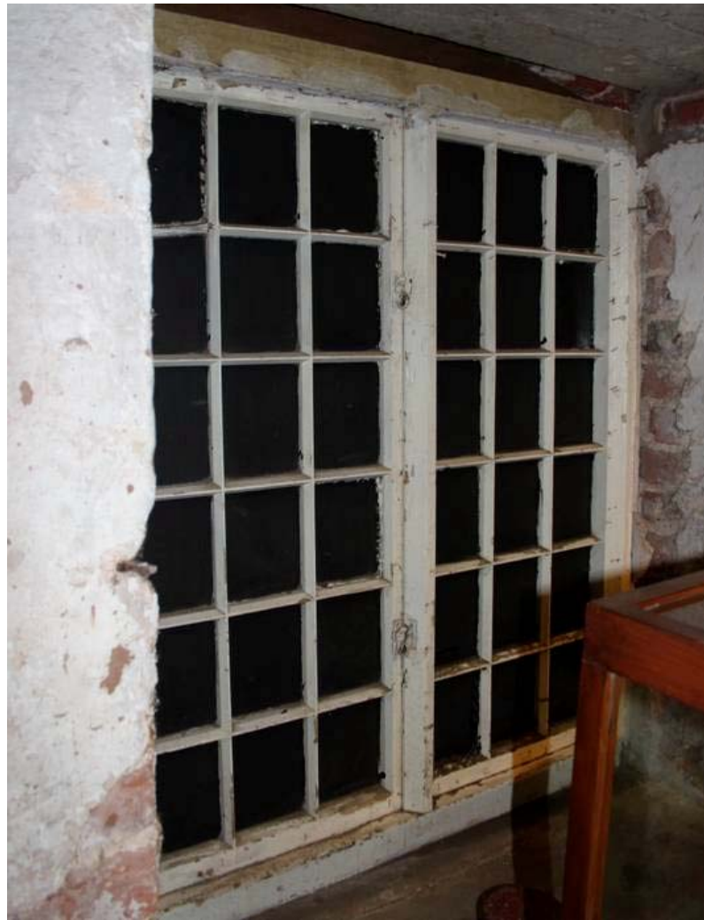
Plate 15: 36-light casement window, which was possibly a survival of the original fenestration
