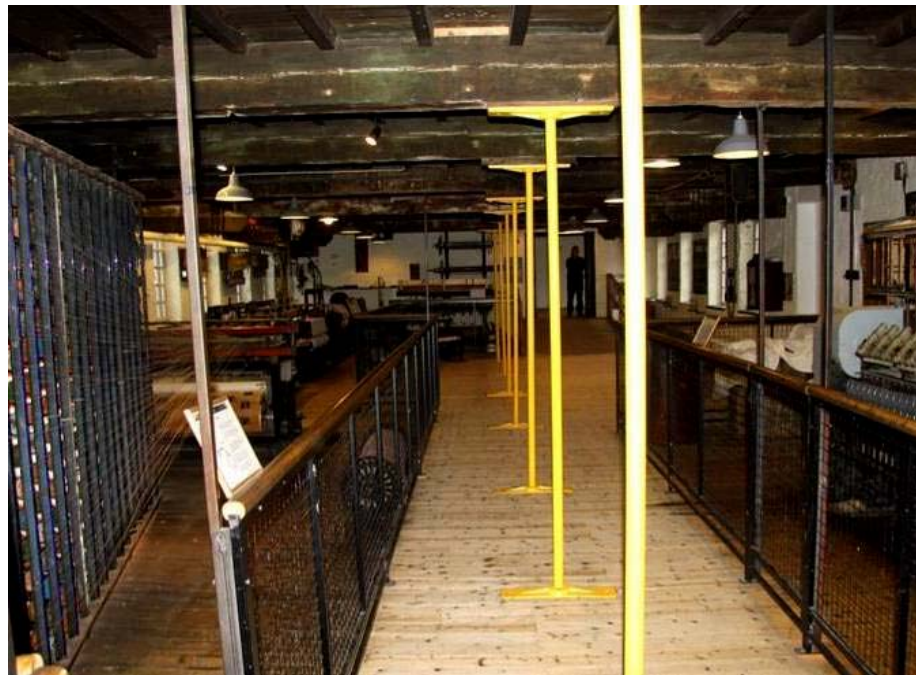
Plate 36: Cast-iron columns on second floor of Old Mill
