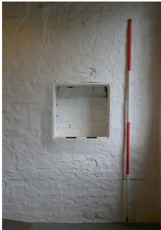
Plate 41: Square cast-iron frame, possibly used for fire fighting equipment
