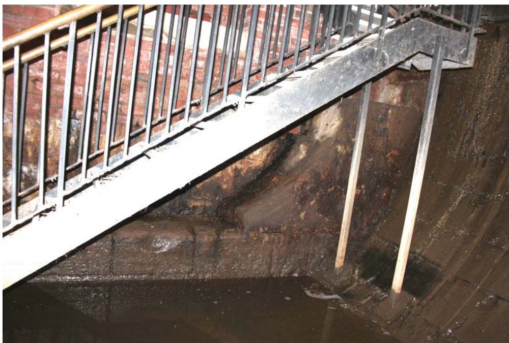
Plate 20: Extant ashlar block side walls
