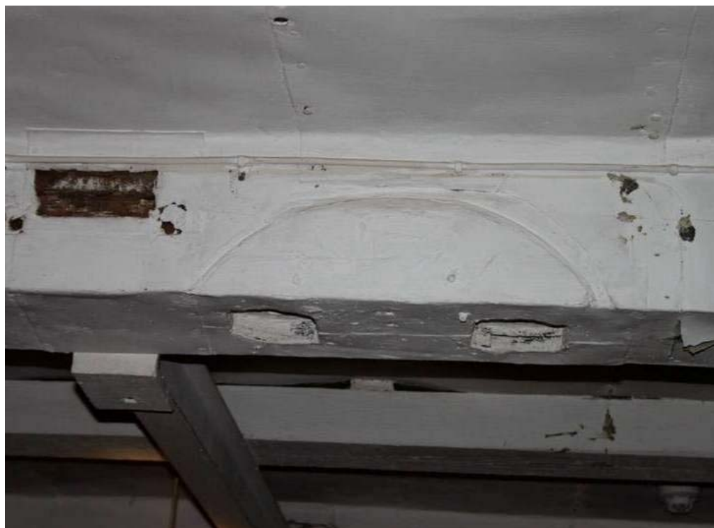
Plate 31: Gouged drum scars on the beam faces, indicating position line shaft
