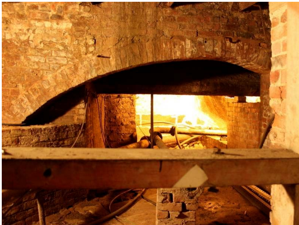
Plate 18: Large flagged chamber beneath the stair tower giving access to the headrace tunnel
