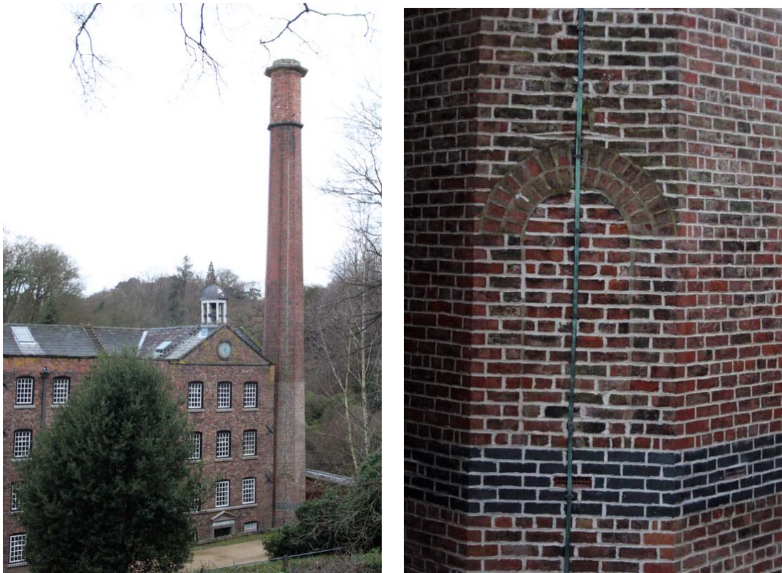
Plates 100 and 101: The octagonal brick chimney located in the re-entrant between stair tower and Old Mill. It has a brick-blocked arched access aperture at first-floor level on its eastern side (right)
