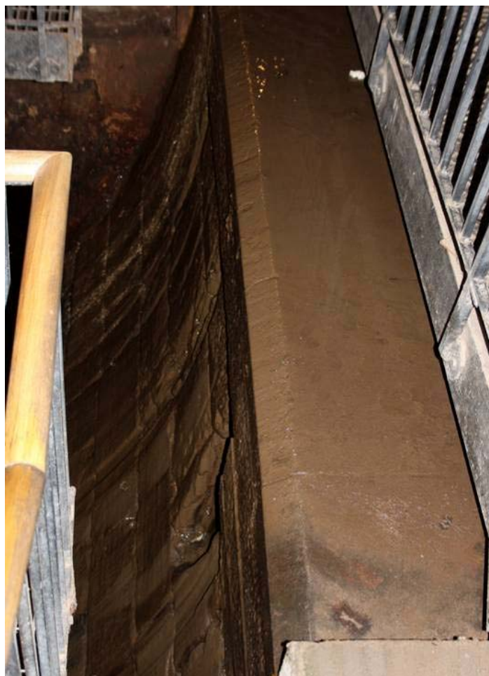
Plate 19: Ashlar block wheel pit
