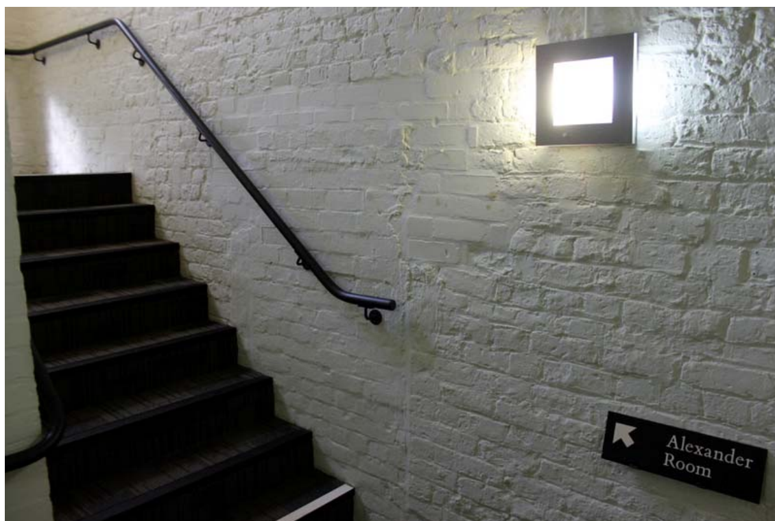
Plate 128: A brick-blocked doorway at ground-floor level
