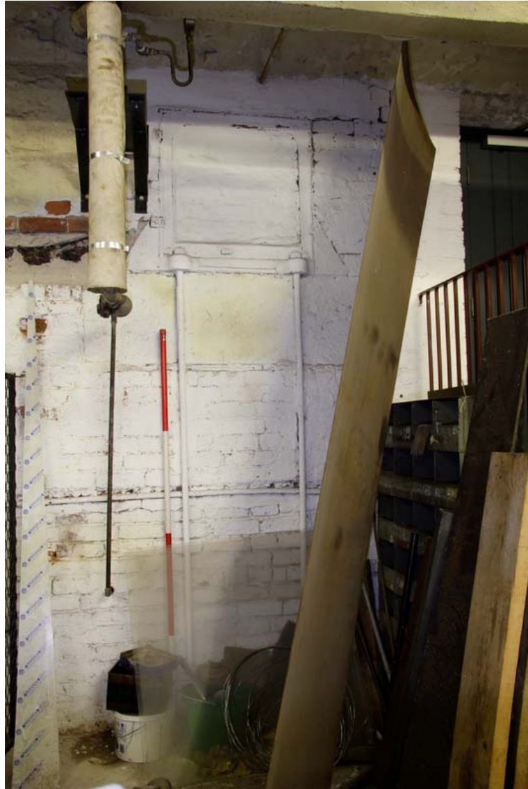
Plate 114: A blocked cast-iron bearing in the northern wall
