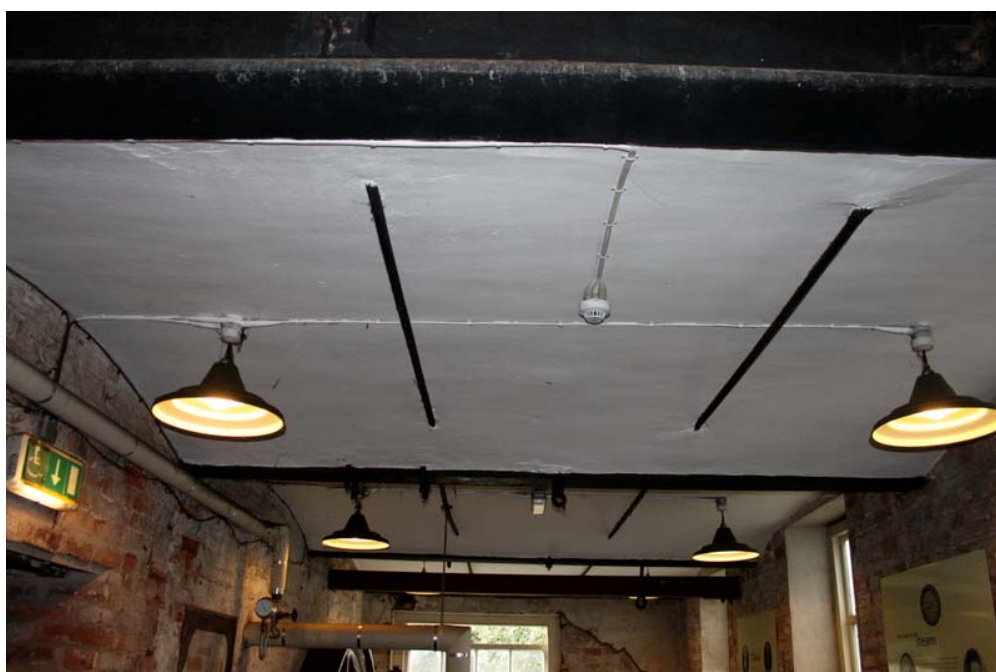
Plate 93: The cast-iron T-section beams braced by tie rods
