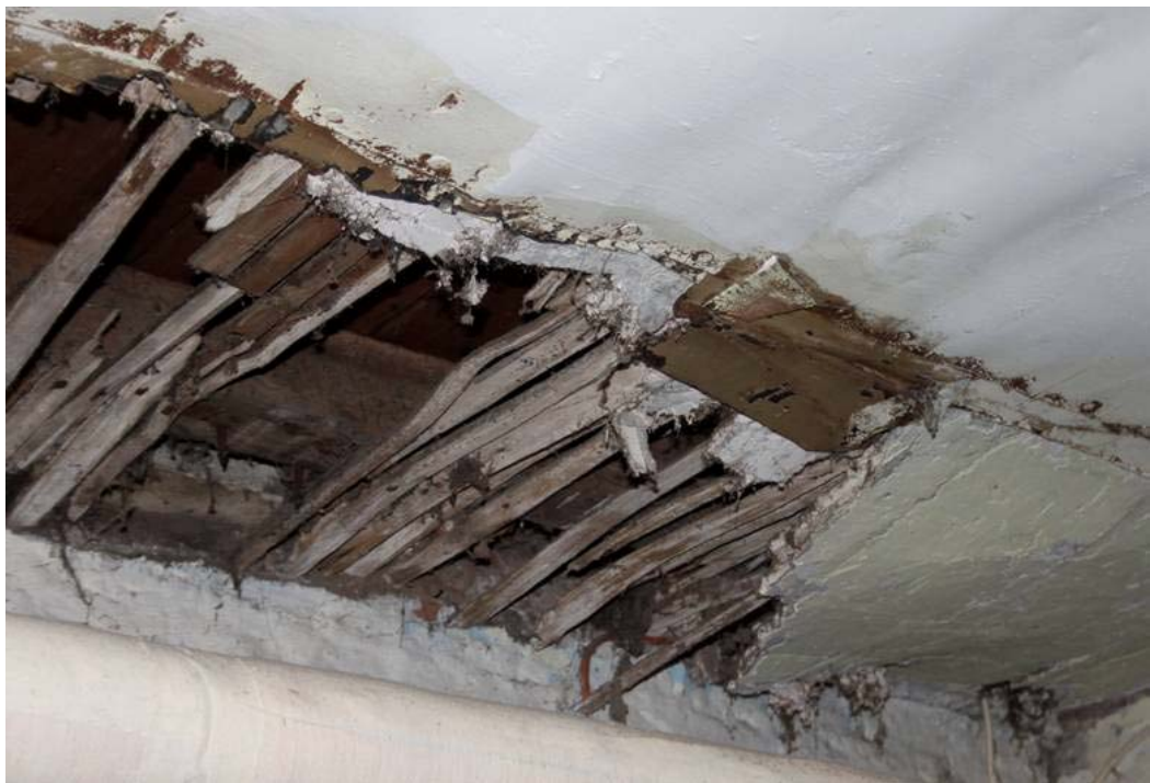
Plate 28: Extant lath and plaster ceiling
