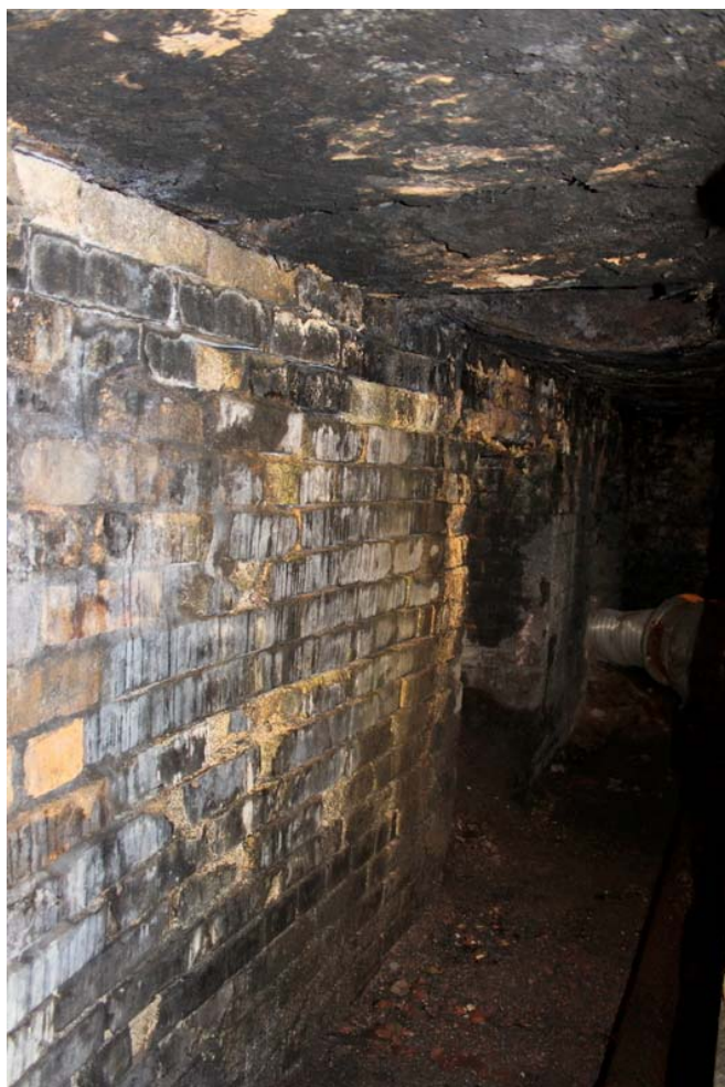
Plate 99: A refractory-lined flue leading to the chimney
