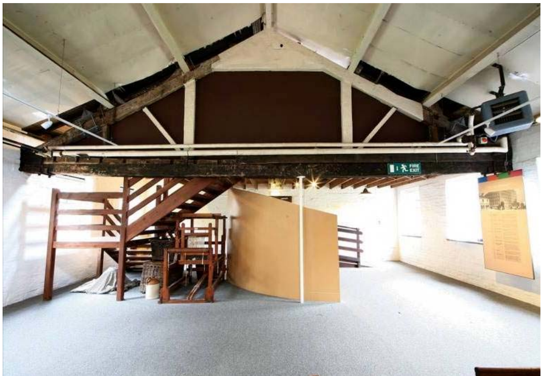
Plate 40: Queen strut truss with metal sheet cladding forming basic fire proofing
