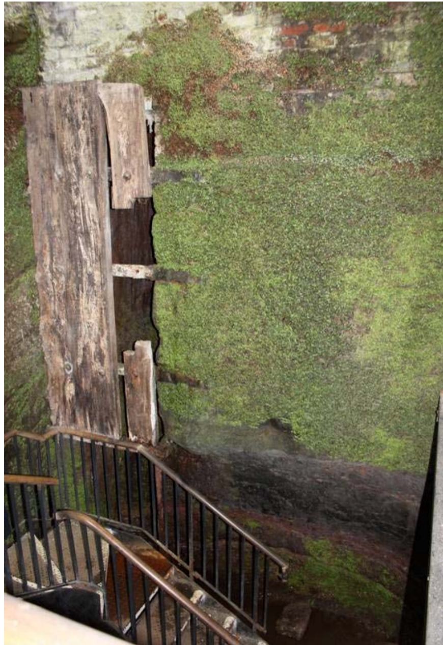
Plate 105: The east wall of the extended boiler house, cut through bedrock, had a vertical coal chute shuttered with timbers
