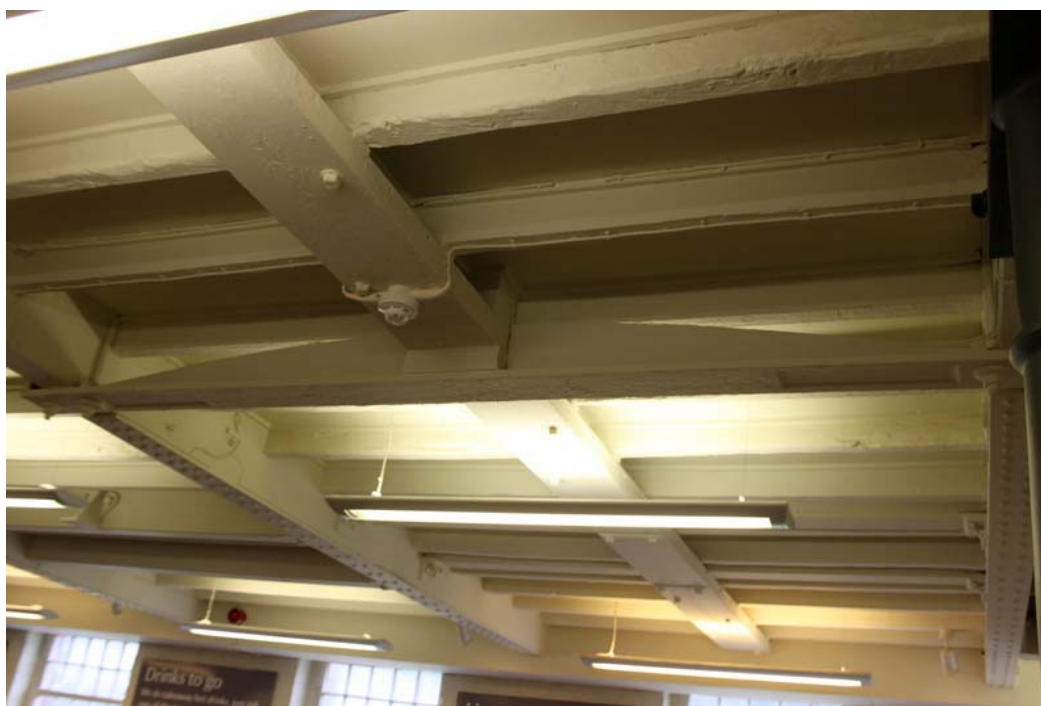
Plate 131: The southern bay is spanned by a whale-backed, T-section beam at ground-floor level
