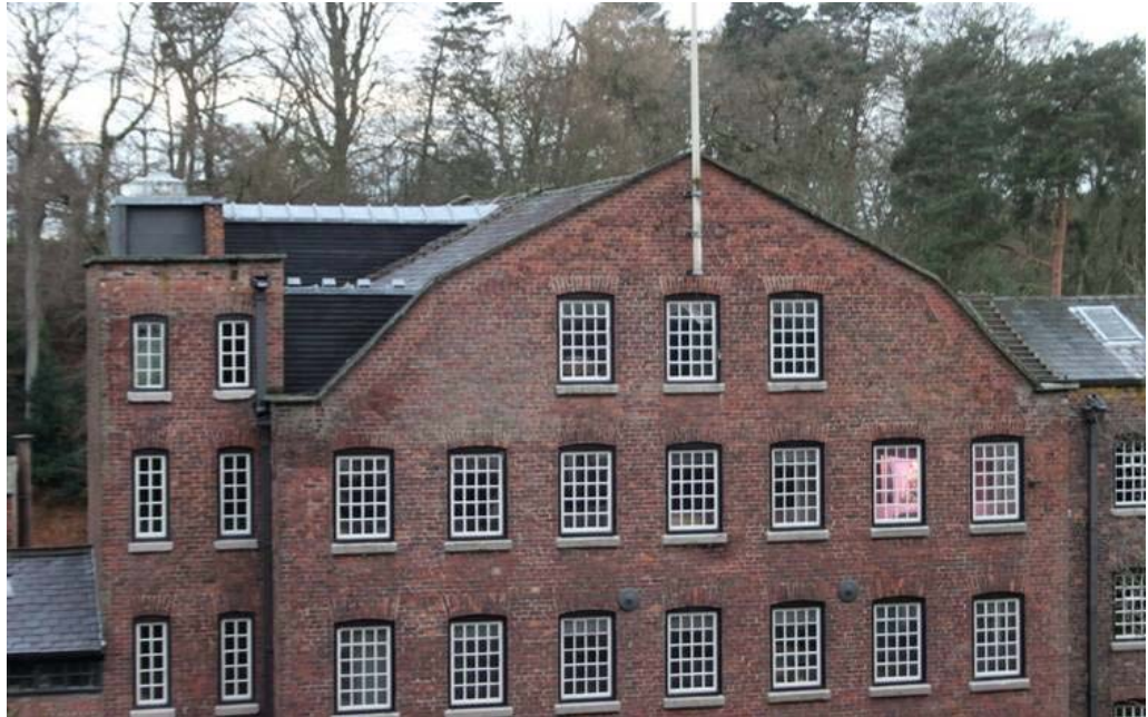
Plate 51: The gable elevation of the New Mill, with mansard roof, has similar windows to those of the Old Mill, with one in each of the seven bays apart from the upper floor
