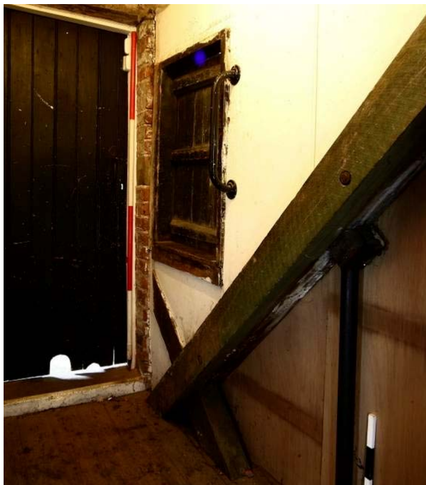
Plate 66: A timber hatch in the passageway of the upper floor of the New Mill, which provides access to the roof
