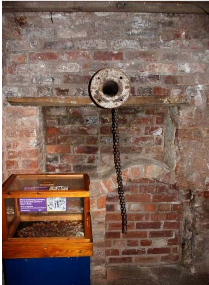
Plate 14: A water pipe, inserted through the wall above blocked aperture
