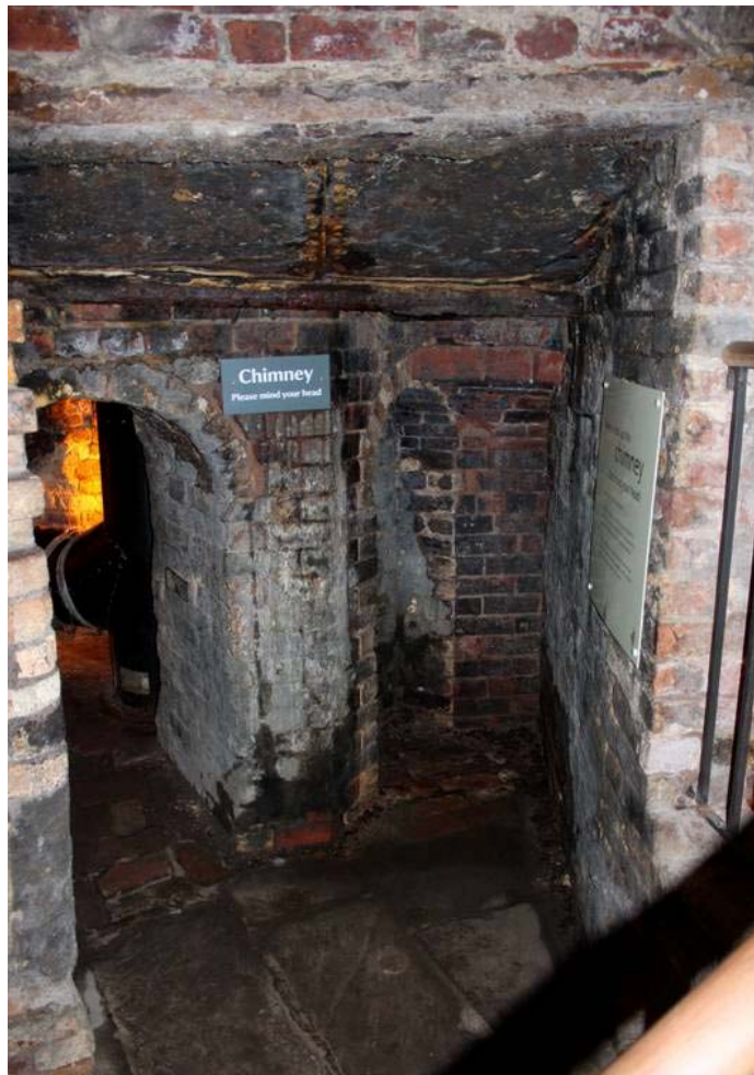
Plate 102: The flues were fed by a wide aperture supported by a T shaped cast-iron lintel
