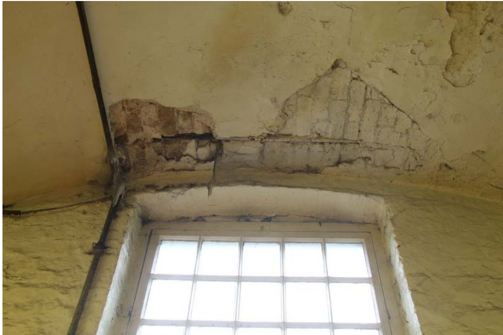
Plate 113: In the wider bays the tie rod was encased within the brickwork of the shallow vault
