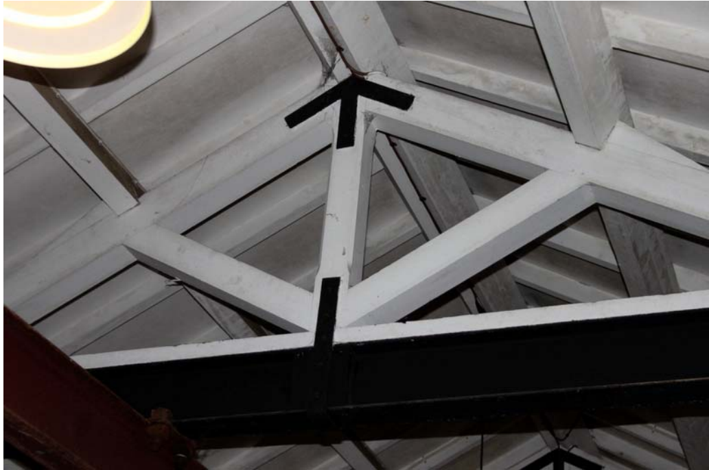
Plate 86: King post trusses, with iron stirrups, forming the hipped roof of the Engine House
