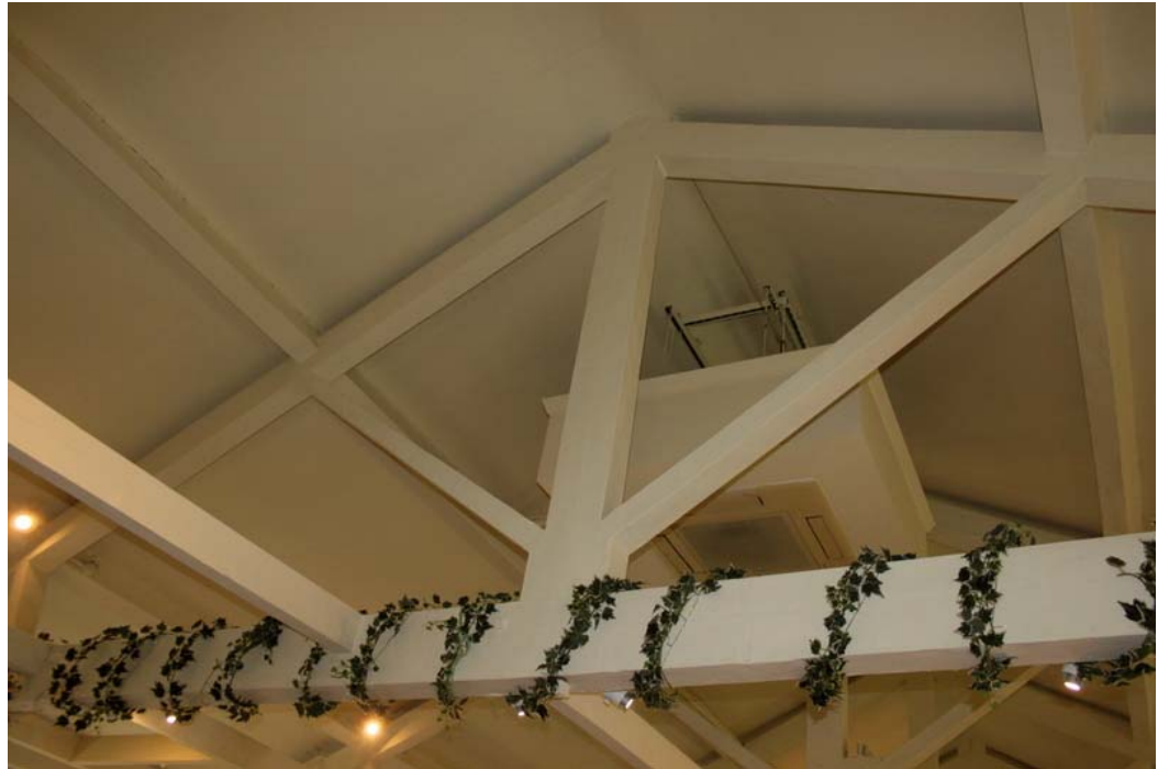
Plate 133: One of the king post trusses, with angled braces to the upper of the two trenched purlins
