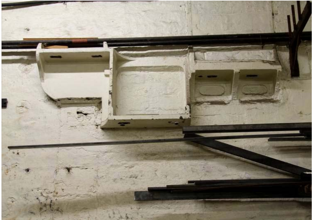
Plate 115: A large cast-iron bearing box and bracket in the south wall
