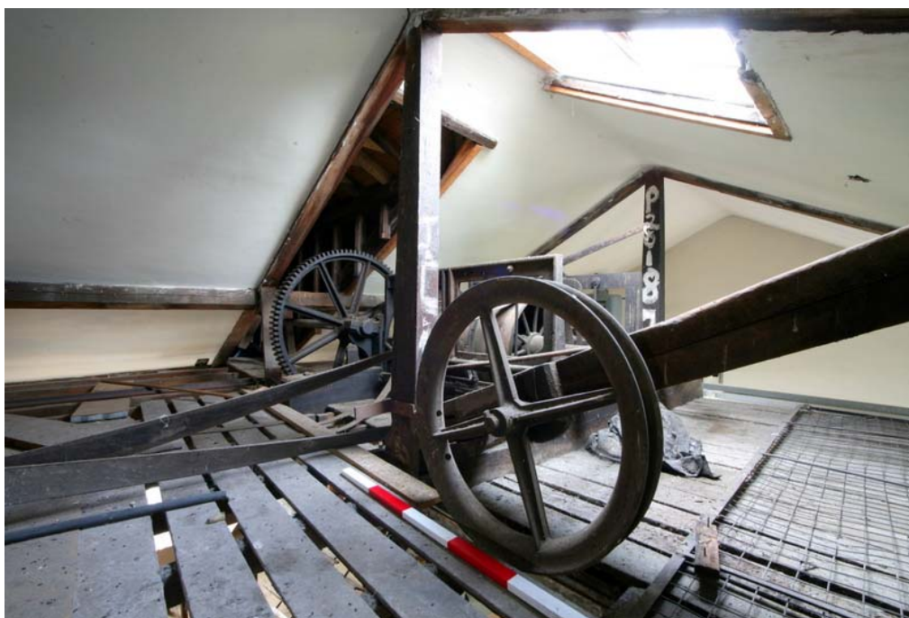
Plate 70: Headgear for the hoist tower in the fourth-floor loft
