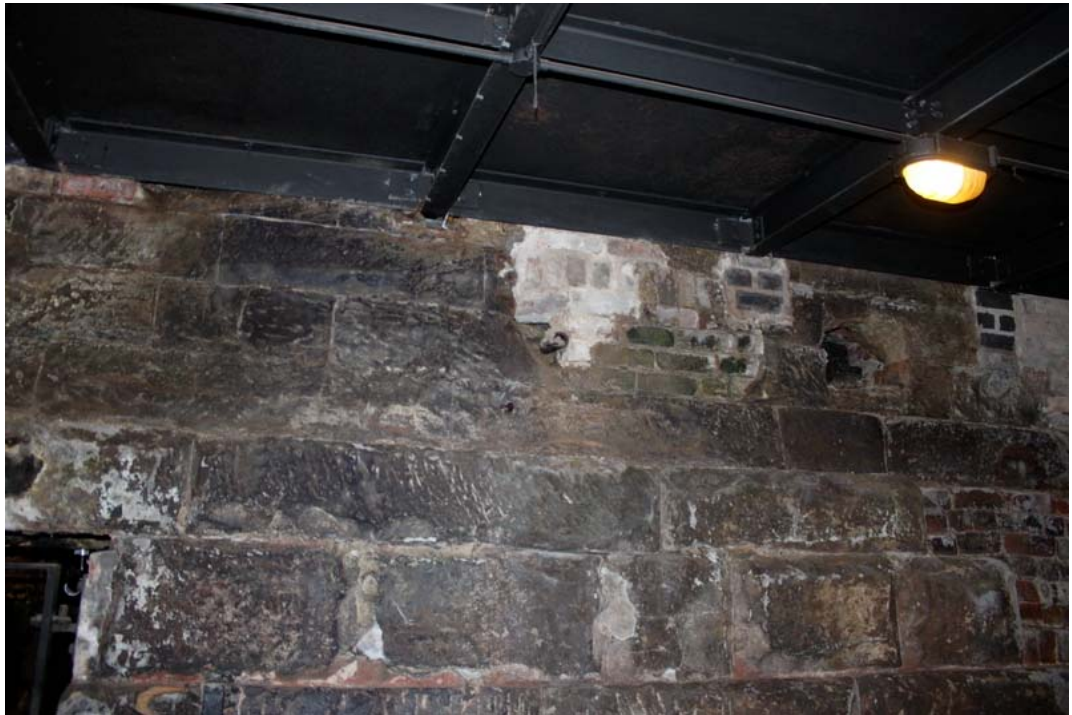
Plate 97: Substantial block work with a blocked semi-circular aperture
