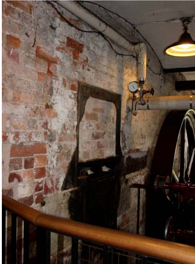
Plate 95: A large cast-iron bearing box possibly for the primary drive shaft
