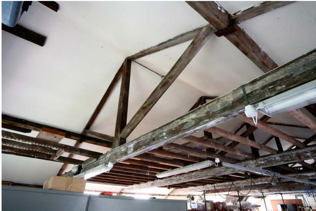
Plate 69: King post truss of the New Mill roof
