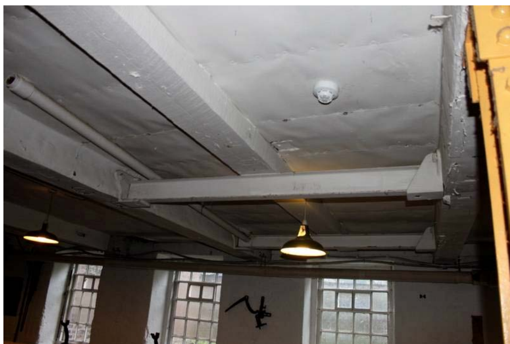
Plate 30: I-section beams, still present across the sixth, eighth and eleventh bays
