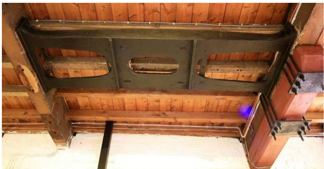
Plate 65: A large cast-iron bearing plate for an upright shaft at the northern end of the bay
