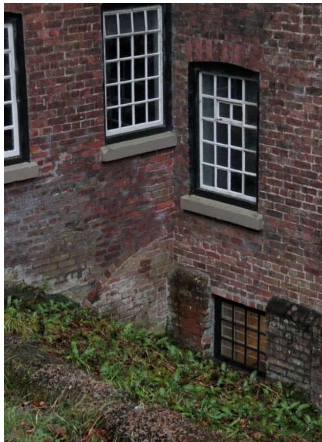
Plate 48: The blocked arched doorway at the re-entrant angle between the Old and New Mills that formerly accessed the wheel chamber
