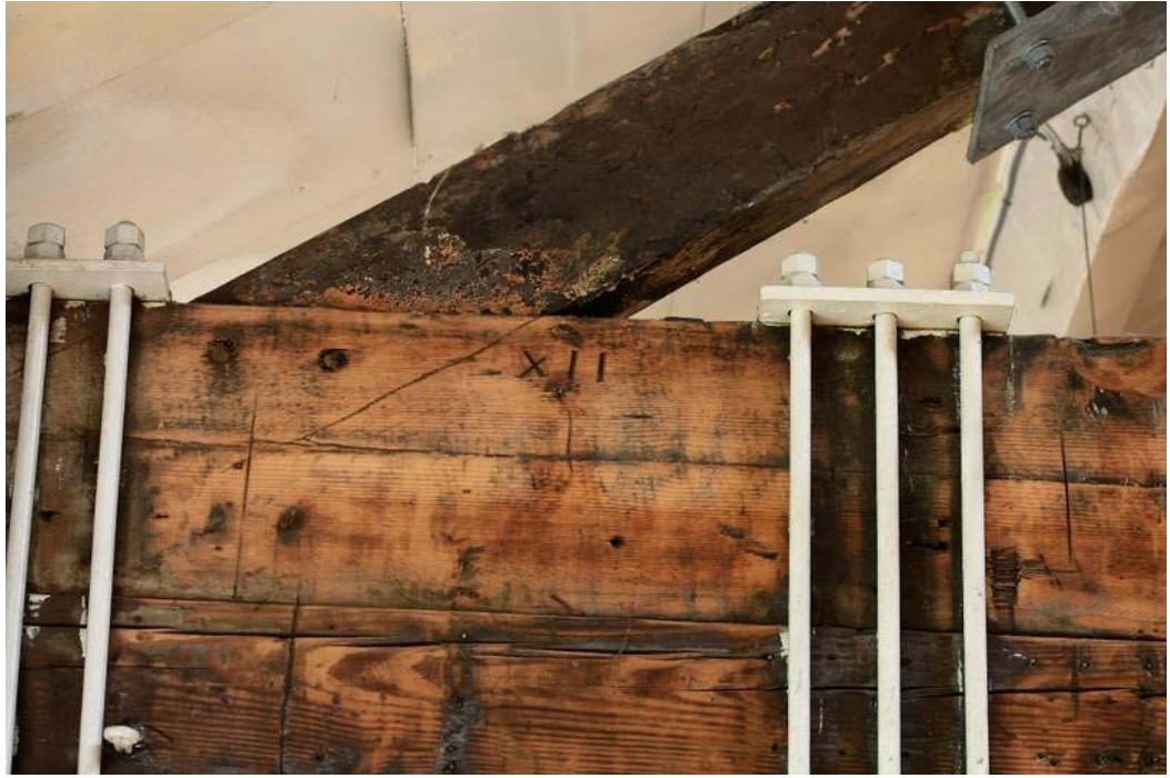
Plate 39: Chiselled numerals on the southern faces of the trusses
