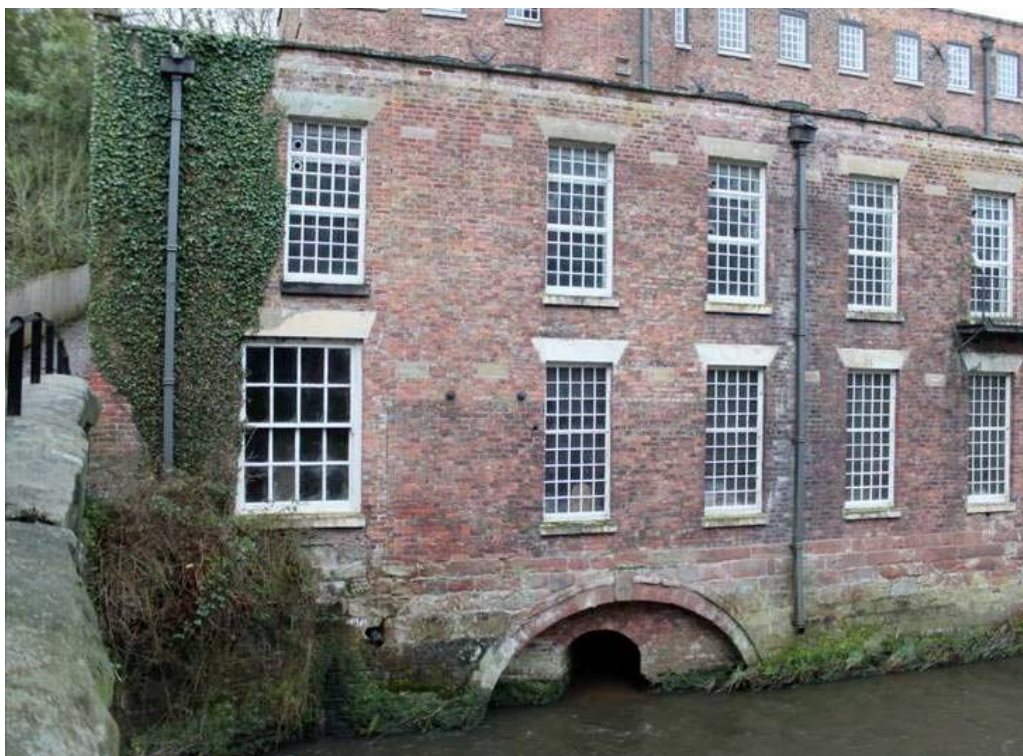
Plate 24: Arched outfall at the eastern end of the tailrace
