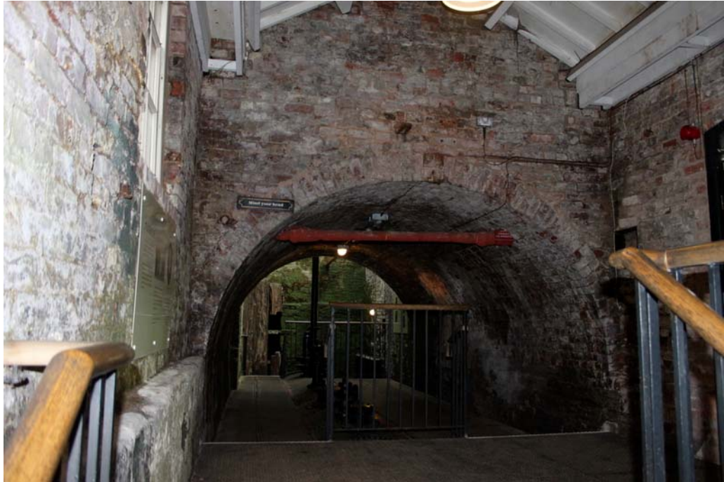
Plate 103: Site of the 1880 boiler in a barrel-vaulted brick chamber beneath the road
