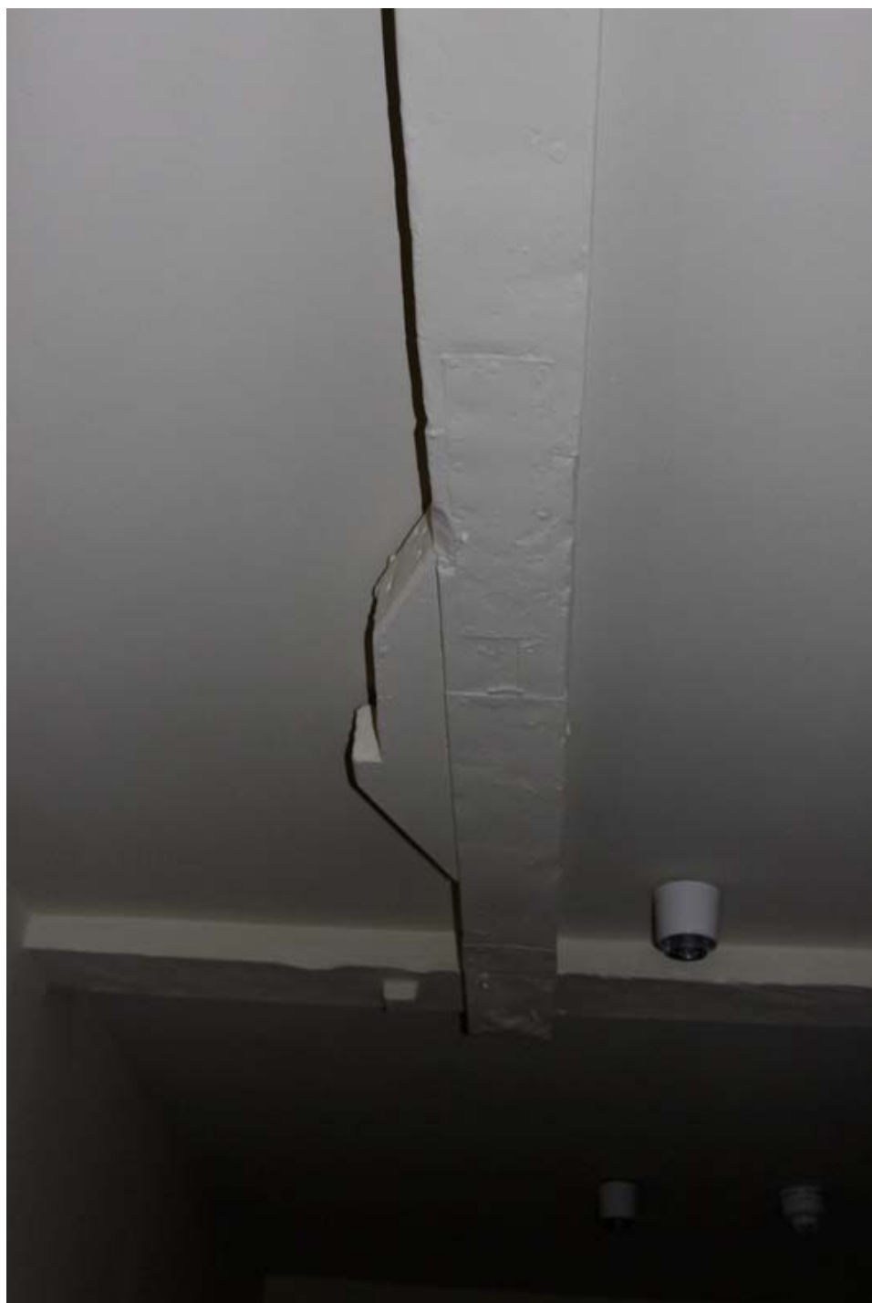
Plate 135: The roof beam the northern bay has a substantial trimmer that may relate to an external hoist, and a notched cleat on its eastern face
