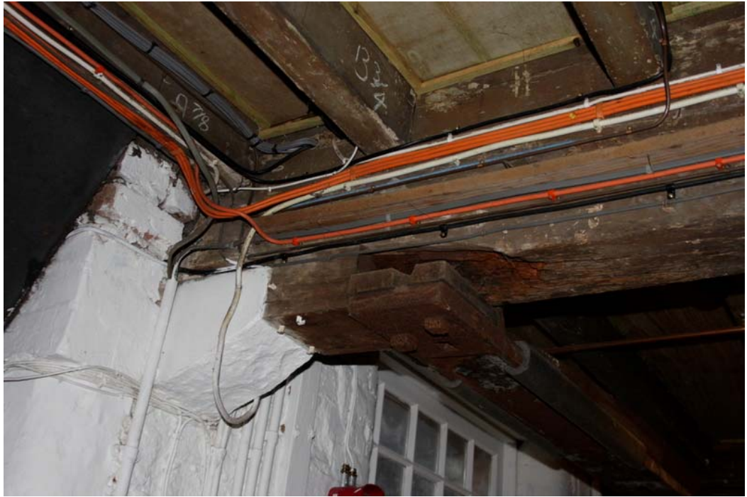
Plate 55: The convex sandstone corbel supporting the beam on the western side of the mill
