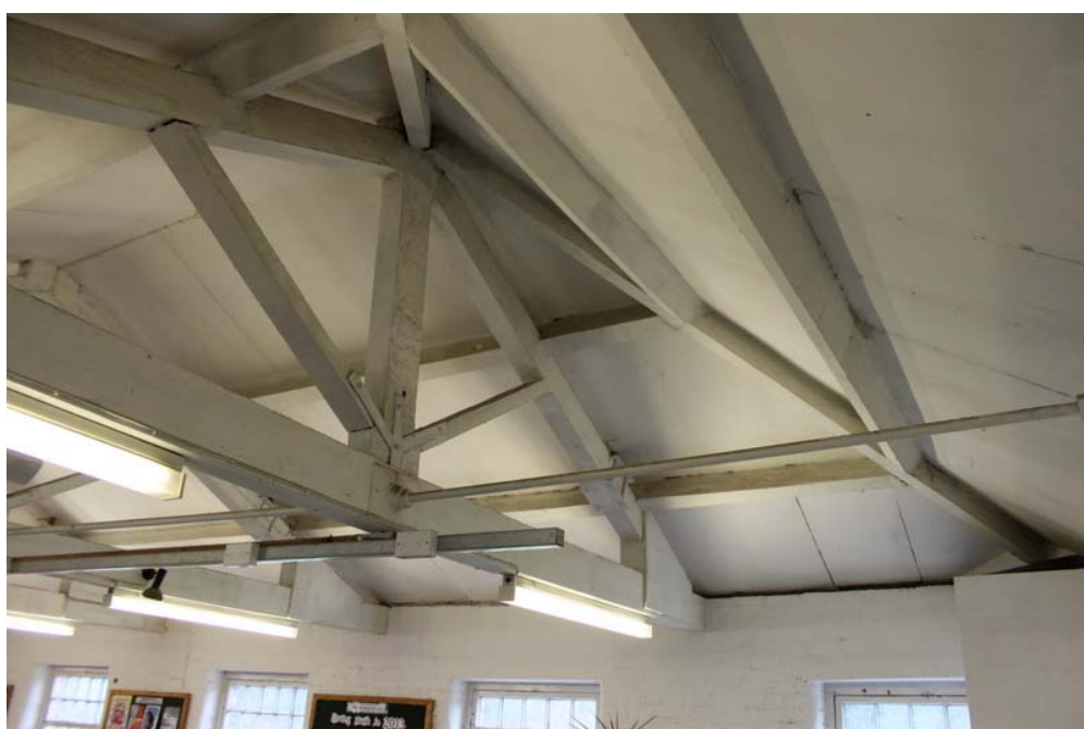
Plate 120: The king post trusses with bolted and bracketed joints and angled braces
