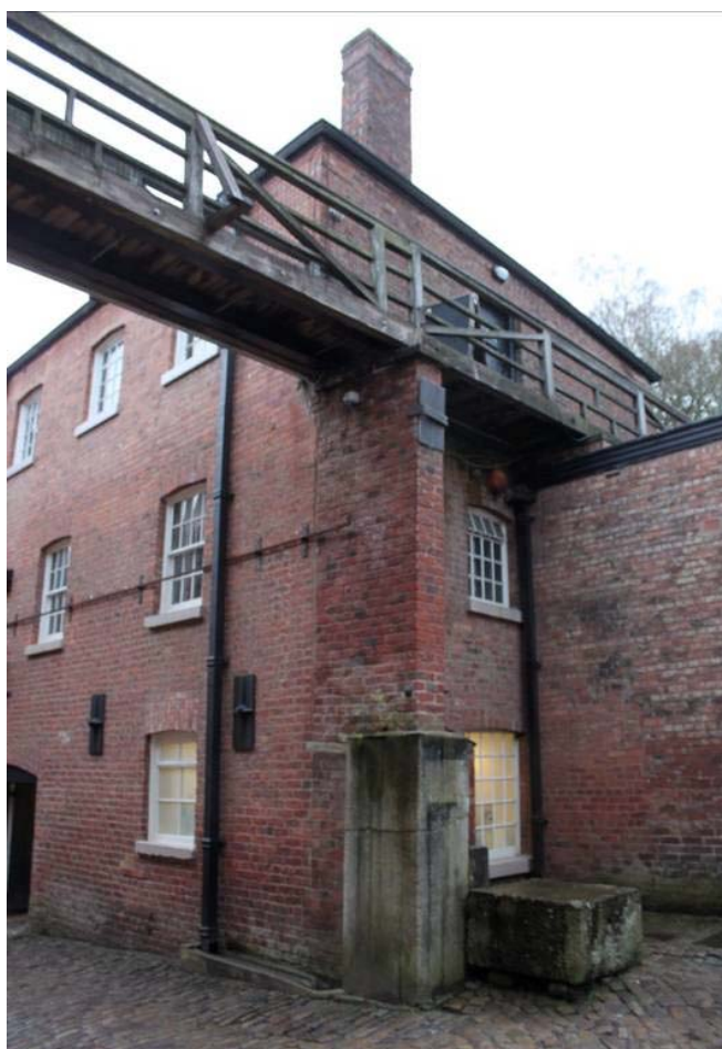
Plate 77: A short stub of wall extending south from the Greg Rooms supporting a pedestrian bridge
