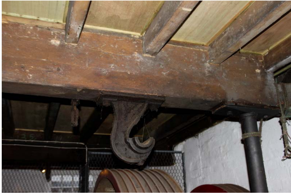
Plate 59: To the west of the upright shaft housing, a J-bracket carried a shaft towards the western wall
