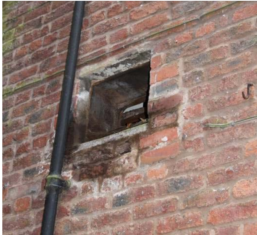
Plate 57: The bay to the west of the hoist tower has a bearing box placed in the external face of the north wall of the Greg Rooms
