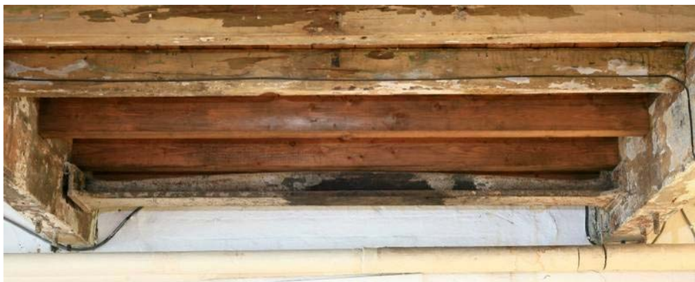
Plate 64: Between the timber beams is a cast iron, closed-web, T-section whale-backed beam across the central bay
