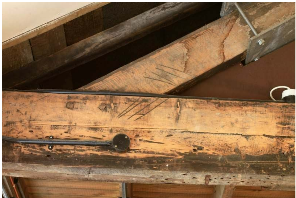
Plate 38: Scored assembly marks cut into southern faces of the trusses
