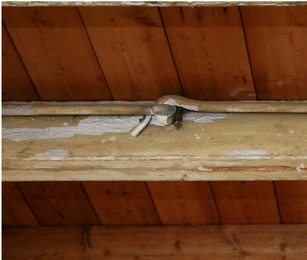
Plate 63: The join of two hooked tie-rods which span east/west across the building
