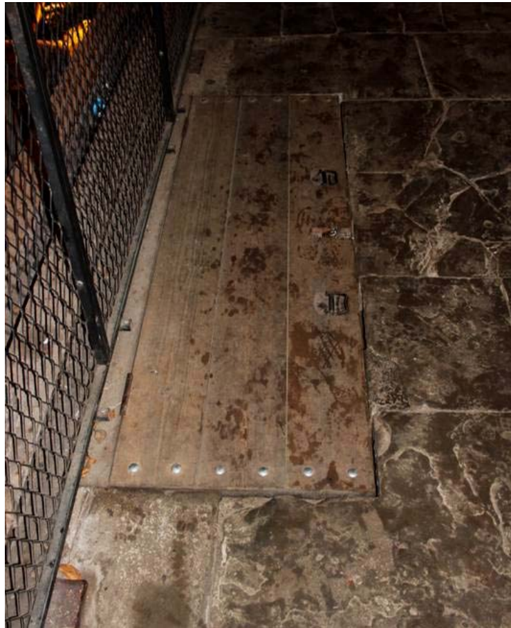
Plate 49: Access to the southern axle was via a timber trap door
