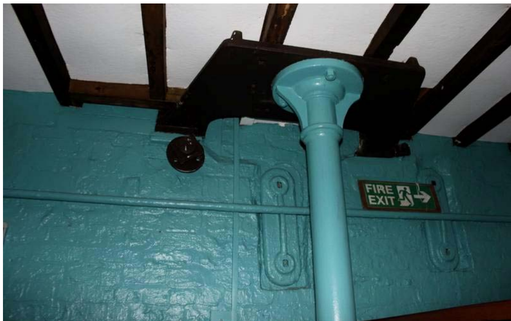
Plate 117: A cast-iron bearing supported by a cylindrical cast iron column
