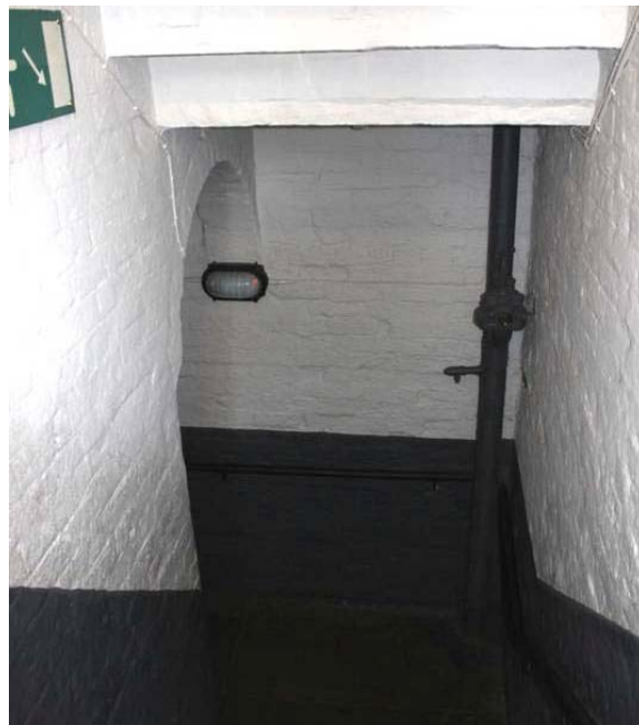
Plate 52: Within the north-western corner of the stair tower was a water pipe for fire-fighting
