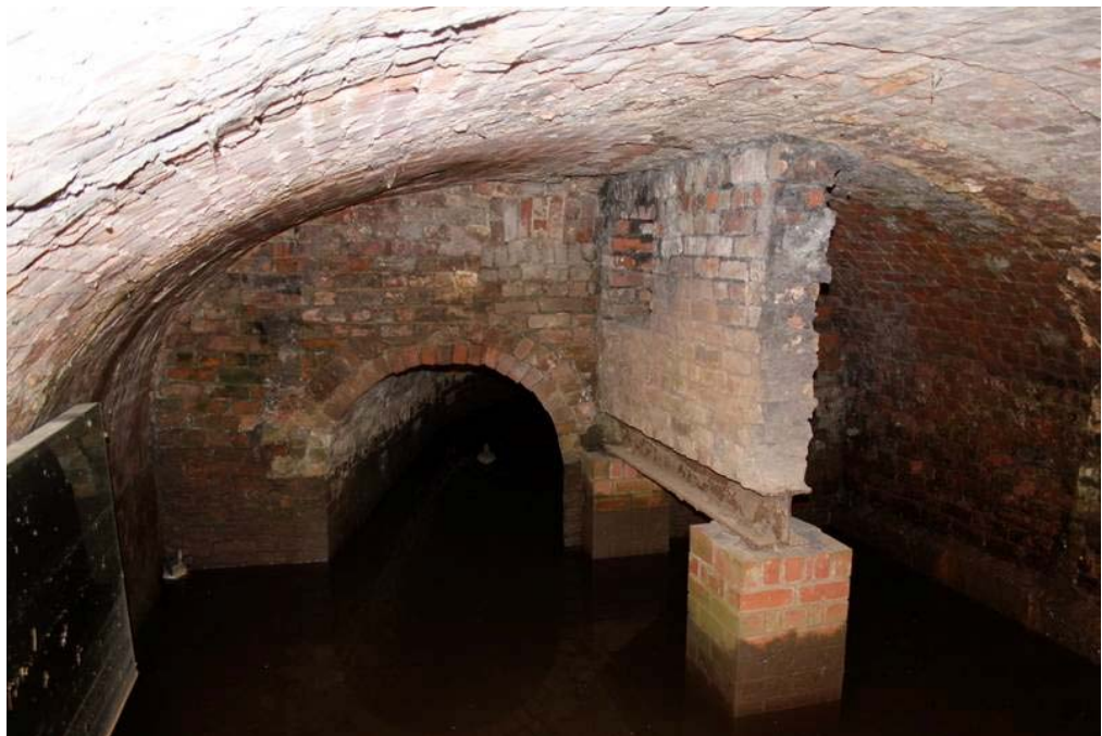
Plate 23: Extant narrower, lower culvert with longitudinal support wall
