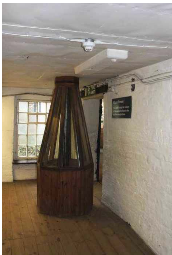
Plate 32: Bevelled timber mounting bracket in the southern bay aligned with the upright shaft
