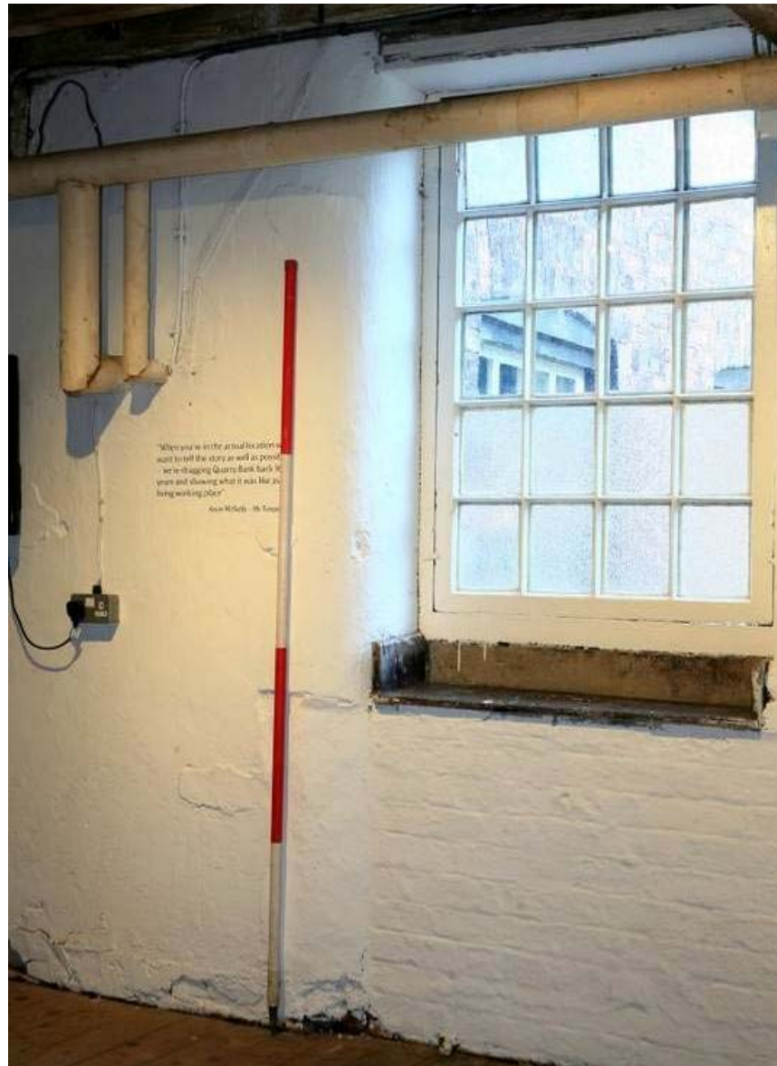
Plate 35: 20 light window frame sitting on chamfered stone blocks
