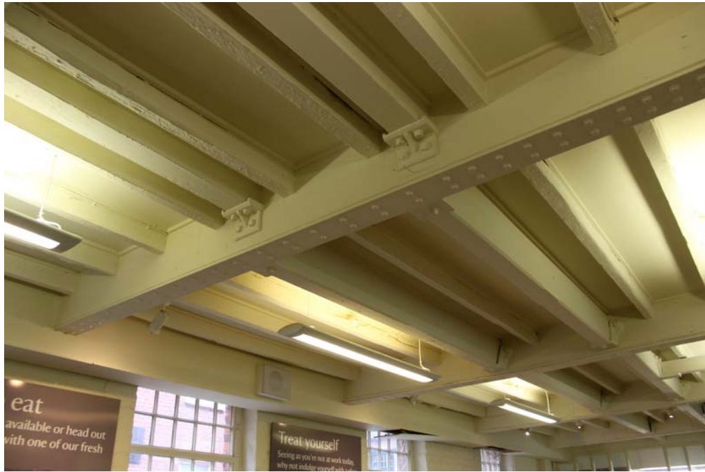
Plate 132: Two rows of trimmer joists, bolted to the face of the ceiling beams, ran the length of the building
