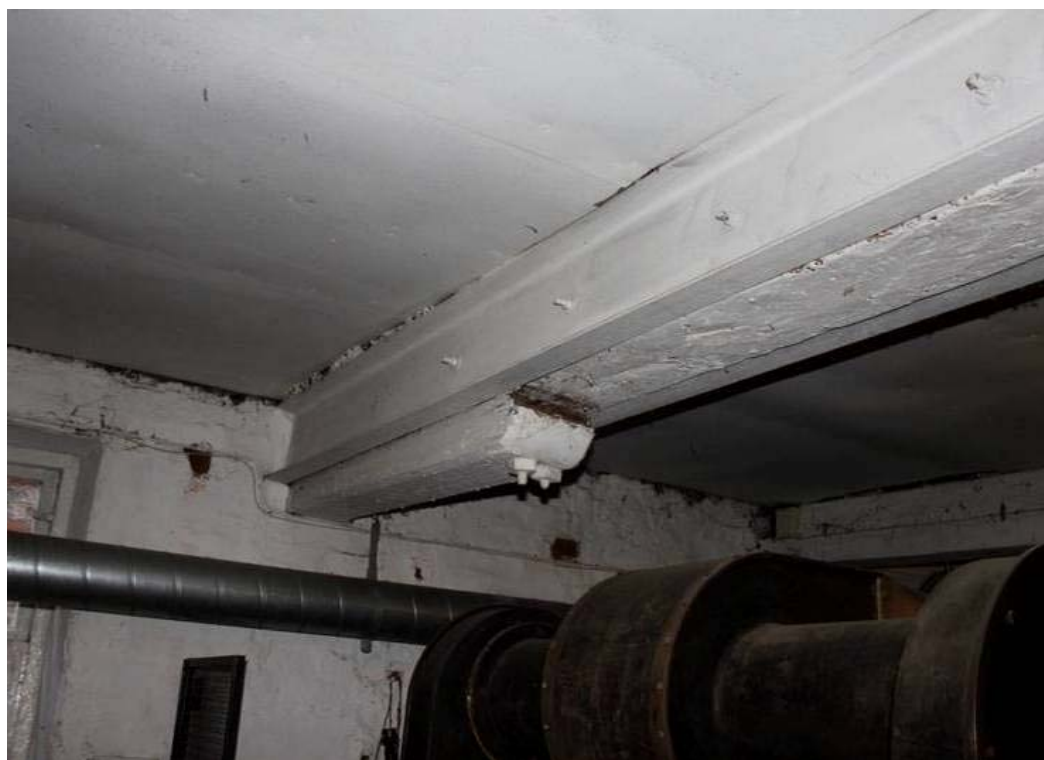
Plate 29: Late I-section steel flitch plates bracing the western part of the second beam
