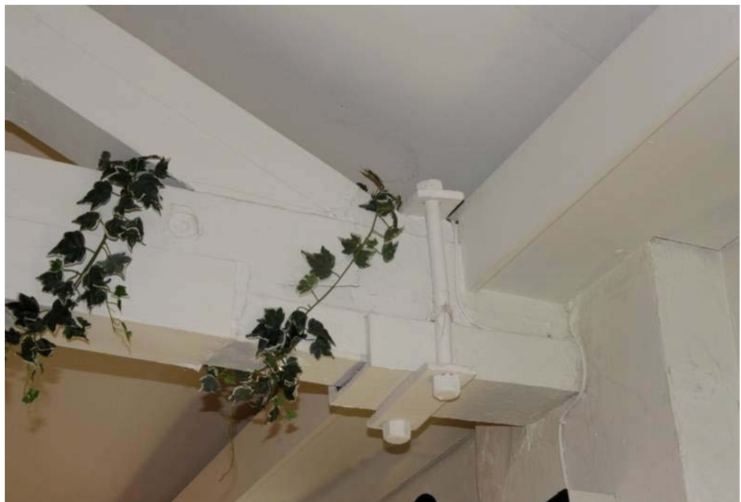
Plate 134: The fifth truss from the southern end has a timber strengthening corbel with steel brackets supporting its eastern end
