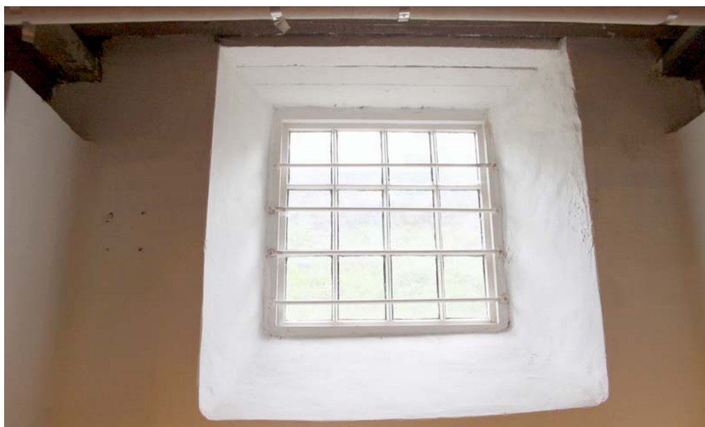
Plate 12: Fixed 12 light timber windows
