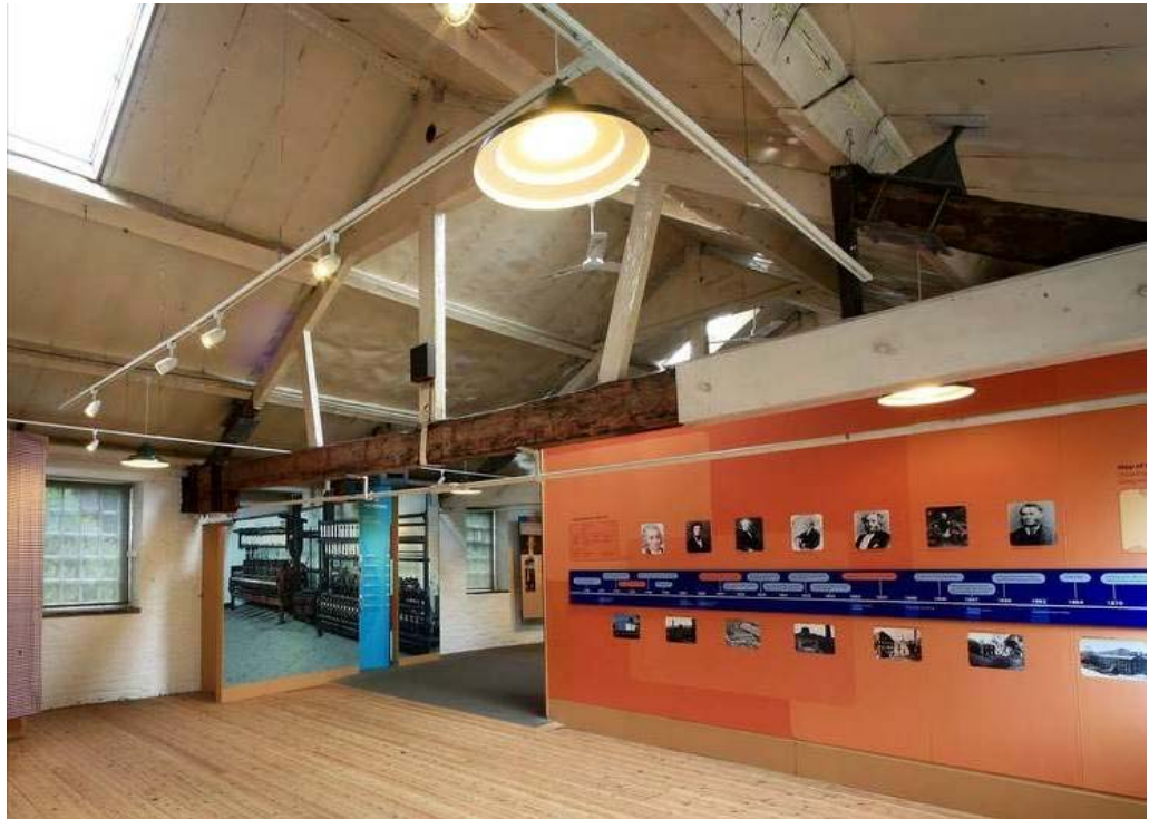
Plate 37: King post trusses in the early part of the mill
