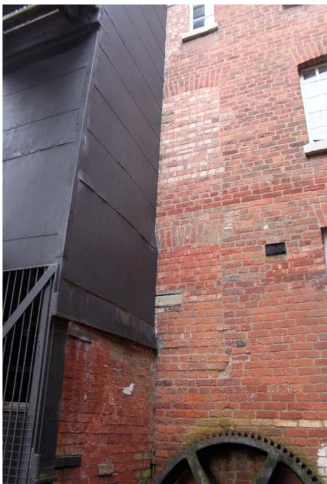
Plate 60: A window in the south wall was brick-blocked during the insertion of the wider hoist tower
