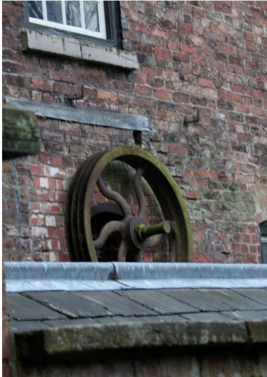
Plate 34: Spoked rope wheel on the exterior of the northern wall
