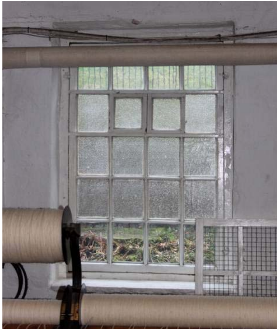
Plate 26: 20-light window frames
