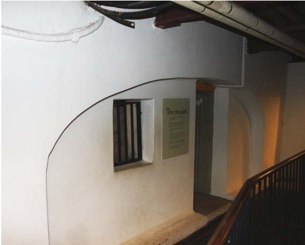
Plate 17: Basket arch rebated into the wall thickness
