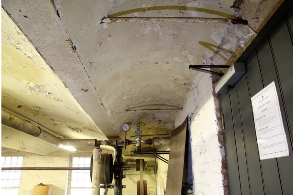
Plate 112: Six cylindrical wrought-iron tie rods span the narrower vaults
