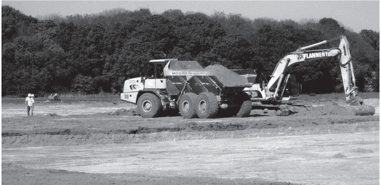
Plate 1 Stripping topsoil from Area 8
