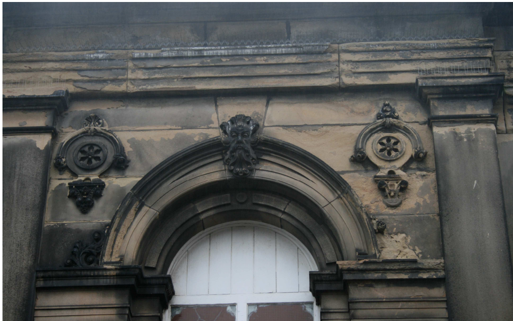
Plate 20: Detail of the head on one of the elaborate windows
