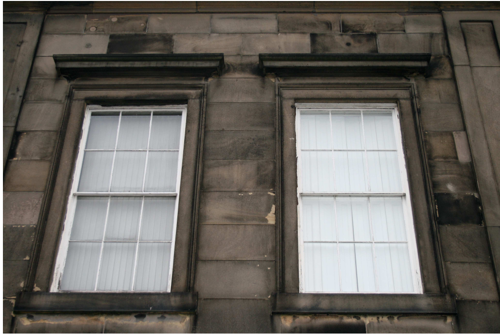
Plate 19: Detail of the taller sash windows on the original phase of the building
