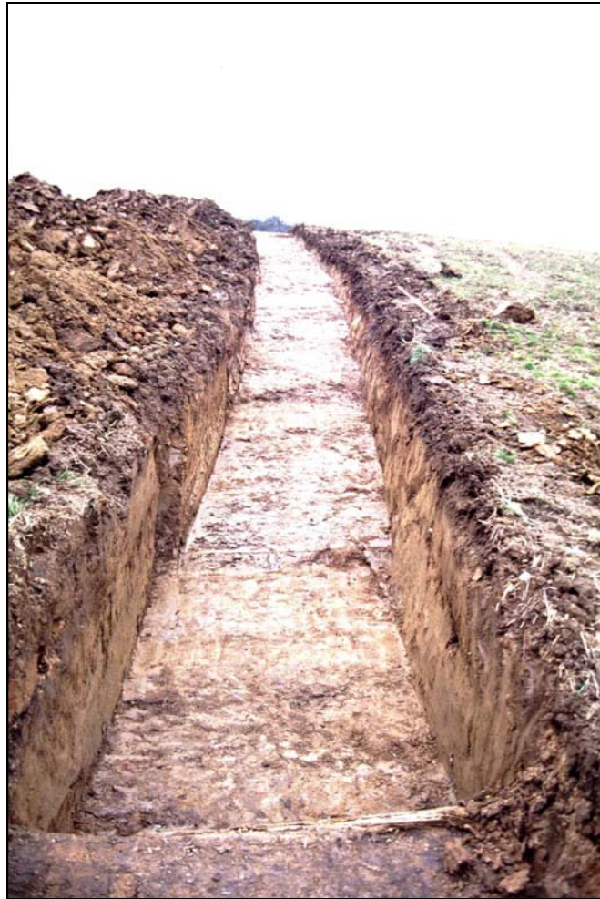
Plate 1: North-east end of Trench 1, showing subsoil depth
